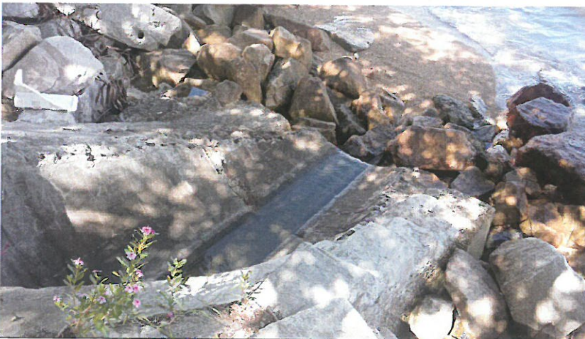
Outfall 1: Clean water is discharging.
