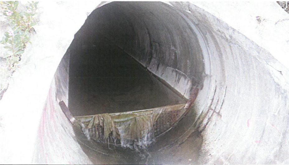
Outfall 1: Clean water is discharging.
