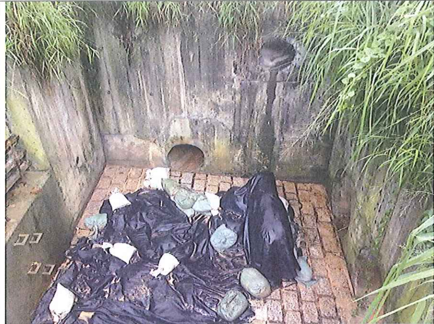
Stream B Outfall: No water is discharging.
