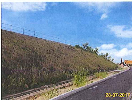
Item 4. Hydro-seeding or sheeting provided at stockpile.
