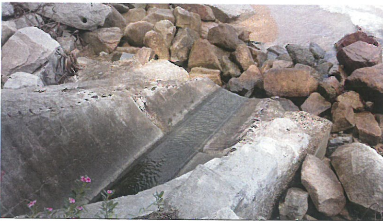
Outfall 1: Clean water is discharging.
