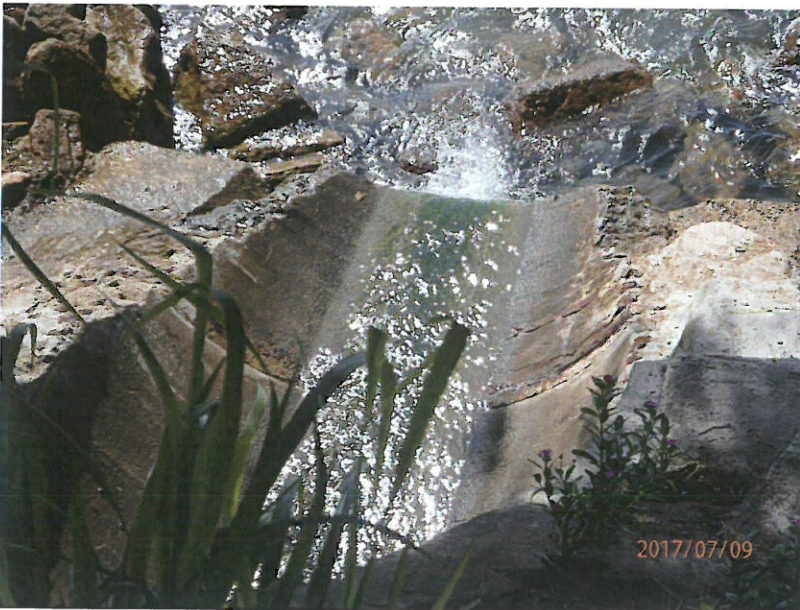
Outfall 1: Clean water is discharging.
