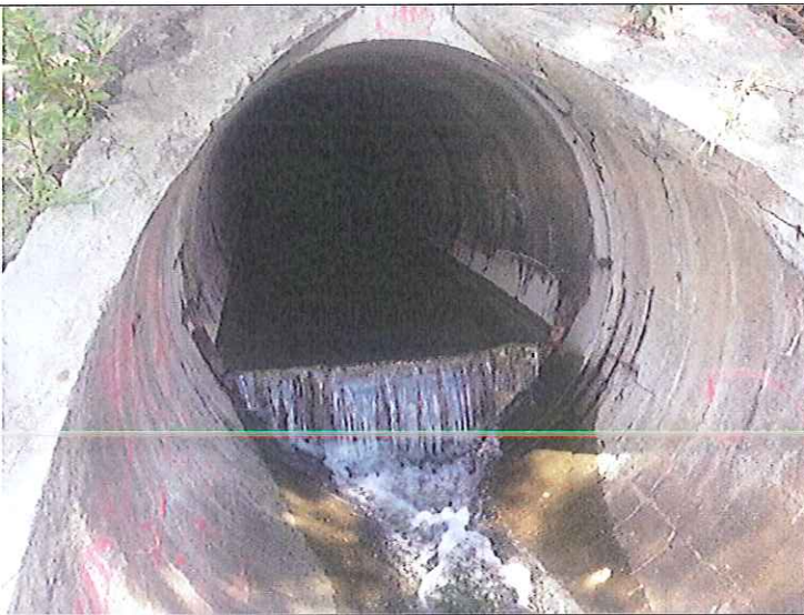
Outfall 1: Clean water is discharging.
