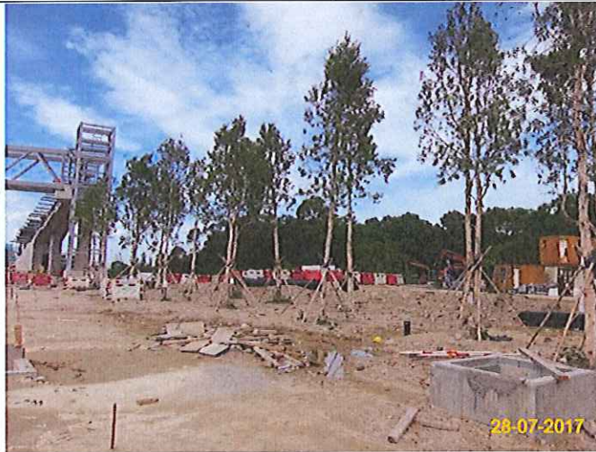
Item 2. Tree Transplanting works conducted on 22-May-17.
