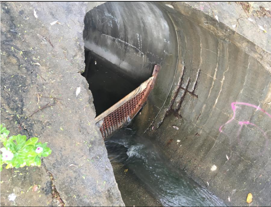
Outfall 1: Clean water is discharging.
