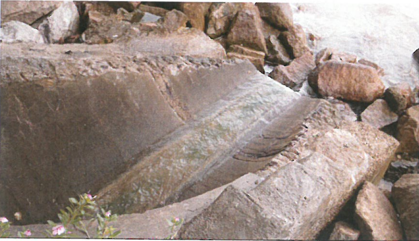
Outfall 1: Clean water is discharging.
