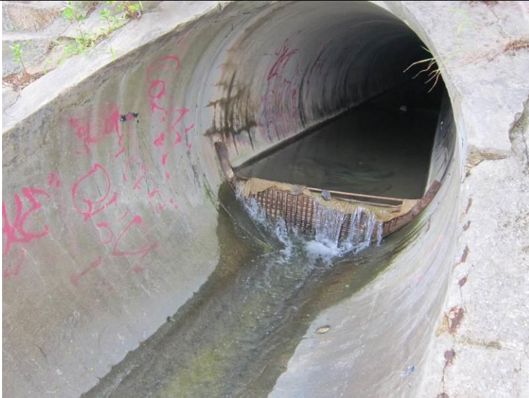
Outfall 1: Clean water is discharging.
