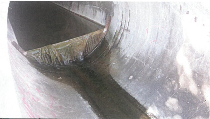
Outfall 1: Clean water is discharging.
