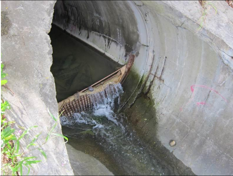
Outfall 1: Clean water is discharging.
