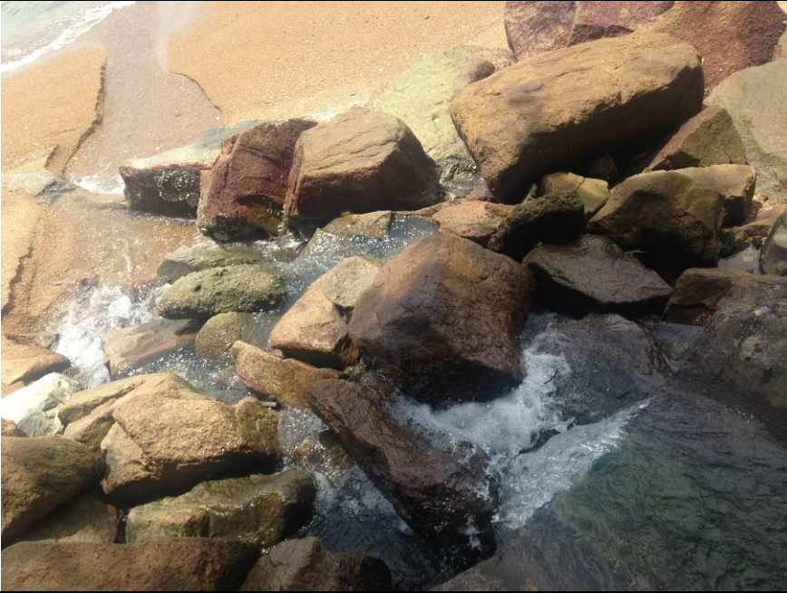
Outfall 1: Clean water is discharging.
