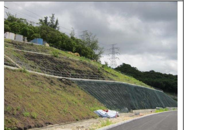
Photo 6 Covered part of the exposed slopes by geotextile net.
