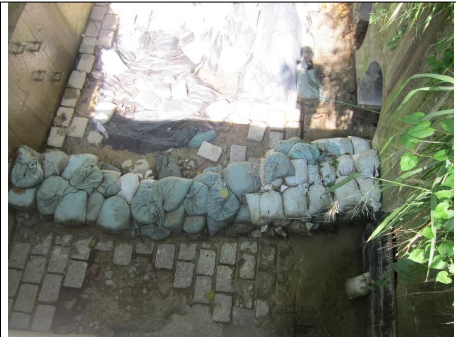
Stream B Outfall: Clean water is discharging.
