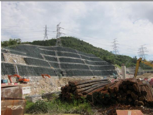
Photo 5 Covered part of the exposed slopes by geotextile net.
