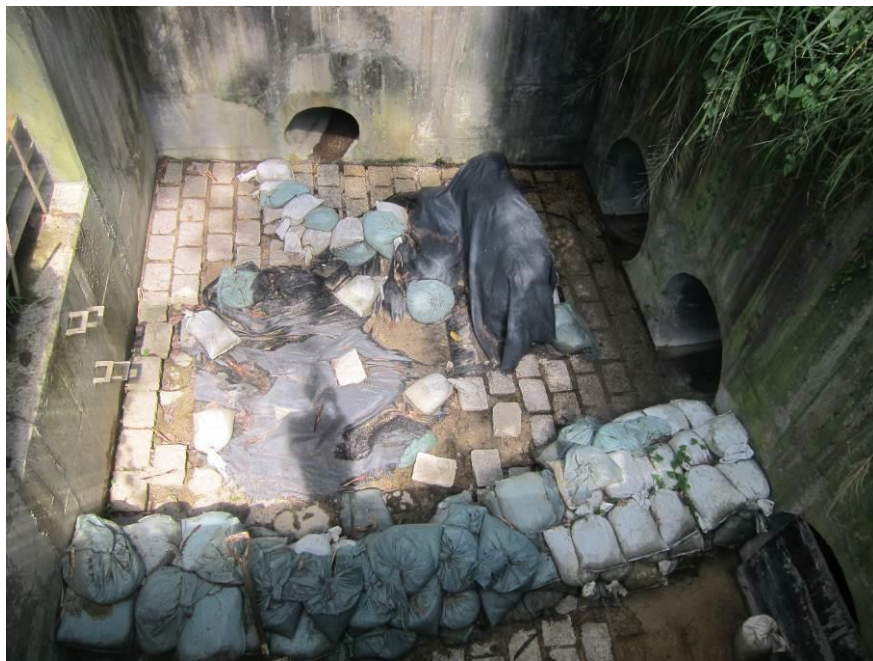
Stream B Outfall: No water is discharging.
