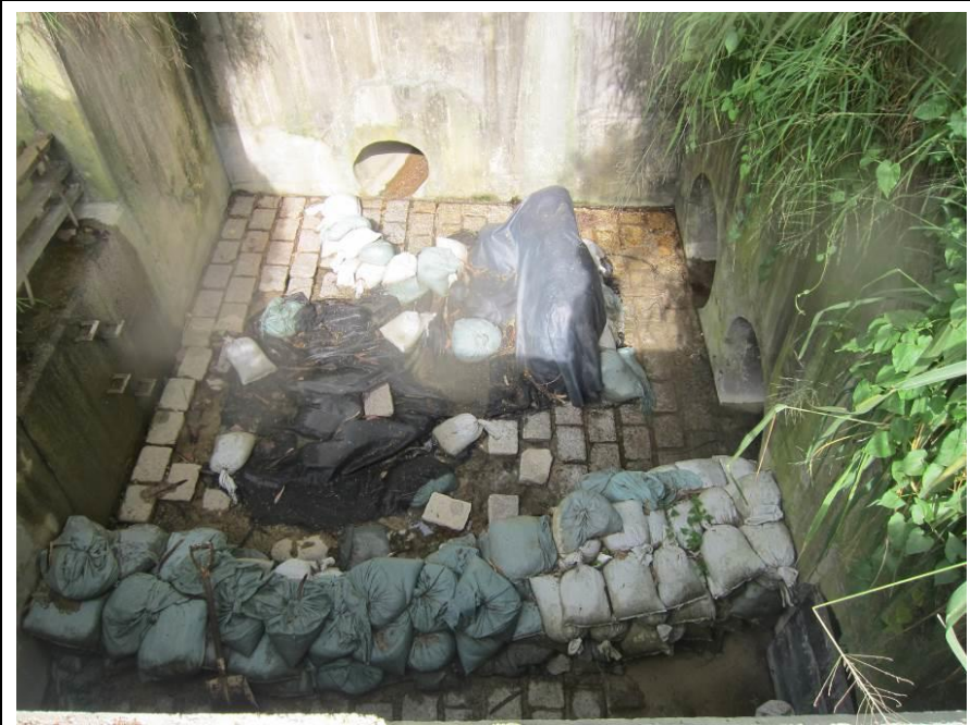
Stream B Outfall: No water is discharging.
