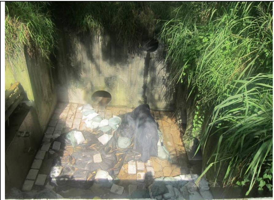
Stream B Outfall: No water is discharging.
