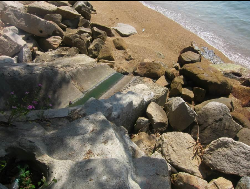
Outfall 1: Clean water is discharging.
