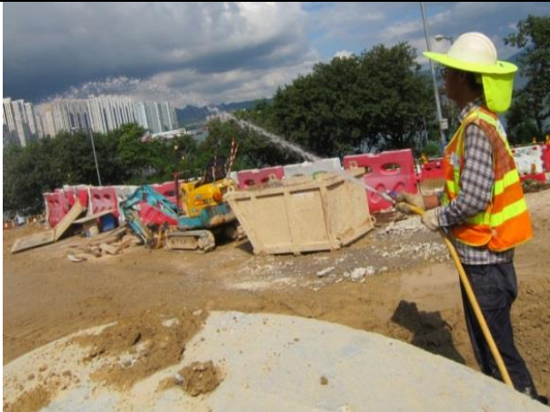
Photo 3 Water spraying by worker for un-accessible area.
