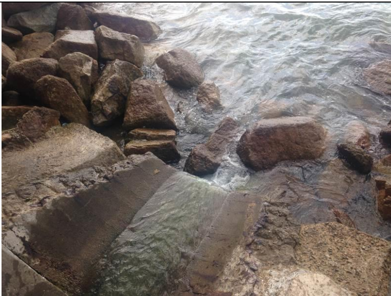
Outfall 1: Clean water is discharging.
