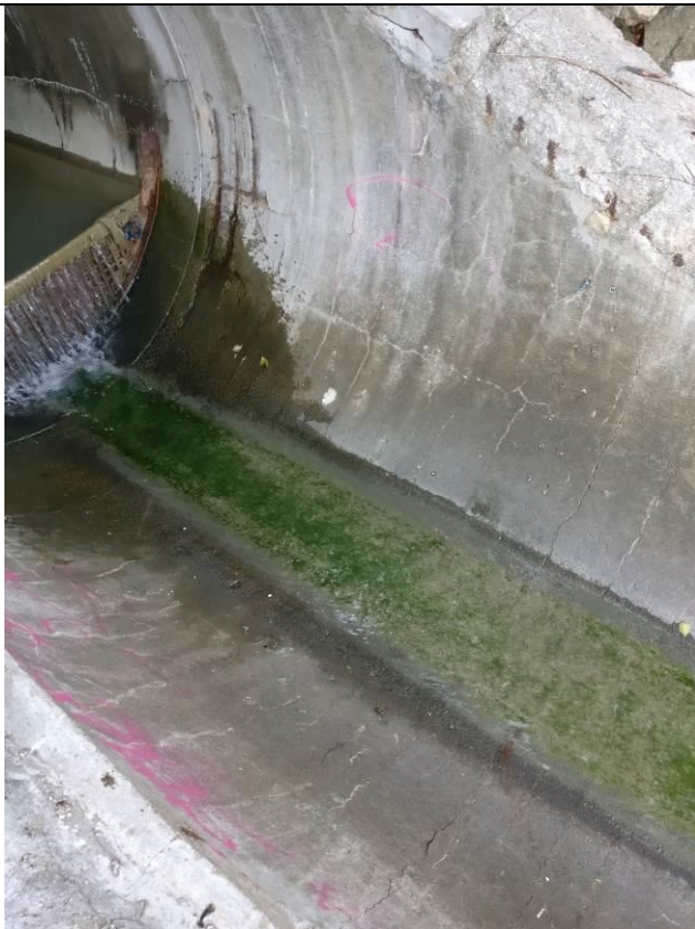
Outfall 1: Clean water is discharging.
