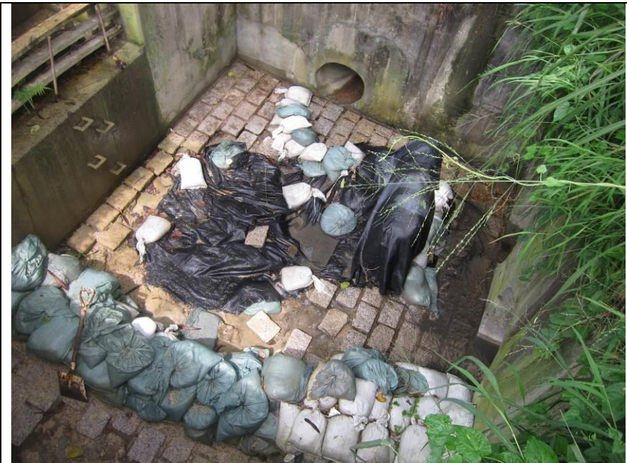
Stream B Outfall: No water is discharging.
