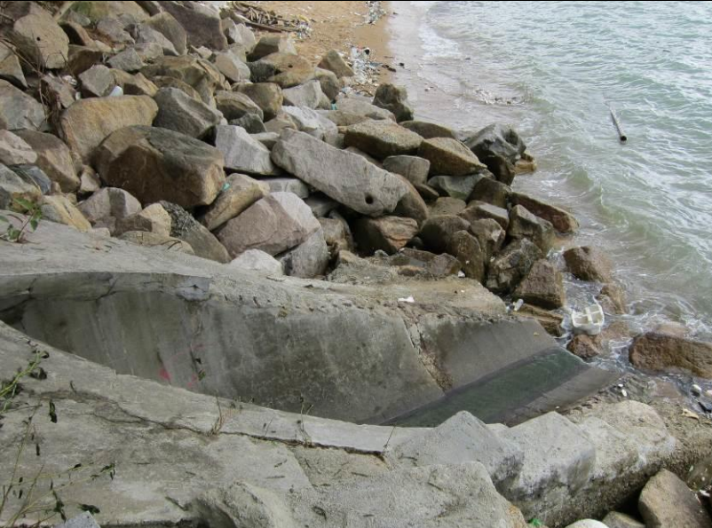
Outfall 1: Clean water is discharging.
