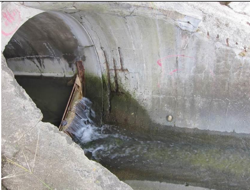
Outfall 1: Clean water is discharging.
