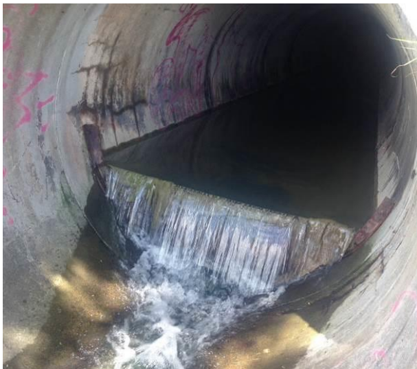
Outfall 1: Clean water is discharging.
