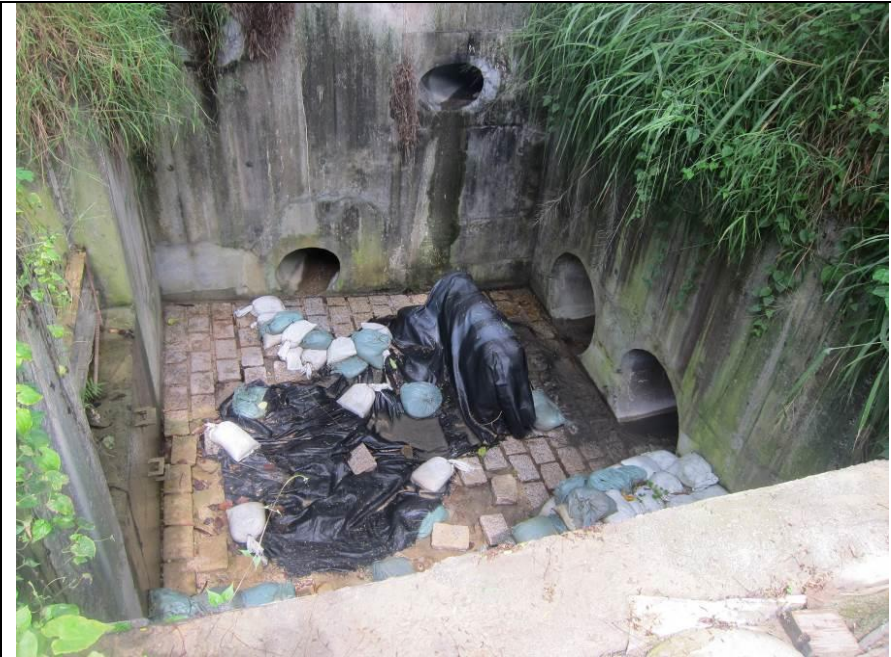
Stream B Outfall: No water is discharging.
