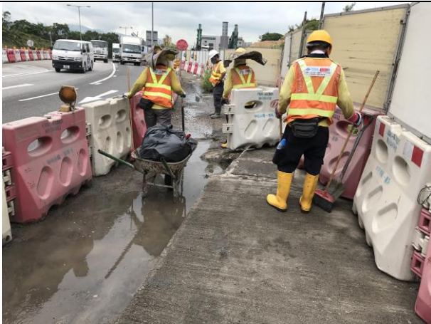
Photo 11 Housekeeping works near Lung Mun Road on 29 July 2017
