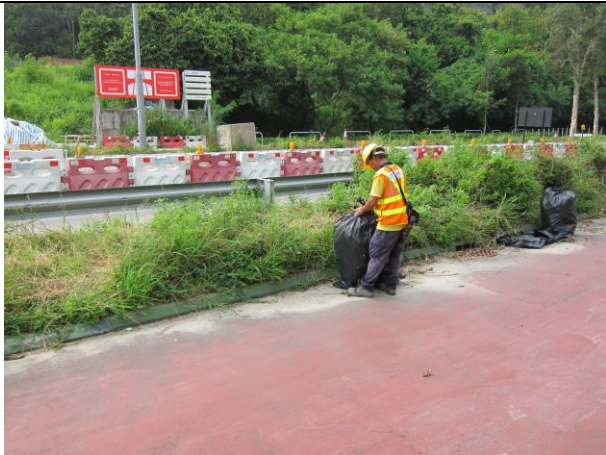
Photo 9 Removal of weed at works area near Butterfly Beach on 29 July 2017
