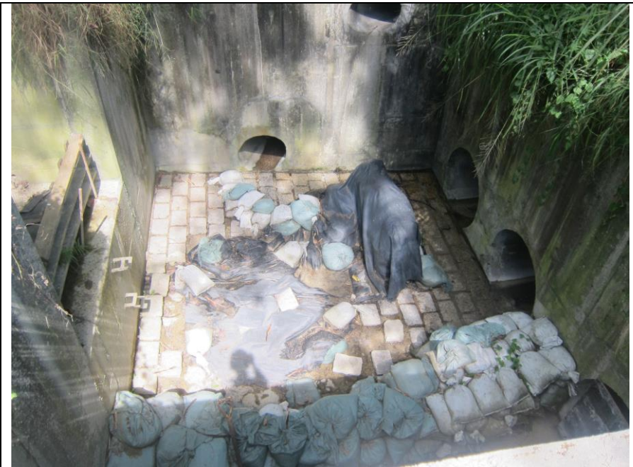
Stream B Outfall: No water is discharging.
