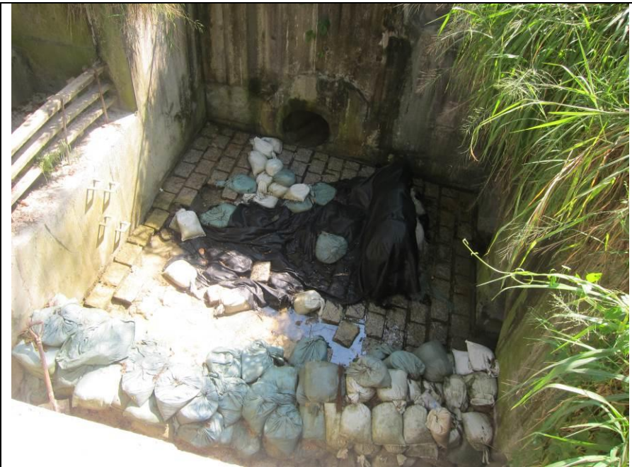
Stream B Outfall: Clean water is discharging.
