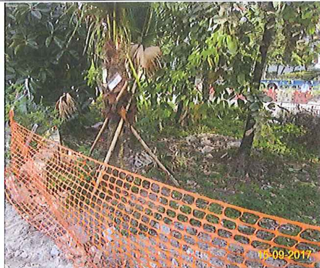
Item 1. Existing trees on boundary of the Project Area should be protected carefully during construction.
