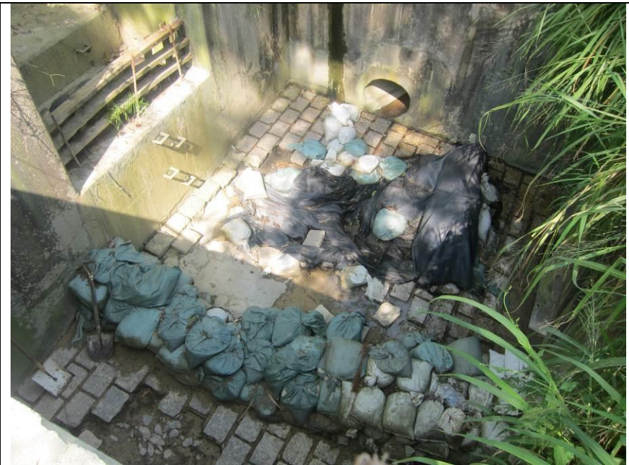
Stream B Outfall: No water is discharging.
