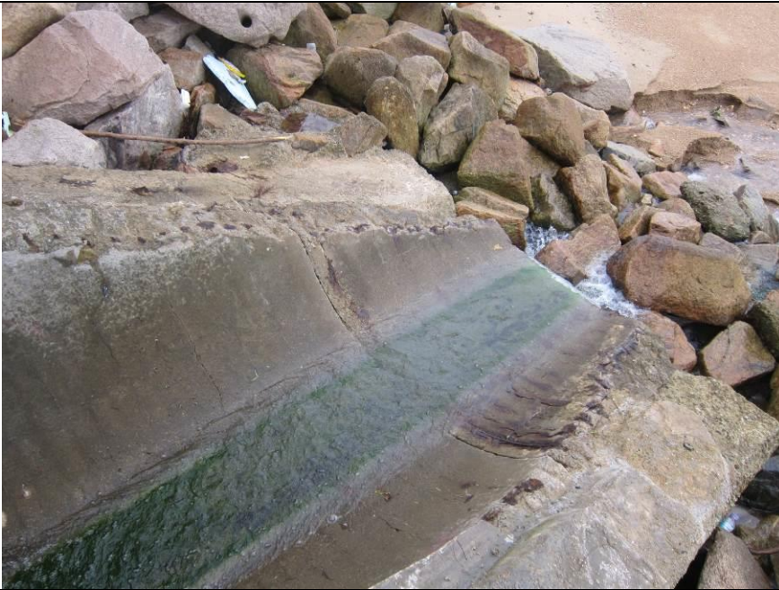
Outfall 1: Clean water is discharging.
