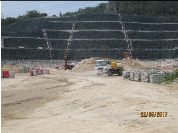
Photo 7 Watering of haul road by water truck to keep road surface wet was observed during the site inspection on 22 August 2017
