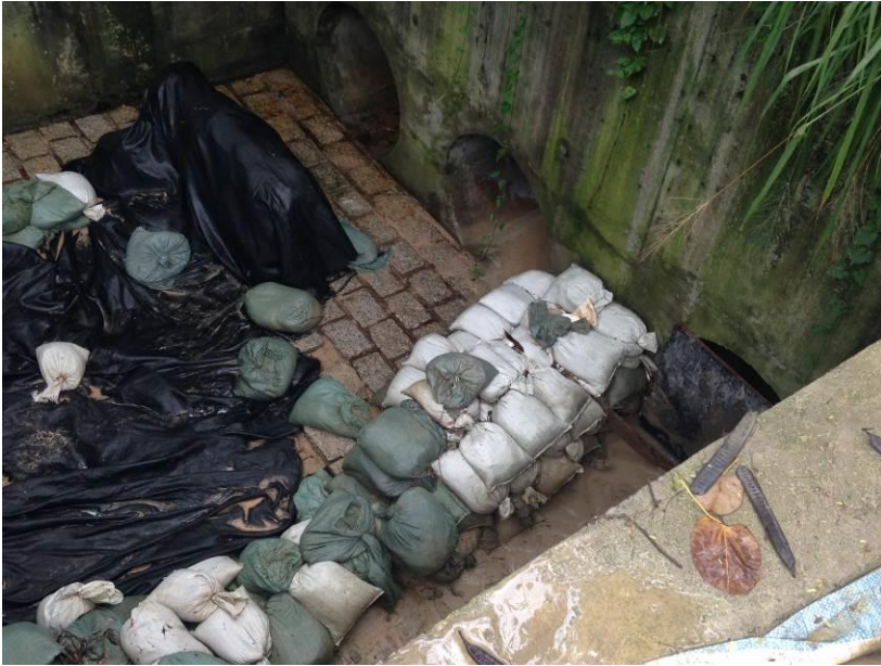
Stream B Outfall: No water is discharging.
