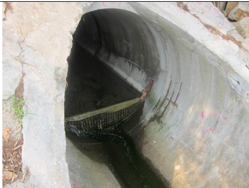
Outfall 1: Clean water is discharging.
