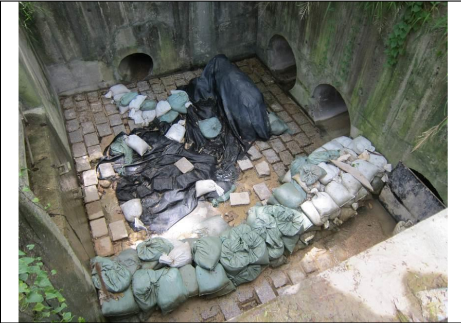
Stream B Outfall: Clean water is discharging.
