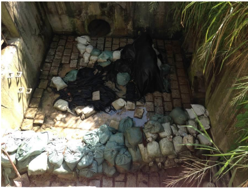
Stream B Outfall: No water is discharging.
