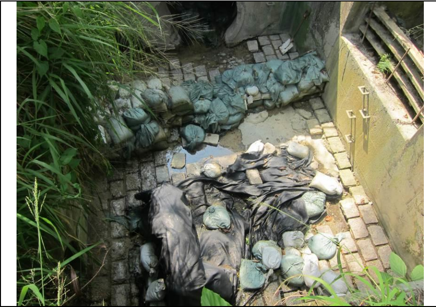
Stream B Outfall: No water is discharging.
