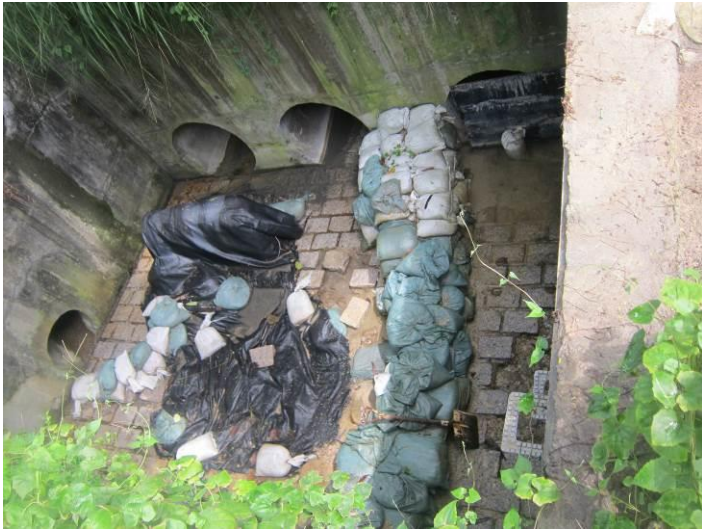
Stream B Outfall: Clean water is discharging.
