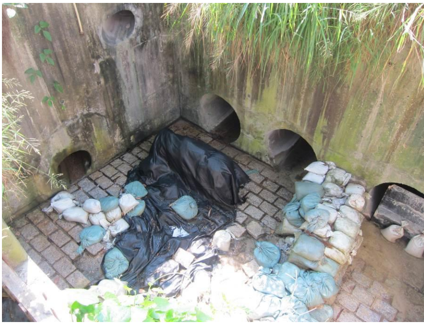
Stream B Outfall: No water is discharging.
