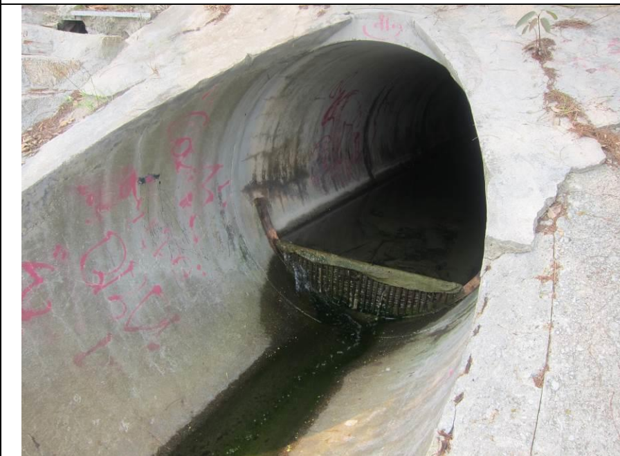
Outfall 1: No water is discharging.
