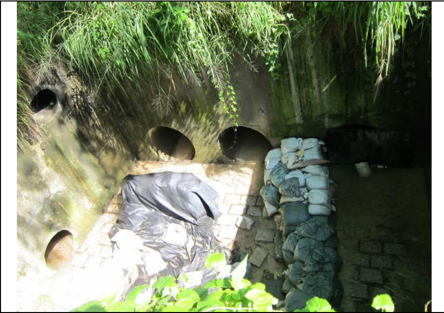
Stream B Outfall: No water is discharging.
