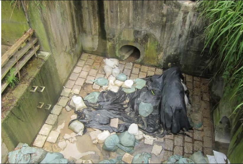
Stream B Outfall: Clean water is discharging.
