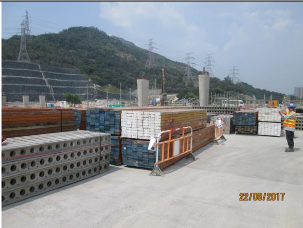
Photo 9 Typhoon precaution works on 22 August 2017.
