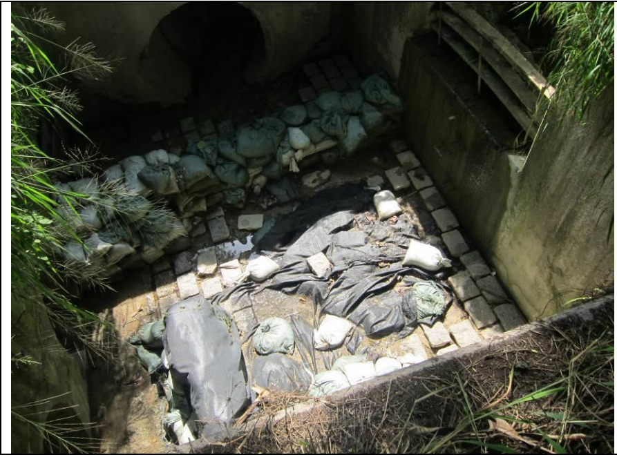
Stream B Outfall: No water is discharging.
