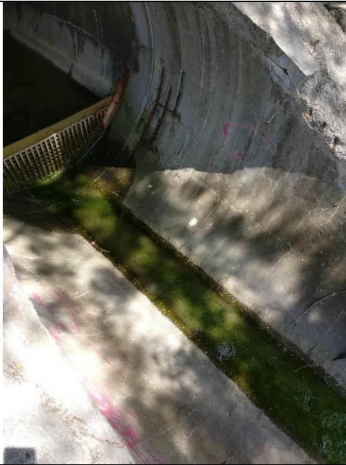
Outfall 1: No water is discharging.
