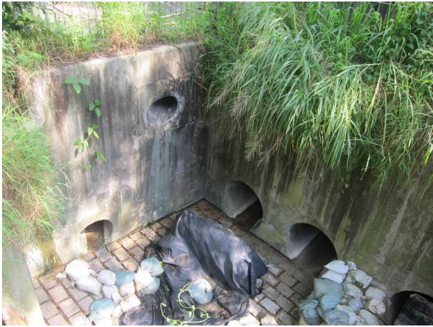
Stream B Outfall: No water is discharging.
