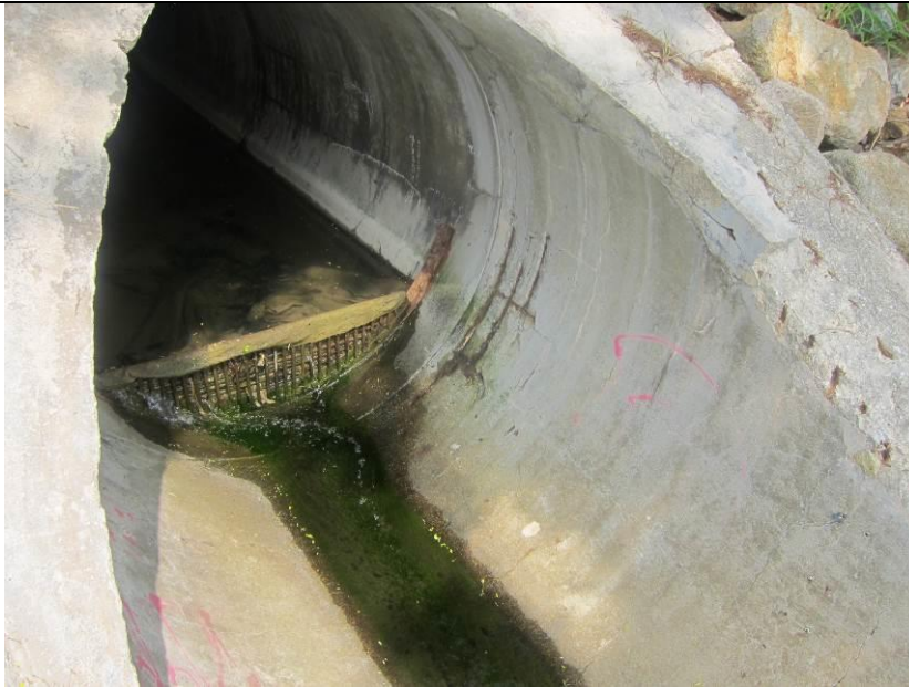
Outfall 1: Clean water is discharging.
