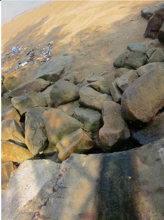
Outfall 1: No water is discharging.
