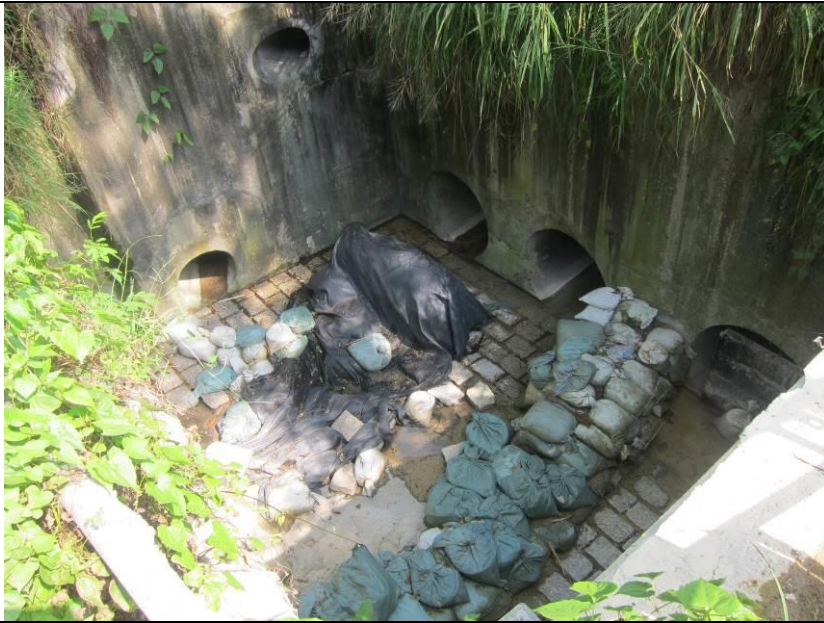
Stream B Outfall: Clean water is discharging.
