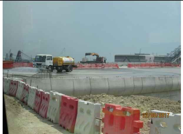
Photo 8 Watering of haul road by water truck to keep road surface wet was observed during the site inspection on 22 August 2017
