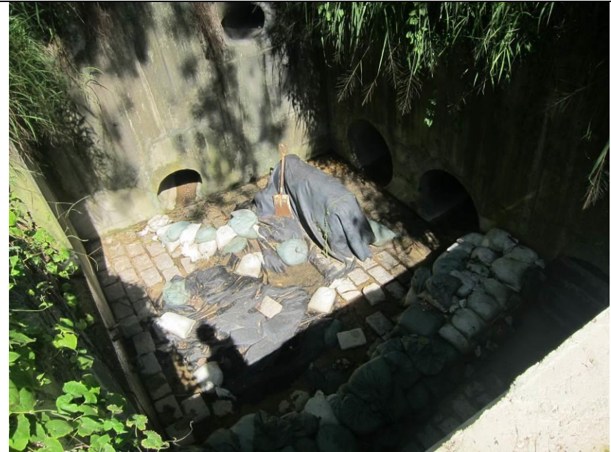
Stream B Outfall: No water is discharging.
