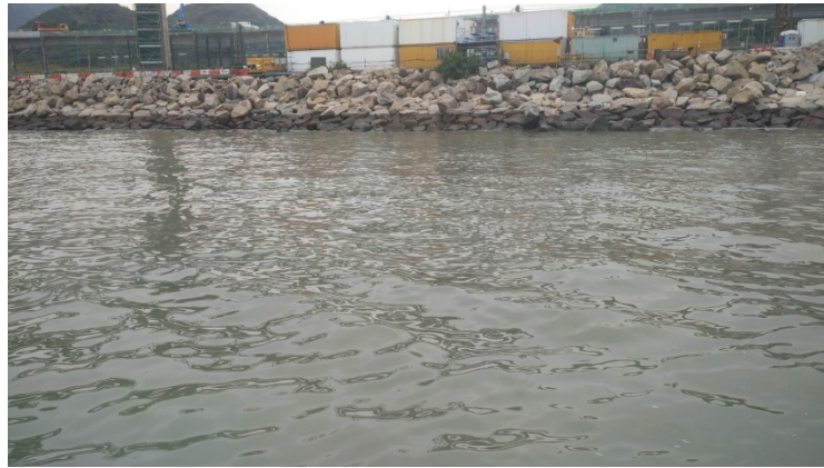
Photo 1 - Mid-Flood at SR4 on 8 November 2017
