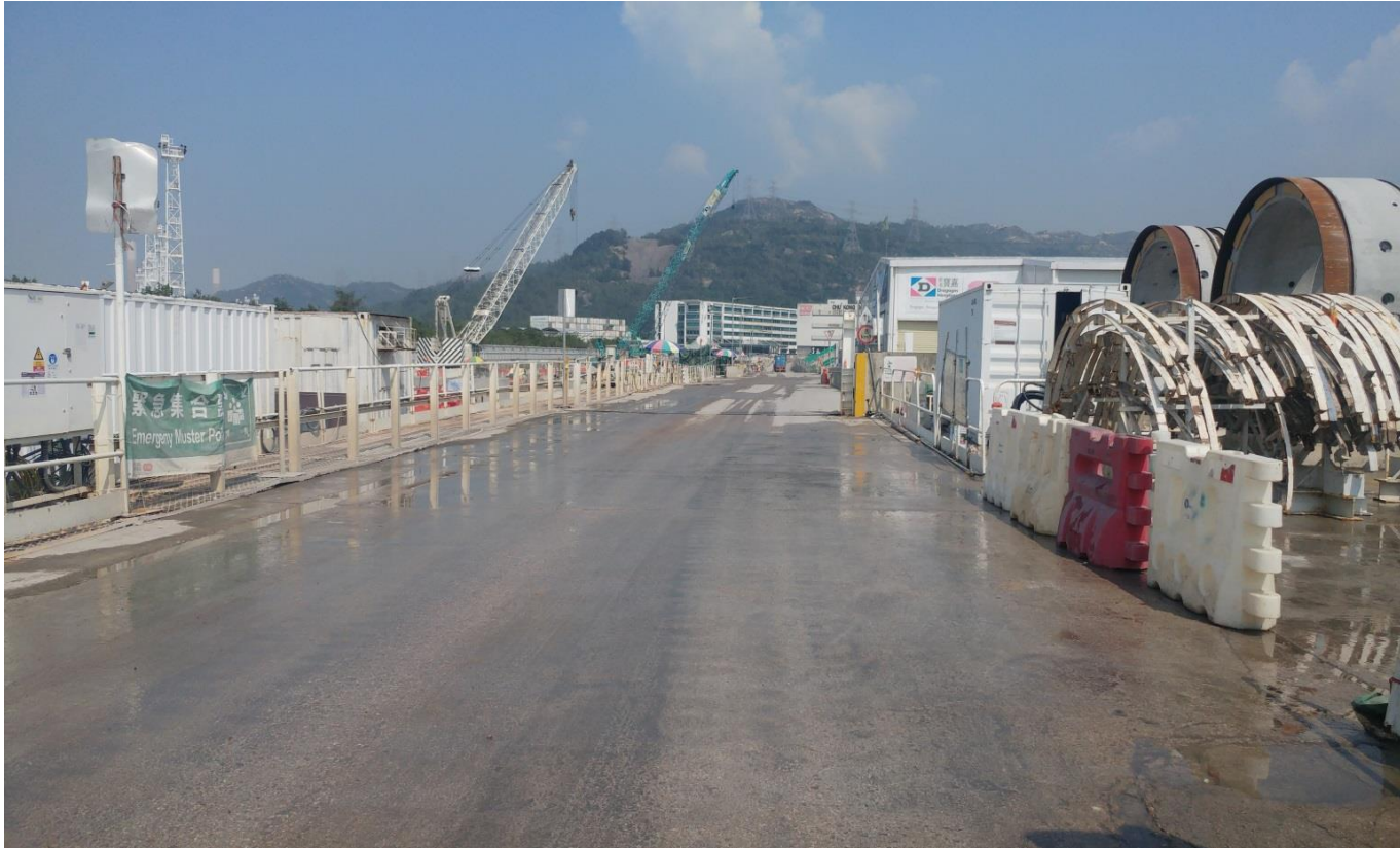
Water spraying was applied frequently during dry conditions.(Works Area Portion N-B)
