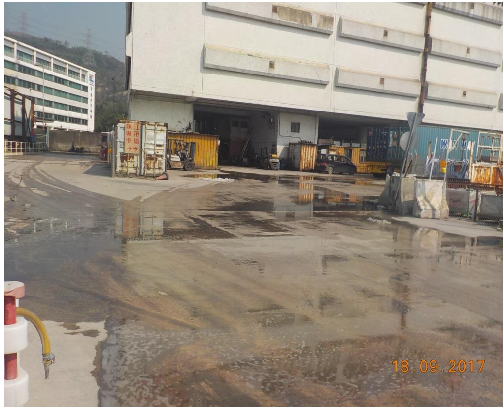
Water spraying was applied frequently during dry conditions. (Works Area Portion N-A)
