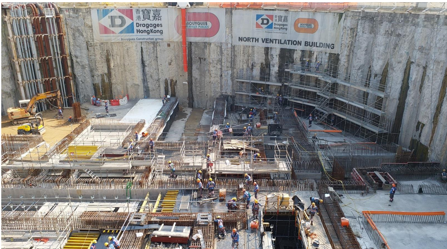
Construction of Ventilation Building. (Works Area Portion N-C)
