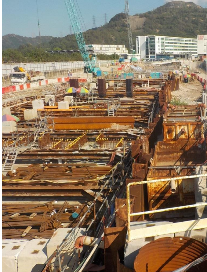
Box Culvert Extension. (Works Area Portion N-A)
