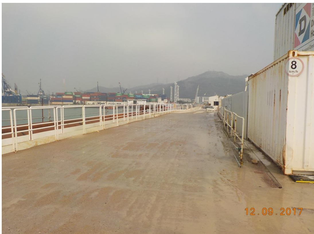
No dust nuisance was observed. (Works Area Portion N-B)
