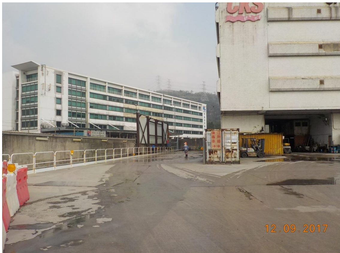
Water spraying was applied frequently during dry conditions. (Works Area Portion N-A)
