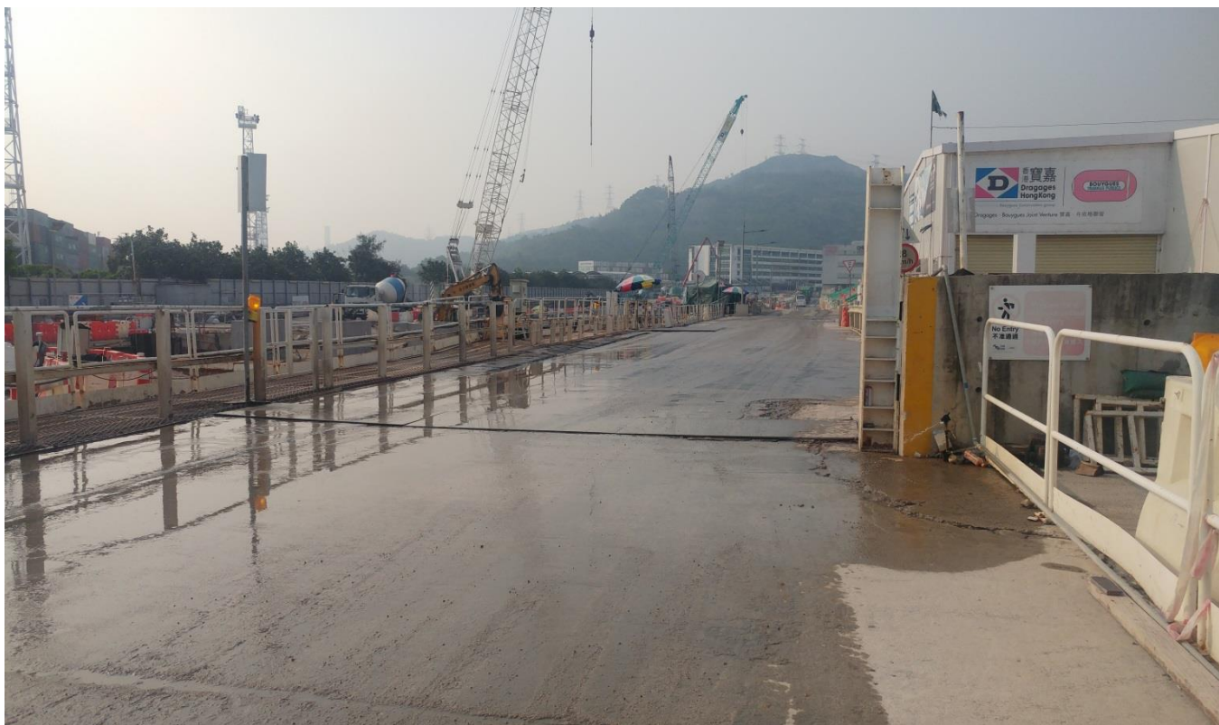
No dust nuisance was observed. (Works Area Portion N-A)
