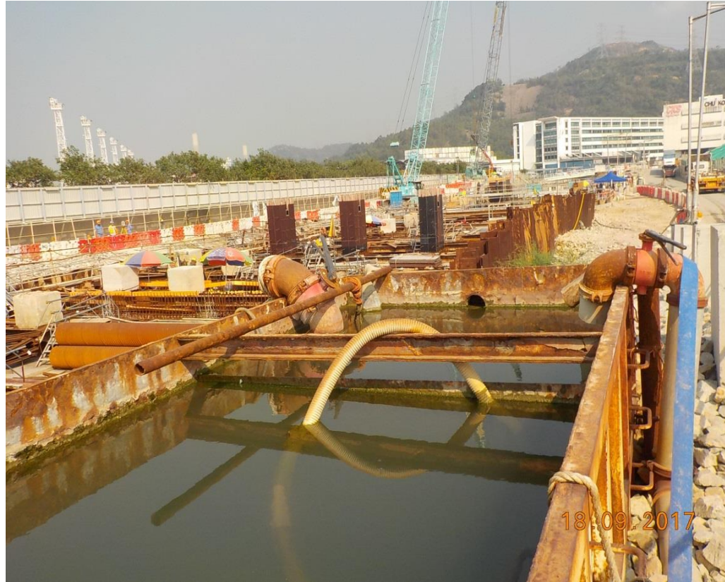
Box Culvert Extension. (Works Area Portion N-A)
