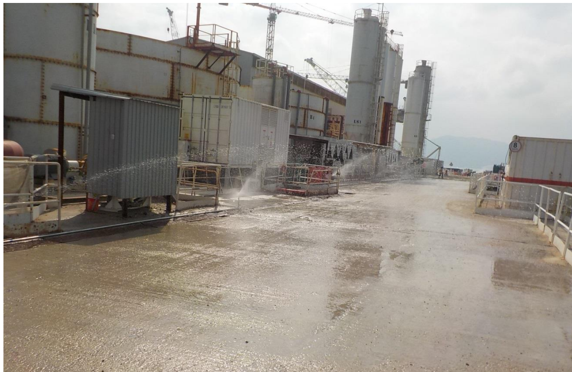
Use of sprinklers for water spraying,. (Works Area Portion N-C)
