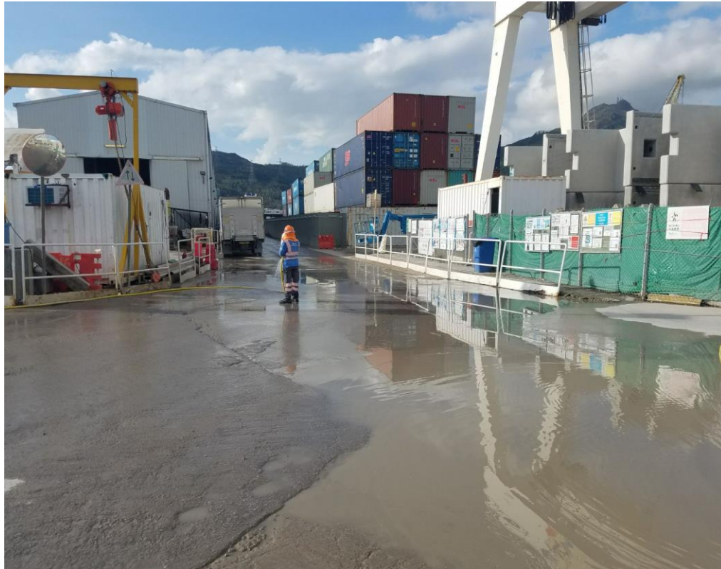
Water spraying was applied frequently during dry conditions.(Works Area Portion N-B)
