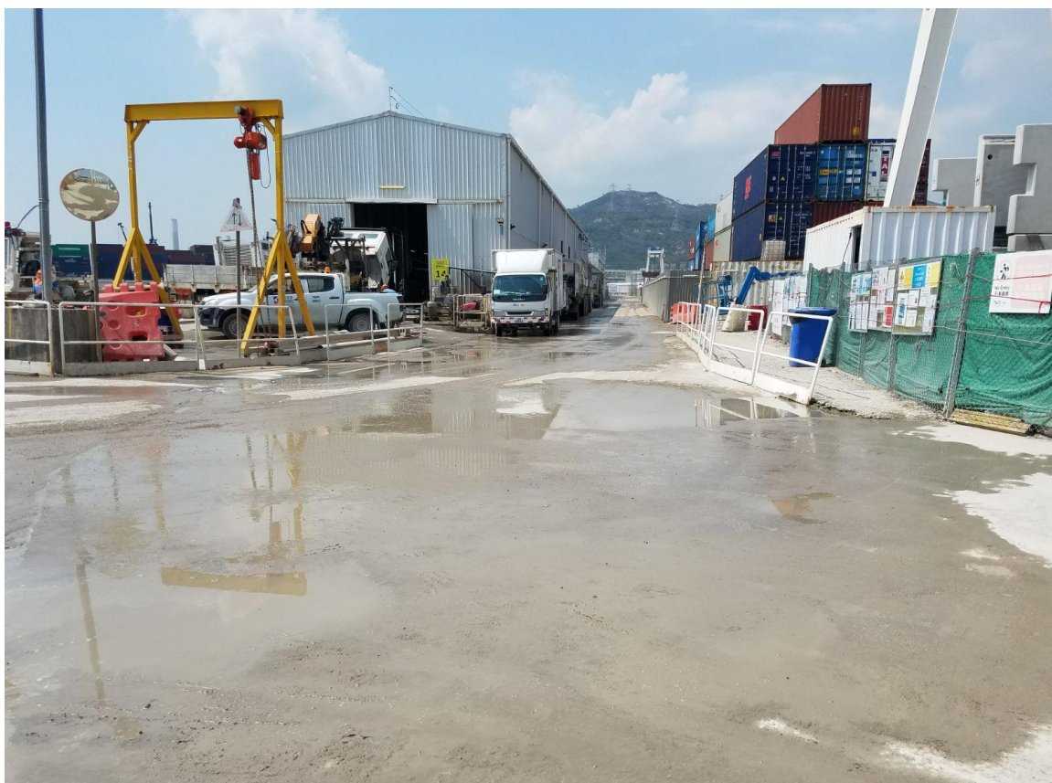
Water spraying was applied frequently during dry conditions.(Works Area Portion N-B)
