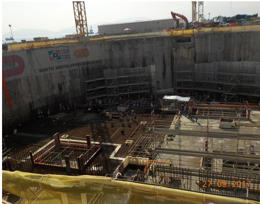
Construction of Ventilation Building. (Works Area Portion N-C)
