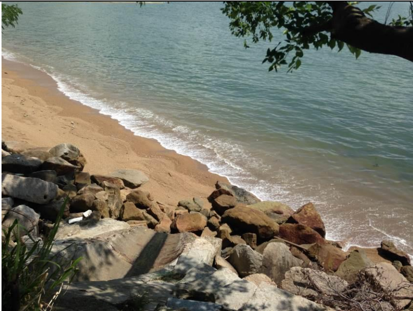
Outfall 1: Clean water is discharging.
