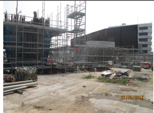
Photo 10 Consecution of column at Portion F on 27 September 2017.
