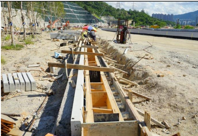
Photo 11 Drainage works at Platform 19.
