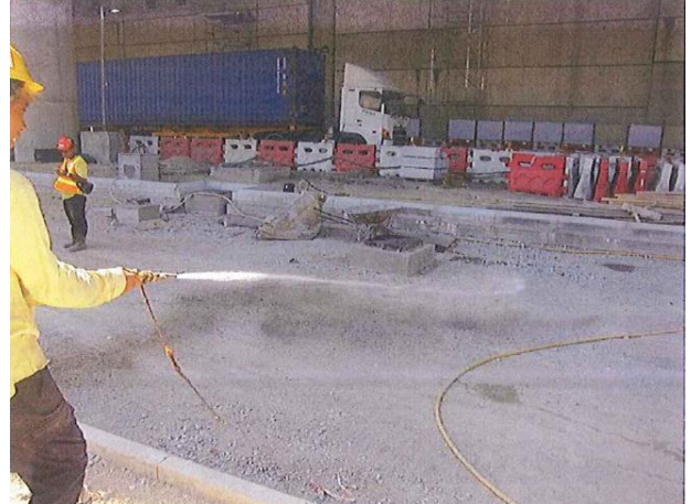
Photo 2 Water spraying by worker for un-accessible area.
