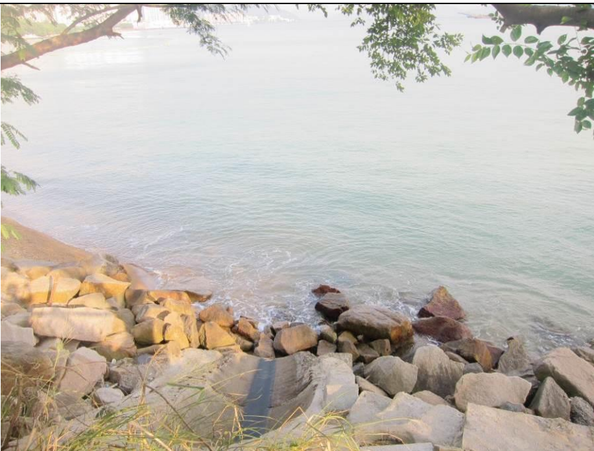
Outfall 1: Clean water is discharging.
