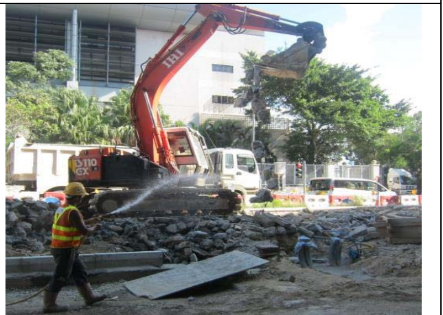
Photo 6 Provide additional water jet for trim formation works.
