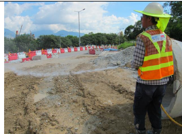
Photo 12 Water spraying for exposed area at Portion H.
