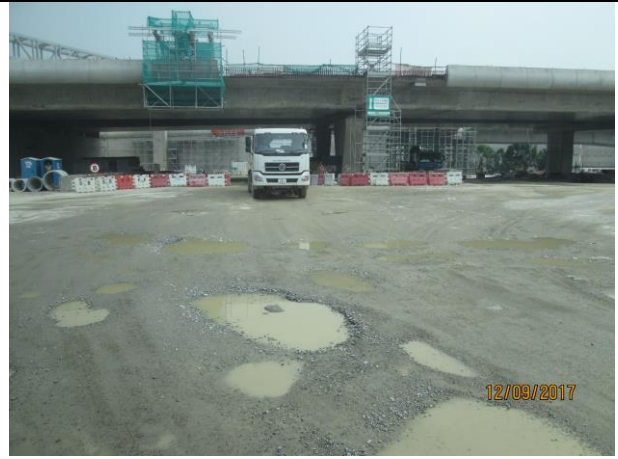
Photo 8 Watering of haul road by water truck to keep road surface wet was observed during the site inspection on 12 September 2017
