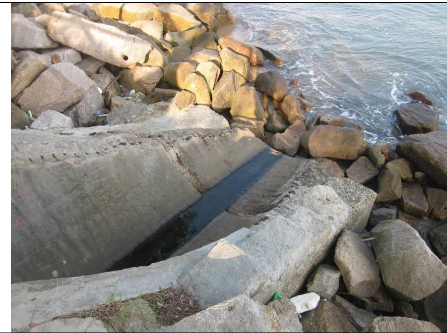
Outfall 1: Clean water is discharging.
