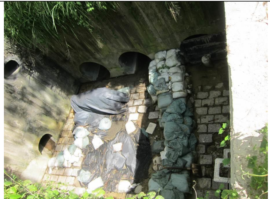
Stream B Outfall: No water is discharging.
