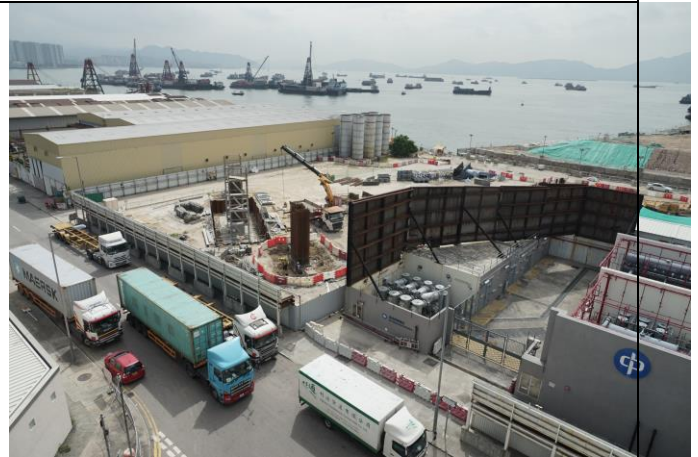
Photo 10 Consecution of column at Portion F on 12 September 2017.
