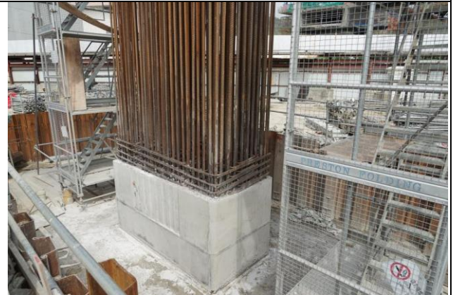
Photo 10 Consecution of column at Portion F on 18 September 2017.
