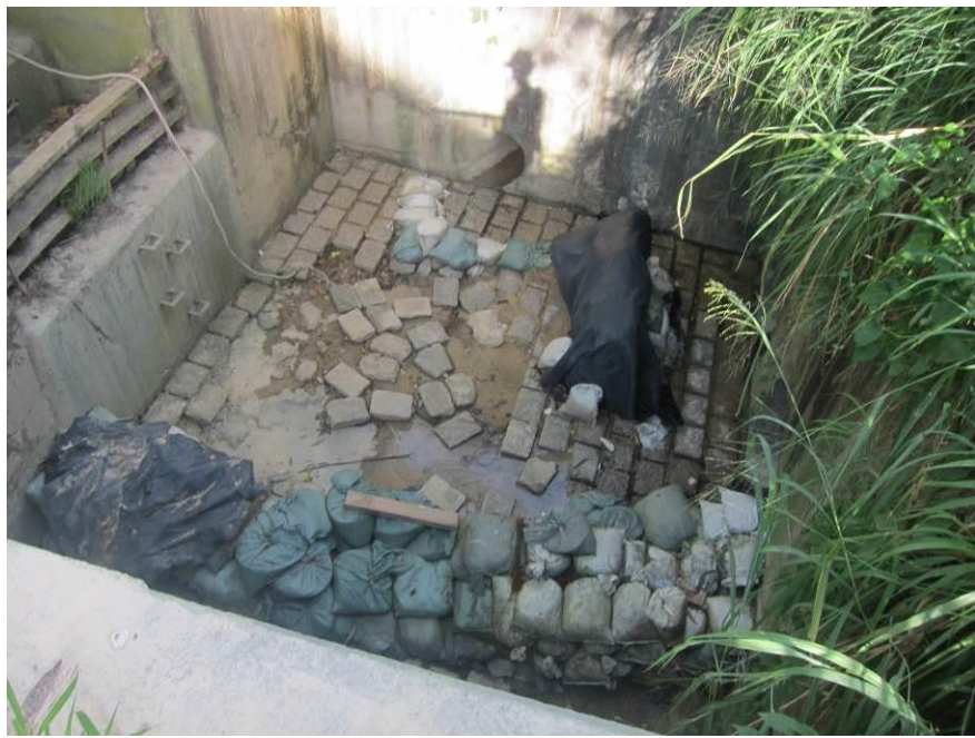
Stream B Outfall: No water is discharging.
