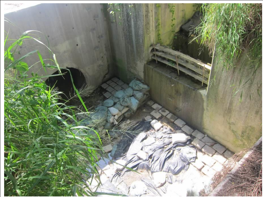
Stream B Outfall: No water is discharging.
