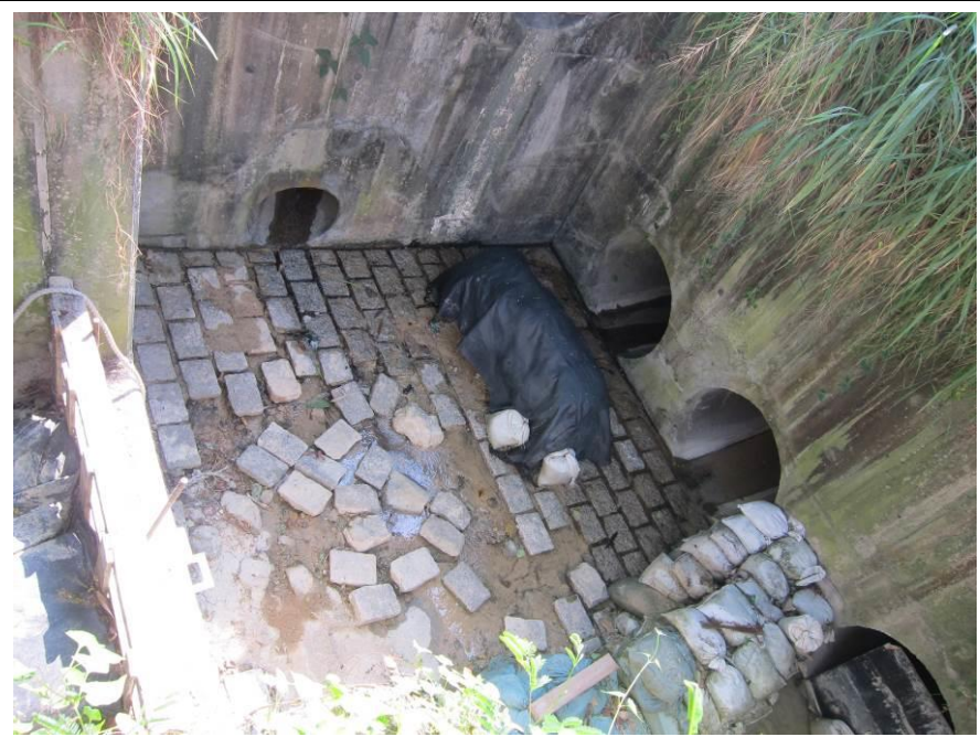
Stream B Outfall: No water is discharging.
