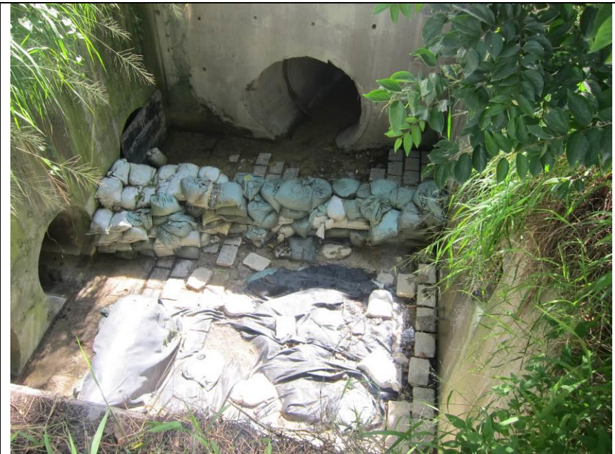
Stream B Outfall: No water is discharging.
