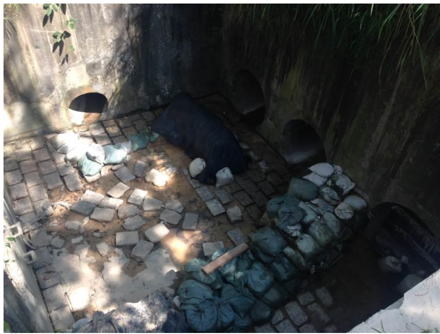
Stream B Outfall: No water is discharging.
