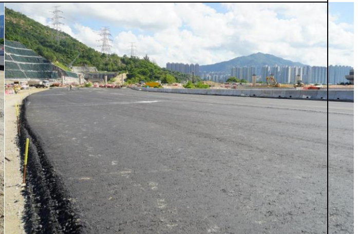
Photo 12 Road pavements works at Platform 19.
