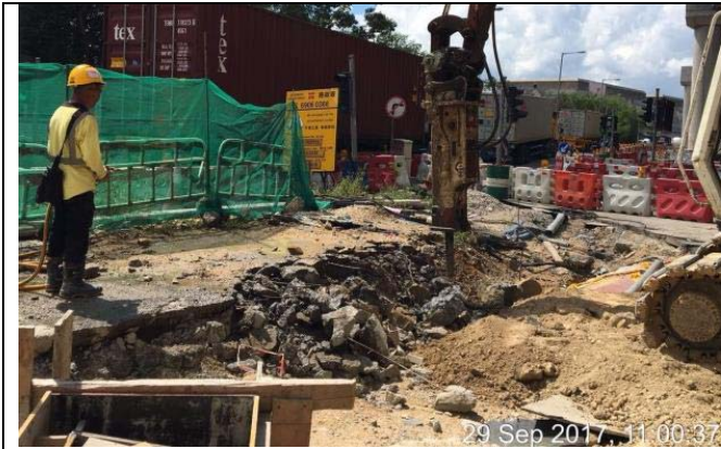
Photo 1 Water spraying for trim formation works on 29 September 2017.
