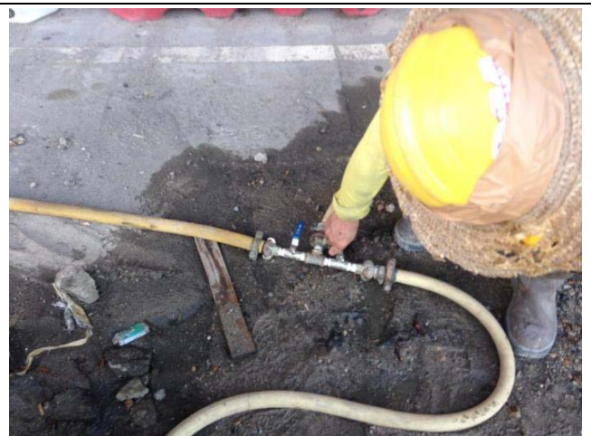
Photo 4 Installation of additional water jet at Lung Mun Road Central Divider.
