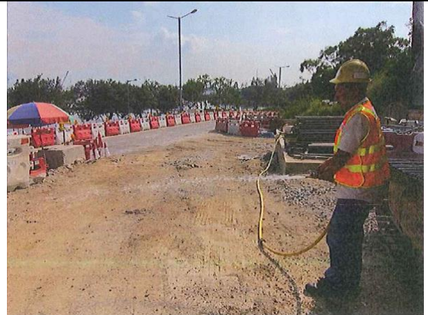
Photo 2 Water spraying by worker for un-accessible area.
