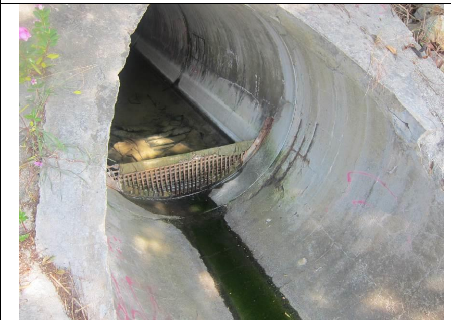
Outfall 1: Clean water is discharging.
