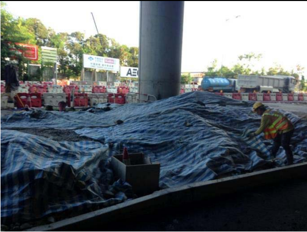
Photo 9 Stockpile was covered with tarpaulin to reduce dust suppression.
