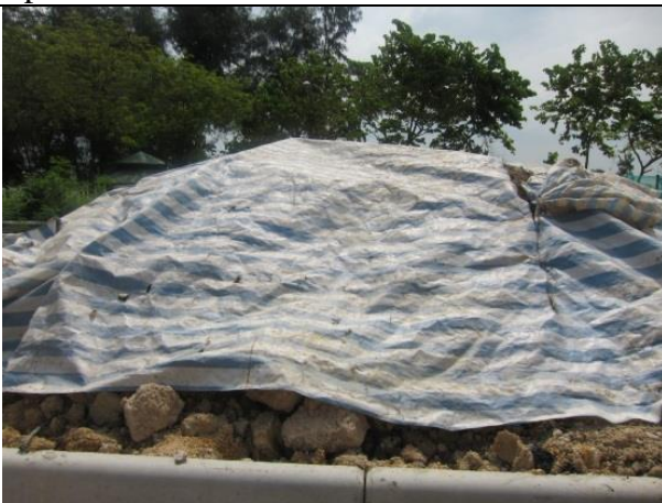
Photo 3 Covered part of the exposed slopes and stockpile by tarpaulin sheet.
