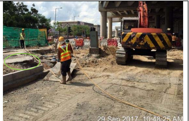
Photo 2 Water spraying for trim formation works on 29 September 2017.
