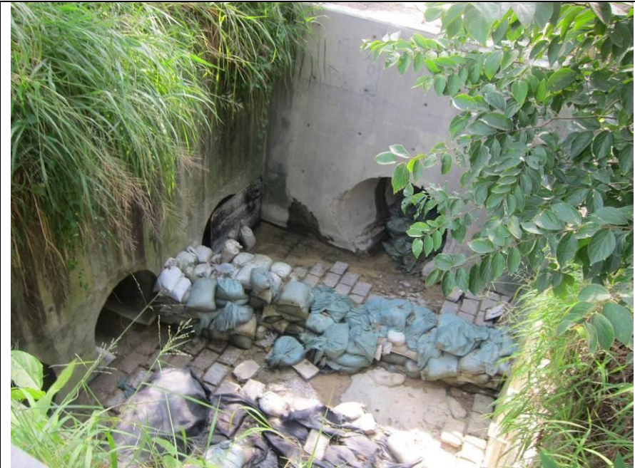
Stream B Outfall: No water is discharging.
