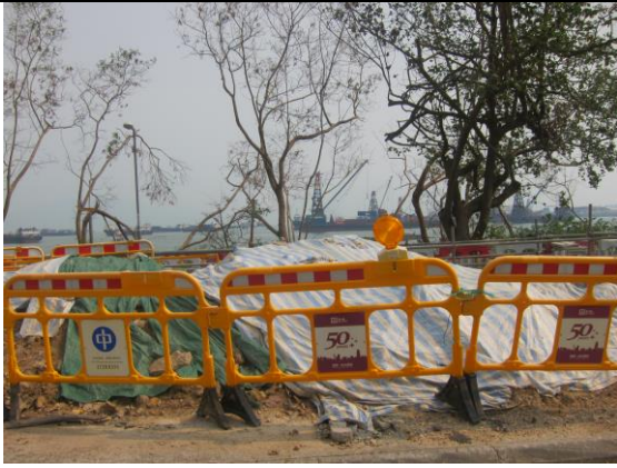
Photo 13 Stockpile at Portion H was covered with tarpaulin.
