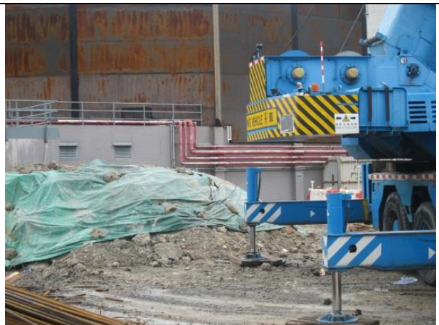
Photo 4 Covered part of stockpile by tarpaulin sheet at Portion F.
