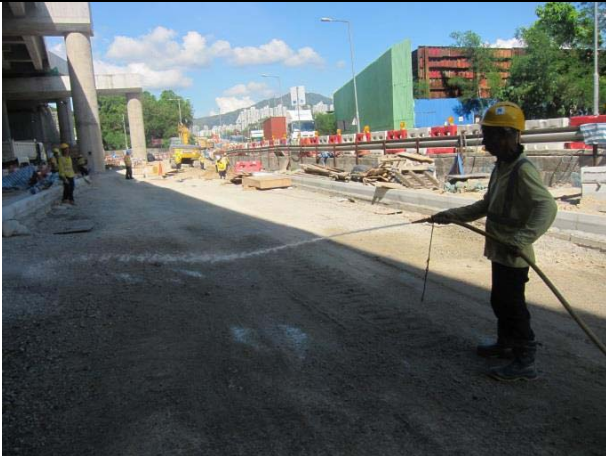
Photo 7 Water spraying at nearby exposed area to reduce dust suppression.
