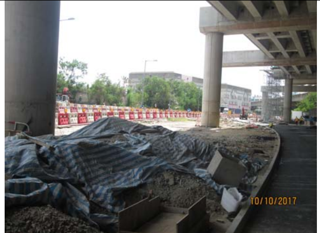
Photo 11 Stockpile covered with tarpaulin was observed during the weekly inspection on 10 October 2017.
