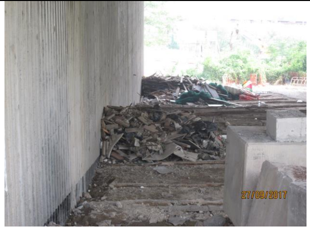
Photo 8 Housekeeping works at TD2 on 27 September 2017
