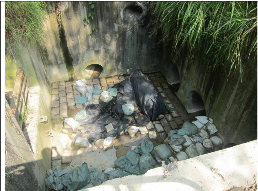
Stream B Outfall: No water is discharging.
