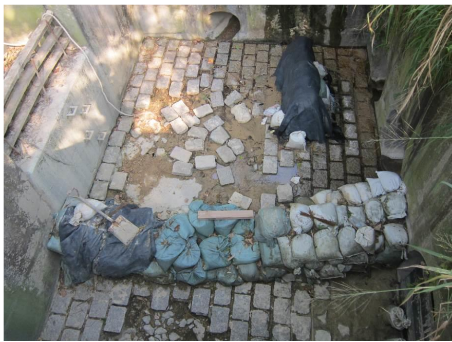
Stream B Outfall: No water is discharging.
