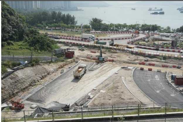
Photo 11 Road and drainage works at Portion H.
