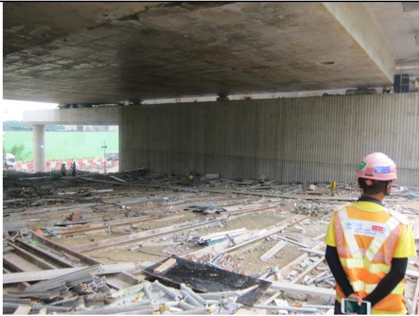
Photo 9 Housekeeping works at TD1 on 12 September 2017.
