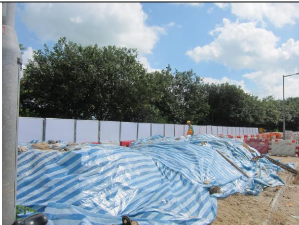
Photo 11 Covered stockpile by tarpaulin sheet at Portion H.
