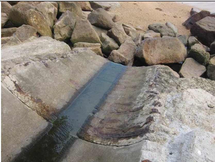
Outfall 1: Clean water is discharging.
