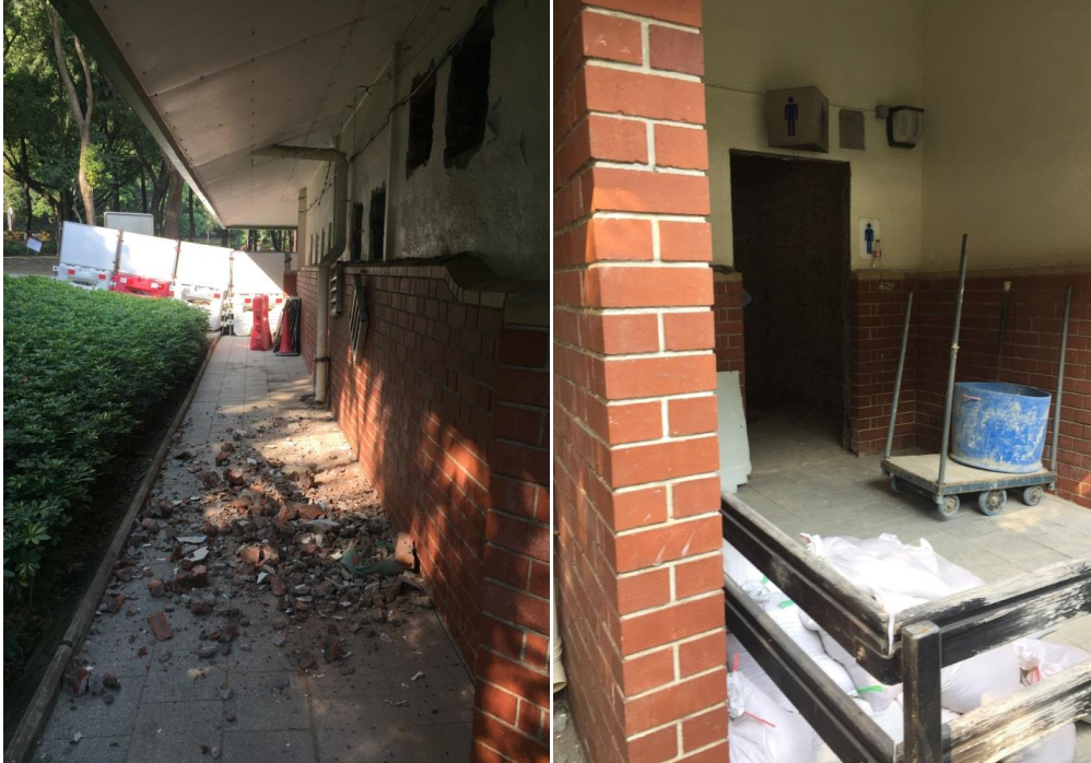
Maintenance works are carried out near ASR10.
