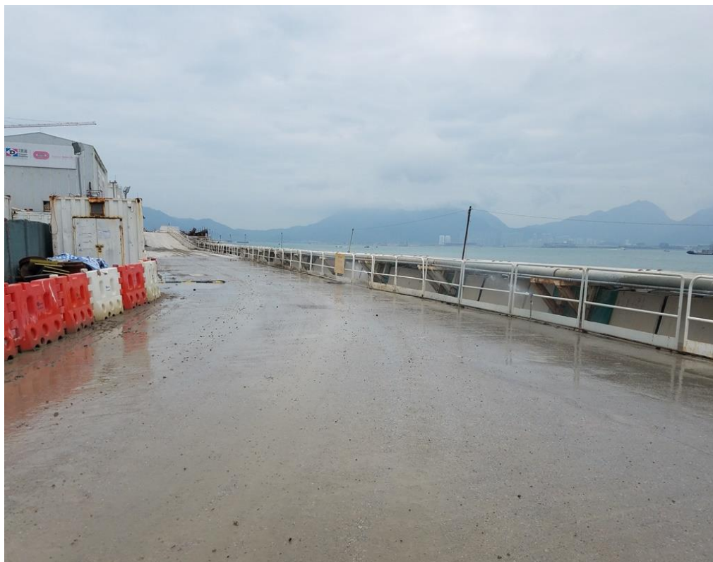
Water spraying was applied frequently during dry conditions.(Works Area Portion N-C)
