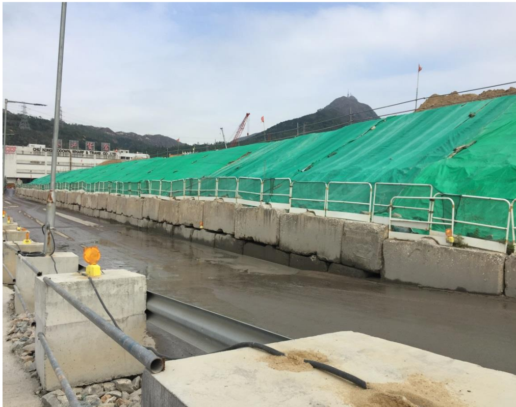
Exposed soil are covered by tarpaulin sheets. (Works Area Portion N-A)
