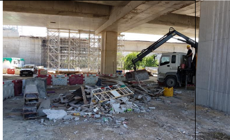
Photo 8 Housekeeping works at Retaining Wall B.
