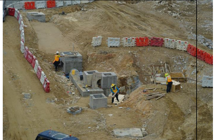
Photo 16 Drainage works at Platform 19
