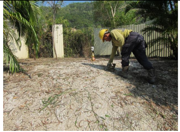
Photo 20 Housekeeping works at existing Grave G1 under Retaining Wall B.
