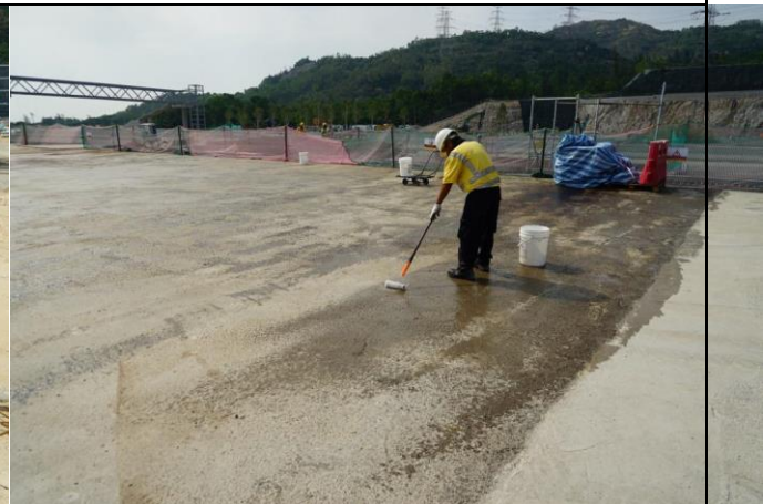
Photo 12 Road works at Retaining Wall B.
