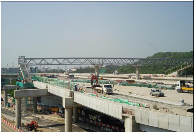
Photo 15 Construction of bus shelter at Retaining Wall B.
