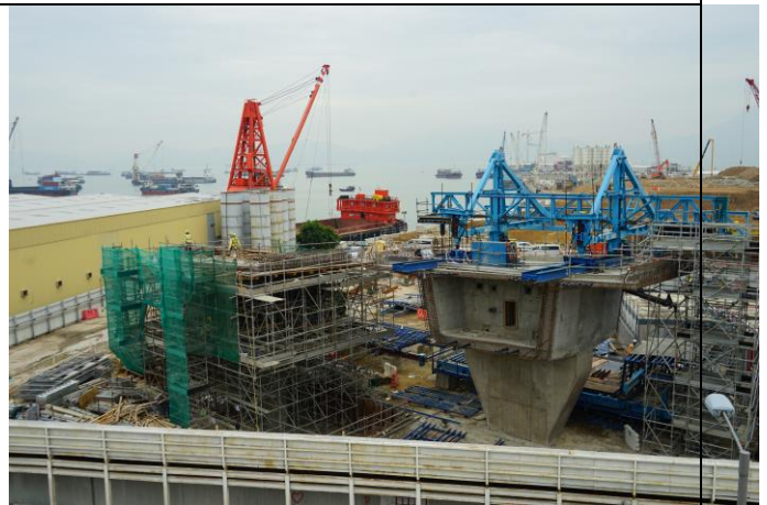
Photo 16 Construction of column at Portion F
