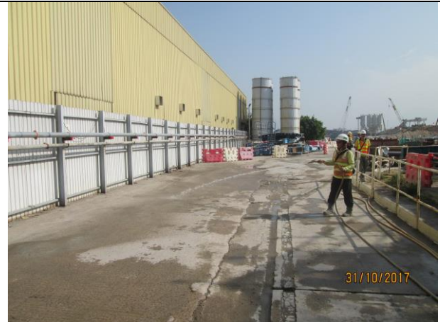
Photo 10 Watering of haul road to keep road surface wet was observed at Portion F during the site inspection on 31 October 2017
