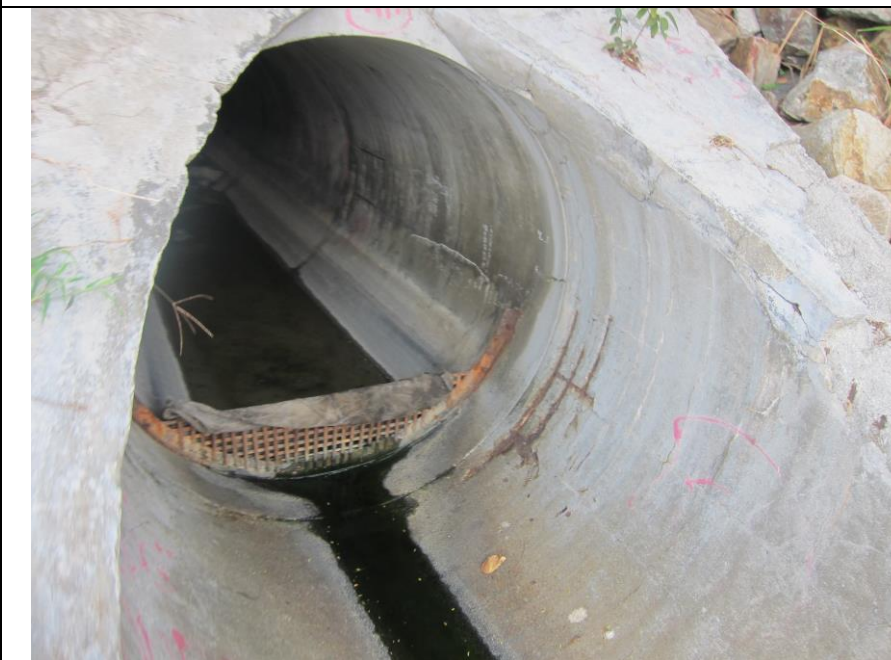
Outfall 1: No water is discharging.
