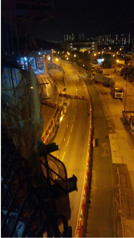
TTA works at Lung Mun Road during Night Time
