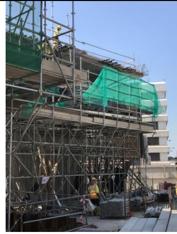
Photo 14 Construction of column at Portion F.
