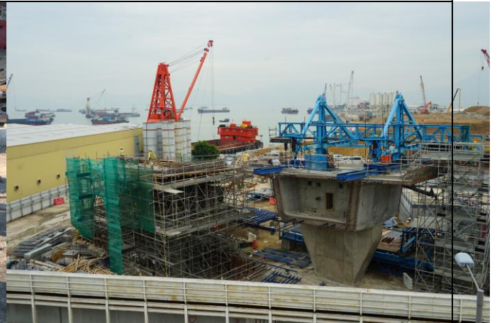
Photo 18 Construction of column at Portion F
