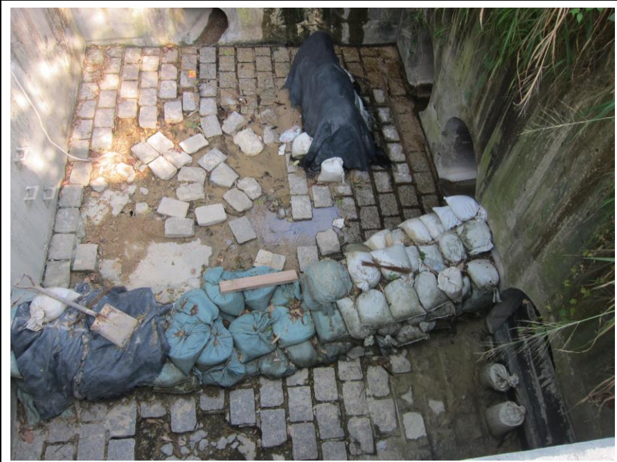
Stream B Outfall: No water is discharging.
