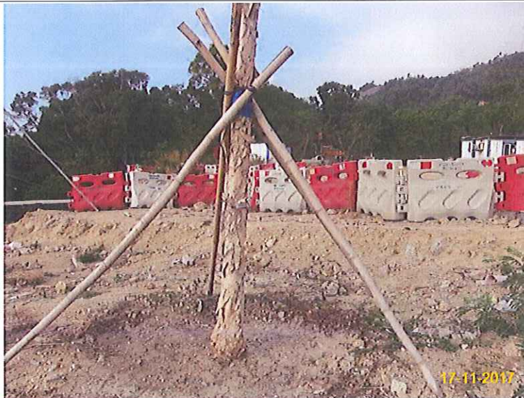
Item 2. Tree Transplanting works conducted on 22-May-17.
