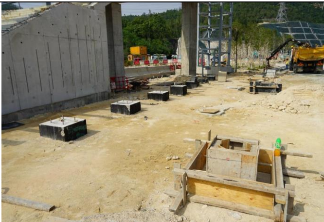
Photo 11 Drainage works at Platform 19.
