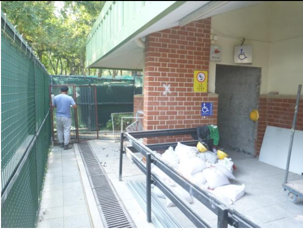
Photo 19 Construction works was undertaken near the ASR10
