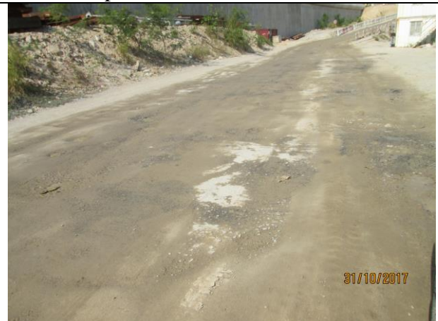
Photo 12 Watering of haul road by water truck to keep road surface wet was observed during the site inspection on 31 October 2017
