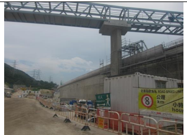
Photo 6 Set speed control at ~8km/hr for all vehicles using the haul road
