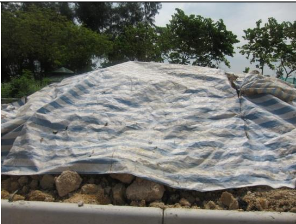
Photo 3 Covered part of the exposed slopes and stockpile by tarpaulin sheet.
