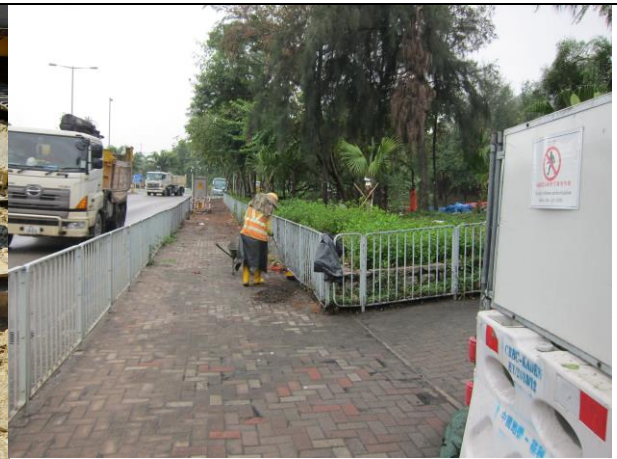
Photo 14 Housekeeping works at Lung Mun Road.
