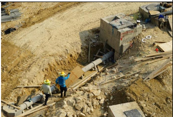
Photo 17 Drainage works at Platform 19.
