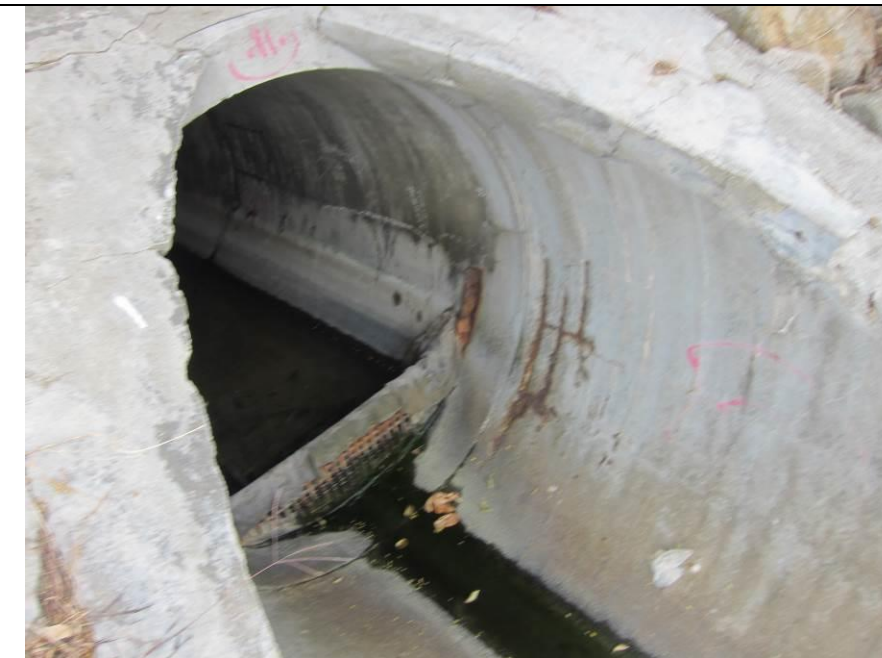
Outfall 1: No water is discharging.
