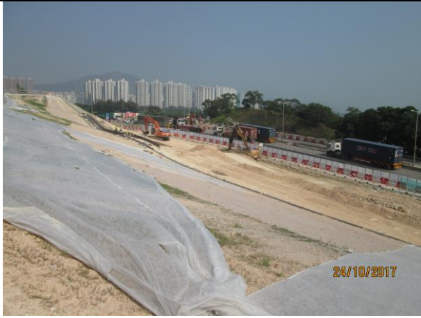
Photo 7 Photo taken of hydro seeding for the exposed sloop at slop 170 during the site inspection on 24 October 2017
