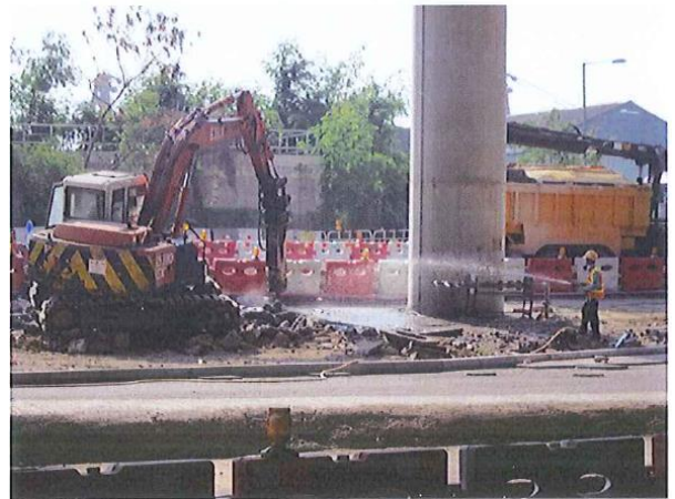
Photo 2 Water spraying by worker for un-accessible area.
