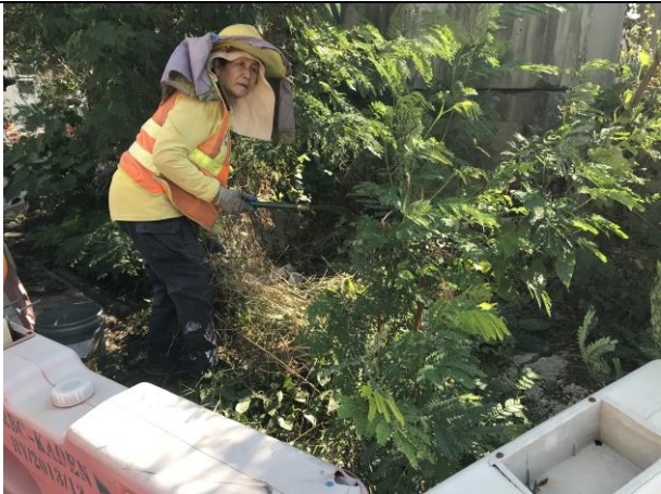
Photo 9 Removal of weeds at Lung Mun Road near Butterfly Beach Laundry.
