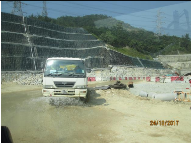
Photo 7 Watering of haul road by water truck to keep road surface wet was observed during the site inspection on 24 October 2017
