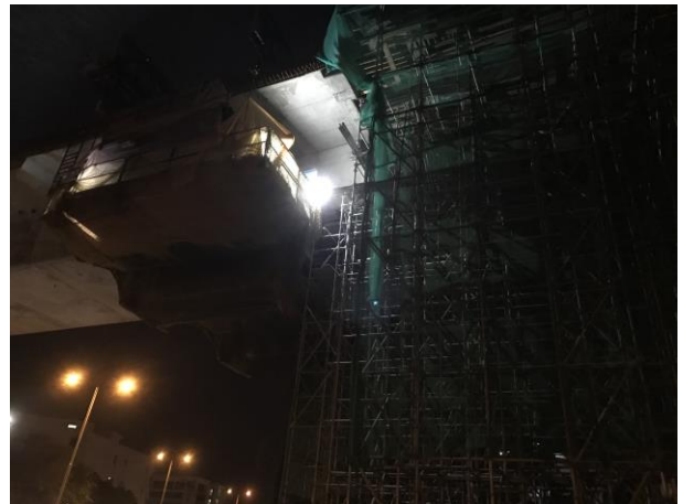
Finishing works at formtraveller during Night Time and limited light was used
