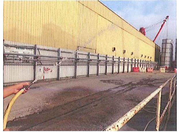
Photo 2 Water spraying by worker for un-accessible area.
