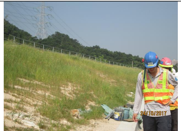
Photo 4 Hydro seeding for the exposed slope at slope 170.
