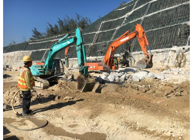
Photo 2 Water spraying by worker for un-accessible area.
