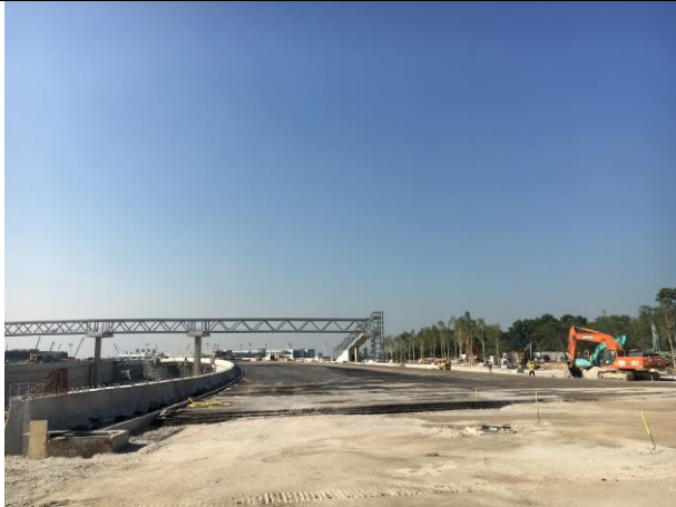
Photo 15 Construction of bus shelter at Retaining Wall B.
