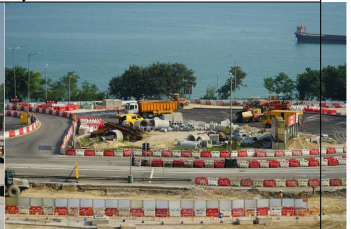
Photo 16 Road pavements works at Lung Mun Road.
