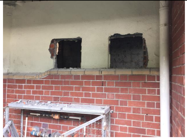
Photo 20 Construction works was undertaken near the ASR10
