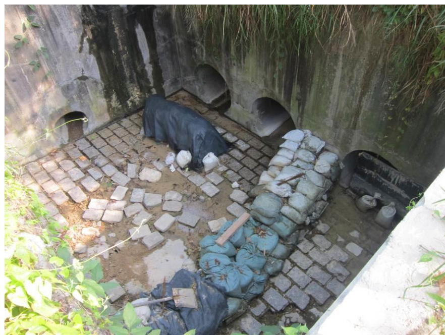
Stream B Outfall: No water is discharging.
