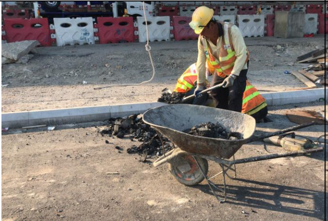
Photo 17 Housekeeping works at Lung Mun Road.
