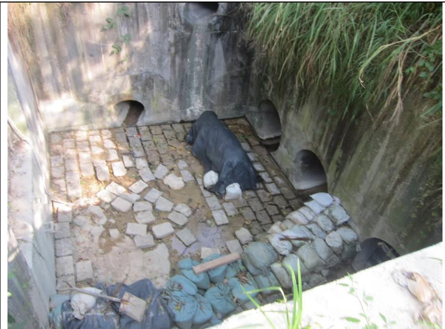
Stream B Outfall: No water is discharging.
