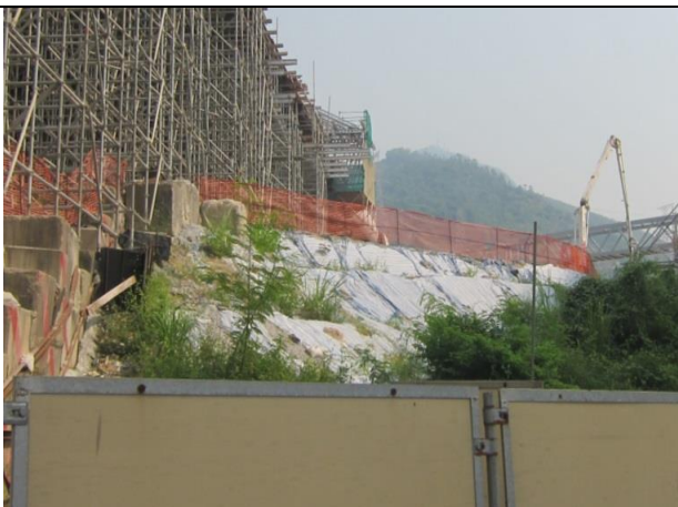
Photo 5 Covered part of the exposed slopes and stockpile by tarpaulin sheet.
