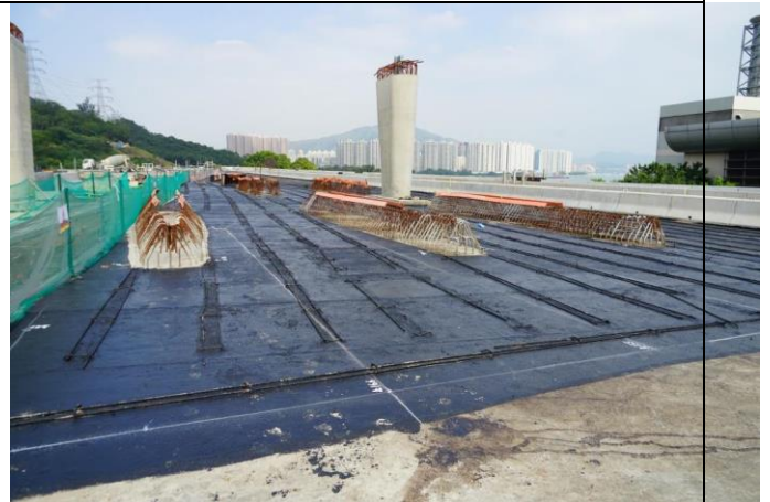
Photo 10 Road works at Retaining Wall B.
