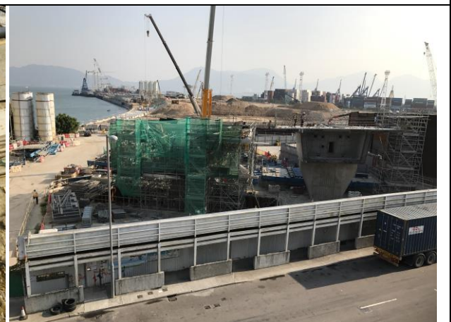
Photo 18 Construction of column at Portion F
