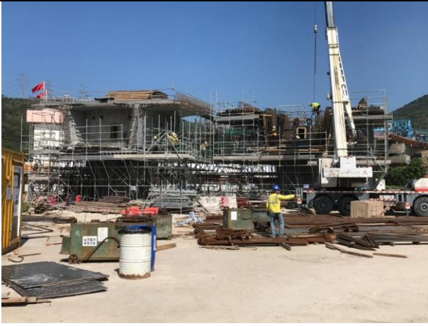
Photo 13 Construction of column at Portion F.
