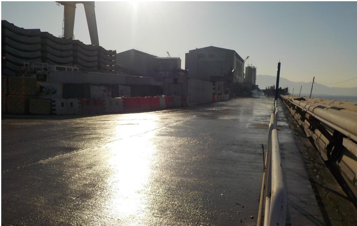
Water spraying was applied frequently during dry conditions.(Works Area Portion N-B)
