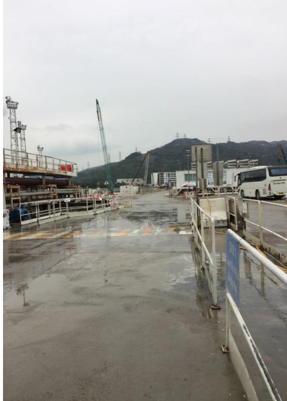
Water spraying was applied frequently during dry conditions.(Works Area Portion N-B)
