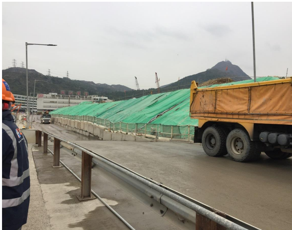
Exposed soil at Portion N-A was also covered by tarpaulin sheets. (Works Area Portion N-A)
