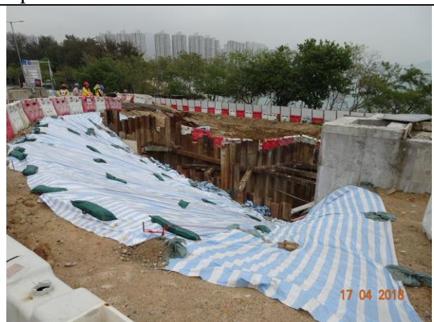
Photo 10 Dust mitigation measure was observed at Portion H during the join site inspection on 17 April 2018
