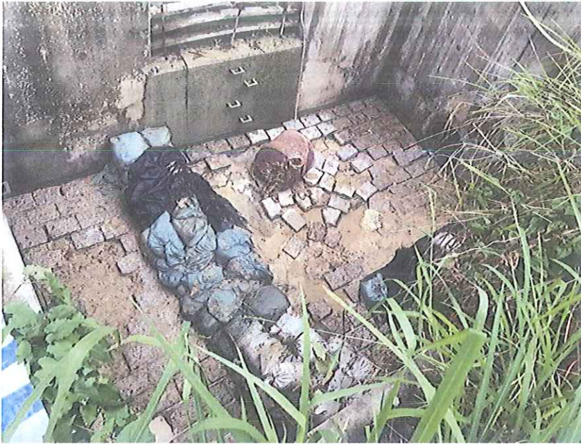
Stream B Outfall: No water is discharging.
