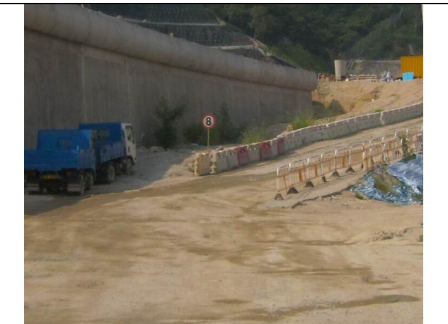
Photo 6 Set speed control at ~8km/hr for all vehicles using the haul road
