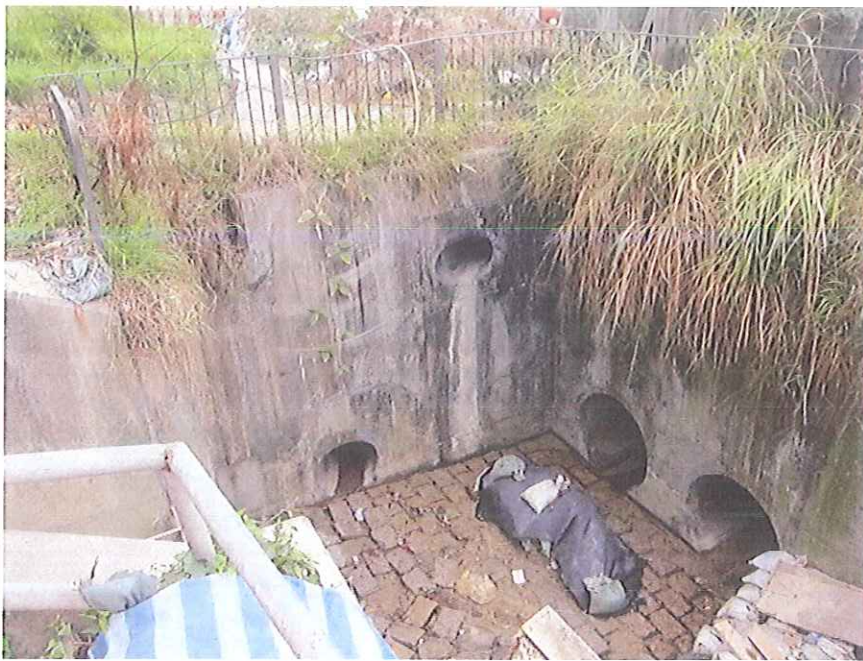
Stream B Outfall: No water is discharging.
