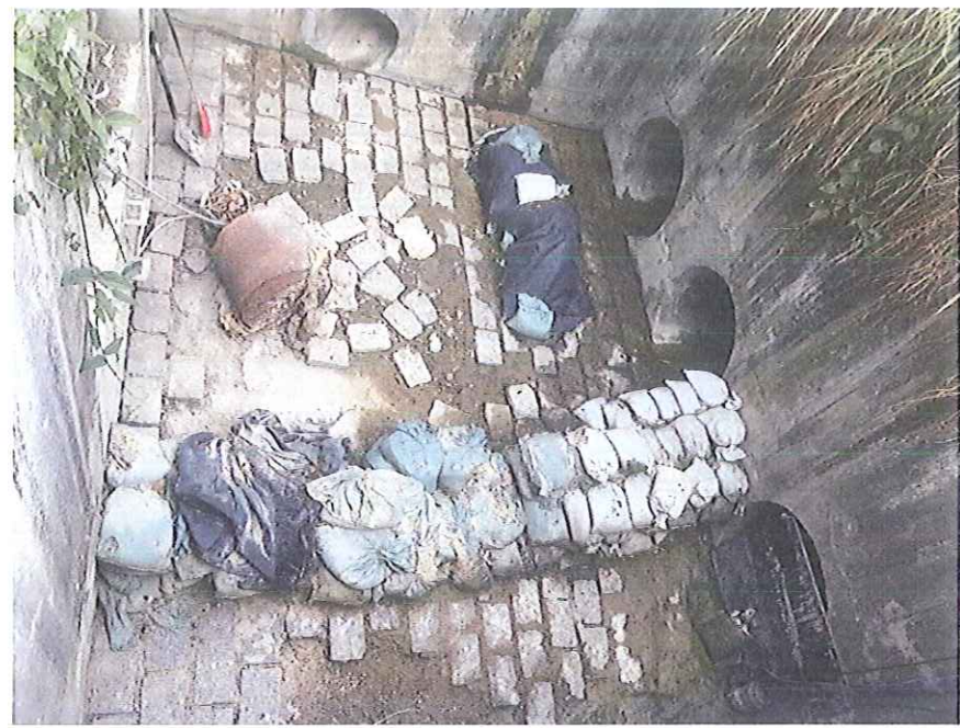
Stream B Outfall: No water is discharging.
