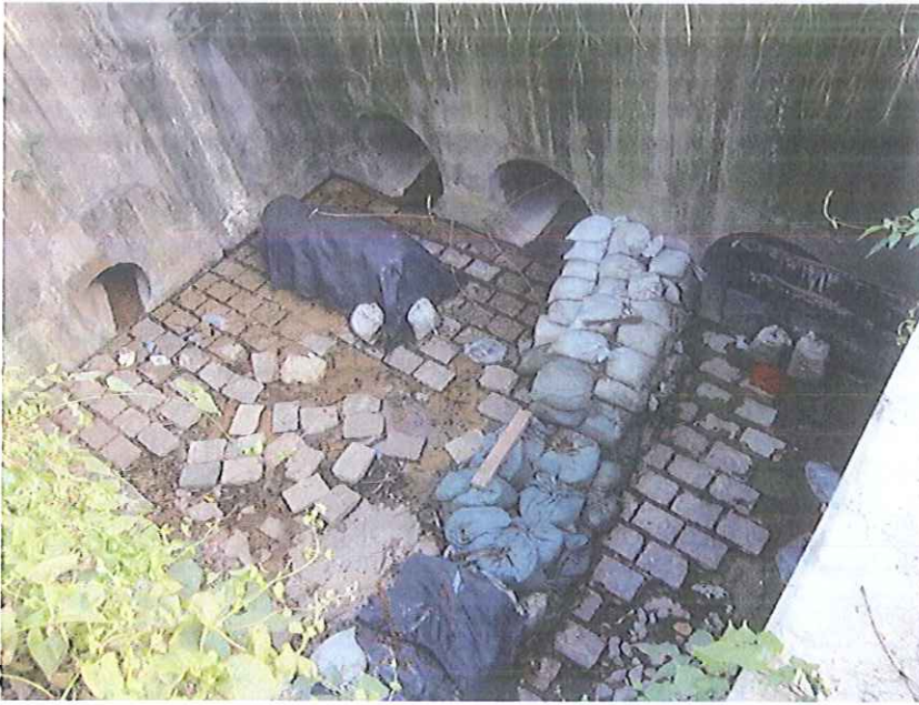
Stream B Outfall: No water is discharging.
