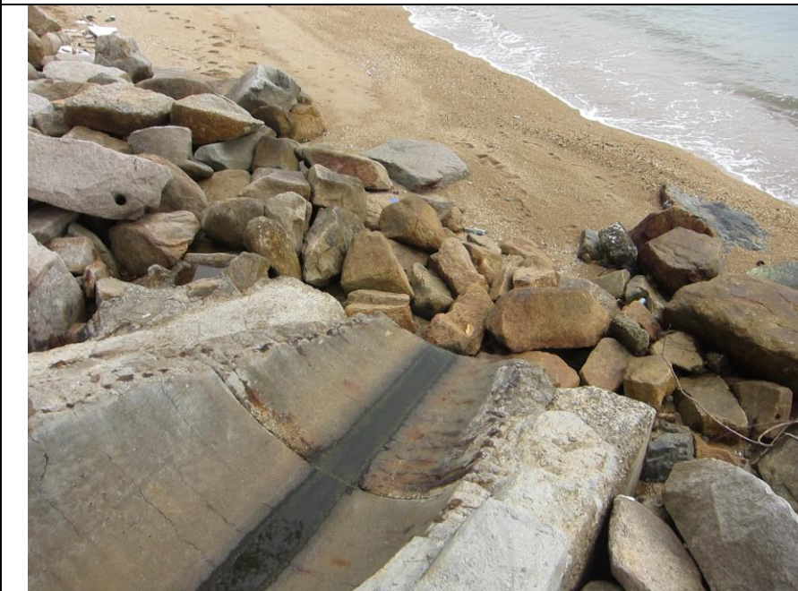
Outfall 1: No water is discharging.
