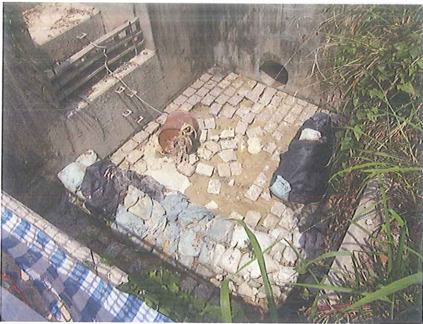
Stream B Outfall: No water is discharging.
