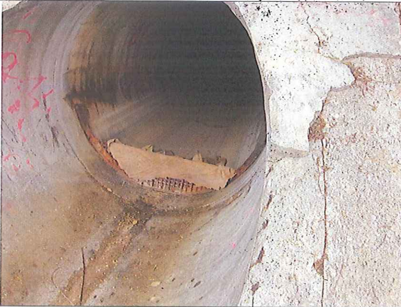
Outfall 1: No water is discharging.
