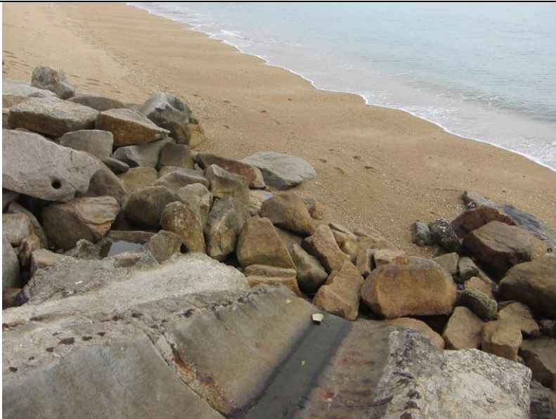
Outfall 1: No water is discharging.
