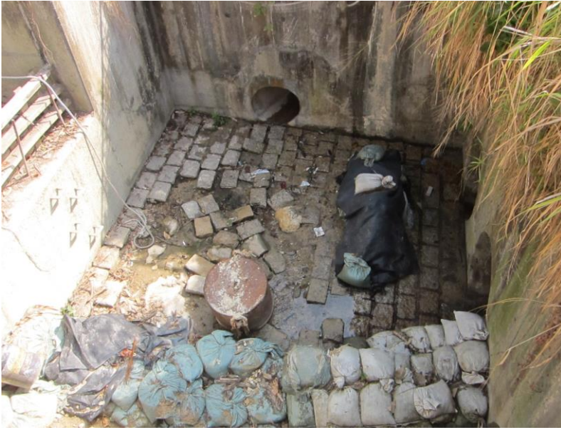
Stream B Outfall: No water is discharging.
