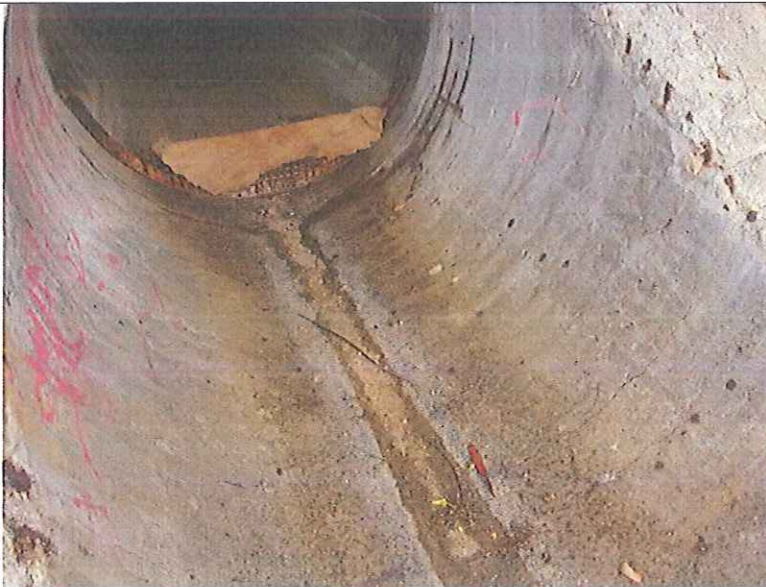
Outfall 1: No water is discharging.
