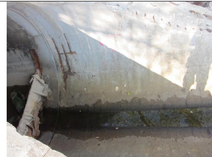
Outfall 1: No water is discharging.
