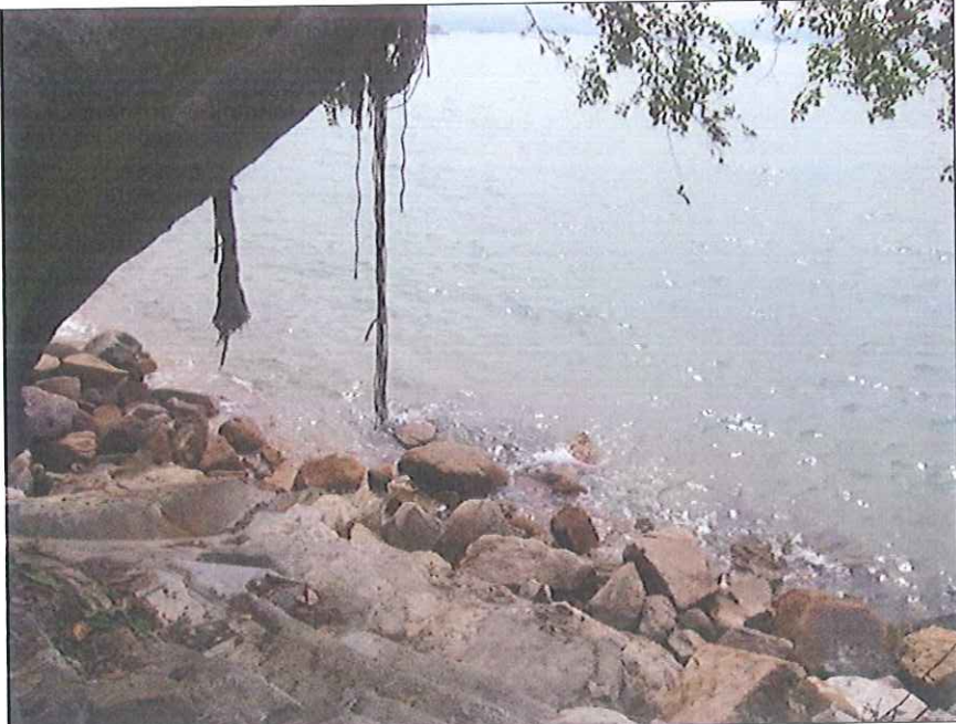
Outfall 1: No water is discharging.
