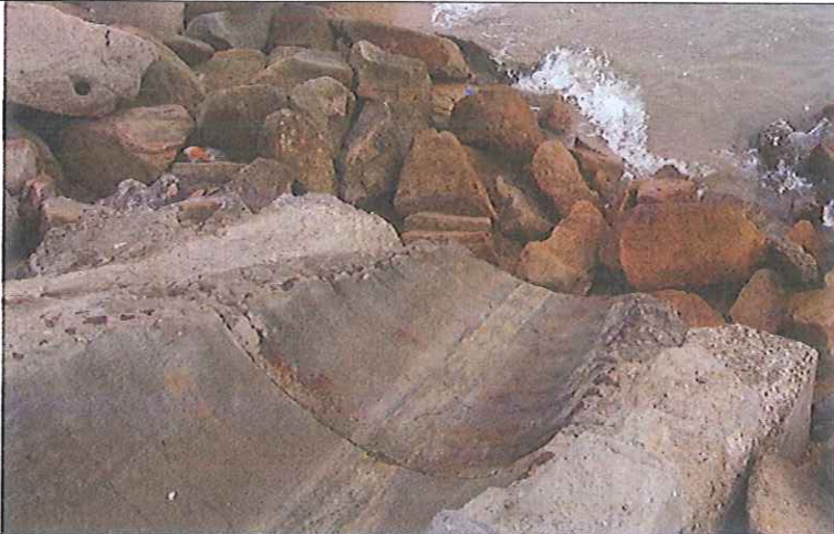
Outfall 1: No water is discharging.
