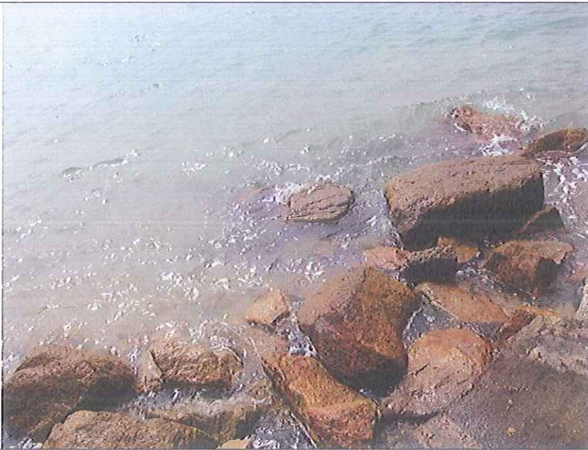
Outfall 1: No water is discharging.
