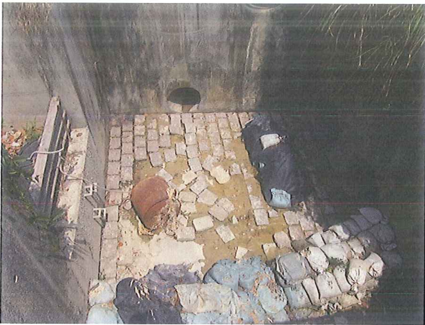
Stream B Outfall: No water is discharging.
