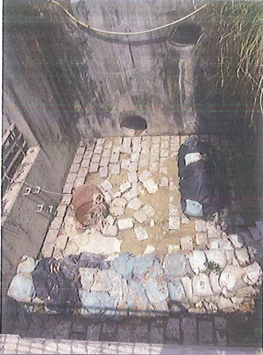
Stream B Outfall: No water is discharging.
