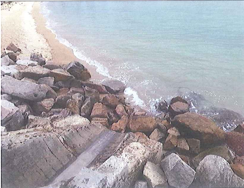
Outfall 1: No water is discharging.
