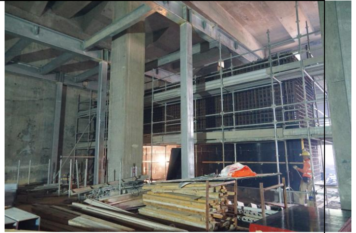
Photo 14 Construction of storage area at Retaining Wall B.
