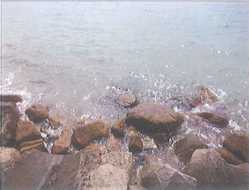
Outfall 1: No water is discharging.
