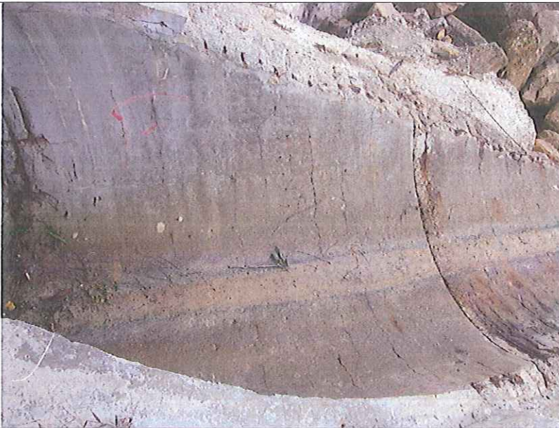
Outfall 1: No water is discharging.
