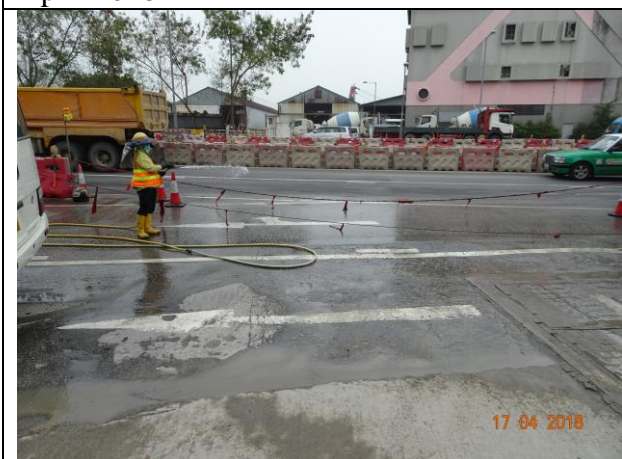
Photo 11 Dust mitigation measure was observed at Lung Mun Road during the join site inspection on 17 April 2018
