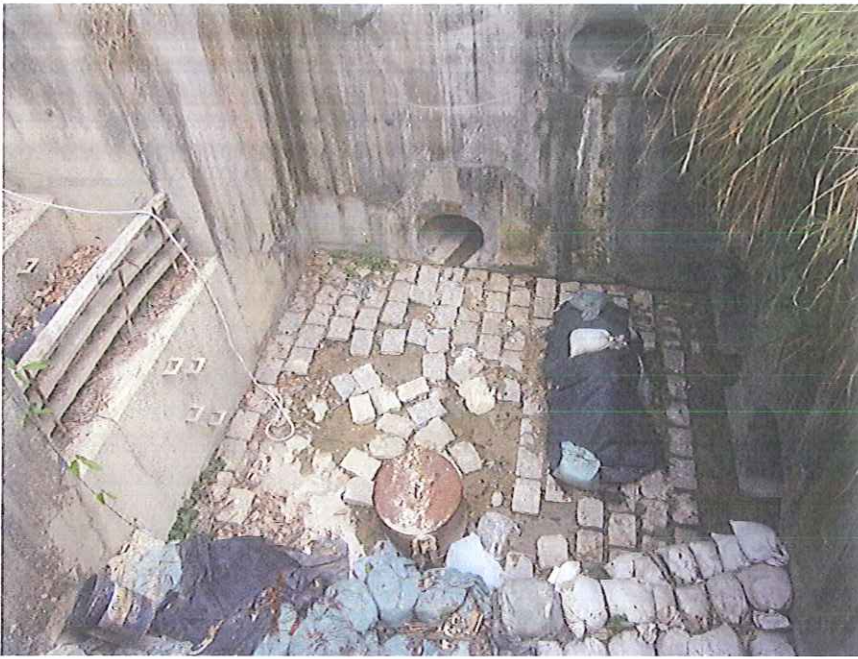
Stream B Outfall: No water is discharging.
