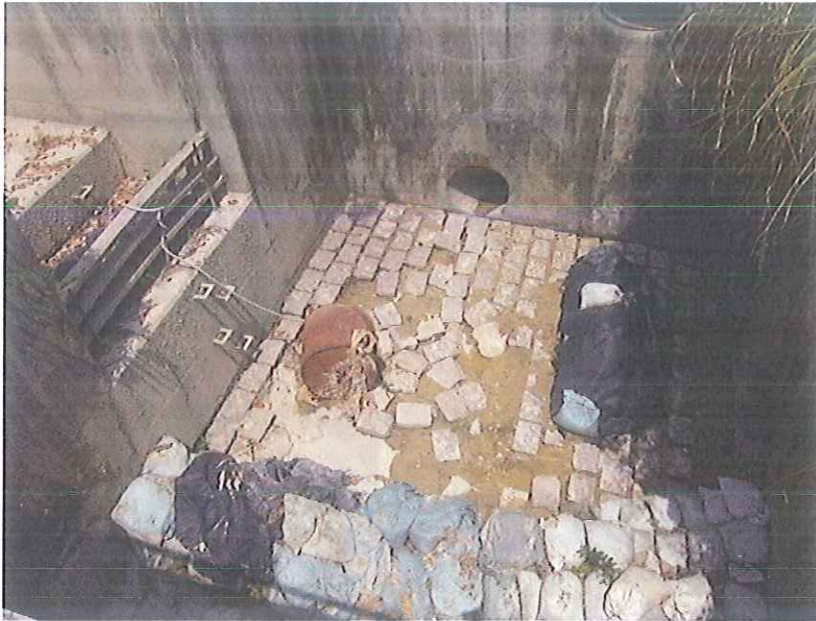
Stream B Outfall: No water is discharging.
