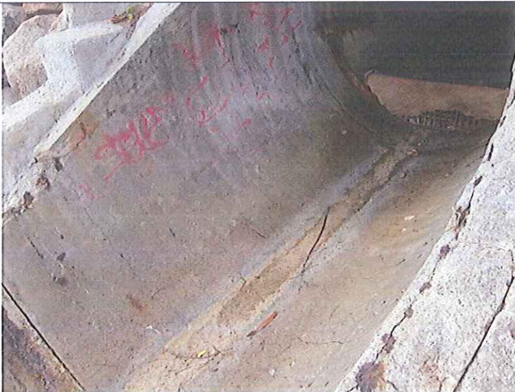
Outfall 1: No water is discharging.
