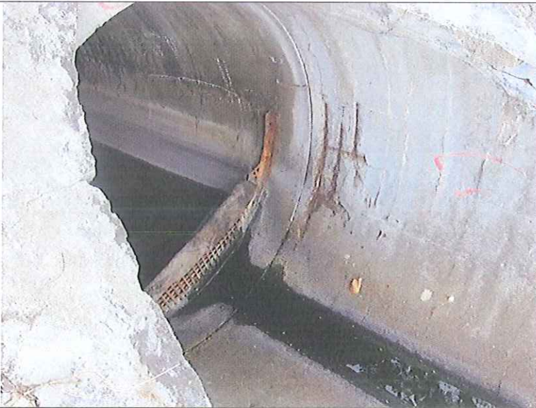
Outfall 1: No water is discharging.
