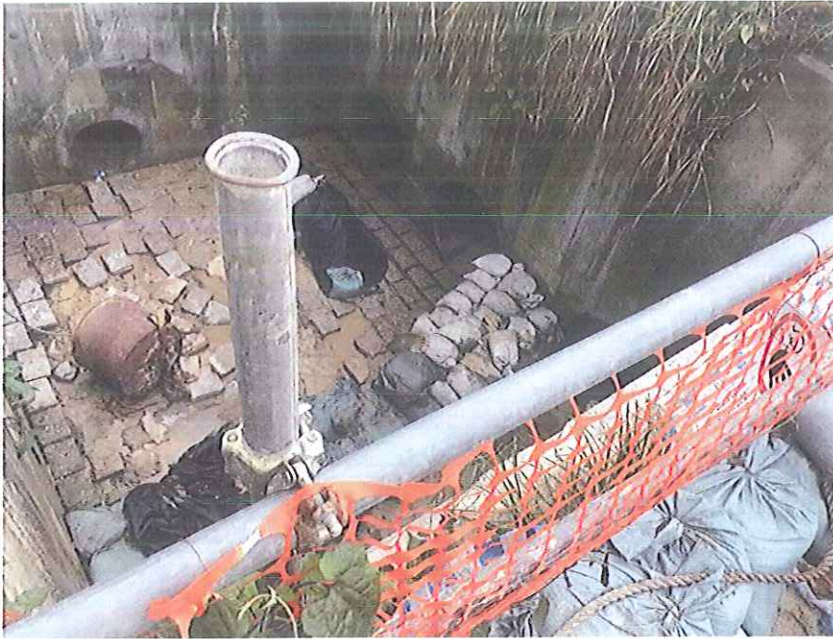
Stream B Outfall: No water is discharging.
