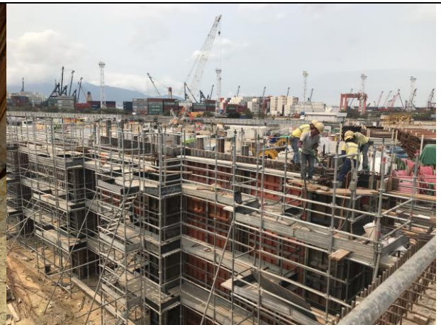
Photo 16 Construction of pile cap at Portion F
