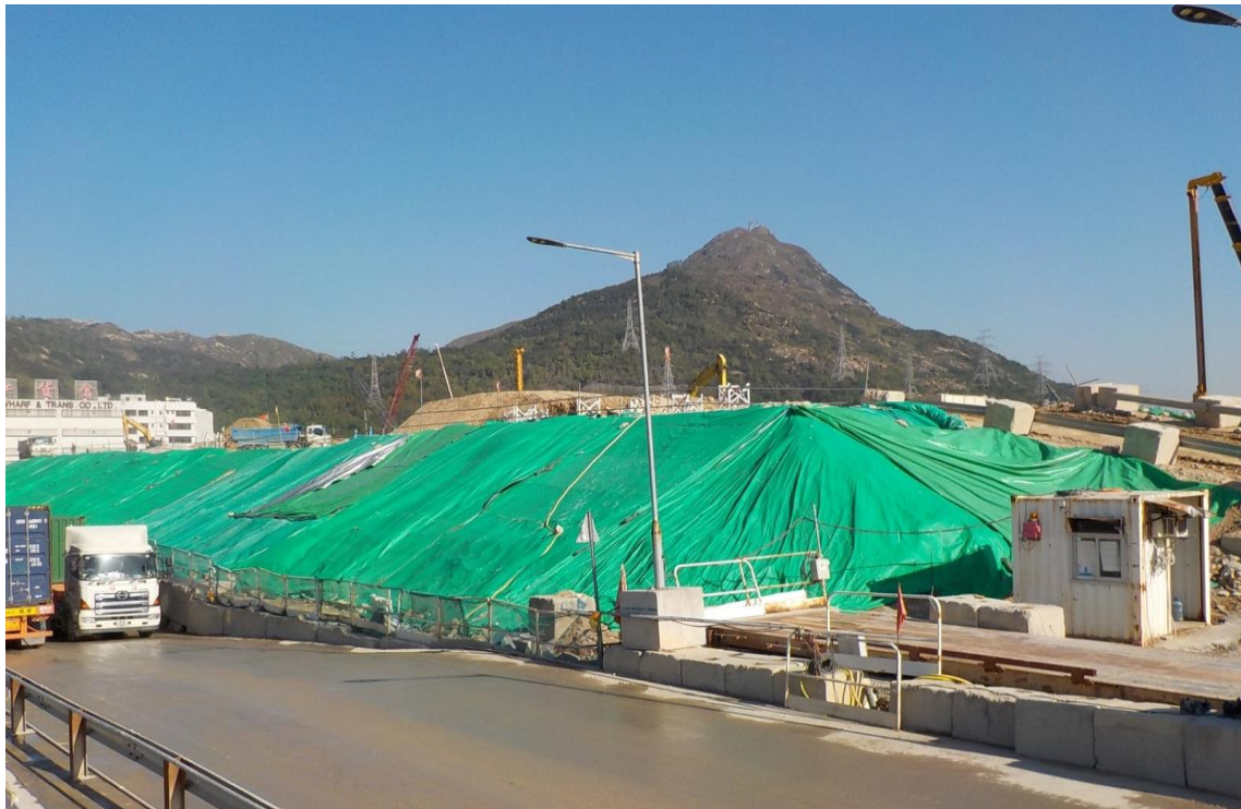
Exposed soil at Portion N-A was covered by tarpaulin sheets. (Works Area Portion N-A)
