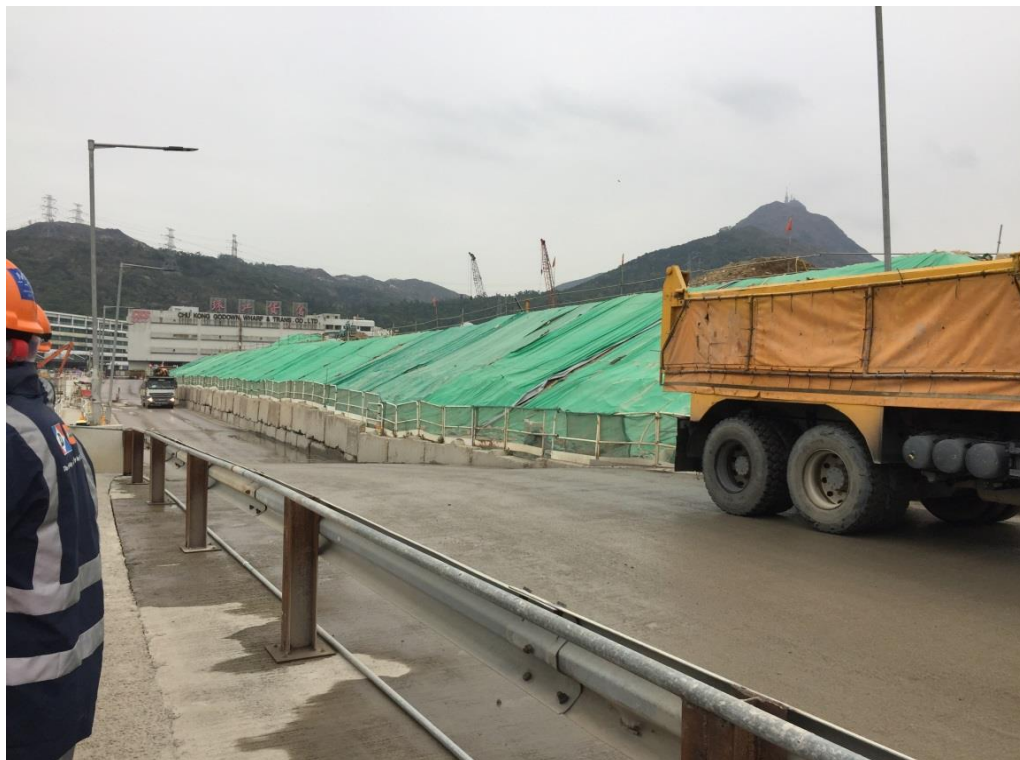
Exposed soil at Portion N-A was also covered by tarpaulin sheets. (Works Area Portion N-A)
