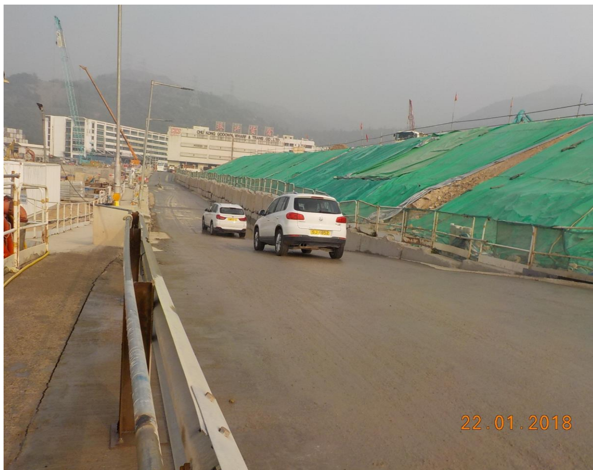
Exposed soil at Portion N-A was covered by tarpaulin sheets. (Works Area Portion N-A)
