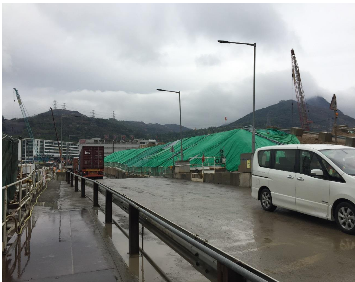
Water spraying was applied to prevent dust impact. (Works Area Portion N-A)
