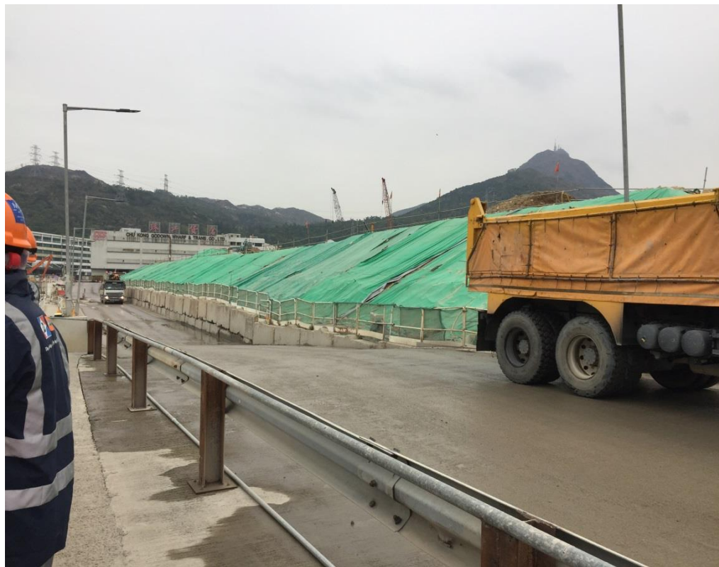
Exposed soil at Portion N-A was also covered by tarpaulin sheets. (Works Area Portion N-A)
