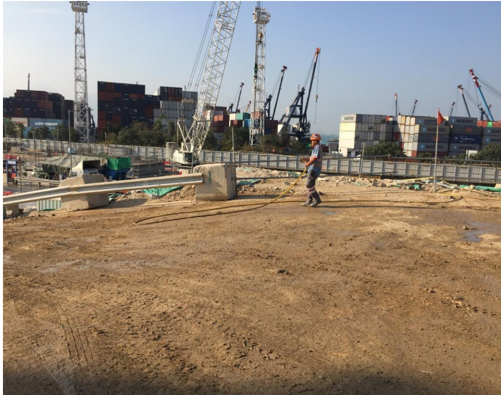
Water spraying was applied frequently during dry conditions.(Works Area Portion N-A)
