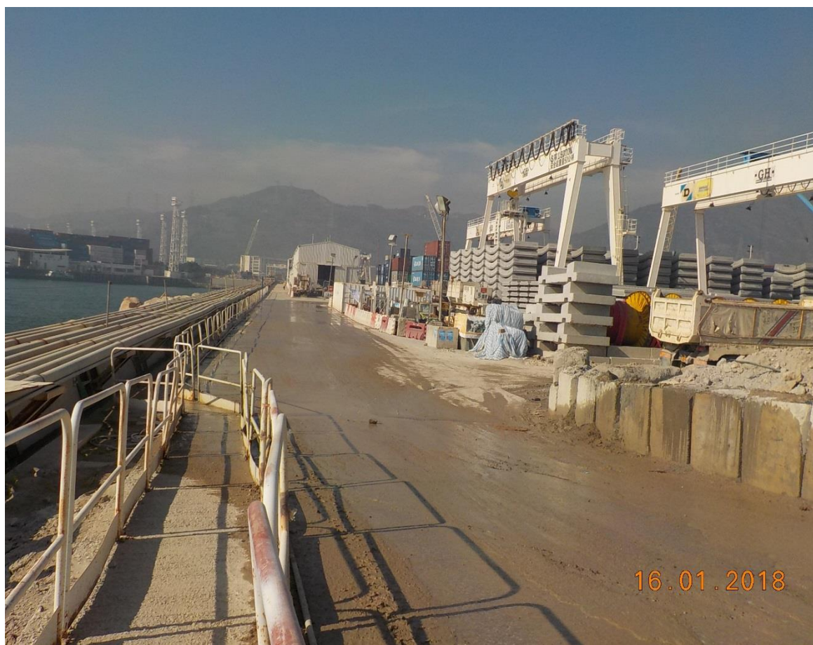
Water spraying was applied to prevent dust impact. (Works Area Portion N-B)
