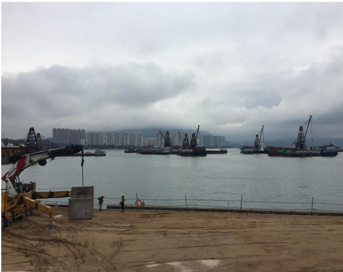
Barges not under this Contract are observed near the site
