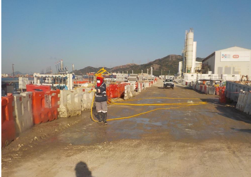
Water spraying was applied frequently during dry condition. (Works Area Portion N-B)
