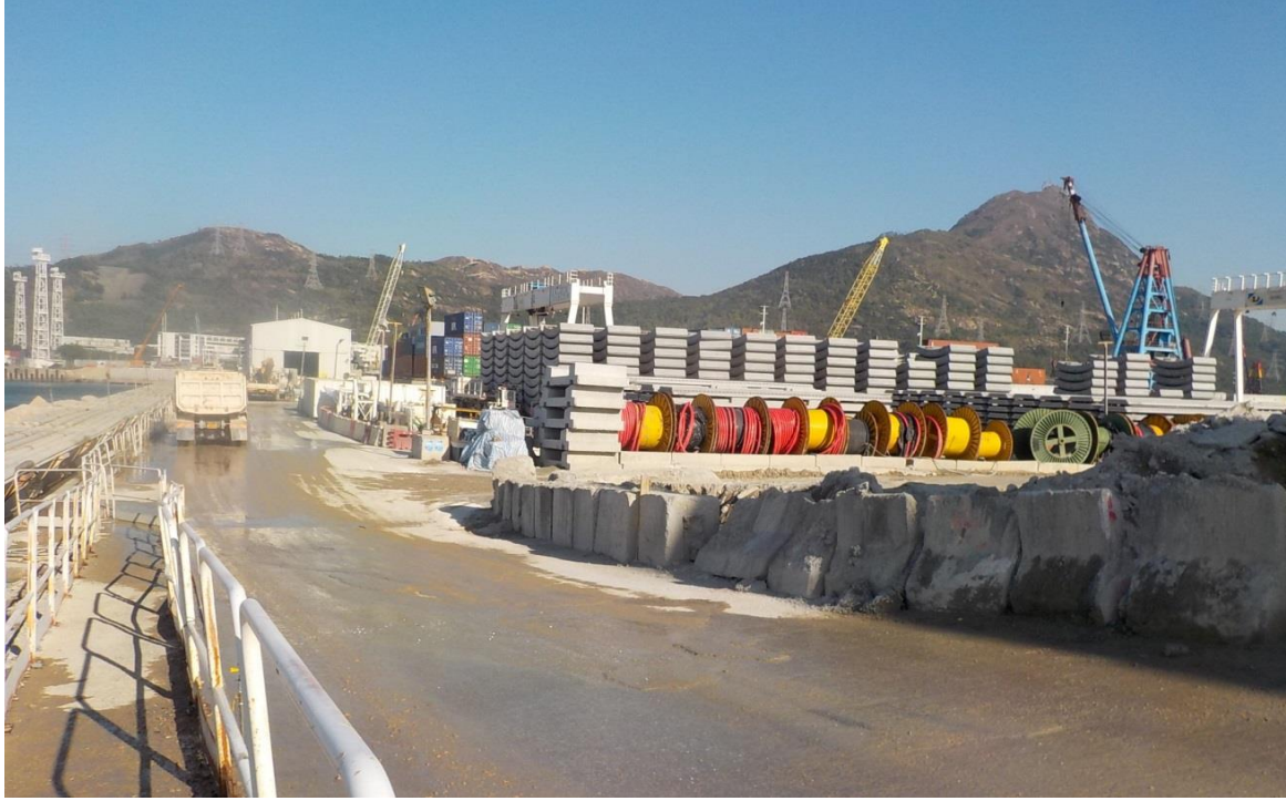
Water spraying was applied frequently during dry conditions.(Works Area Portion N-C)
