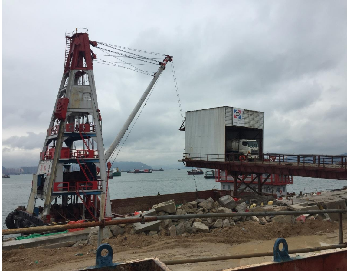
Barge for transportation of C&D material
