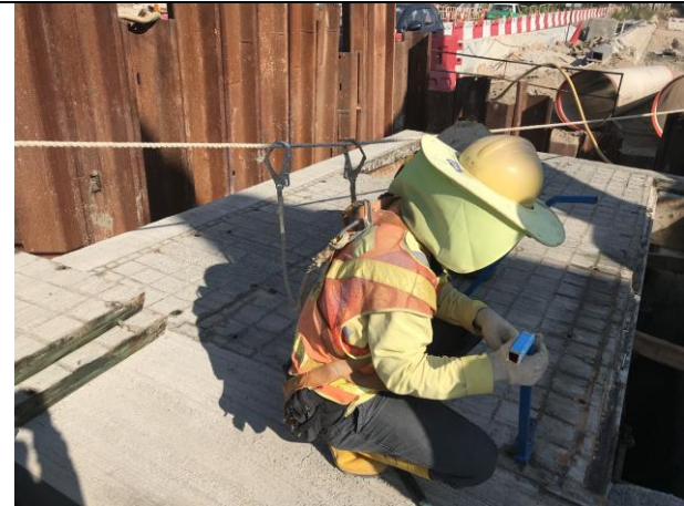
Photo 16 Drainage works at Platform 19
