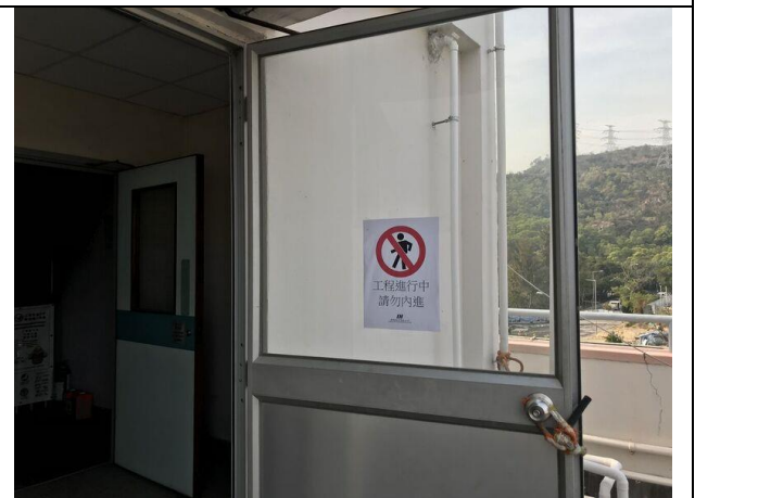
Photo 18 Photo taken on 6 February 2018 at the roof top of Pillar Point Fire Station
