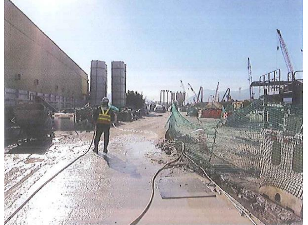
Photo 2 Water spraying by worker for un-accessible area.
