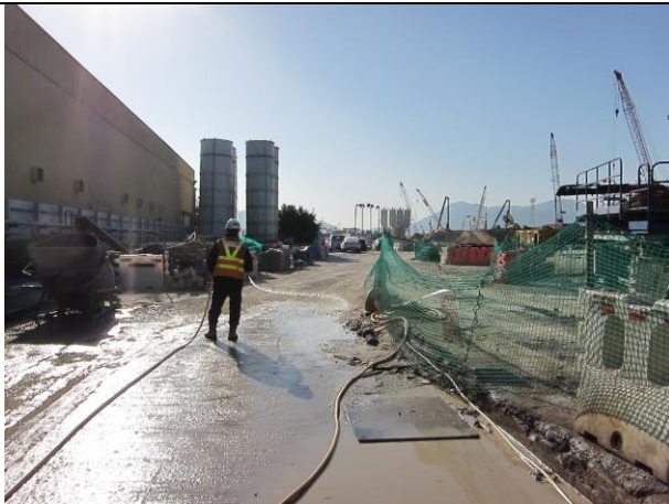
Dust mitigation measures at Portion F
