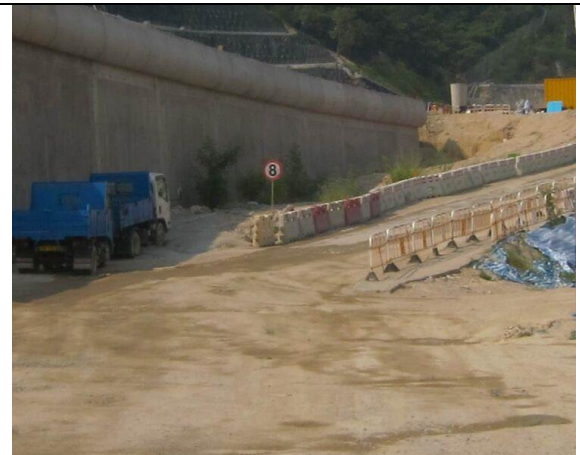
Photo 6 Set speed control at ~8km/hr for all vehicles using the haul road
