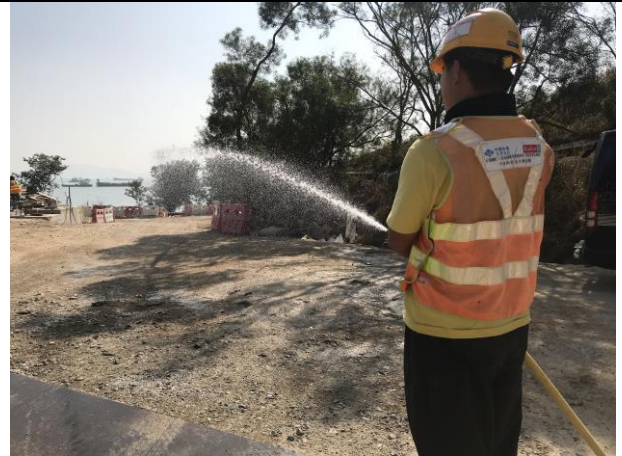
Photo 2 Water spraying by worker for un-accessible area.
