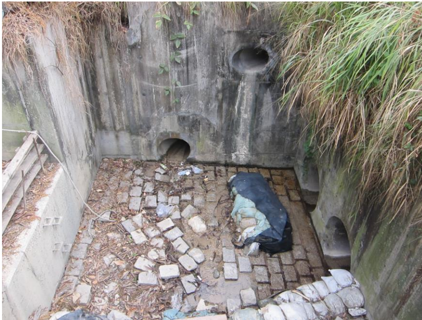
Stream B Outfall: No water is discharging.
