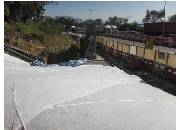
Photo 4 Hydro seeding for the exposed slope at slop 170
