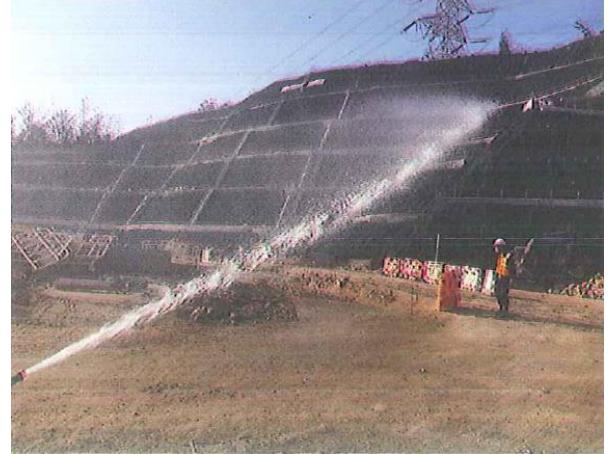
Photo 2 Water spraying by worker for un-accessible area.
