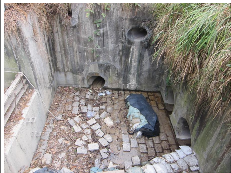
Stream B Outfall: No water is discharging.
