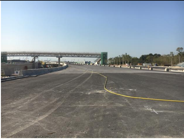
Photo 13 Road pavement works at Platform 19
