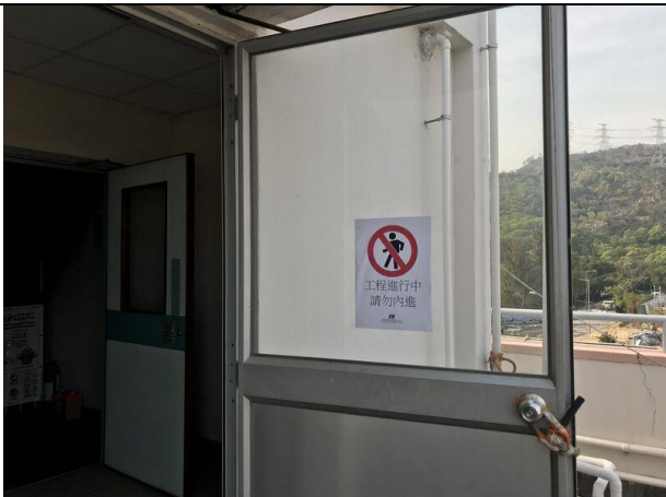
Photo 17 Photo taken on 6 February 2018 at the roof top of Pillar Point Fire Station
