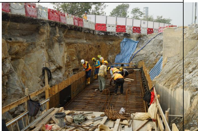
Photo 12 Construction of drainage a Portion H
