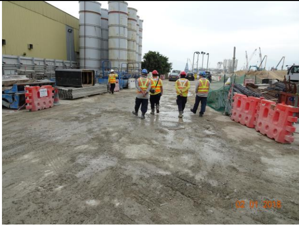
Photo 7 Watering of haul road to keep road surface wet was observed during the joint site inspection on 2 January 2018
