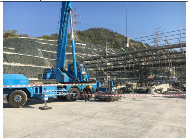
Photo 12 Construction of Canopy at TD1
