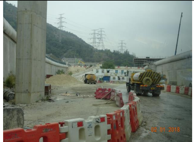
Photo 10 Watering of haul road by water truck to keep road surface wet was observed during the site inspection on 2 January 2018
