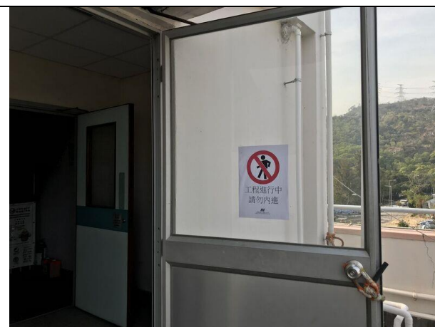
Photo 16 Photo taken on 6 February 2018 at the roof top of Pillar Point Fire Station
