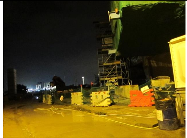
Night Condition at Portion F on 30 January 2018 10:00 pm
