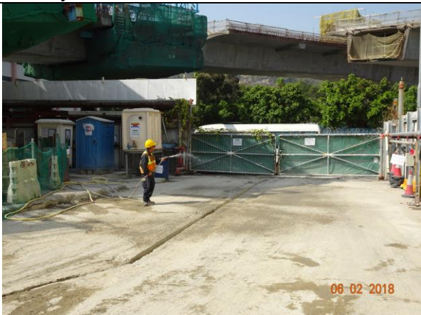
Photo 11 Watering of haul road to keep road surface wet was observed during the site inspection on 6 February 2018
