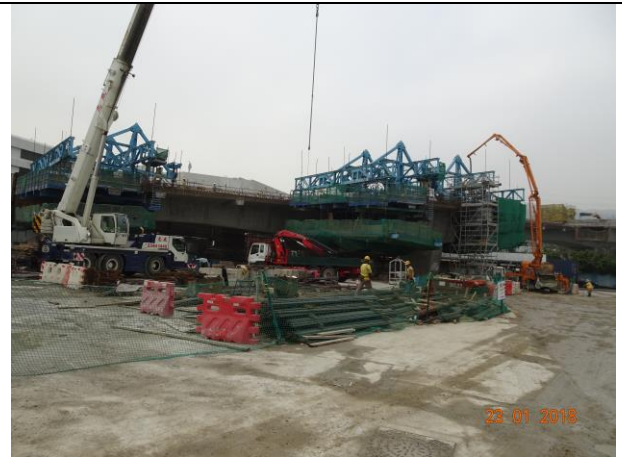
Most construction area at Portion F was hard paved
