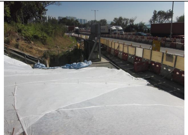
Photo 4 Hydro seeding for the exposed slope at slop 170
