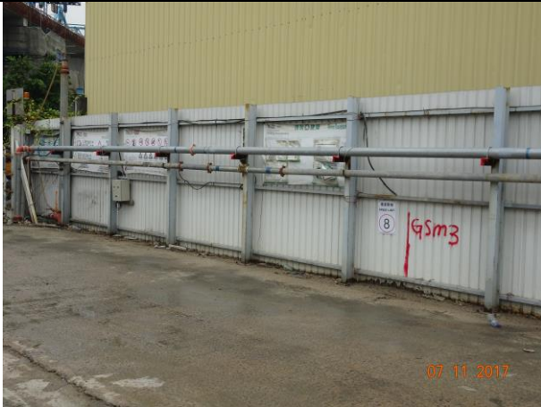
Photo 9 Set speed control at ~8km/hr for all vehicles using the haul road at Portion F
