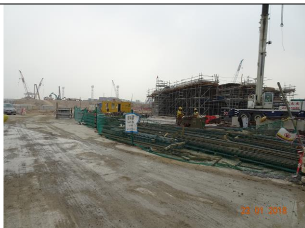
Photo 9 Site area keeping wet was observed at Portion F during the join site inspection on 23 January 2018
