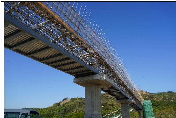
Photo 15 Construction of bamboo scaffolding at footbridge
