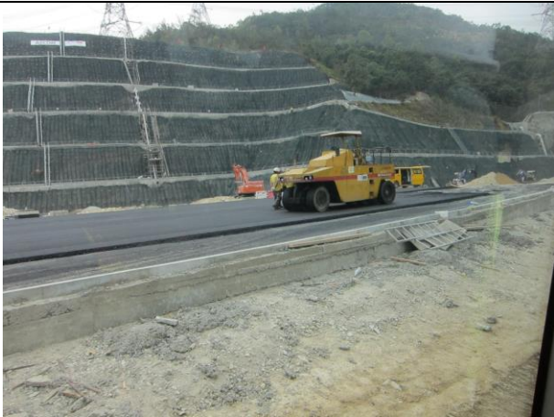
Photo 15 Road pavement works at Platform 19
