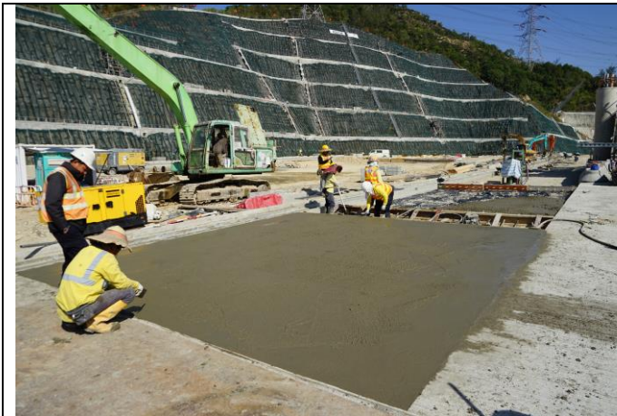
Photo 13 Road pavement works at Platform 19
