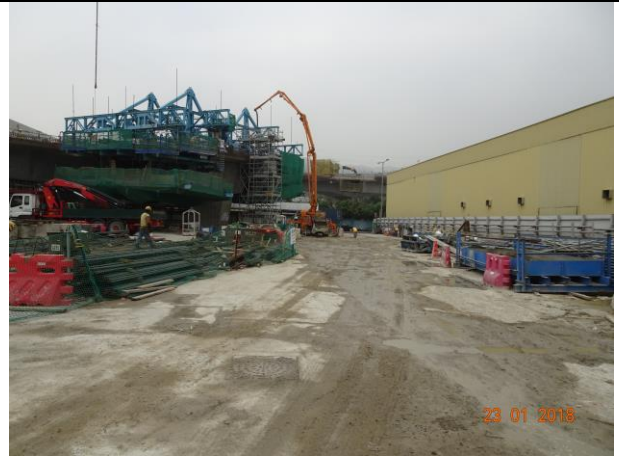
Keeping road surface wet to reduce dust impact at Portion F was observed during the weekly site inspection on 23 January 2018
