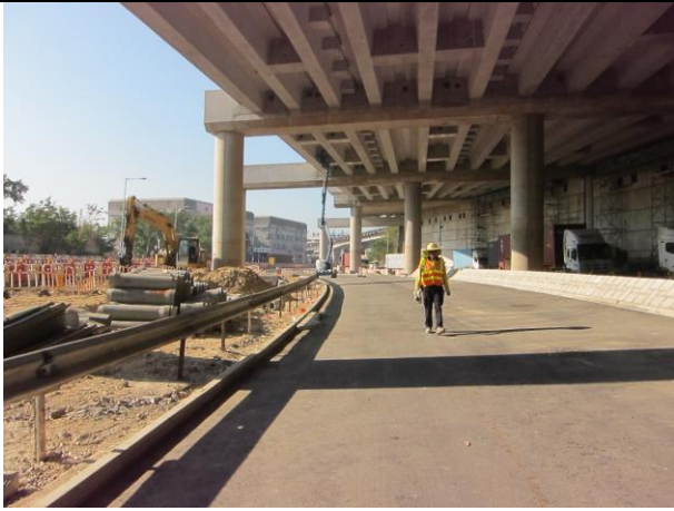
Photo 13 Housekeeping works at LMR
