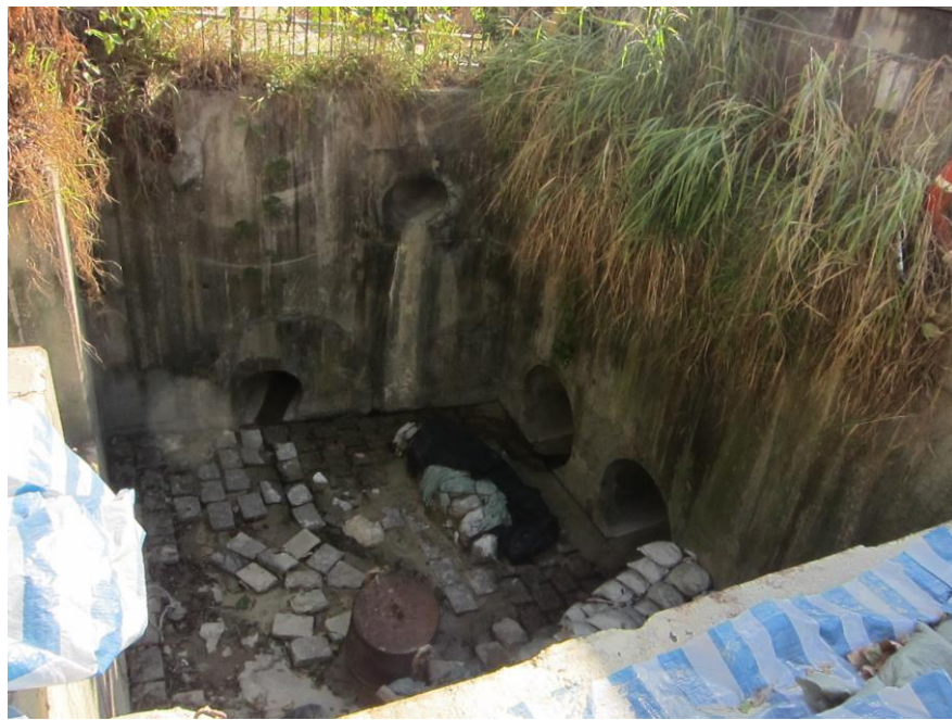
Stream B Outfall: No water is discharging.
