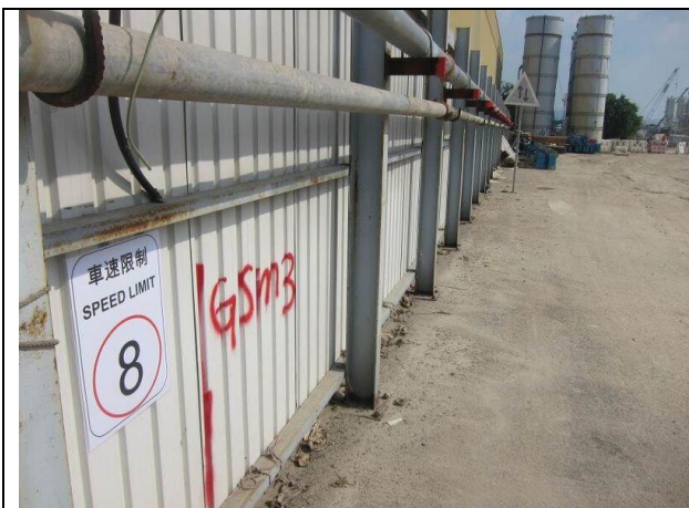
Photo 7 Set speed control at ~8km/hr for all vehicles using the haul road at Portion F
