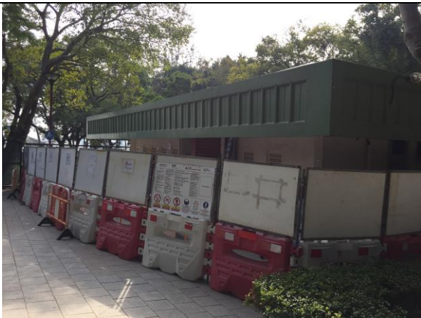
Photo 17 Construction works was undertaken at public toilet near the ASR10
