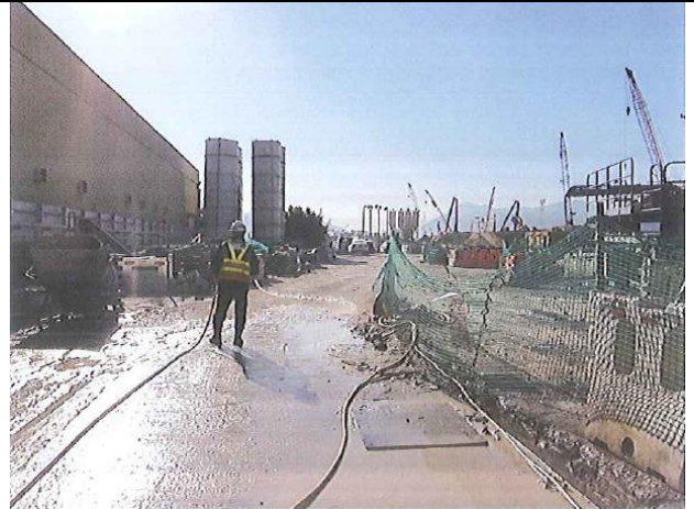
Photo 2 Water spraying by worker for un-accessible area.
