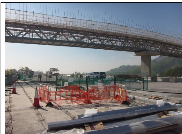
Photo 13 Construction of bamboo scaffolding at footbridge
