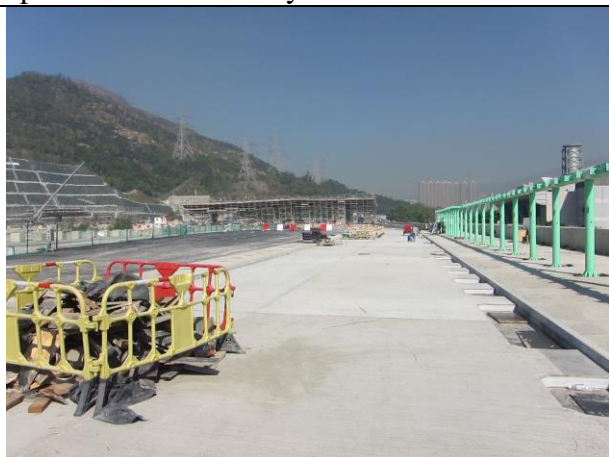
Photo 11 Road pavement works at Platform 19
