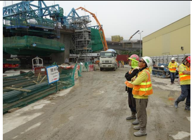
Photo 10 Site area keeping wet was observed at Portion F during the join site inspection on 16 January 2018
