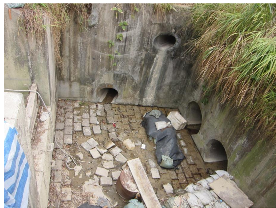
Stream B Outfall: No water is discharging.
