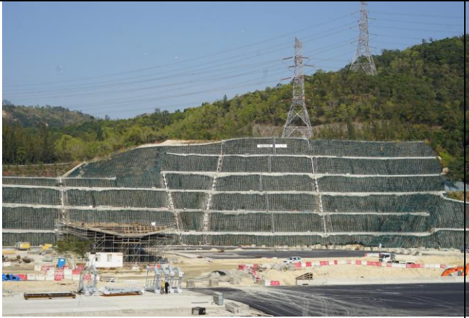
Photo 13 Road pavement works at Platform 19
