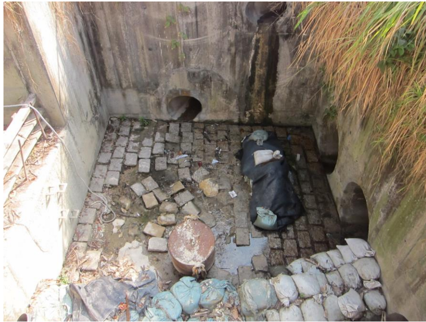
Stream B Outfall: No water is discharging.
