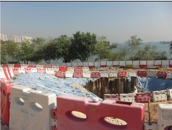
Photo 5 Covered part of the exposed slopes and stockpile by tarpaulin sheet.
