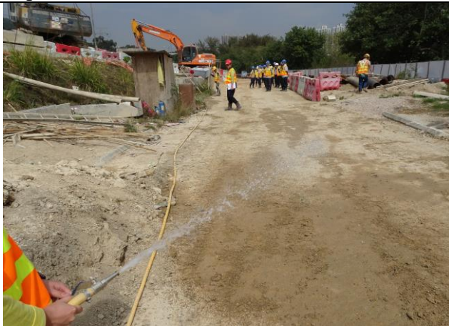
Photo 3 Water spraying by worker for un-accessible area.
