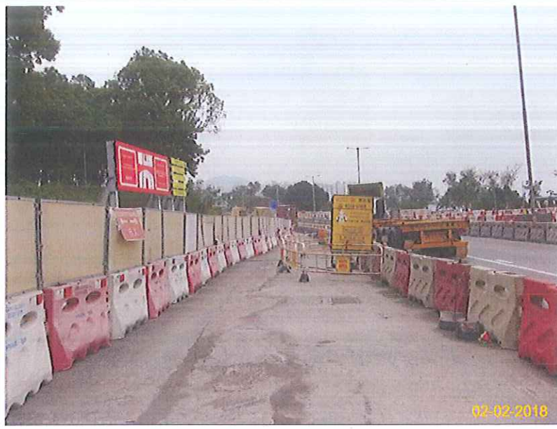
Item 5. Hoarding with panel around works area & Item 6. Temporary traffic management lighting.
