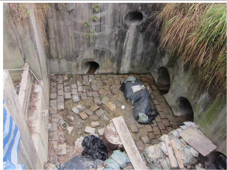
Stream B Outfall: No water is discharging.
