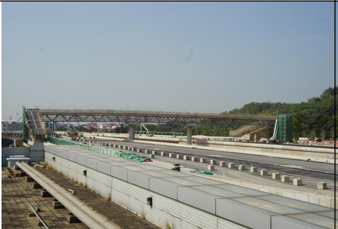
Photo 15 Construction of canopy at TD1
