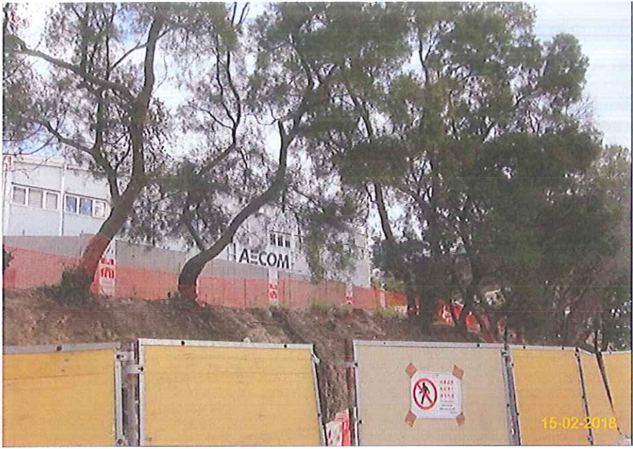
Item 1. Existing trees on boundary of the Project Area should be protected carefully during construction.
