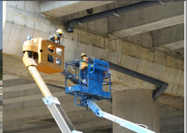
Photo 16 Construction of drainage at Lung Mun Road
