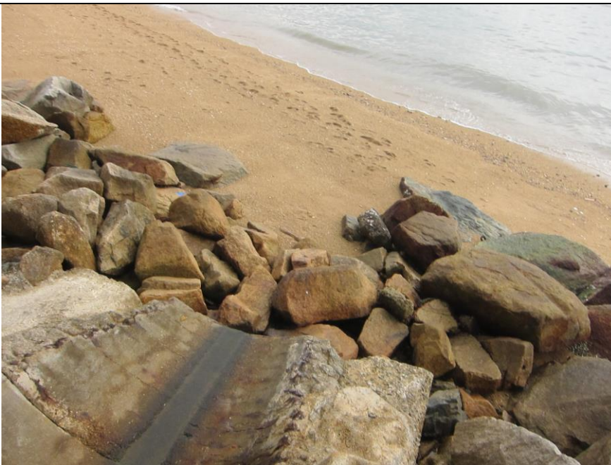
Outfall 1: No water is discharging.
