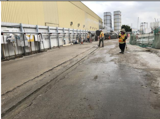
Photo 3 Water spraying by worker for un-accessible area.
