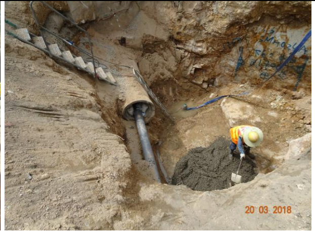
Photo 14 Drainage works at Underpass
