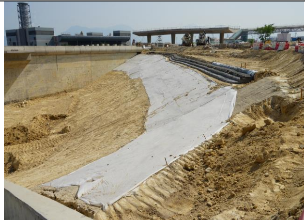
Photo 4 Hydro seeding for the exposed slope
