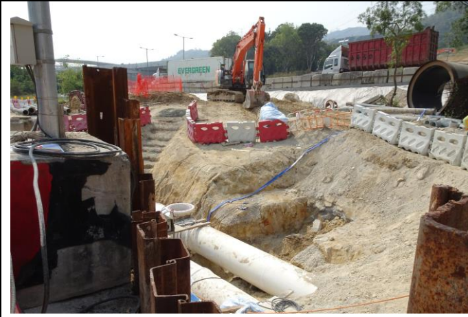
Photo 13 Drainage works at Portion H
