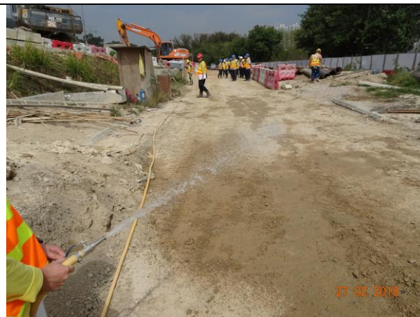
Photo 8 Site area keeping wet was observed at Portion H during the join site inspection on 27 February 2018
