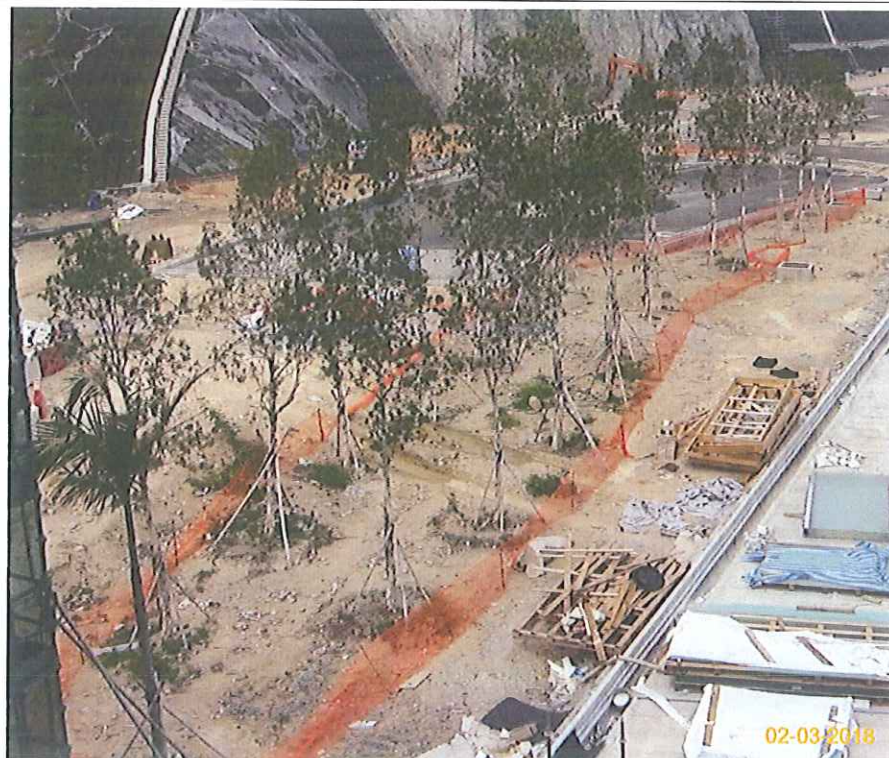
Item 2. Tree Transplanting works conducted on 22-May-17.
