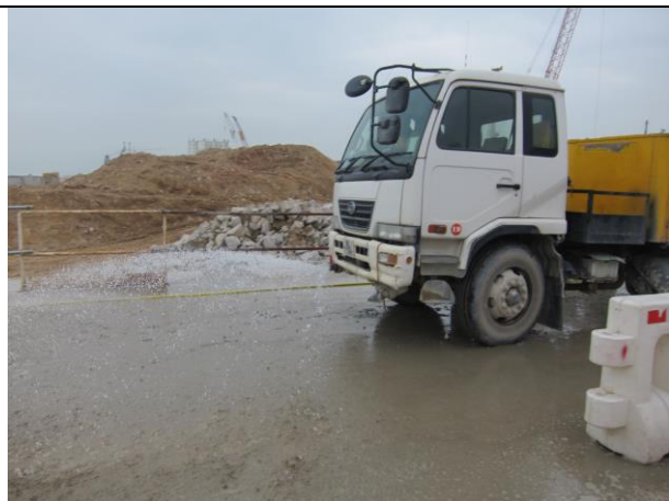
Photo 11 Water spraying for exposed area and stockpile at Portion F
