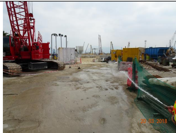
Photo 8 Site area keeping wet was observed at Portion F during the join site inspection on 20 March 2018
