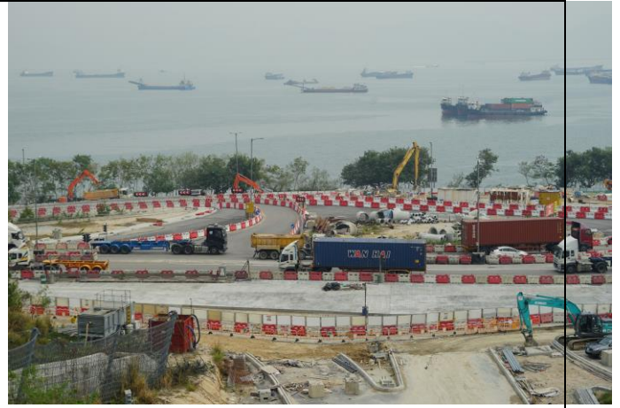
Photo 14 Temporary traffic arrangement at Lung Mun Road.
