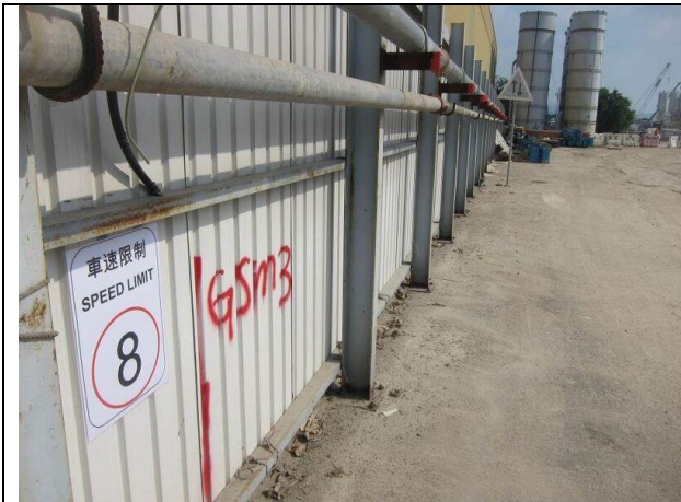
Photo 7 Set speed control at ~8km/hr for all vehicles using the haul road at Portion F
