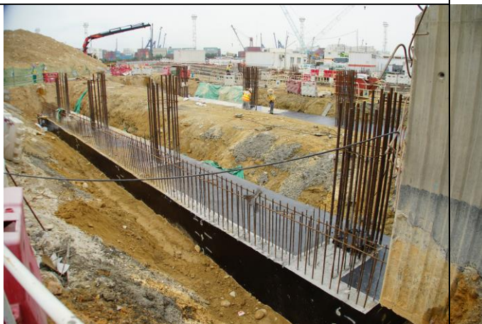
Photo 12 Construction of pile cap at Portion F
