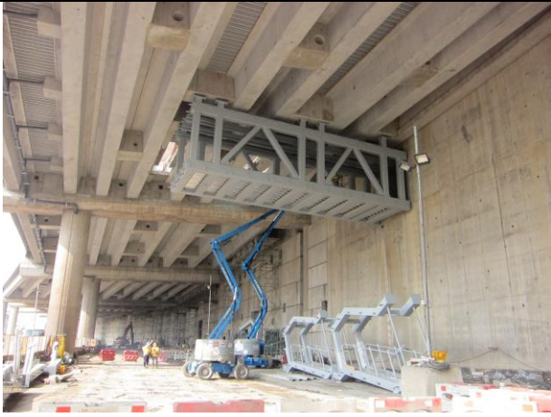
Photo 13 Construction of storage area at Retaining Wall B
