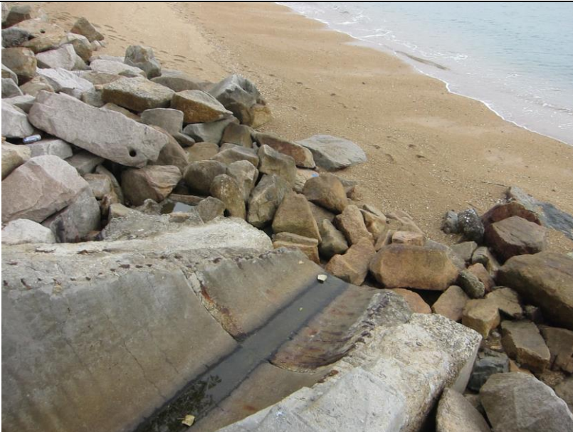
Outfall 1: No water is discharging.
