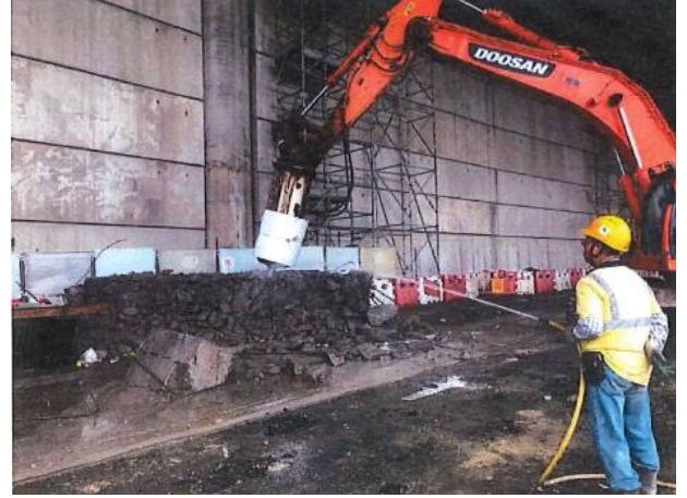
Photo 2 Water spraying by worker for un-accessible area.
