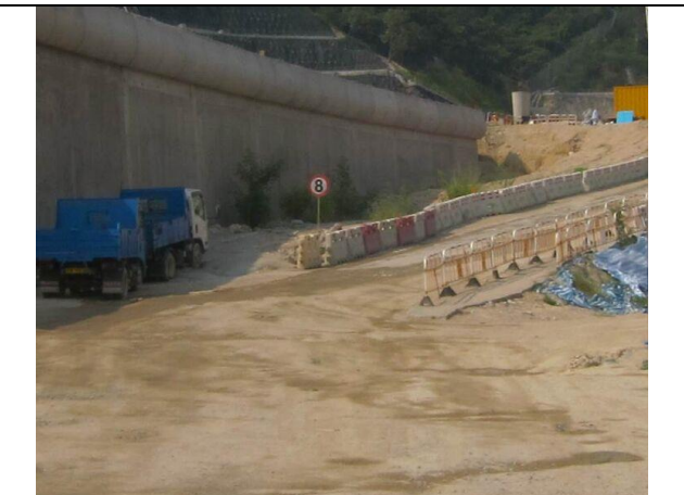
Photo 6 Set speed control at ~8km/hr for all vehicles using the haul road
