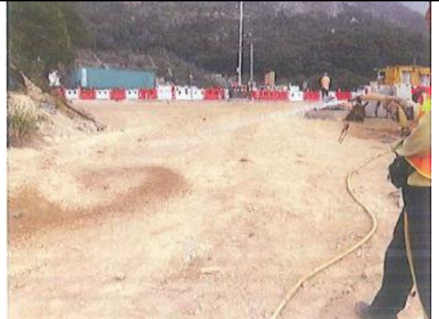
Photo 2 Water spraying by worker for un-accessible area.
