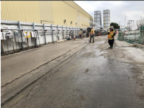
Photo 3 Water spraying by worker for un-accessible area.
