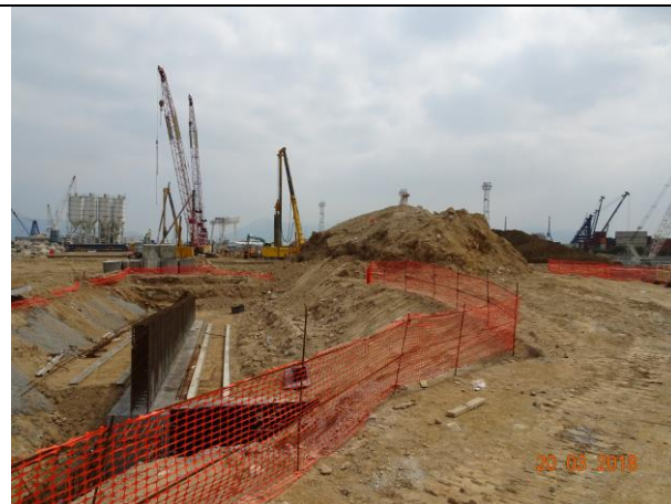
Photo 10 Construction of pile cap at Portion F
