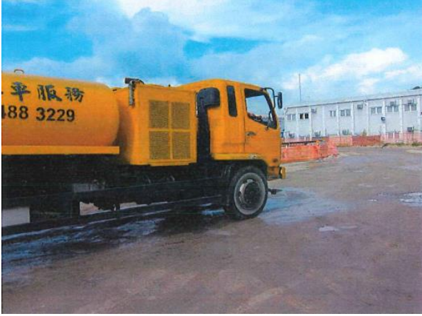
Photo 1 Watering of haul road by water truck to keep road surface wet
