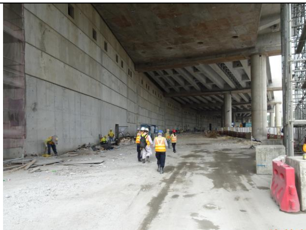
Photo 12 Construction of storage area at Retaining Wall B
