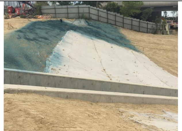
Photo 4 Hydro seeding for the exposed slope at Retaining Wall B
