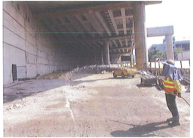
Photo 2 Water spraying by worker for un-accessible area.
