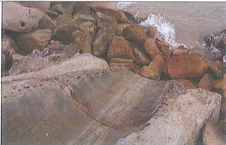
Outfall 1: No water is discharging.
