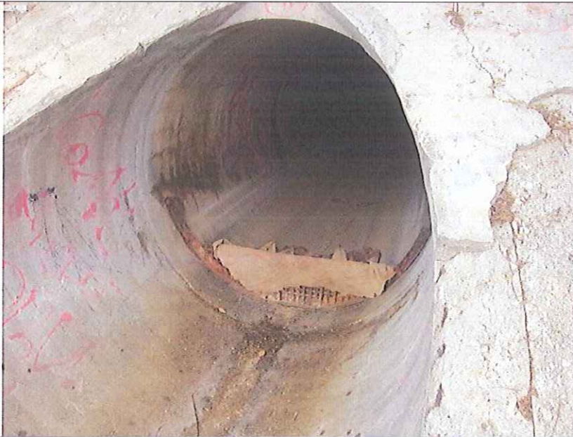
Outfall 1: No water is discharging.
