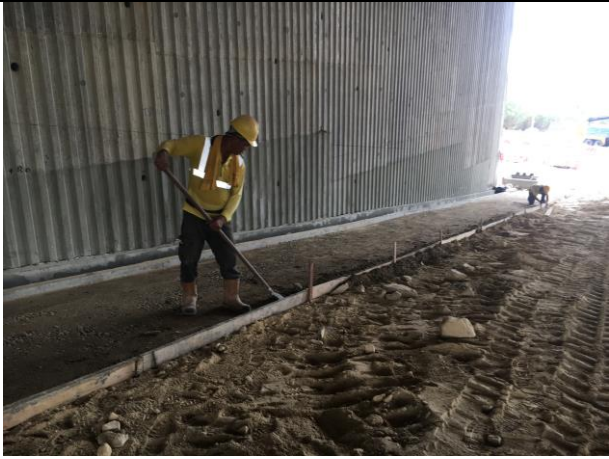
Photo 13 Drainage works at Platform 19
