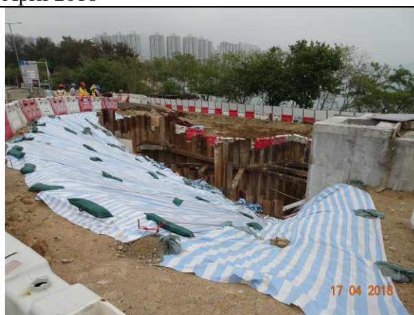
Photo 10 Dust mitigation measure was observed at Portion H during the join site inspection on 17 April 2018
