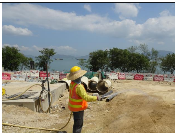
Photo 8 Site area keeping wet was observed at Portion H during the join site inspection on 10 April 2018
