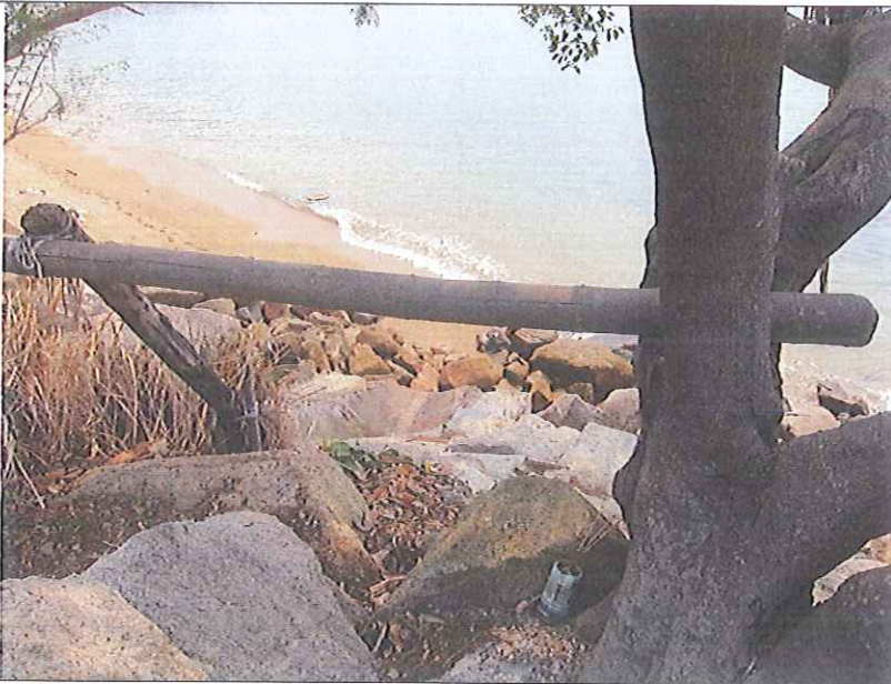
Outfall 1: No water is discharging.
