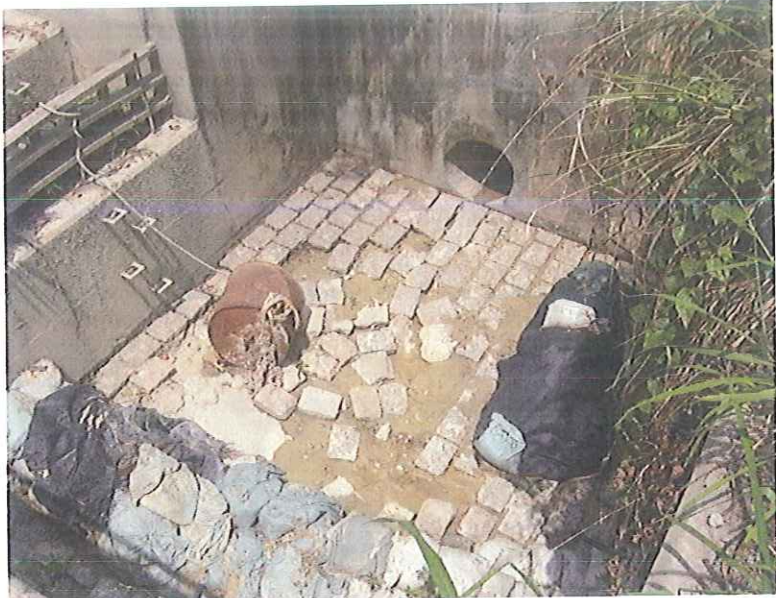
Stream B Outfall: No water is discharging.
