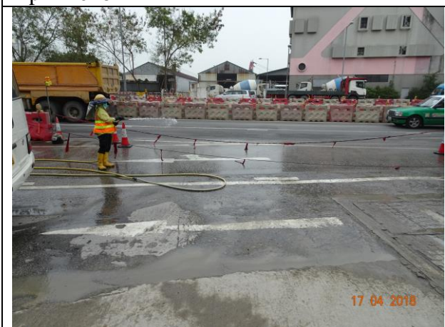
Photo 11 Dust mitigation measure was observed at Lung Mun Road during the join site inspection on 17 April 2018
