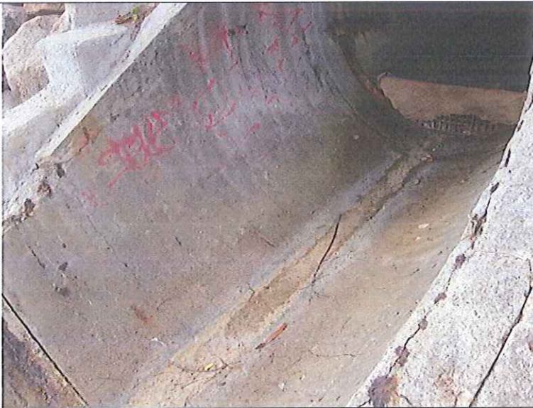
Outfall 1: No water is discharging.
