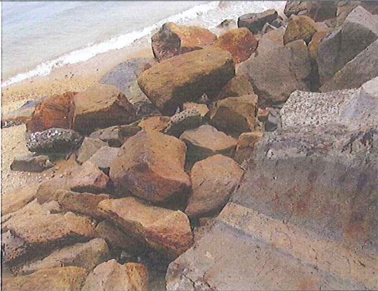
Outfall 1: No water is discharging.
