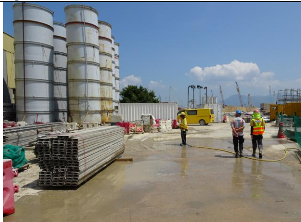
Photo 3 Water spraying by worker for at Portion F.
