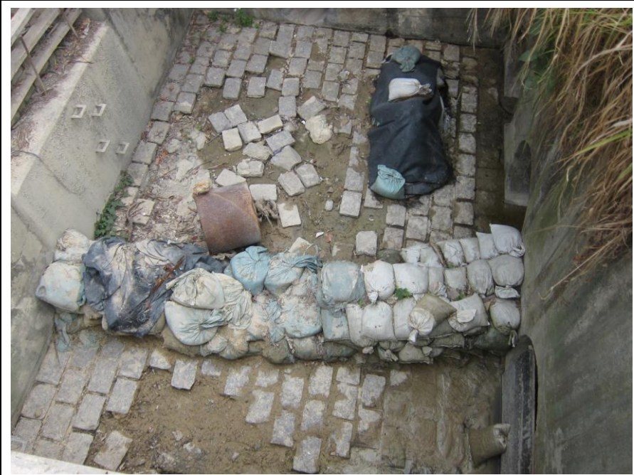
Stream B Outfall: No water is discharging.
