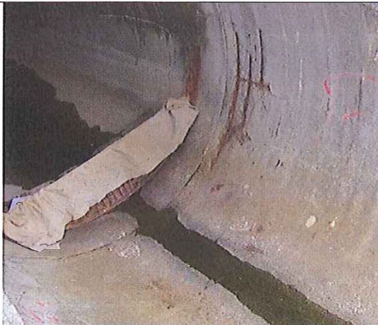
Outfall 1: Clean water is discharging.
