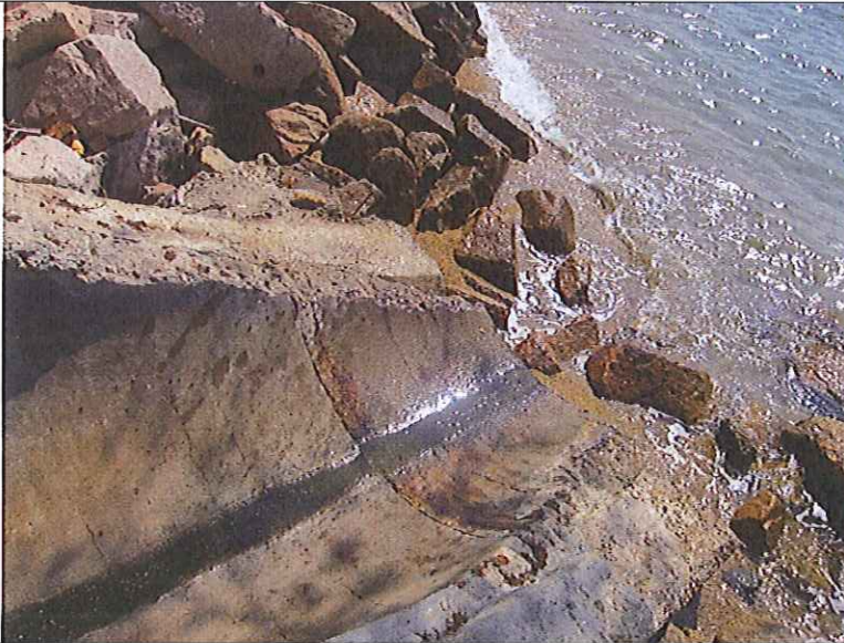
Outfall 1: Clean water is discharging.
