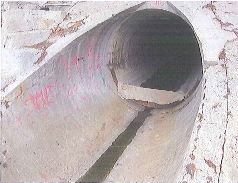
Outfall 1: No water is discharging.
