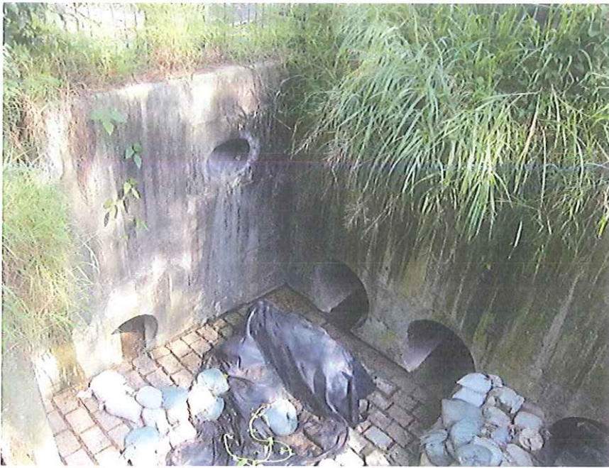
Stream B Outfall: No water is discharging.
