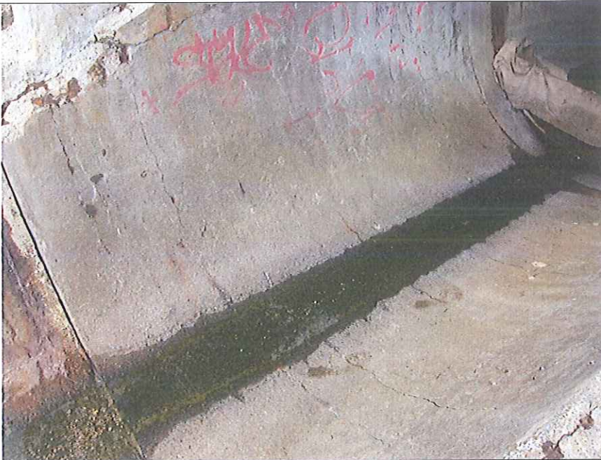
Outfall 1: No water is discharging.
