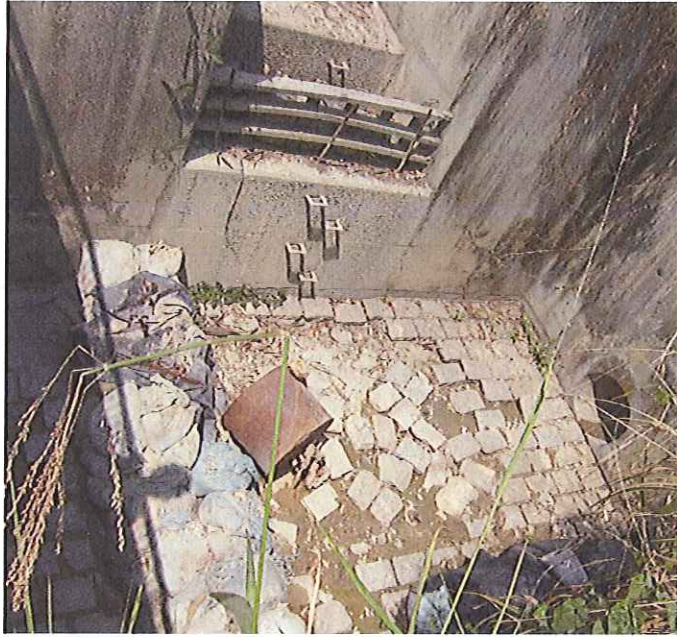
Stream B Outfall: No water is discharging.
