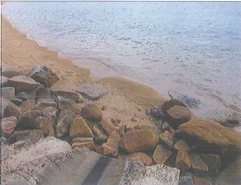
Outfall 1: No water is discharging.
