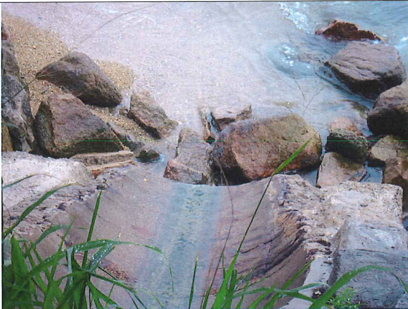
Outfall 1: Clean water is discharging.
