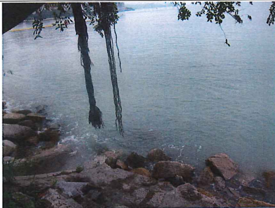
Outfall 1: Clean water is discharging.
