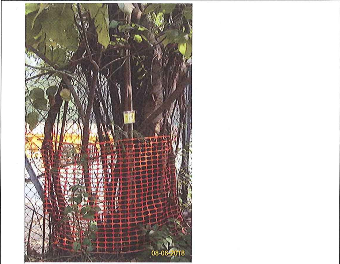
Item 1. Existing trees on boundary of the Project Area should be protected carefully during construction.
