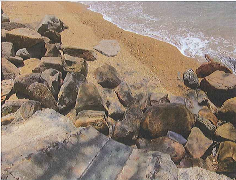
Outfall 1: Clean water is discharging.
