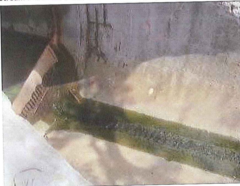
Outfall 1: Clean water is discharging.
