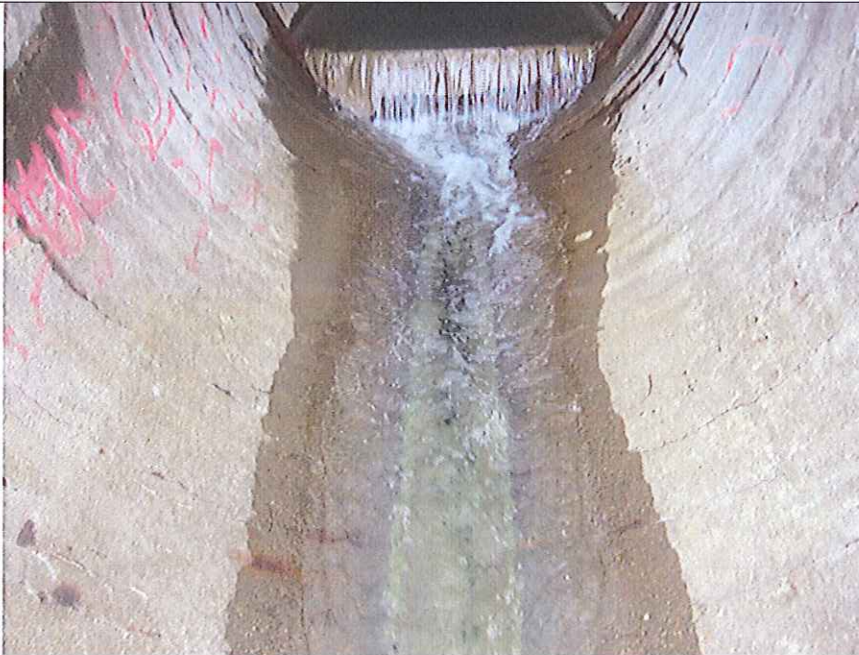
Outfall 1: Clean water is discharging.
