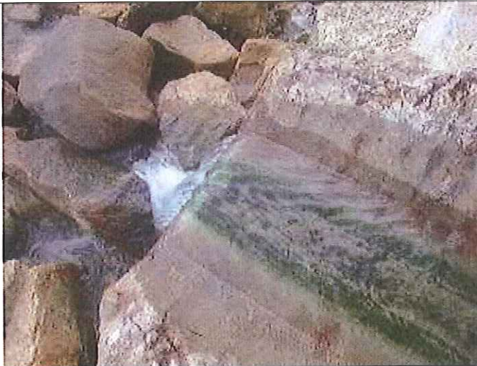
Outfall 1: Clean water is discharging.
