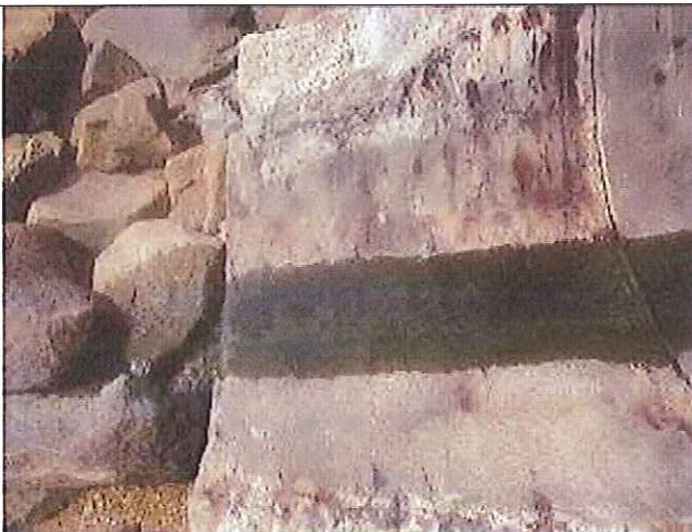
Outfall 1: Clean water is discharging.
