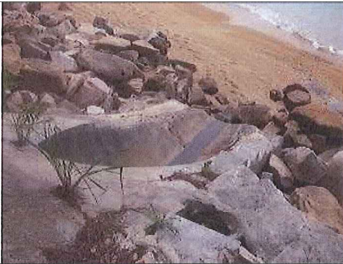
Outfall 1: Clean water is discharging.
