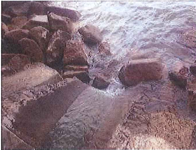
Outfall 1: Clean water is discharging.
