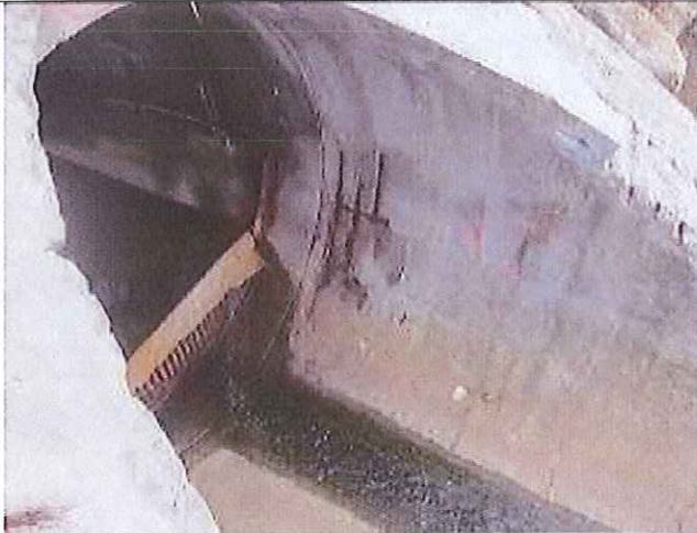
Outfall 1: Clean water is discharging.
