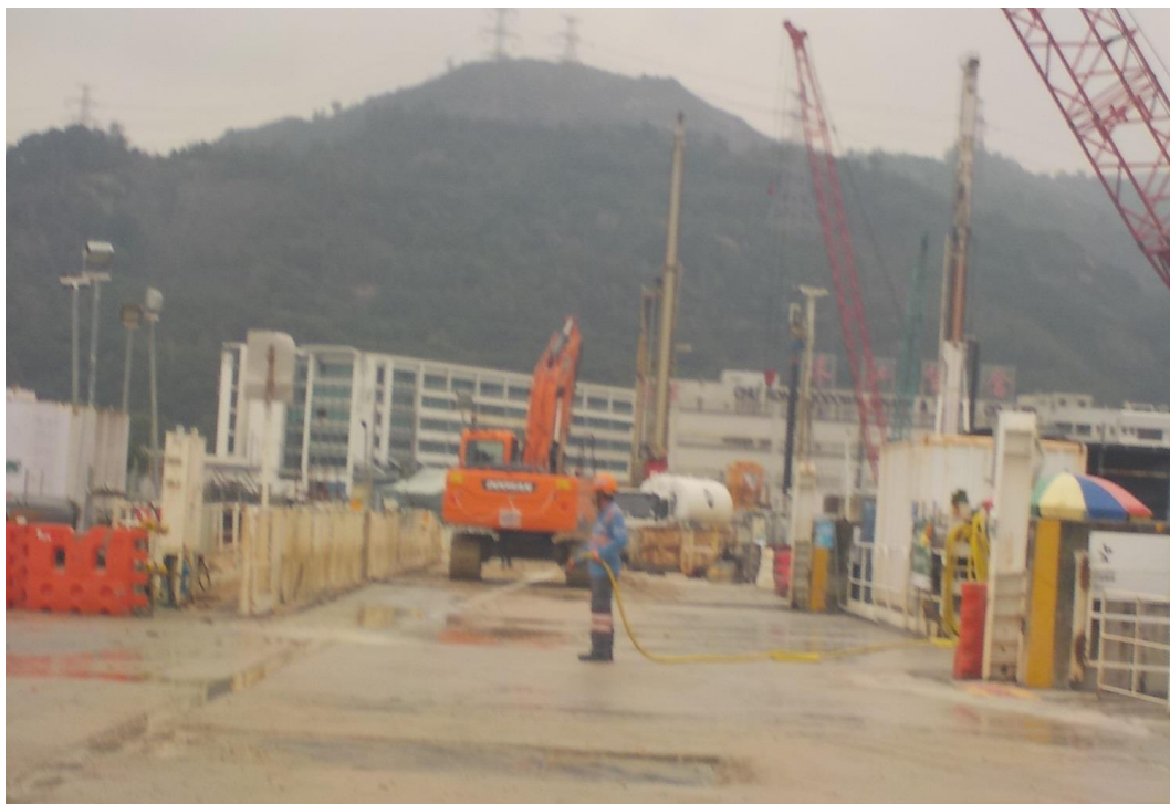
Water spraying was applied frequently on site. (Works Area Portion N-A)
