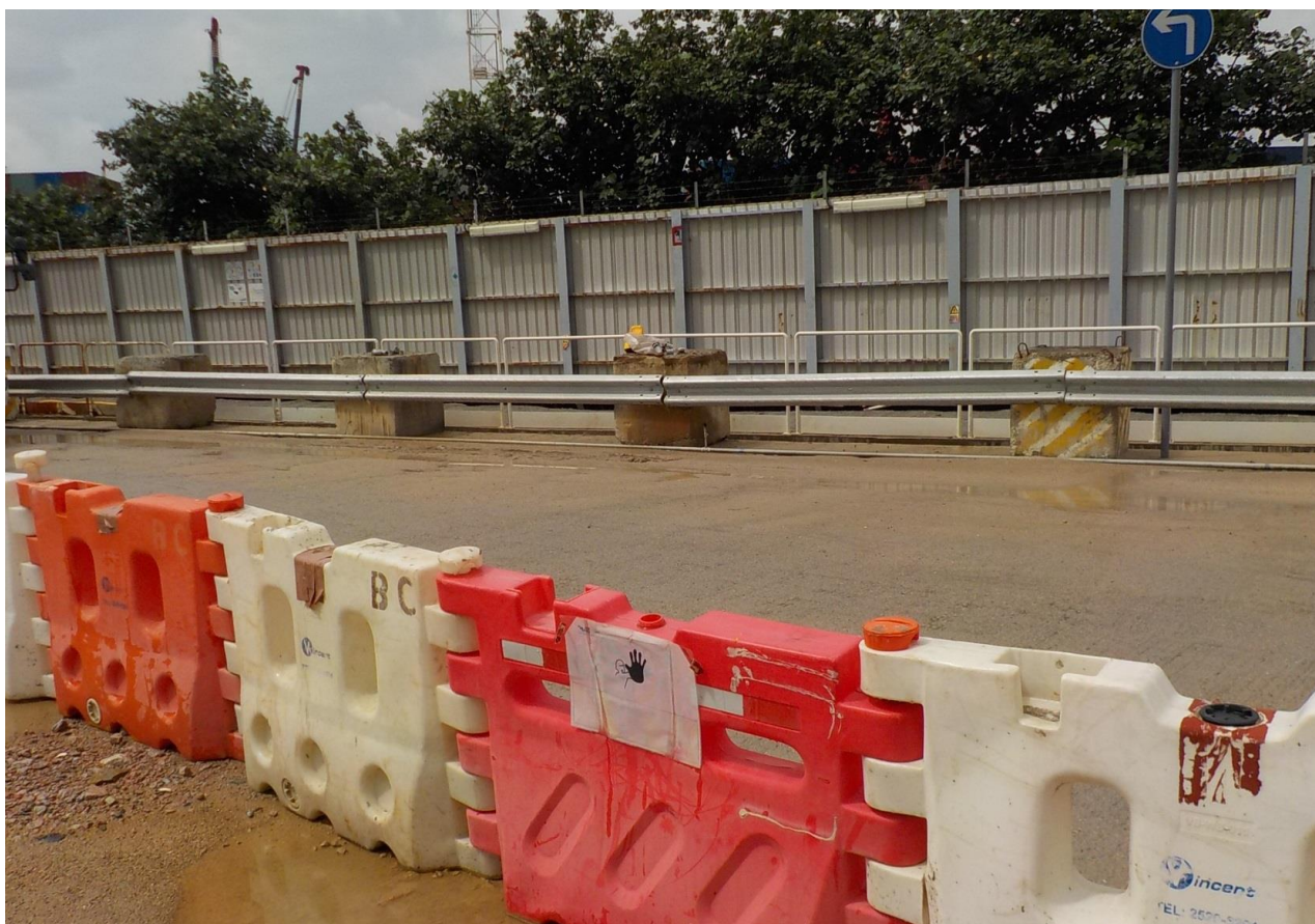
Water spraying was applied to prevent dust.
