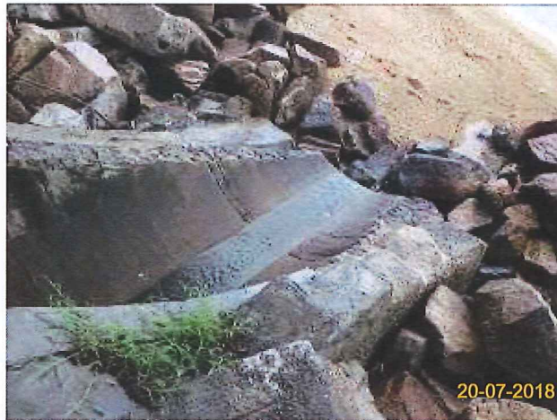
Item 7. Ensure no run-off into water body.(Outfall 1)
