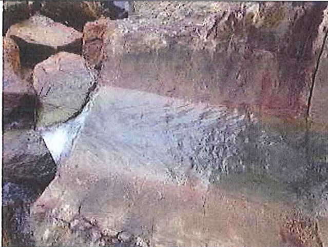
Outfall 1: Clean water is discharging.
