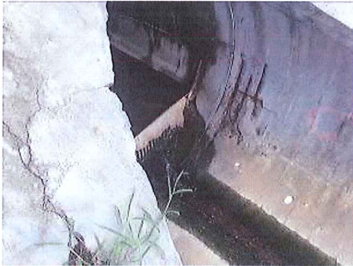
Outfall 1: Clean water is discharging.
