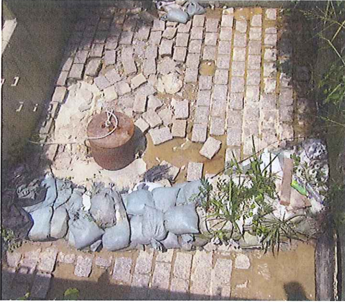
Stream B Outfall: Clean water is discharging.
