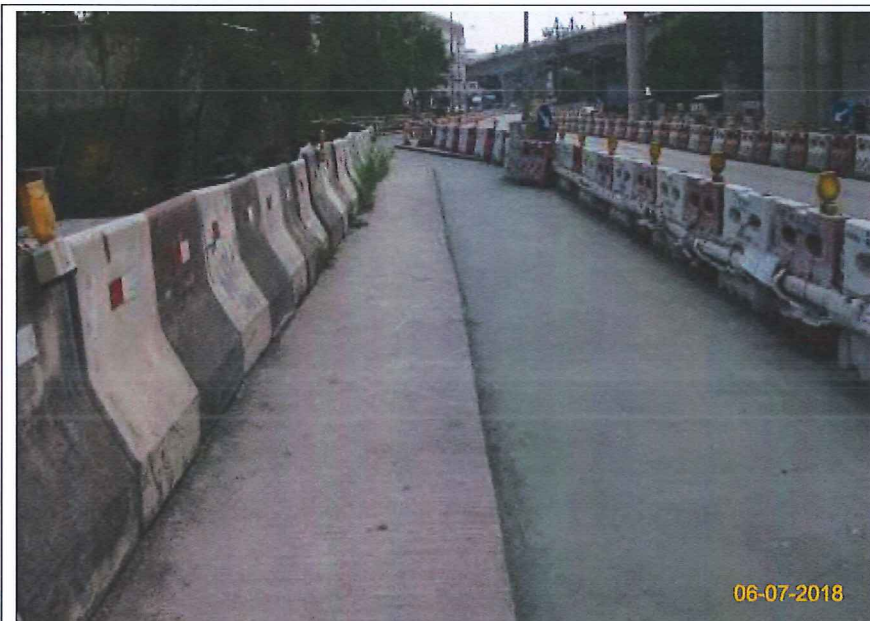
Item 5. Hoarding with panel around works area & Item 6. Temporary traffic management lighting.
