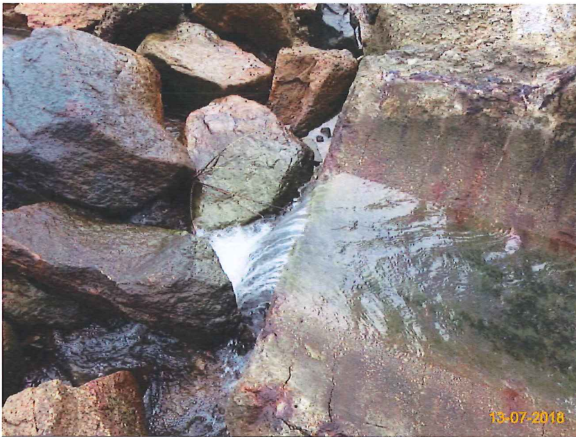
Item 7. Ensure no run-off into water body.(Outfall 1)
