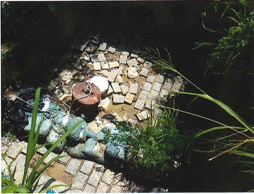
Stream B Outfall: No water is discharging.
