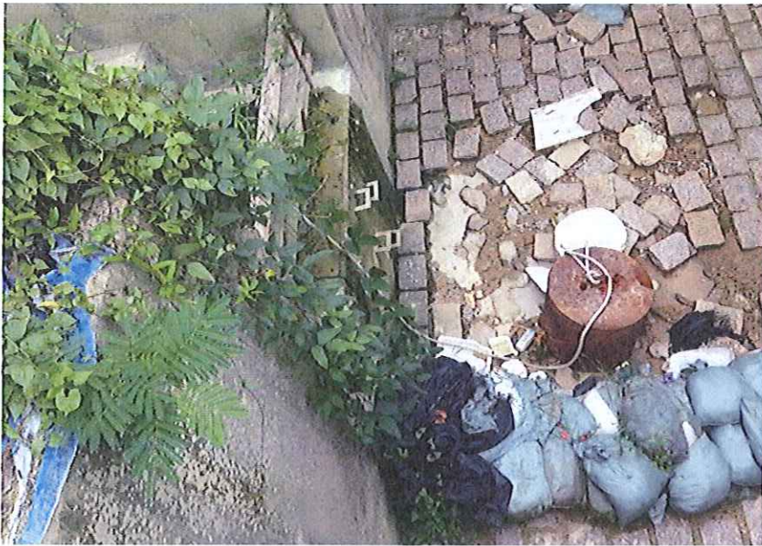
Stream B Outfall: Clean water is discharging.
