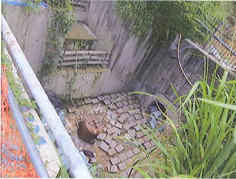
Stream B Outfall: No water is discharging.
