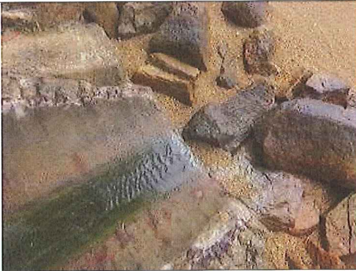
Outfall 1: Clean water is discharging.
