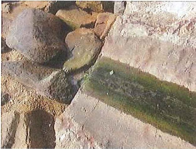
Outfall 1: Clean water is discharging.
