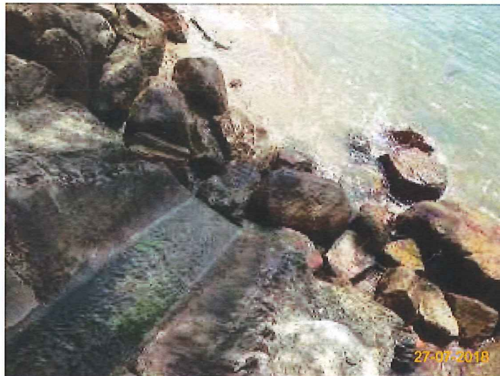
Item 7. Ensure no run-off into water body.(Outfall 1)
