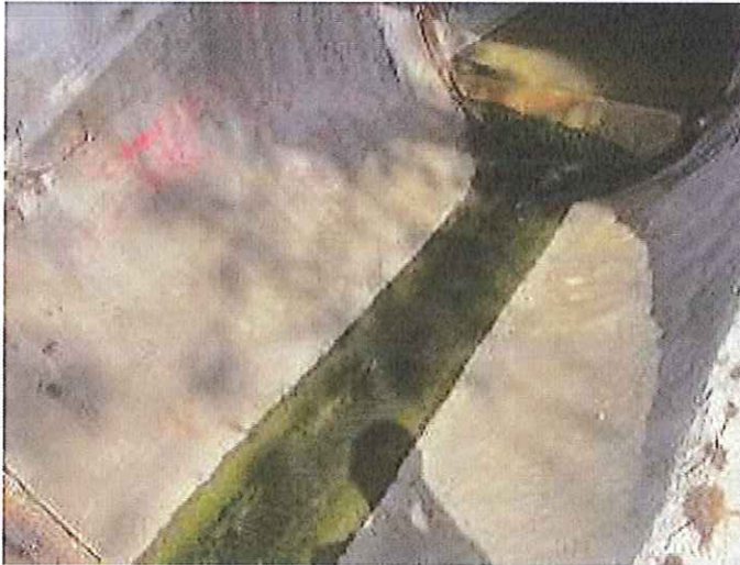
Outfall 1: Clean water is discharging.
