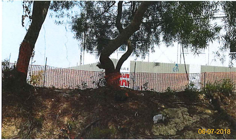
Item 1. Existing trees on boundary of the Project Area should be protected carefully during construction.
