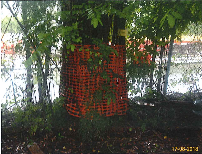
Item 1. Existing trees on boundary of the Project Area should be protected carefully during construction.
