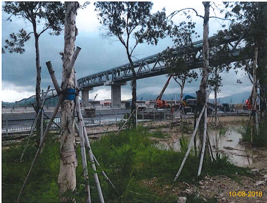
Item 2. Tree Transplanting works conducted on 22-May-17.
