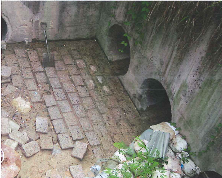
Stream B Outfall: Clean water is discharging.
