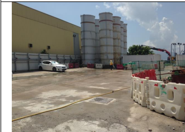
Photo 11 Water spraying by worker at Portion F during normal construction day.
