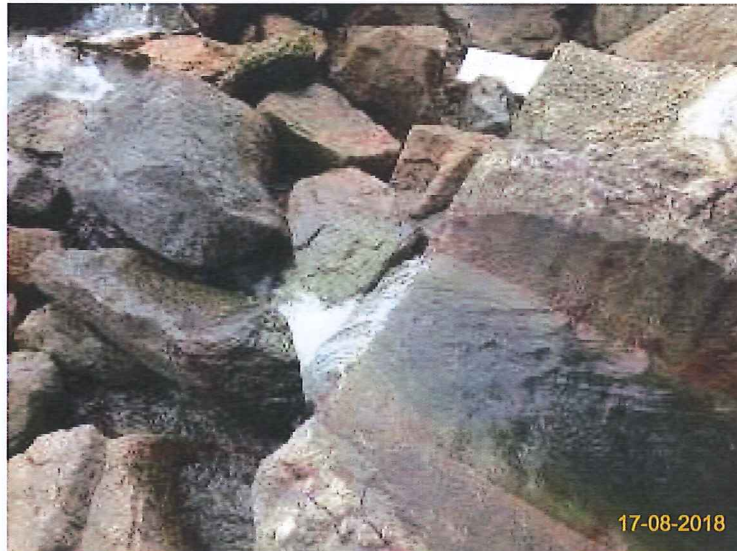
Item 7. Ensure no run-off into water body.(Outfall 1)
