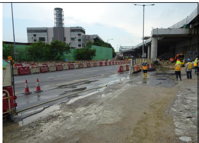
Photo 8 Dust mitigation measure was observed at Lung Mun Road during the joint site inspection on 28 August 2018.
