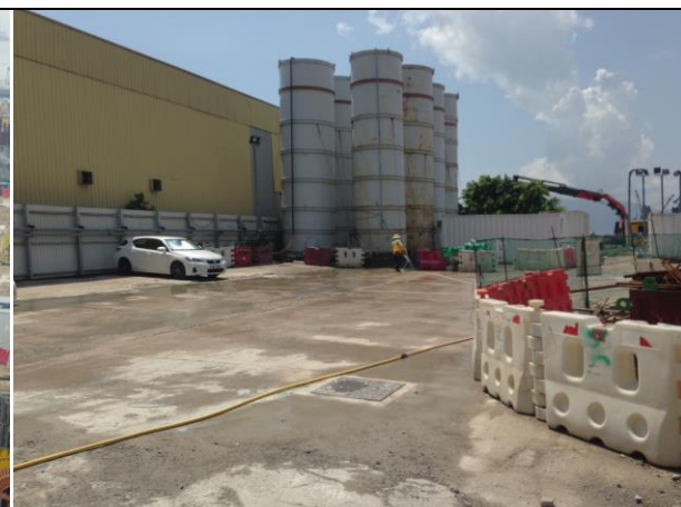
Photo 12 Water spraying by worker at Portion F during normal construction day.
