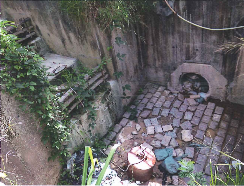
Stream B Outfall: Clean water is discharging.
