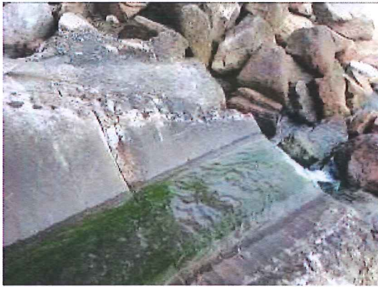
Outfall 1: Clean water is discharging.
