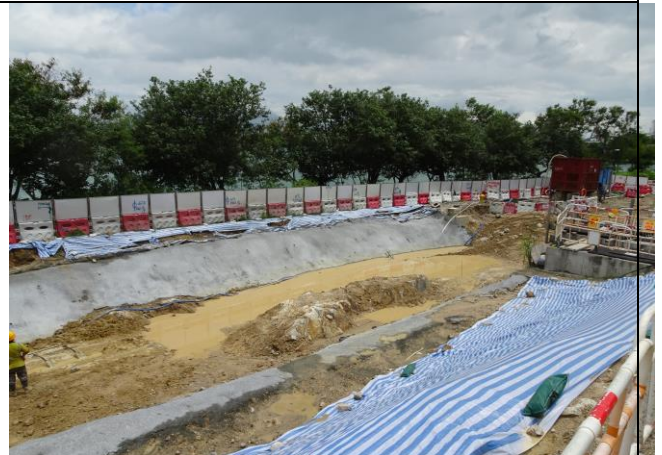
Photo 4 Covered part of the exposed slopes and stockpile by tarpaulin sheet.
