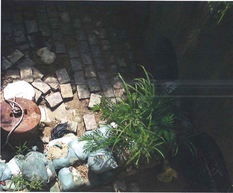
Stream B Outfall: Clean water is discharging.
