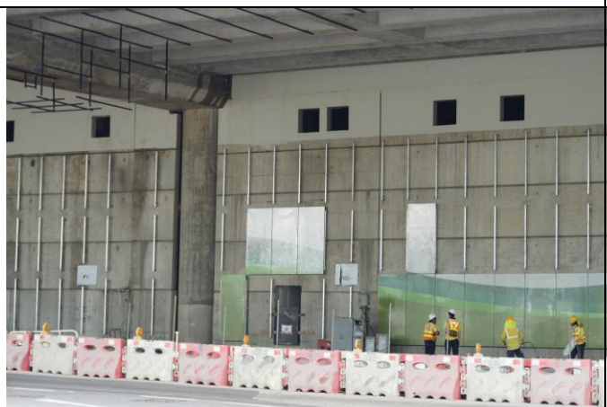
Photo 9 Installation of VE panels at Retaining Wall B
