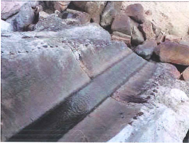
Outfall 1: Clean water is discharging.
