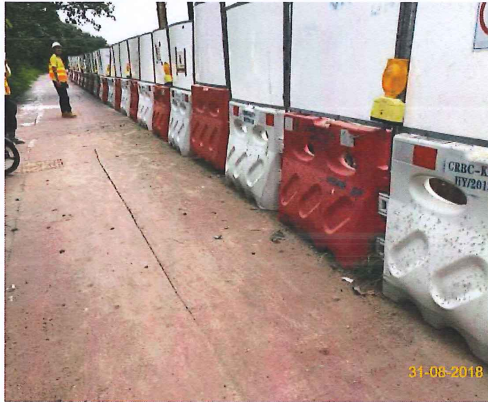
Item 5. Hoarding with panel around works area & Item 6. Temporary traffic management lighting.
