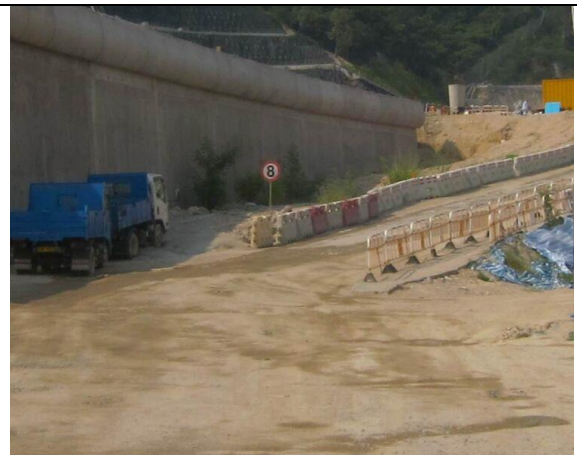
Photo 6 Set speed control at ~8km/hr for all vehicles using the haul road
