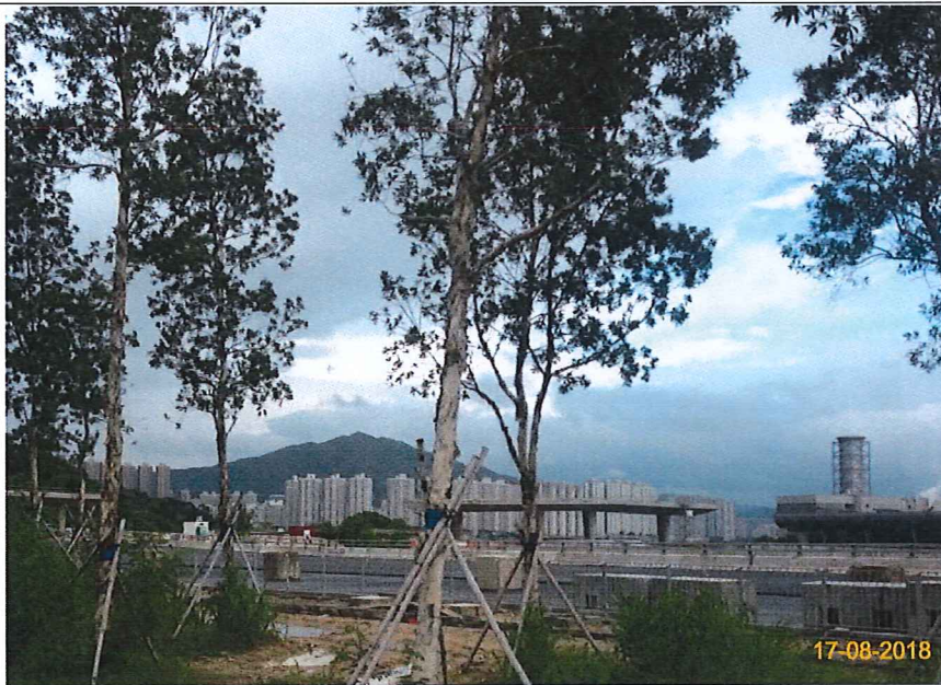
Item 2. Tree Transplanting works conducted on 22-May-17.
