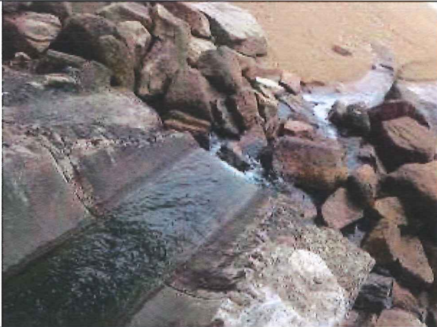
Outfall 1: Clean water is discharging.
