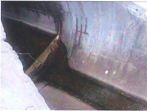
Outfall 1: Clean water is discharging.
