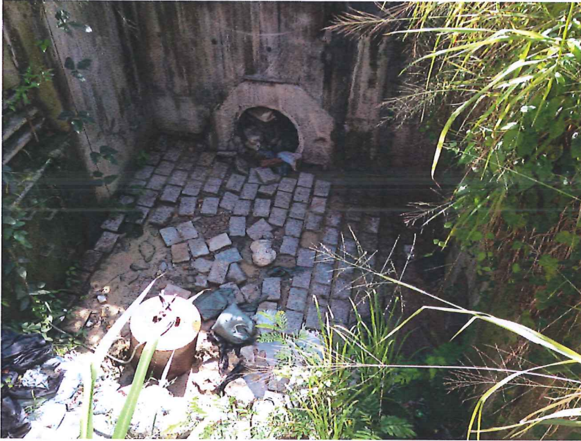
Stream B Outfall: No water is discharging.
