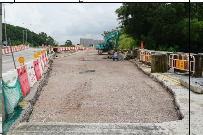
Photo 10 Drainage works at Portion H
