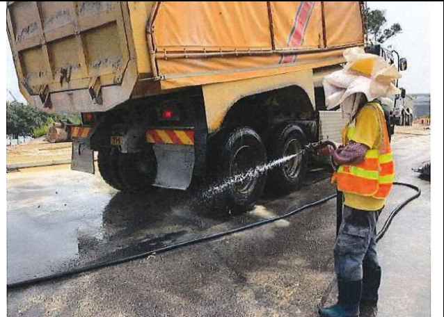
Photo 2 Water spraying by worker for un-accessible area.
