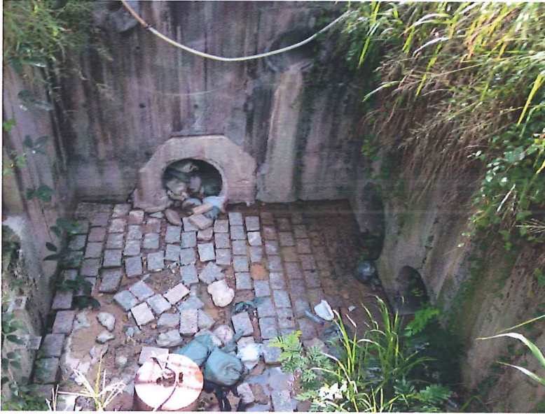
Stream B Outfall: Clean water is discharging.
