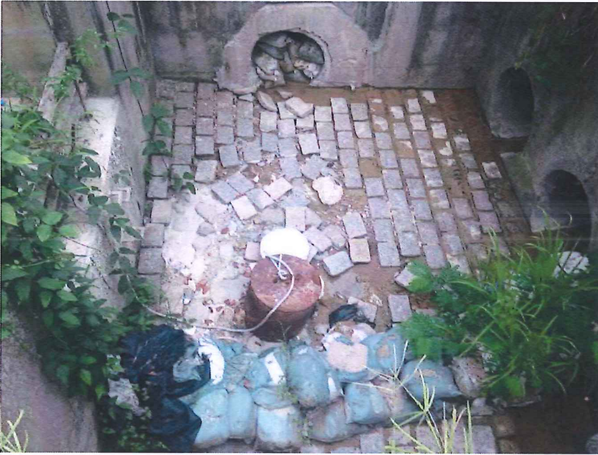
Stream B Outfall: Clean water is discharging.
