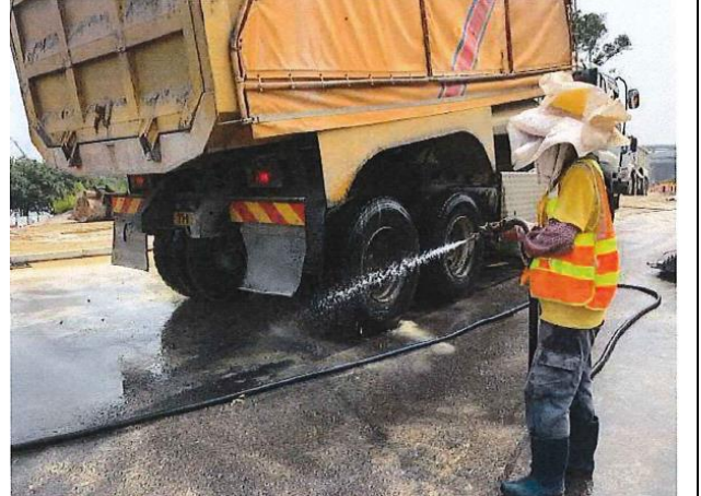
Photo 2 Water spraying by worker for un-accessible area.
