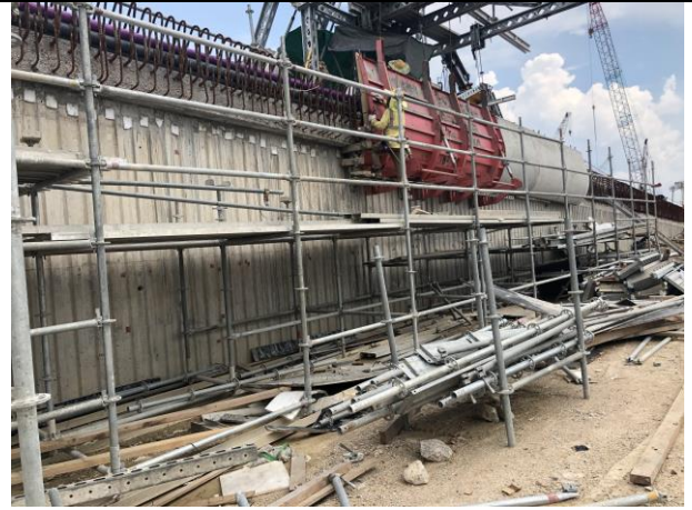
Photo 14 Construct of Parapet at Portion F
