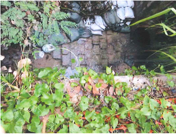
Stream B Outfall: Clean water is discharging.
