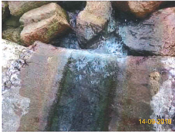
Item 7. Ensure no run-off into water body.(Outfall 1)
