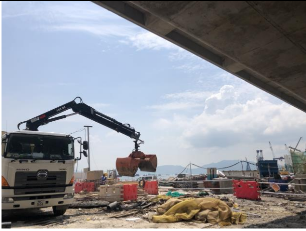
Photo 13 Housekeeping works at Portion F
