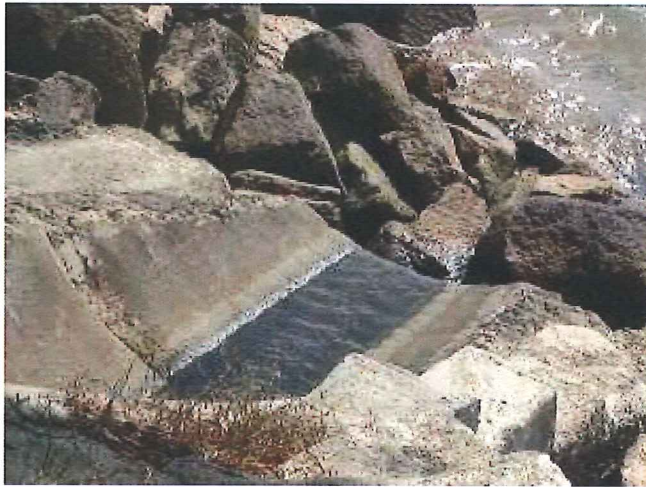
Outfall 1: Clean water is discharging.
