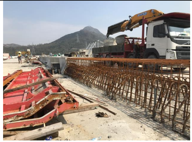
Photo 14 Construct of Parapet at Portion F
