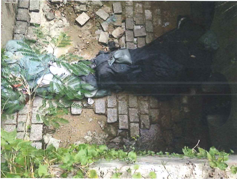
Stream B Outfall: Clean water is discharging.
