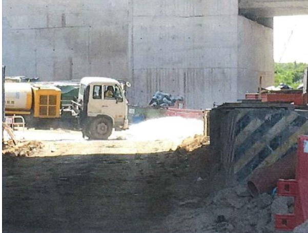
Photo 1 Watering of haul road by water truck to keep road surface wet
