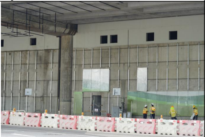
Photo 11 Installation of VE panels at Retaining Wall B
