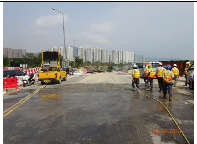
Photo 8 Dust mitigation measure was observed at site haul road during the join site inspection on 26 September 2018.
