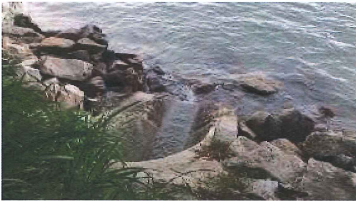
Outfall 1: Clean water is discharging.
