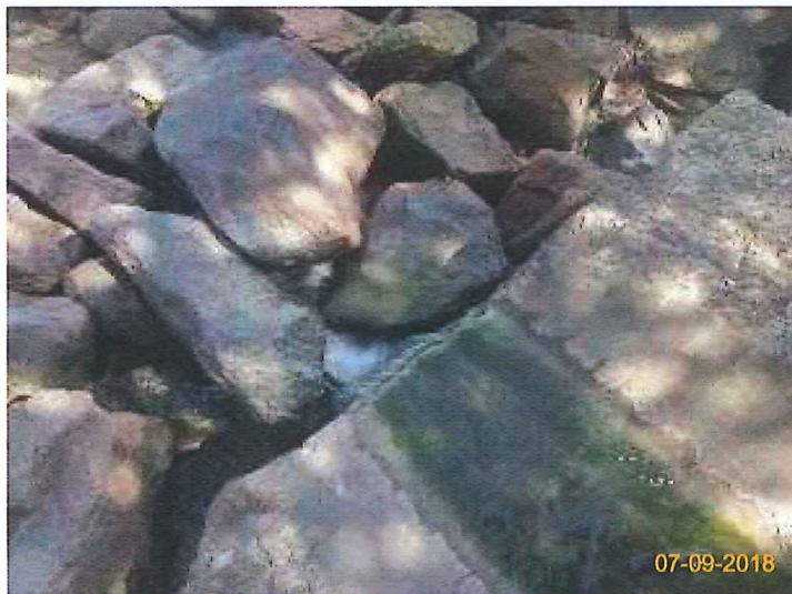
Item 7. Ensure no run-off into water body.(Outfall 1)
