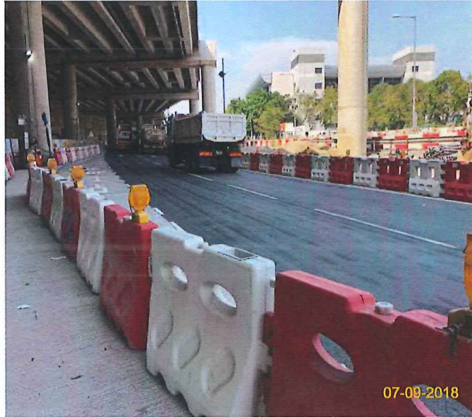
Item 5. Hoarding with panel around works area & Item 6. Temporary traffic management lighting.
