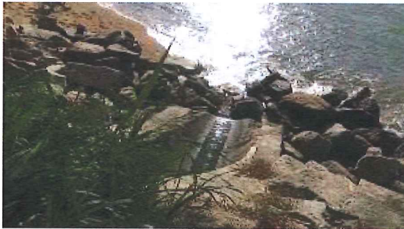
Outfall 1: Clean water is discharging.
