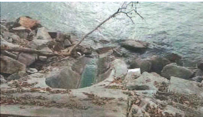
Outfall 1: Clean water is discharging.
