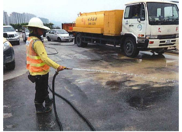
Photo 2 Water spraying by worker for un-accessible area.
