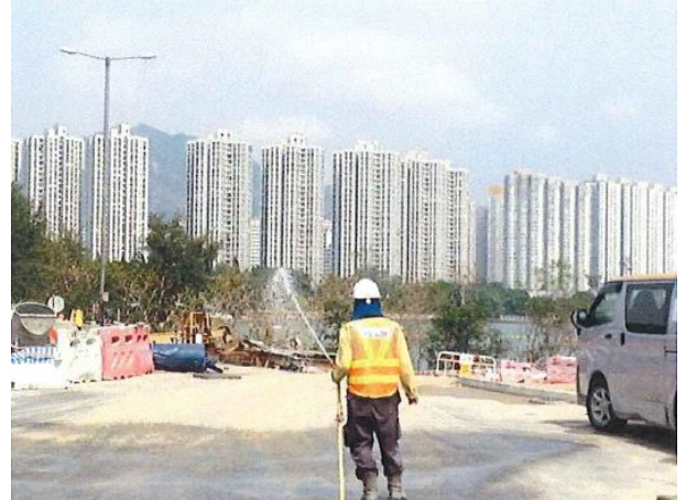
Photo 2 Water spraying by worker for un-accessible area.
