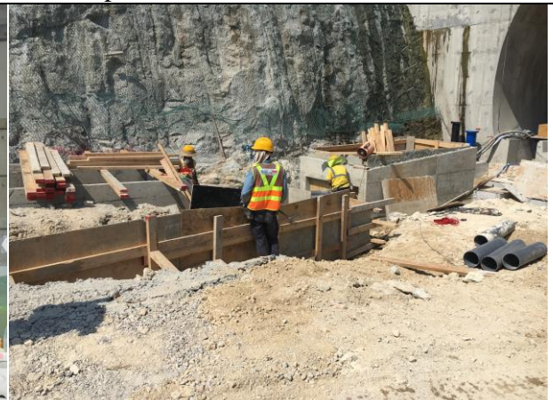
Photo 12 Drainage works at +19 platform
