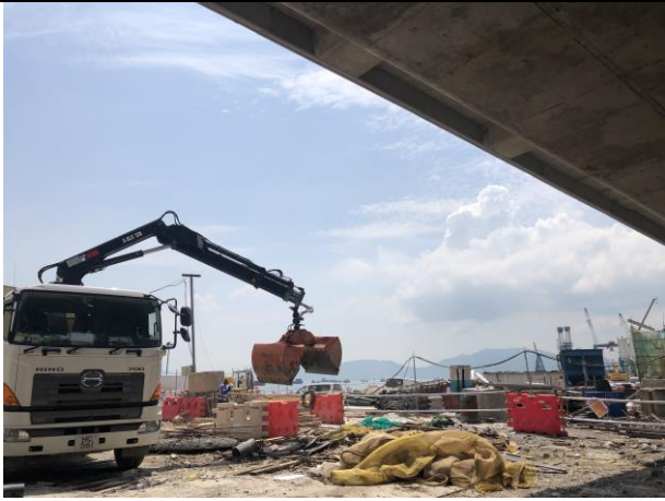
Photo 13 Housekeeping works at Portion F
