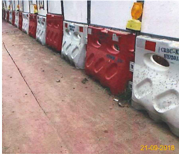
Item 5. Hoarding with panel around works area & Item 6. Temporary traffic management lighting.
