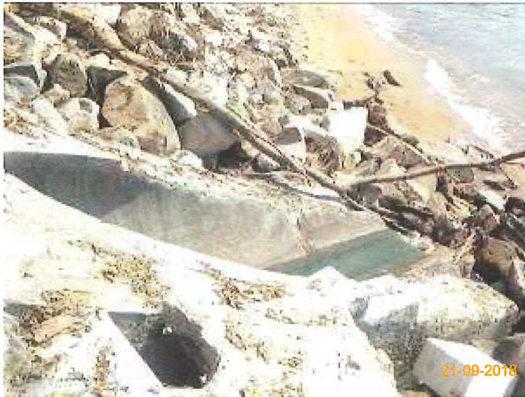
Item 7. Ensure no run-off into water body.(Outfall 1)
