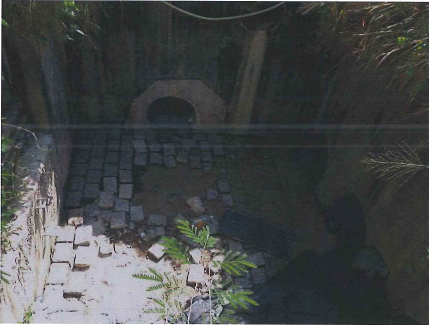
Stream B Outfall: Clean water is discharging.
