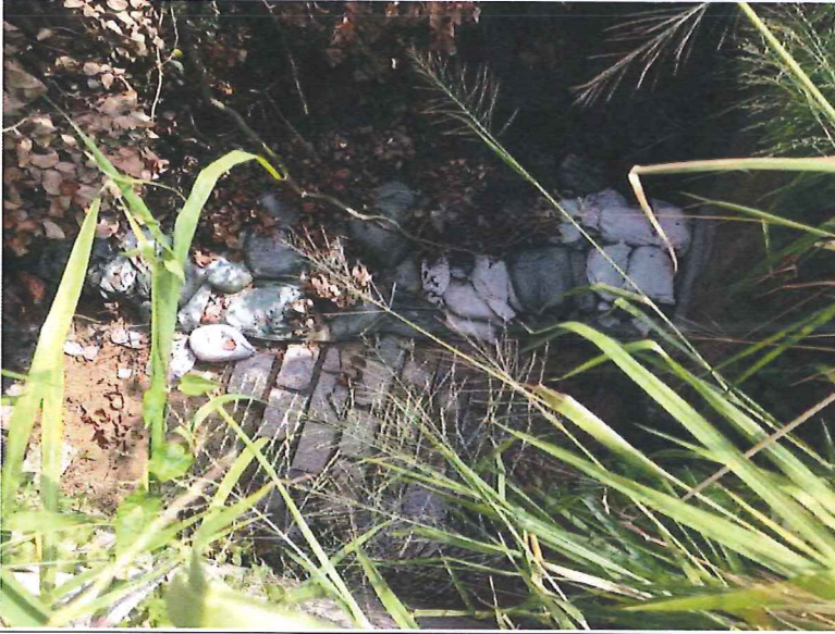
Stream B Outfall: No water is discharging.
