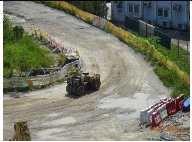
Photo 8 Dust mitigation measure was observed at site haul road during the join site inspection on 4 September 2018.
