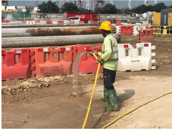
Photo 1 - Watering of unpaved roads to maintain a wet condition (4 October 2018)
