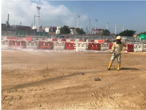
Photo 1 - Watering of unpaved roads to maintain a wet condition (10 October 2018)
