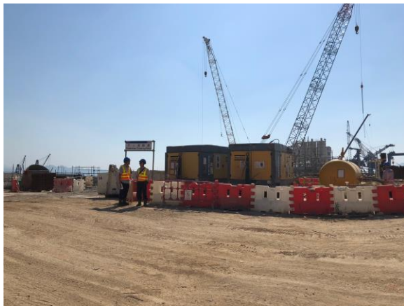
Photo 2 - Unpaved roads were maintained in a wet condition (5 October 2018)
