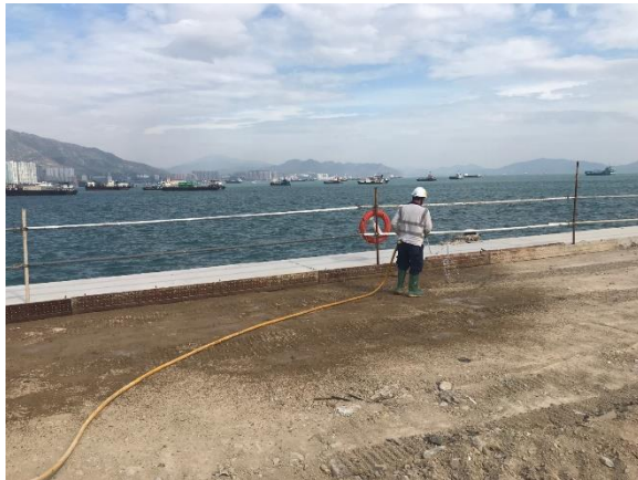
Photo 2 - Watering of unpaved roads near Fire Services Department Building and Customs & Excise Department Building to maintain a wet condition (6 November 2018)
