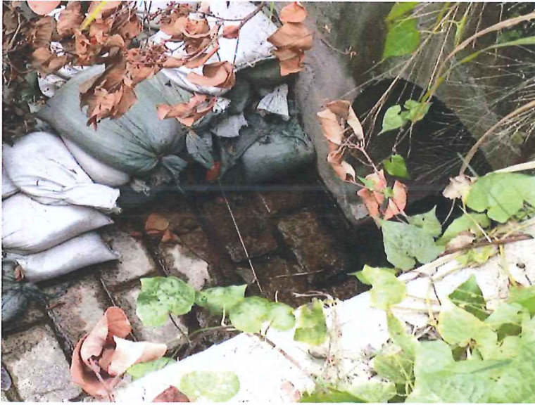
Stream B Outfall: Clean water is discharging.
