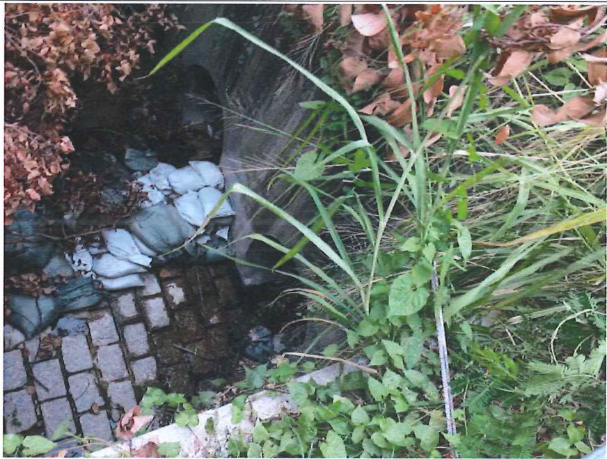
Stream B Outfall: No water is discharging.
