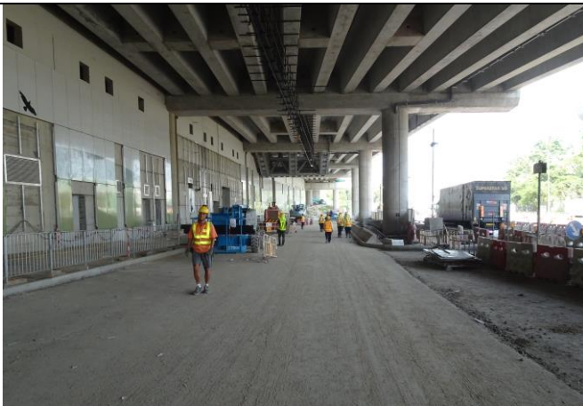
Photo 11 Installation of VE panels at Retaining Wall B
