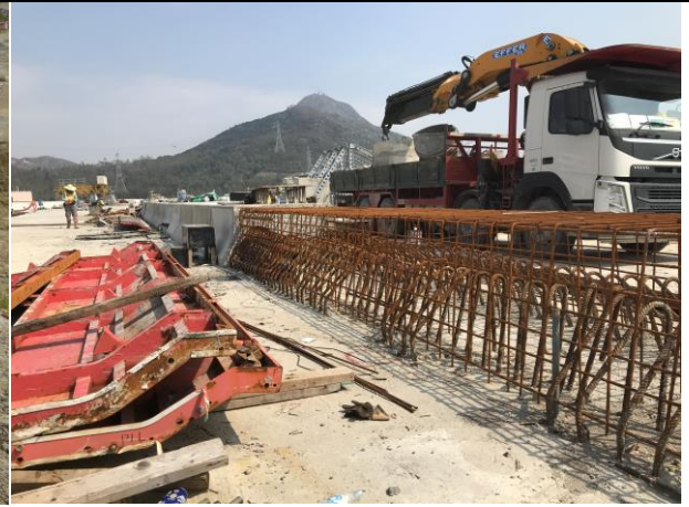
Photo 14 Construct of Parapet at Portion F
