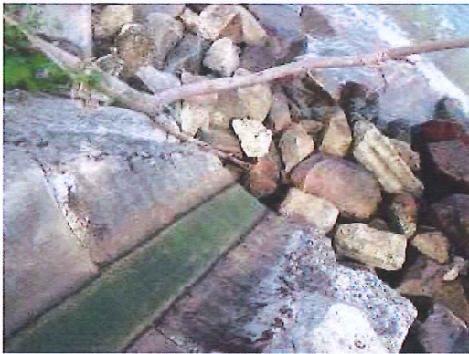
Outfall 1: Clean water is discharging.
