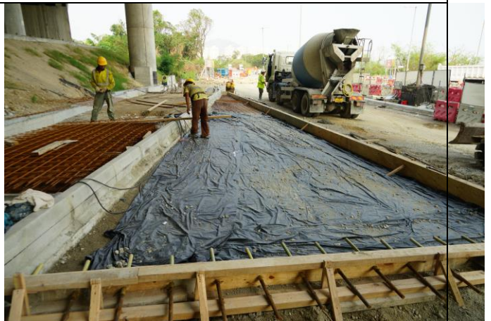
Photo 12 Road and Drainage Works at LMR Central Median
