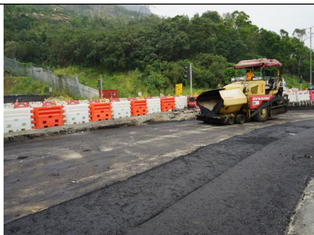
Photo 14 Road and Drainage Works at Lung Mun Road Central Median
