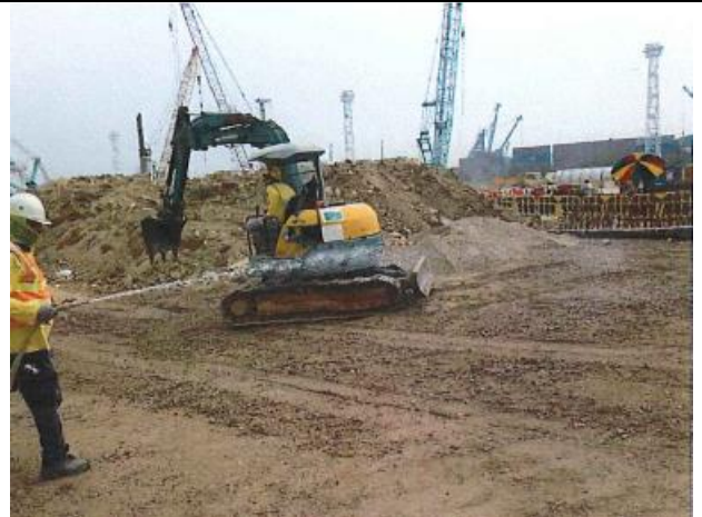
Photo 2 Water spraying by worker for un-accessible area.
