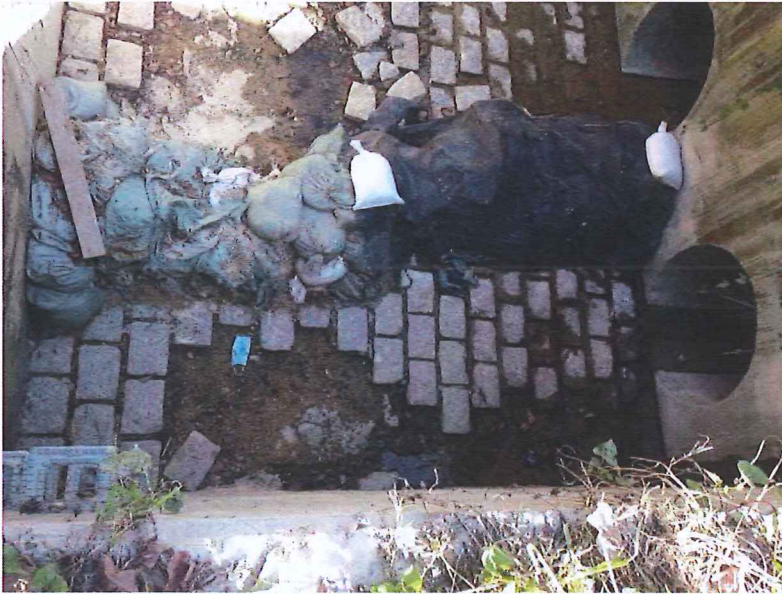
Stream B Outfall: No water is discharging.
