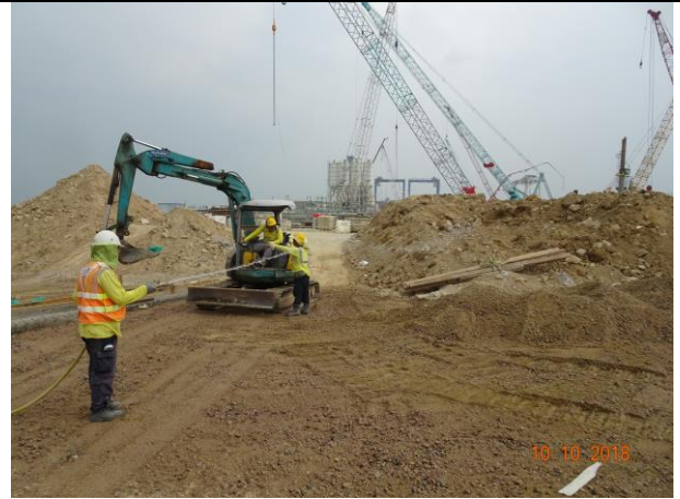
Photo 10 Dust mitigation measure was observed for the stockpile and site haul road at portion F during the join site inspection on 10 October 2018.
