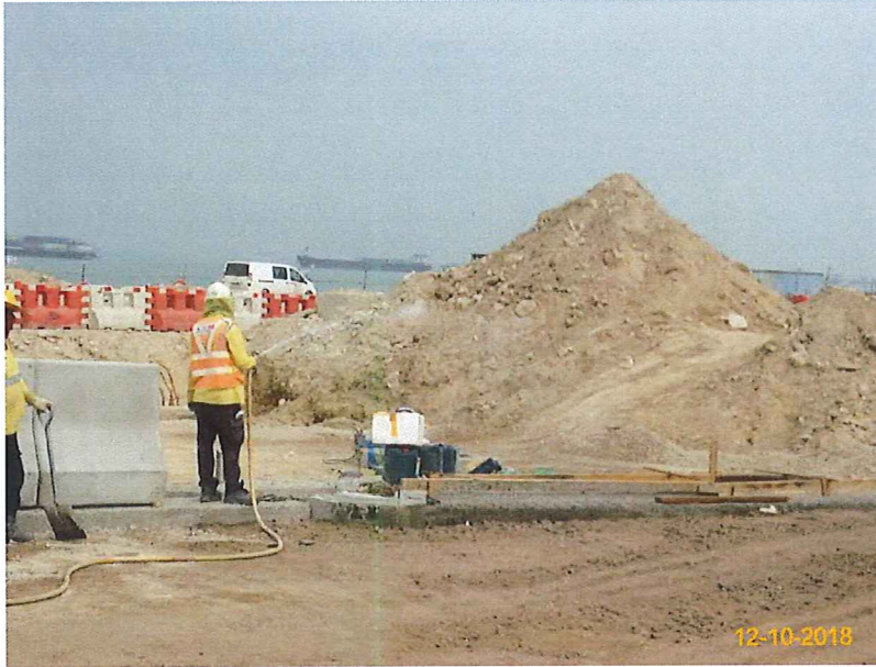
Item 4. Water spraying was provided for the stockpile at portion F
