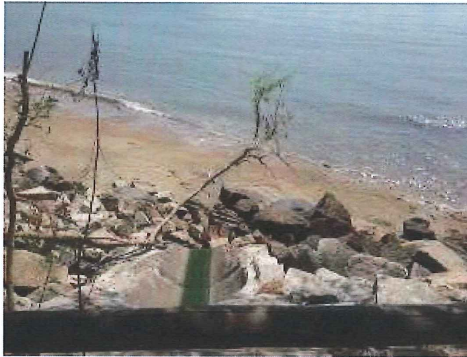
Outfall 1: Clean water is discharging.
