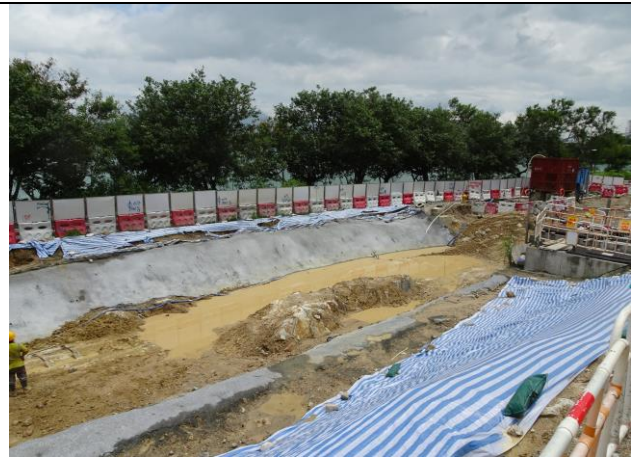
Photo 4 Covered part of the exposed slopes and stockpile by tarpaulin sheet.
