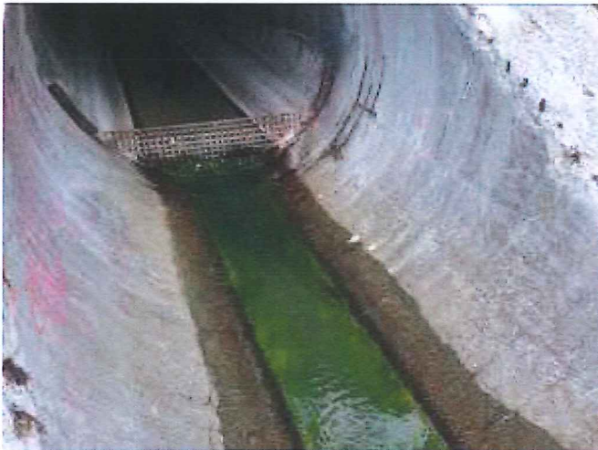
Outfall 1: No water is discharging.
