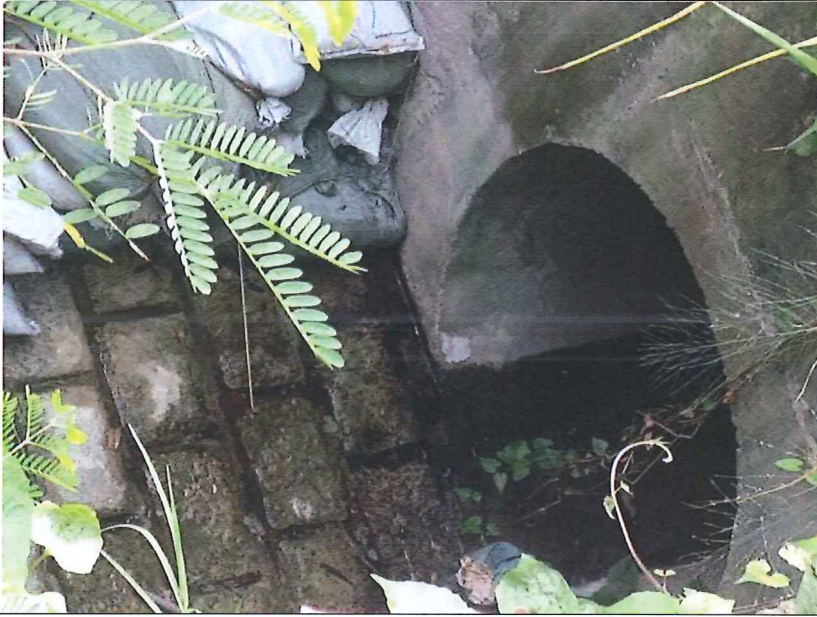
Stream B Outfall: Clean water is discharging.
