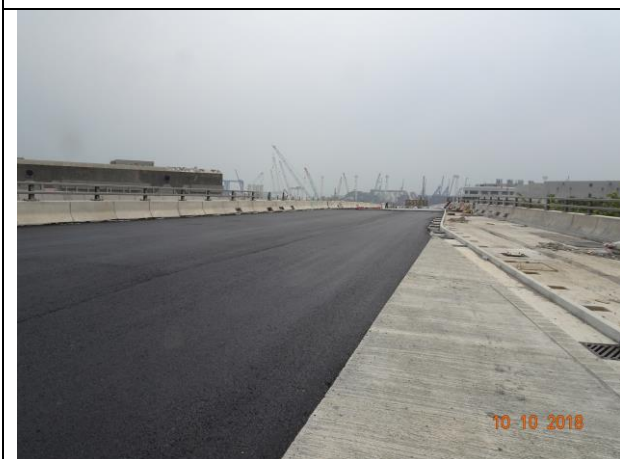
Photo 15 Stockpile stored at Portion F was backfilled and most of the site area was hard paved
