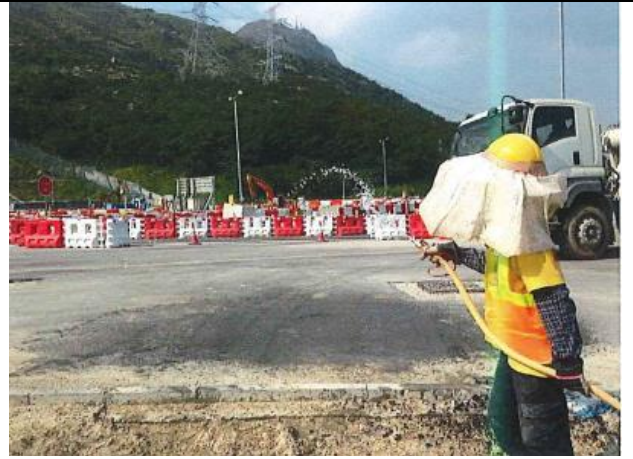
Photo 2 Water spraying by worker for un-accessible area.
