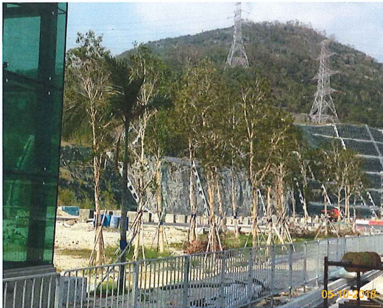
Item 2. Tree Transplanting works conducted on 22-May-17.
