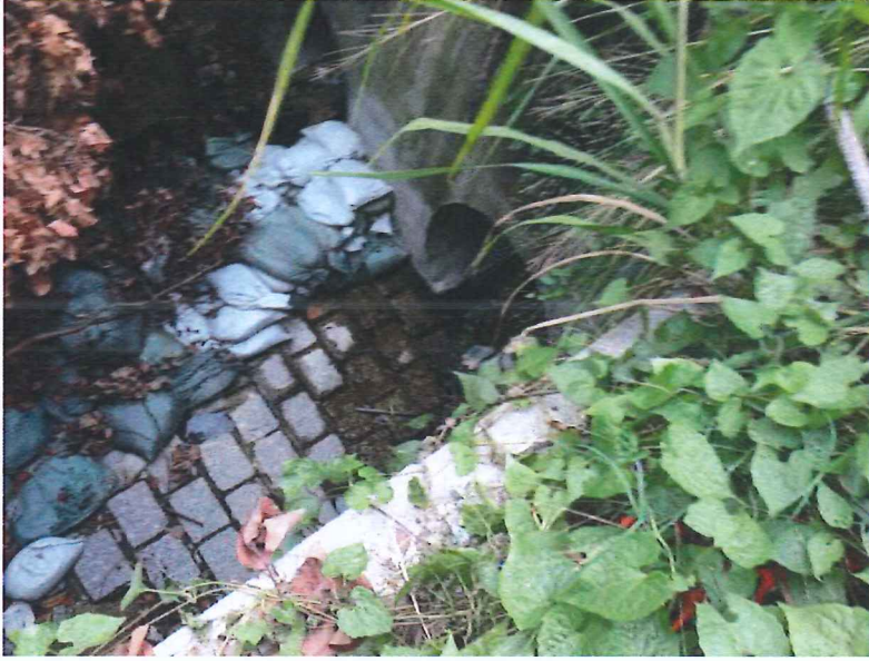
Stream B Outfall: No water is discharging.
