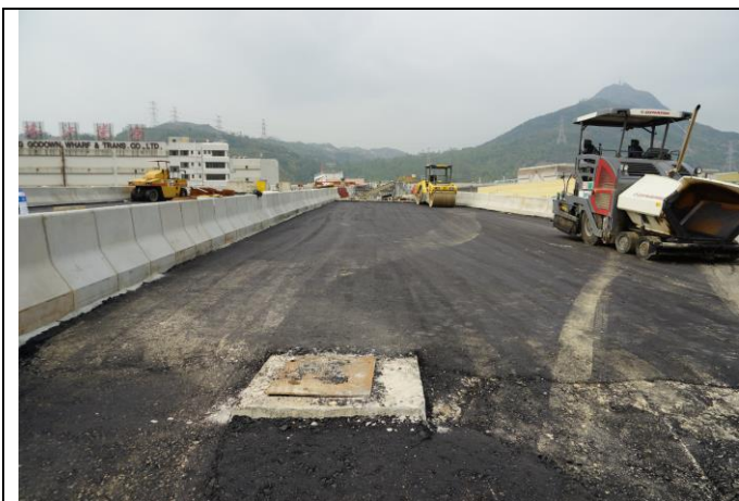
Photo 13 Construction of Parapet at Portion F
