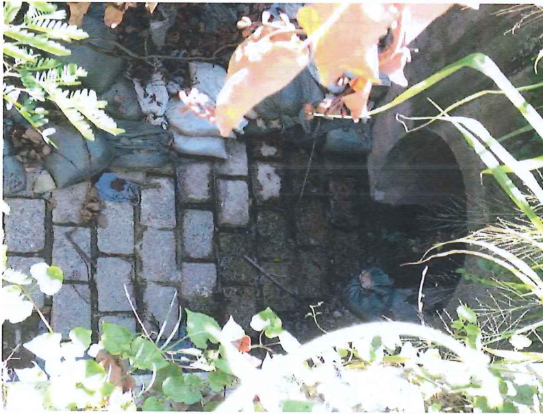
Stream B Outfall: Clean water is discharging.
