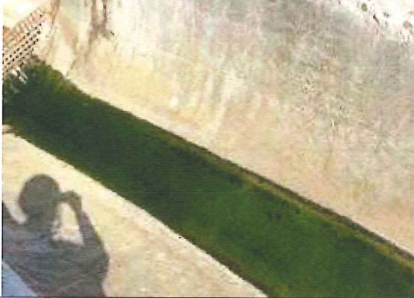
Outfall 1: Clean water is discharging.
