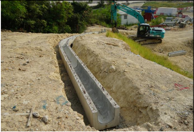
Photo 13 Drainage Works at at +19 Platform
