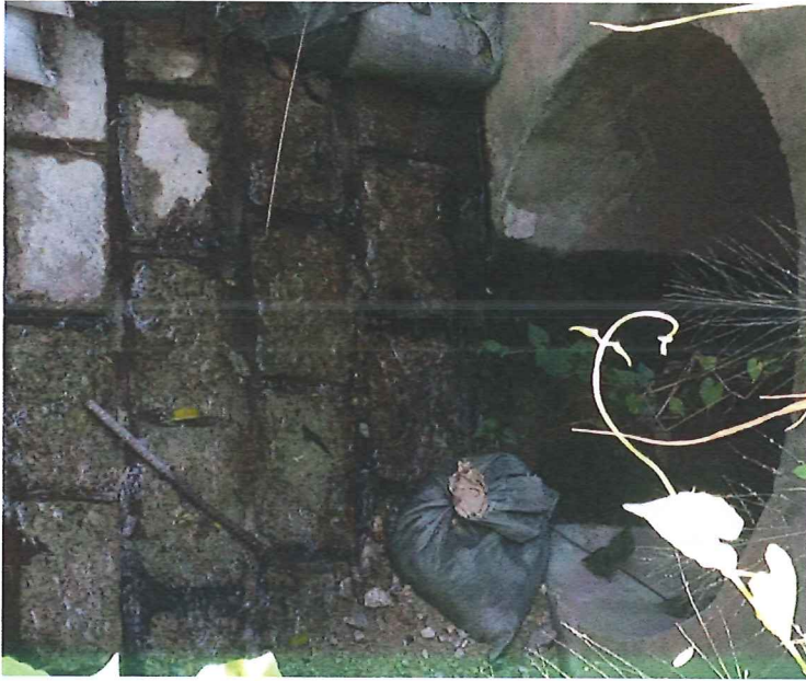
Stream B Outfall: Clean water is discharging.
