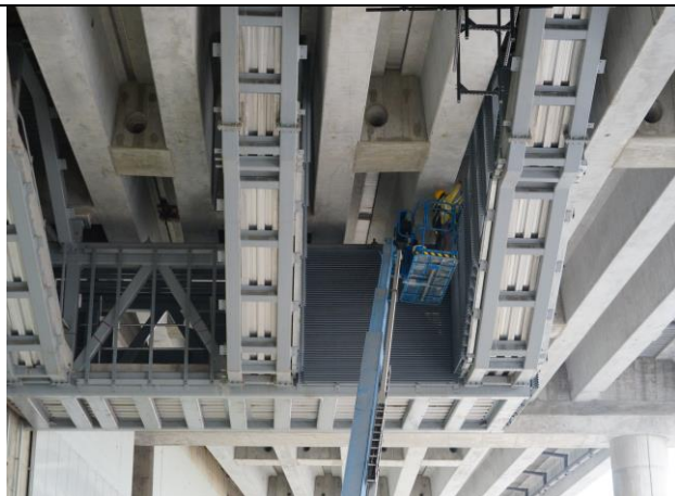
Photo 12 E&M Works at Retaining Wall B
