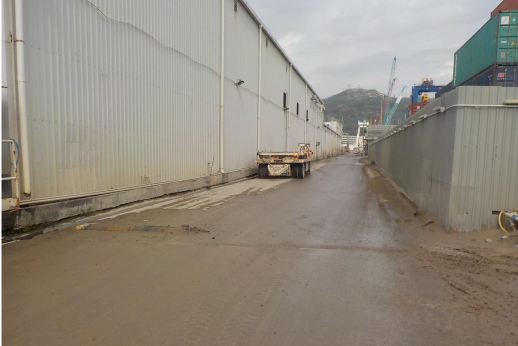
Water spraying was applied on the main haul road. (Works Area Portion N-A)
