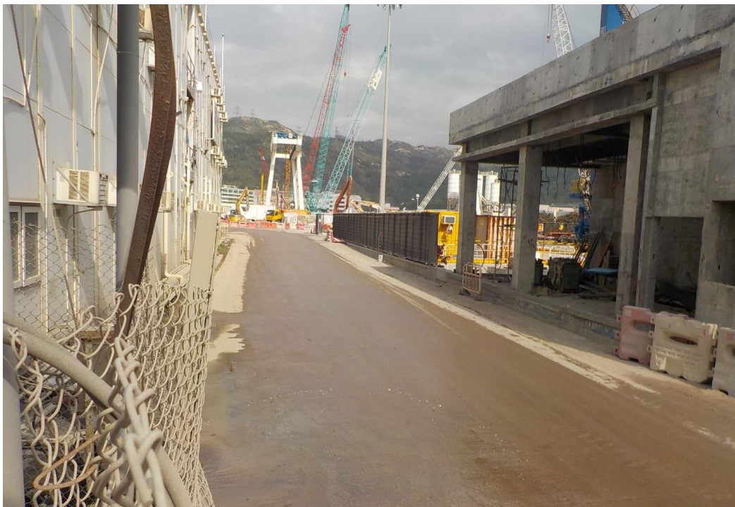
Water spraying was applied on the main haul road. (Works Area Portion N-C)
