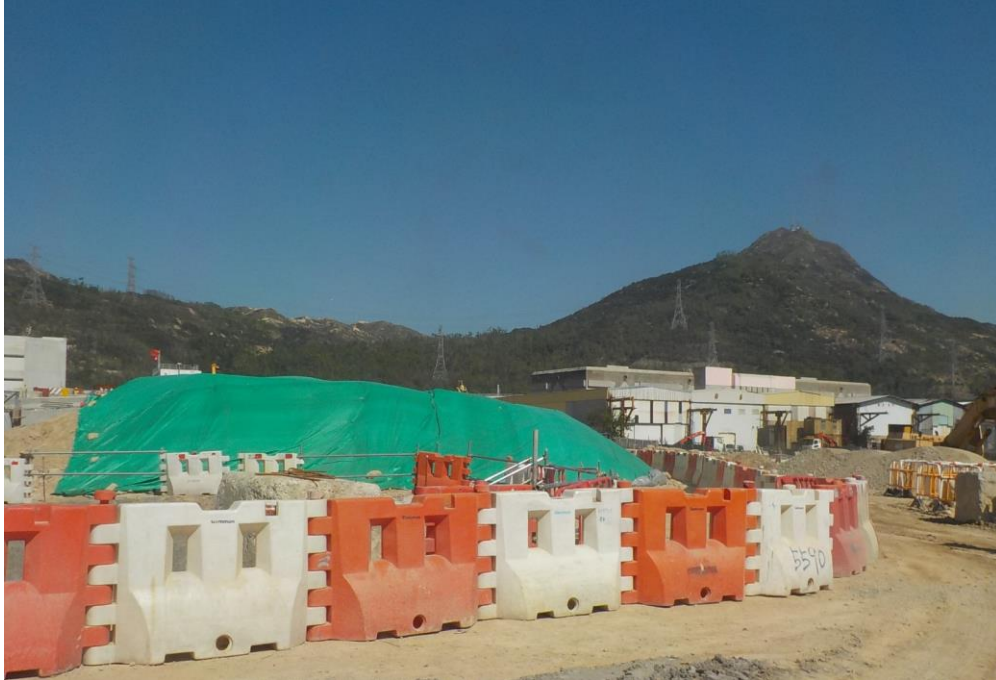
Exposed soil is covered by tarpaulin sheets. (Works Area Portion N-A)
