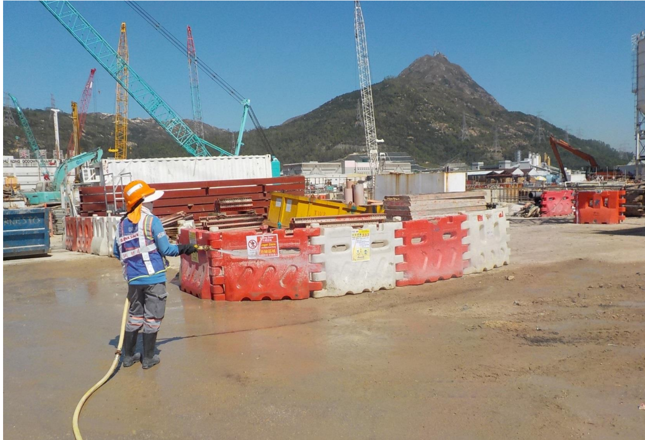
Water spraying was applied to prevent dust. (Works Area Portion N-A)
