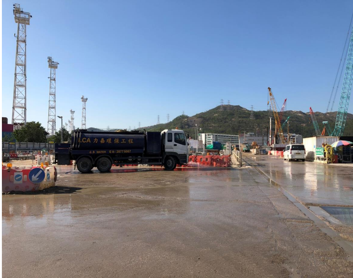
Water truck was used for dust control. (Works Area Portion N-A)
