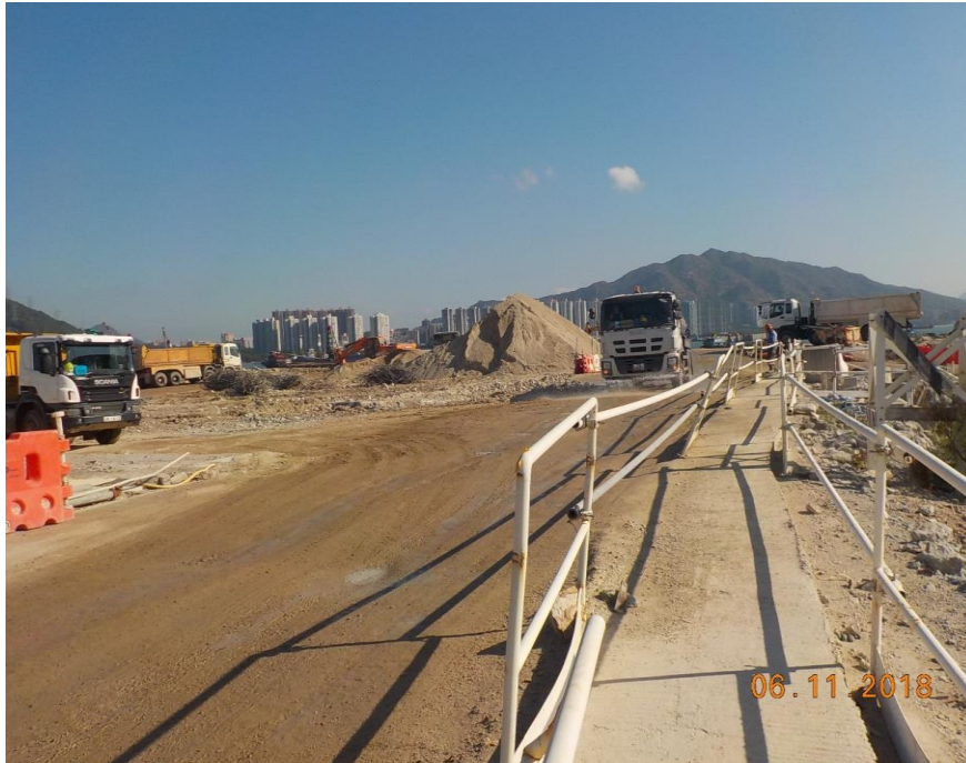
Water truck was used for dust control during surcharge removal. (Works Area Portion N-C)
