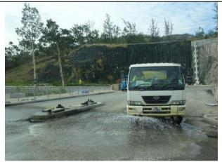
**Photo 11** Dust mitigation measure was observed at site haul road during the joint site inspection on 13 November 2018.
