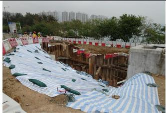
**Photo 5** Covered part of the exposed slopes and stockpile by tarpaulin sheet.
