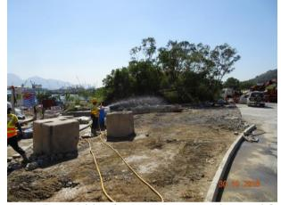
**Photo 9** Dust mitigation measure was observed for the exposed area and site haul road at portion H during the joint site inspection on 30 October 2018.
