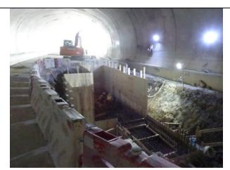
Photo 17 Drainage Works at Underpass
