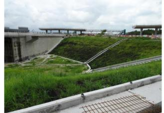
Photo 3 Hydro seeding for the exposed slope at Retaining Wall B.
