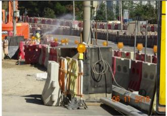
**Photo 9** Dust mitigation measure was observed at site haul road during the joint site inspection on 6 November 2018.
