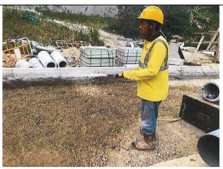
Photo 2 Water spraying by worker for unaccessible area.
