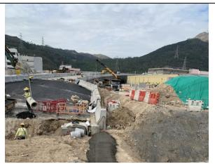
Photo 13 Drainage Works at Portion F
