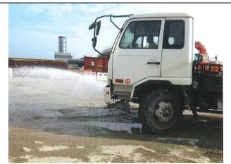
Photo 1 Watering of haul road by water truck to keep road surface wet
