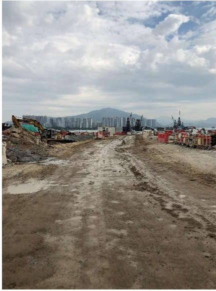
Photo 3 - Unpaved roads were maintained in a wet condition (9 November 2018)
