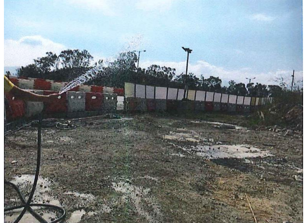
Photo 2 Water spraying by worker for un-accessible area.
