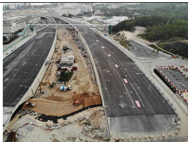
Photo 12 Road marking works at Bridge G
