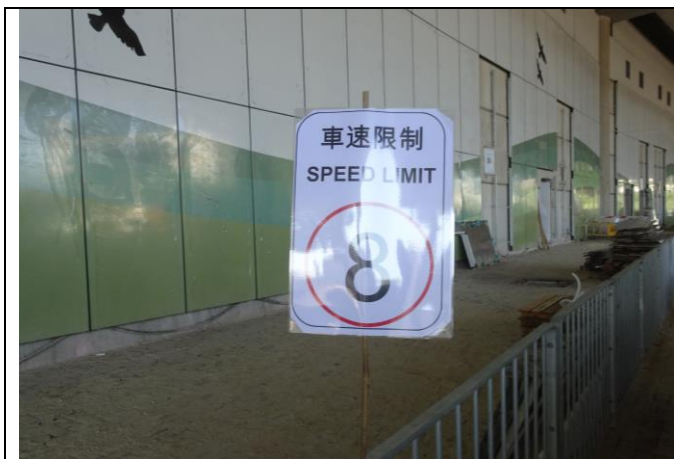
Photo 7 Set speed control at ~8km/hr for all vehicles using the haul road at Lung Mun Road.
