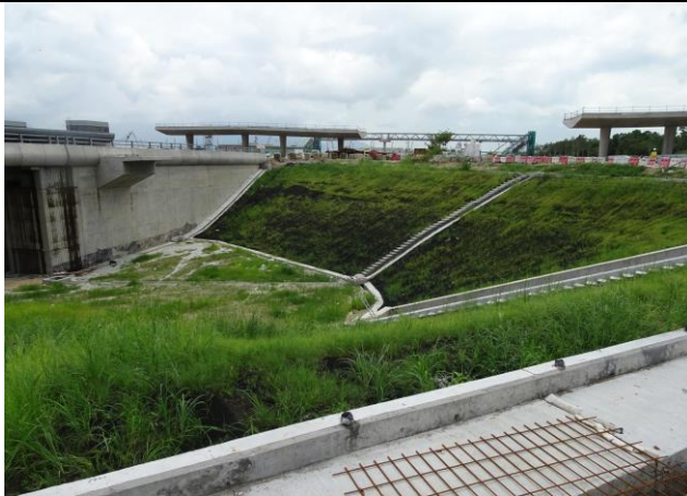
Photo 3 Hydro seeding for the exposed slope at Retaining Wall B.
