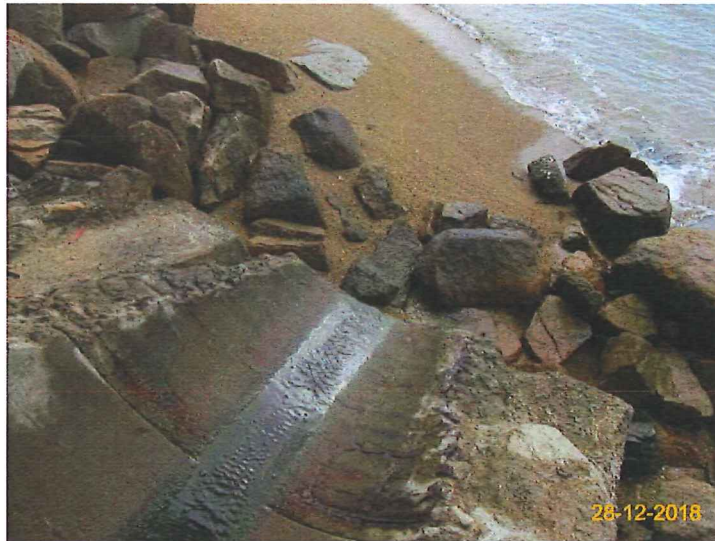
Item 7. Ensure no run-off into water body.(Outfall 1)
