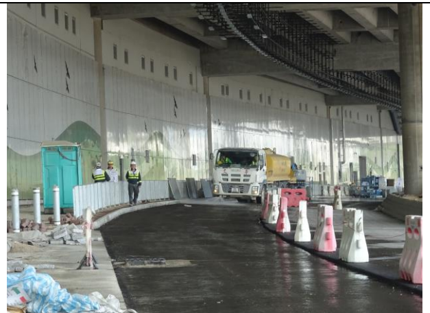
Photo 10 Dust mitigation measure was observed at site haul road during the joint site inspection on 18 December 2018.
