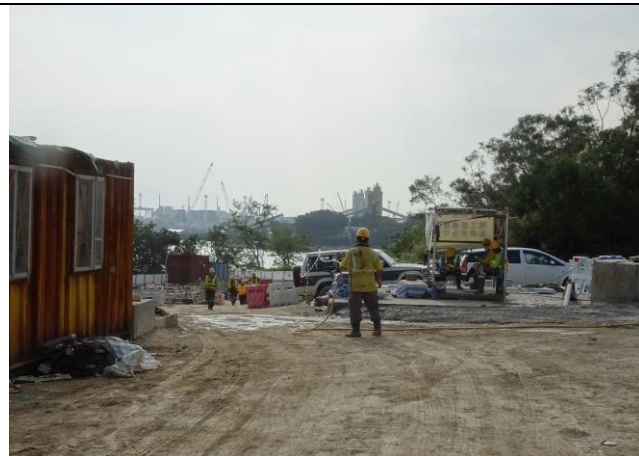
Photo 9 Dust mitigation measure was observed at site haul road during the joint site inspection on 18 December 2018.
