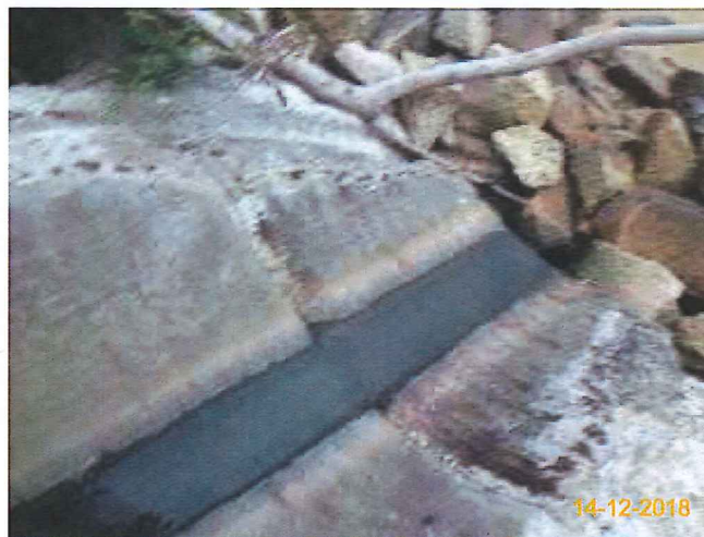
Item 7. Ensure no run-off into water body.(Outfall 1)
