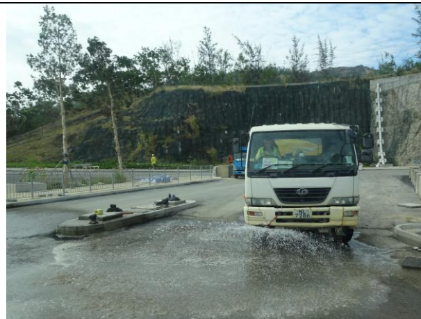
Photo 8 Dust mitigation measure was observed at site haul road during the joint site inspection on 4 December 2018.
