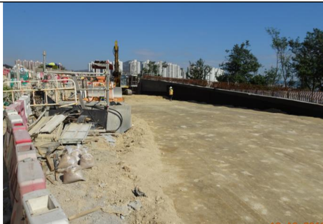
Photo 11 Drainage Works at Portion H
