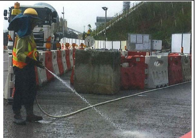
Photo 2 Water spraying by worker for un-accessible area.
