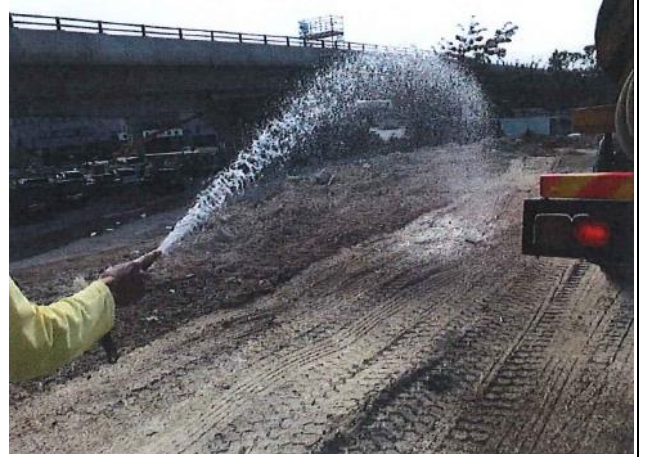
Photo 2 Water spraying by worker for un-accessible area.
