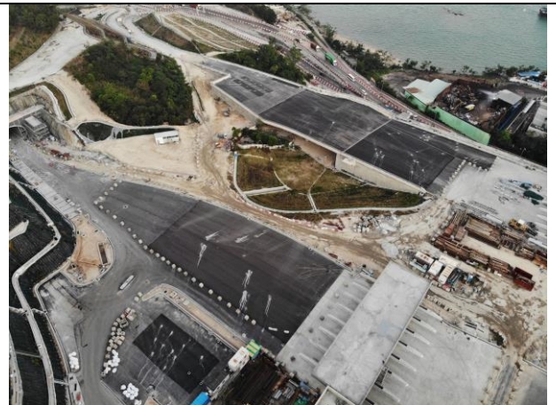
Photo 12 Road marking works at Bridge G
