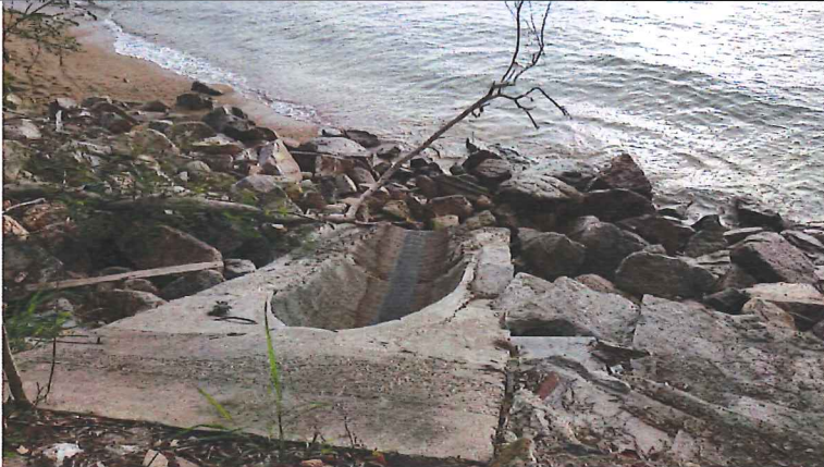
Outfall 1: No water is discharging.
