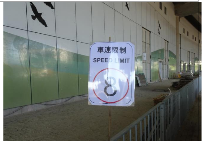
Photo 6 Set speed control at ~8km/hr for all vehicles using the haul road
