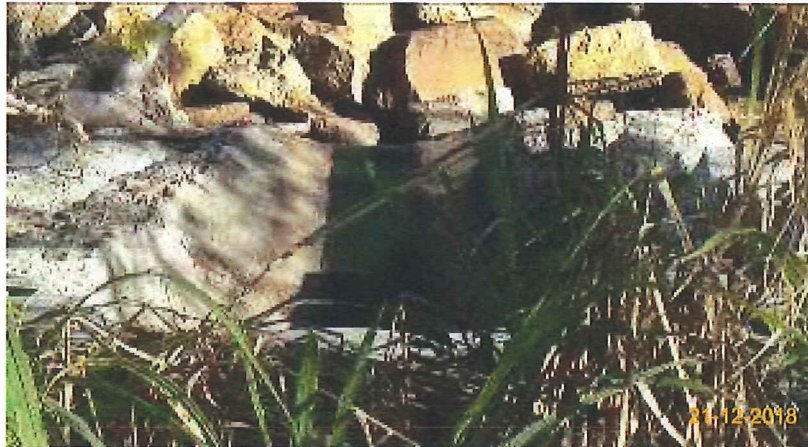
Item 7. Ensure no run-off into water body.(Outfall 1)
