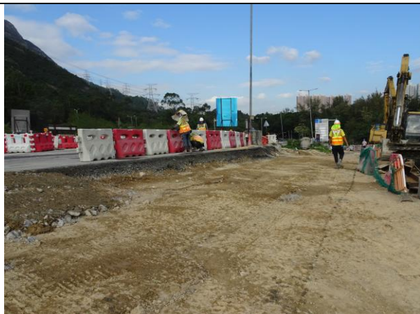
Photo 9 Water spraying for the haul road was observed during the joint site inspection on 4 December 2018.
