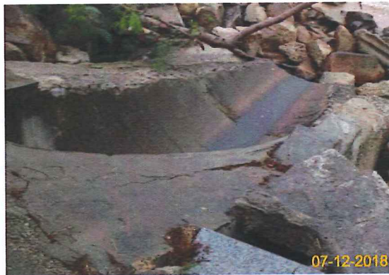
Item 7. Ensure no run-off into water body.(Outfall 1)
