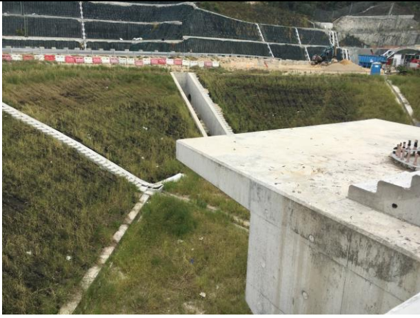
Photo 13 Drainage Works at +19 Platform
