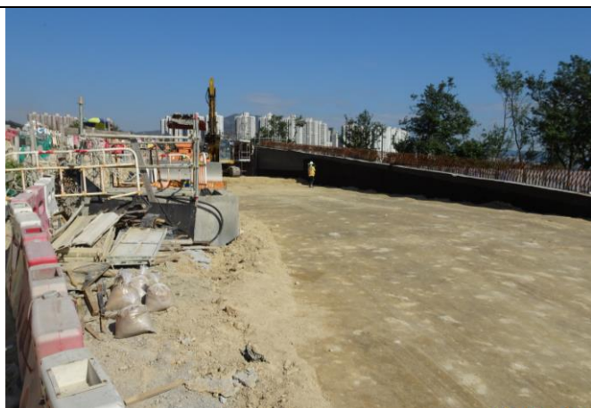
Photo 11 Drainage Works at Portion H
