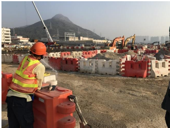
Photo 2- Watering of unpaved roads near Administration Building and Maintenance Depot
