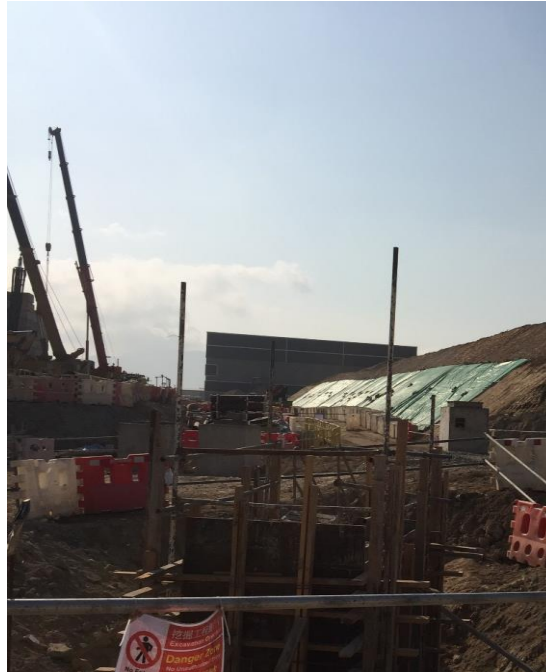
Exposed soil was covered by tarpaulin sheets to prevent dust. (Works Area Portion N-C)
