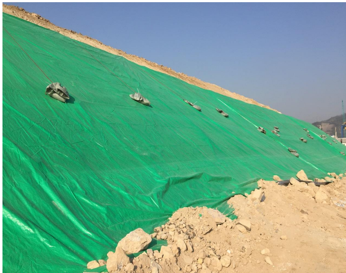
Exposed soil is covered by tarpaulin sheets to prevent dust. (Works Area Portion N-C)
