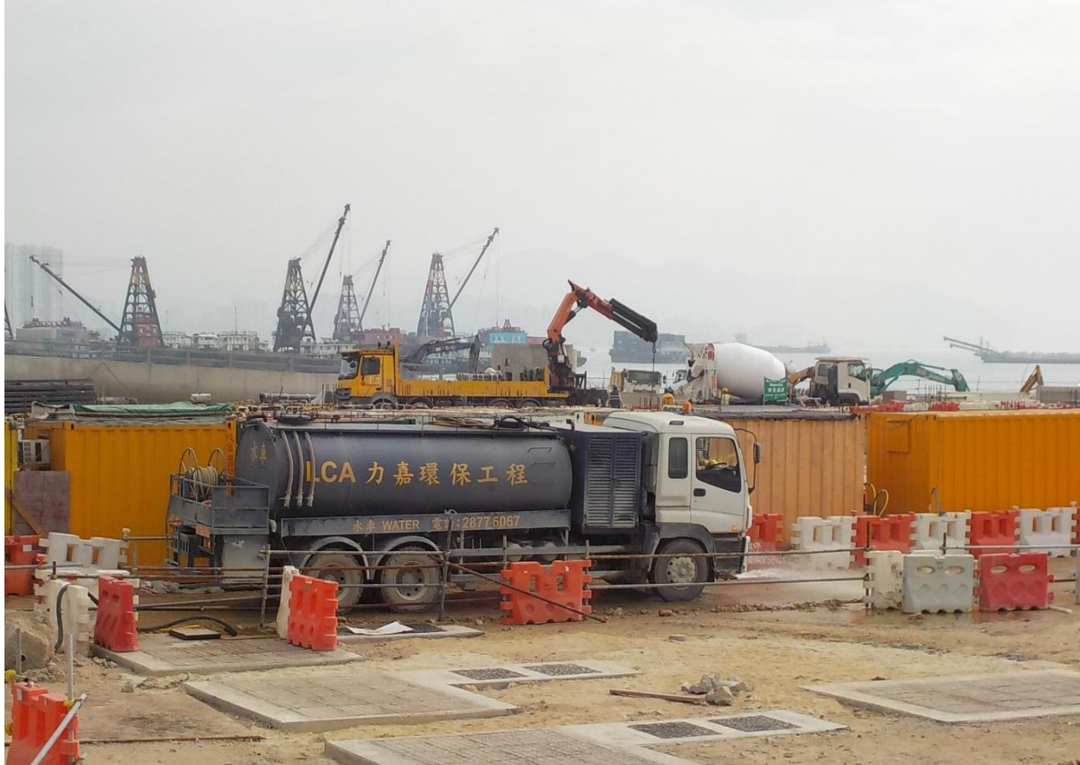
Water truck is used for water spraying to prevent dust. (Works Area Portion N-A)
