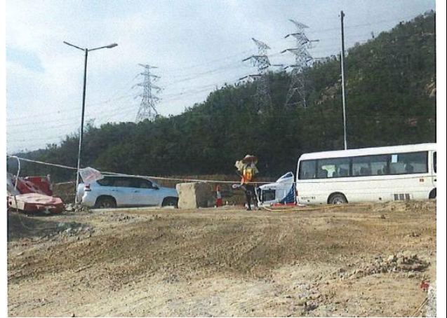
Photo 2 Water spraying by worker for un-accessible area.
