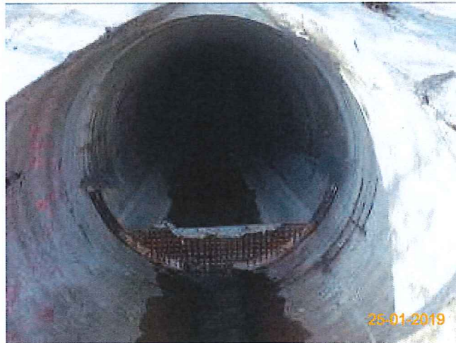
Item 7. Ensure no run-off into water body.(Outfall 1)
