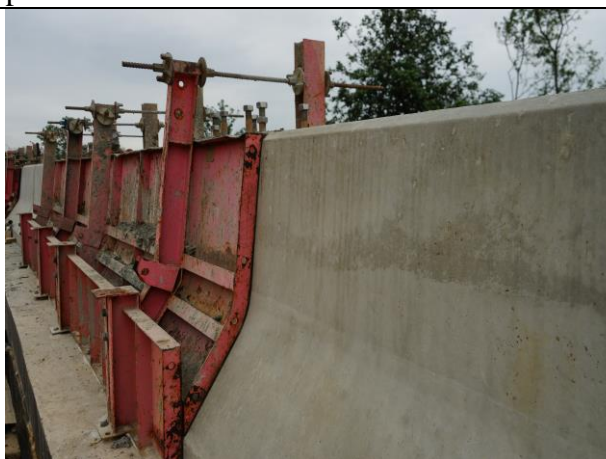
Photo 12 Construction of Retaining wall G & parapet at Portion H
