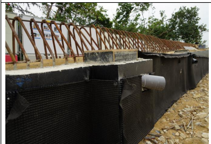
Photo 11 Construction of Retaining wall G & parapet at Portion H
