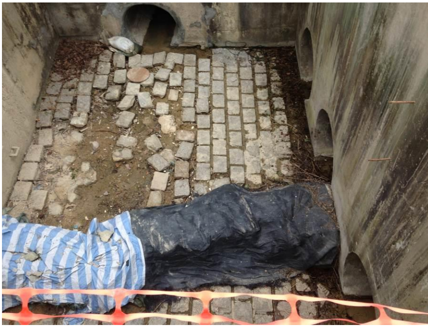
Stream B Outfall: No water is discharging.
