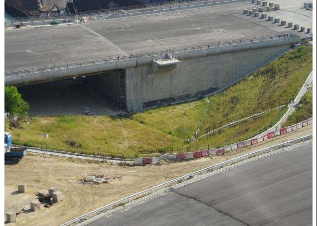
Photo 4 Hydro seeding for the exposed slope.
