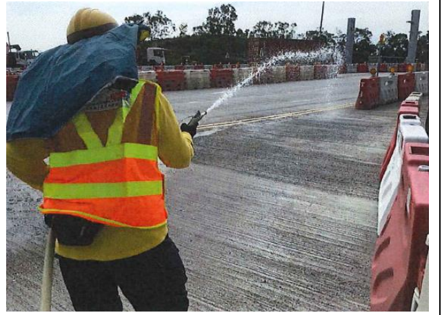
Photo 2 Water spraying by worker for un-accessible area.
