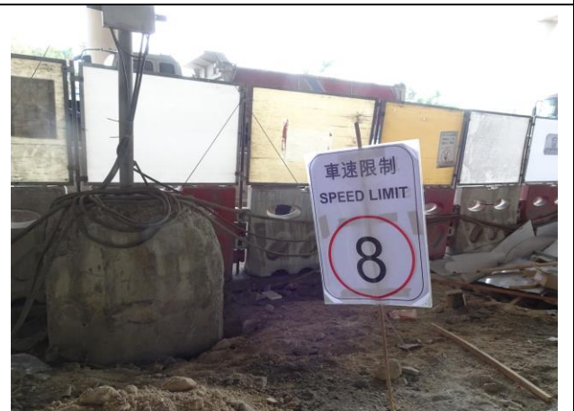
Photo 6 All vehicles using the haul road had enhanced to control the speed below 8km/hr to reduce dust emission.
