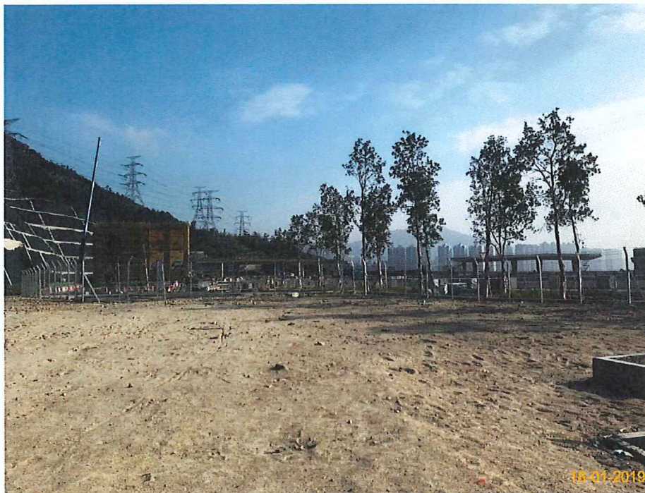
Item 2. Tree Transplanting works conducted on 22-May-17.
