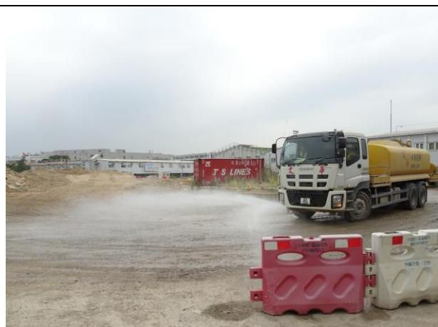
Photo 8 Water spraying was observed at site haul road during the joint site inspection on 8 January 2019.
