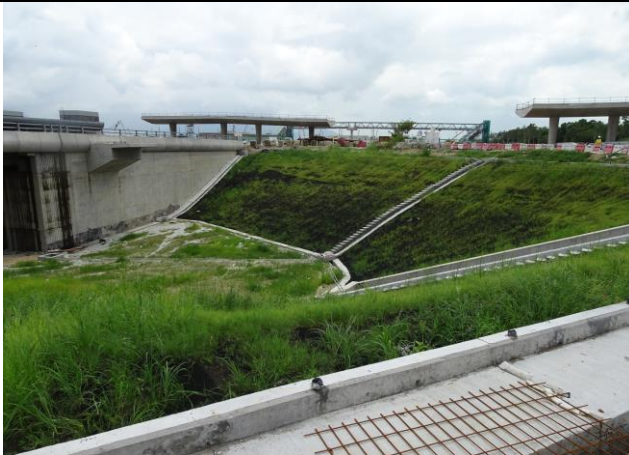
Photo 3 Hydro seeding for the exposed slope at Retaining Wall B.
