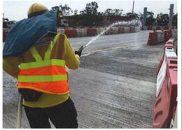
Photo 2 Water spraying by worker for un-accessible area.
