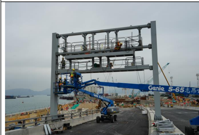
Photo 11 Installation of sign gantries at Bridge G
