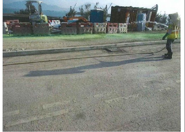
Photo 2 Water spraying by worker for un-accessible area.
