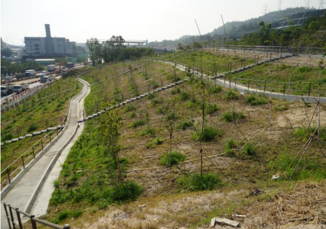
Photo 3 Hydro seeding for the exposed slope.
