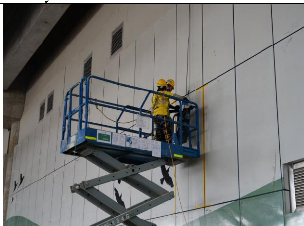
Photo 12 Installation of VE panels at Retaining Wall B
