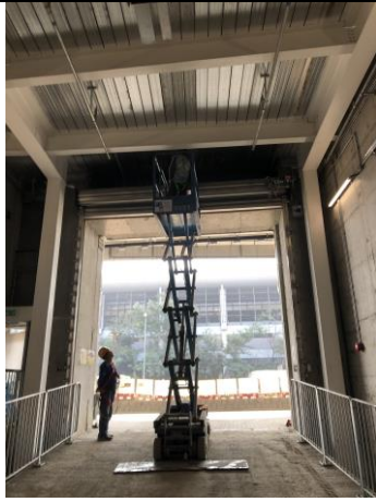
Photo 13 E&M works at the storage room at Retaining Wall B
