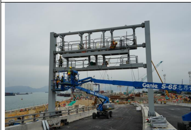
Photo 11 Installation of sign gantries at Bridge G
