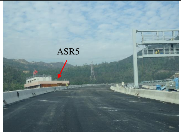
Photo 14 All of the site area near ASR5 were hard paved
