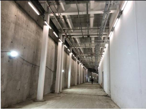
Photo 13 E&M works at the storage room at Retaining Wall B
