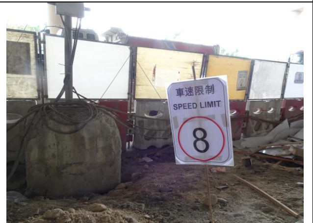
Photo 6 All vehicles using the haul road had enhanced to control the speed below 8km/hr to reduce dust emission.
