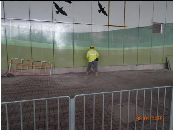
Photo 13 Installation of VE panels at Retaining Wall B
