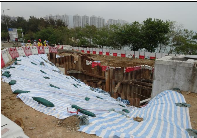
Photo 5 Covered part of the exposed slopes and stockpile by tarpaulin sheet.
