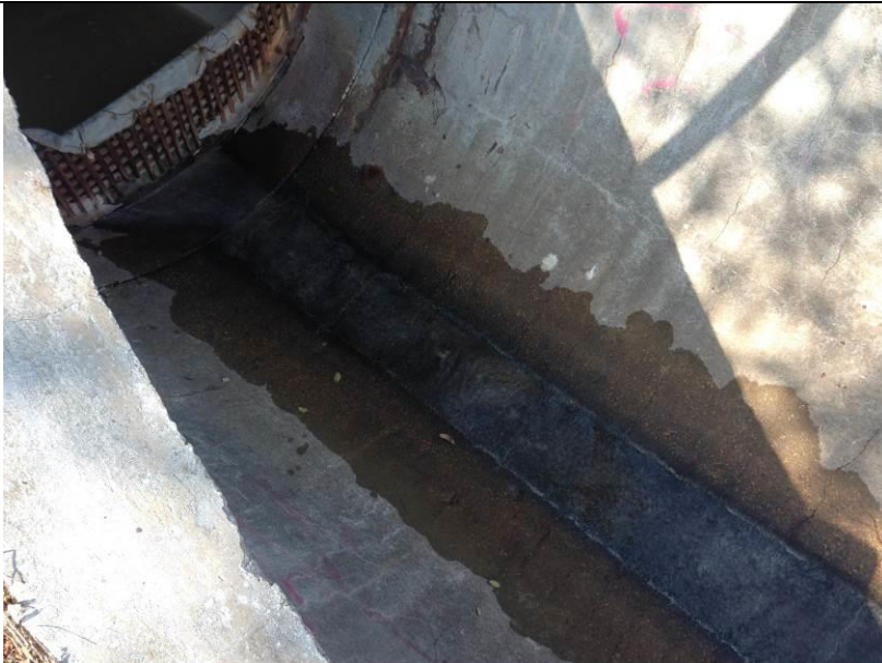
Outfall 1: Clean water is discharging.
