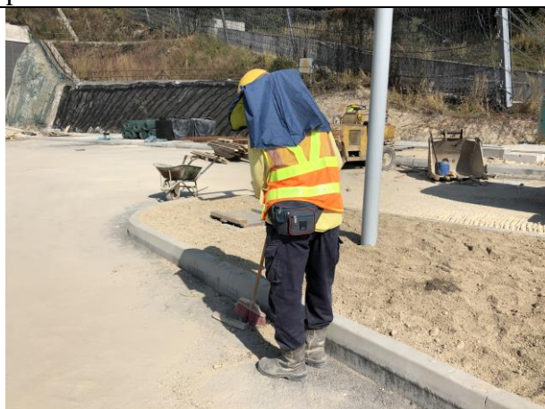
Photo 11 Housekeeping works at Lung Mun Road central median
