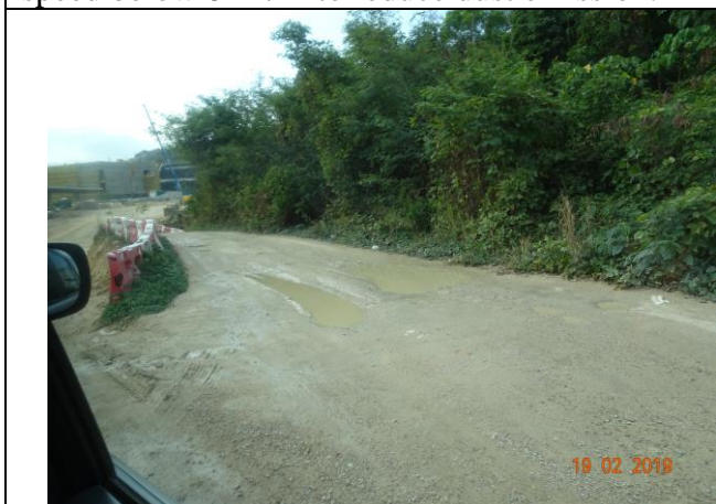
Photo 9 Water spraying was observed at site haul road during the joint site inspection on 19 February 2019.
