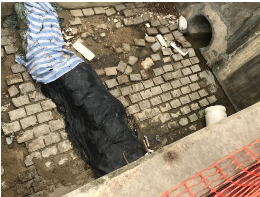
Stream B Outfall: No water is discharging.
