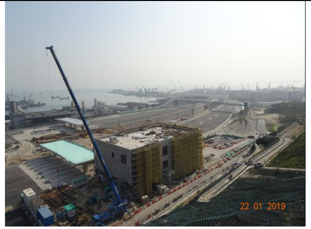
Photo 14 All of the site area near ASR1 were hard paved
