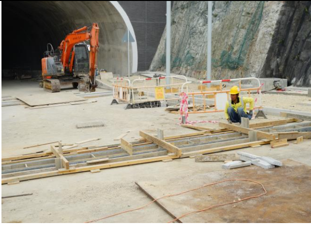
Photo 13 Drainage Works at East Portal
