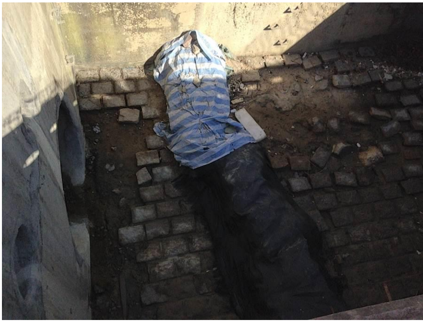
Stream B Outfall: No water is discharging.
