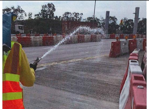
Photo 2 Water spraying by worker for un-accessible area.
