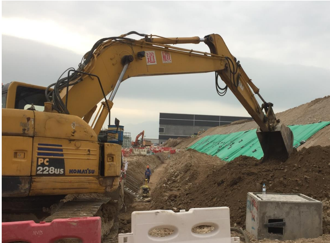
Exposed soil was covered by tarpaulin sheet to prevent dust. (Works Area Portion N-C)
