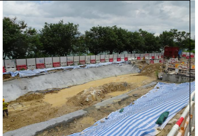
Photo 4 Covered part of the exposed slopes and stockpile by tarpaulin sheet.
