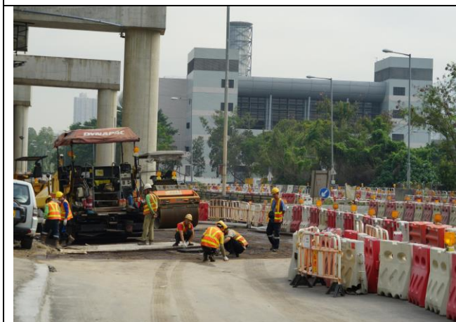
Photo 11 Road pavement works at Lung Mun Road
