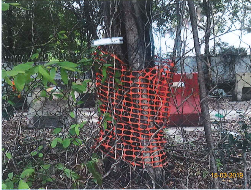
Item 1. Existing trees on boundary of the Project Area should be protected carefully during construction.
