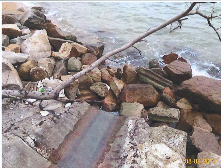
Item 7. Ensure no run-off into water body.(Outfall 1)
