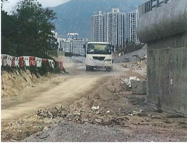
Photo 1 Watering of haul road by water truck to keep road surface wet
