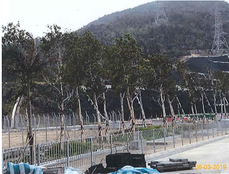
Item 2. Tree Transplanting works conducted on 22-May-17.
