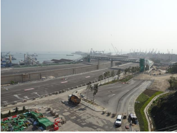
Photo 13 All of the site area at Portion F were hard paved
