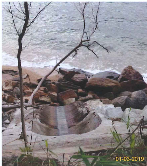
Item 7. Ensure no run-off into water body.(Outfall 1)
