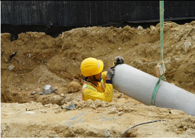
Photo 13 Drainage works at Portion H
