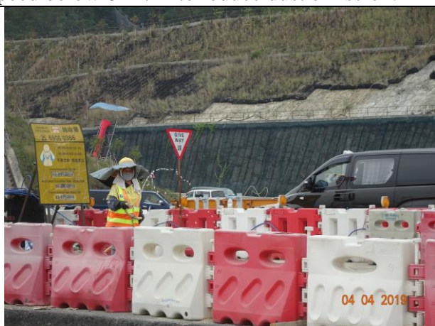
Photo 9 Water spraying was observed at works area during the joint site inspection on 4 April 2019.
