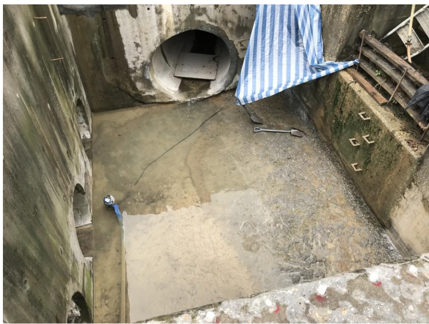
Stream B Outfall: No water is discharging.
