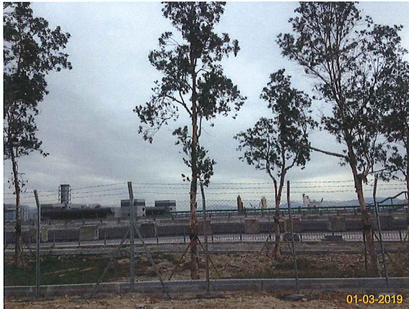
Item 2. Tree Transplanting works conducted on 22-May-17.
