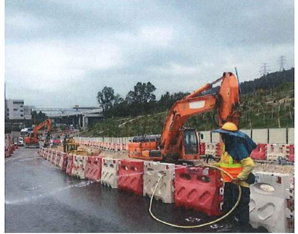
Photo 2 Water spraying by worker for un-accessible area.
