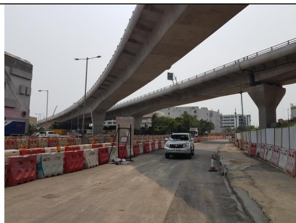
Photo 8 During the joint site inspection on 26 March 2019 most of the site area was hard paved.
