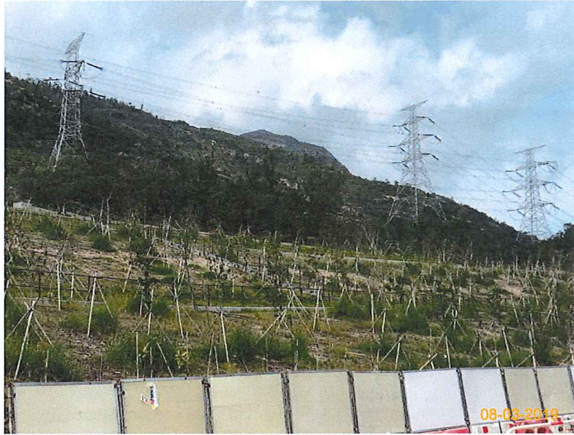
Item 3. Landscape works such as slope planting was commenced.
