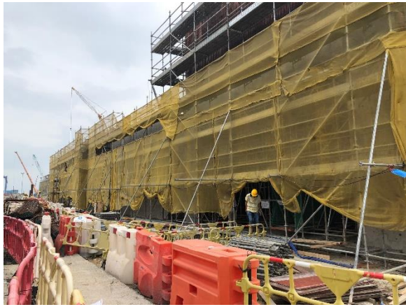
Photo 1 - Structure building at Maintenance Depot
