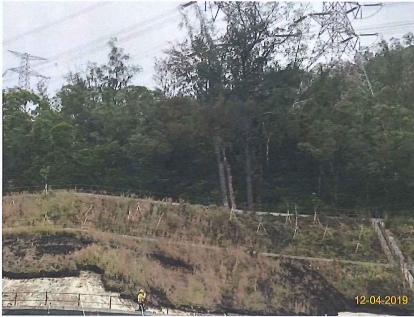
Item 3. Landscape works such as slope planting was commenced.
