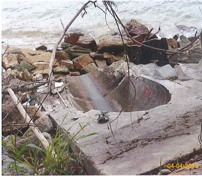
Item 7. Ensure no run-off into water body.(Outfall 1)
