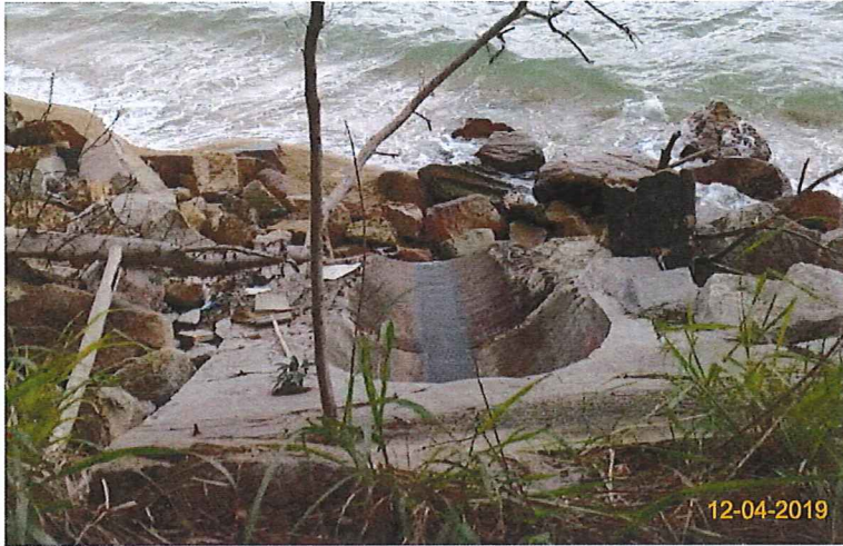
Item 7. Ensure no run-off into water body.(Outfall 1)
