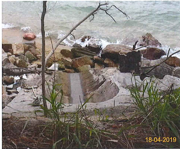
Item 7. Ensure no run-off into water body.(Outfall 1)
