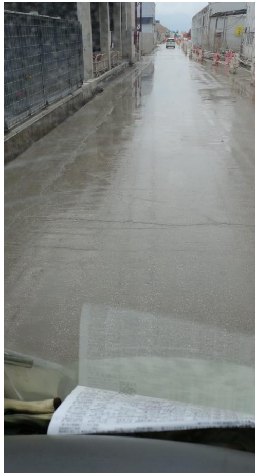
Water spraying was applied on main haul road near Amenities.
