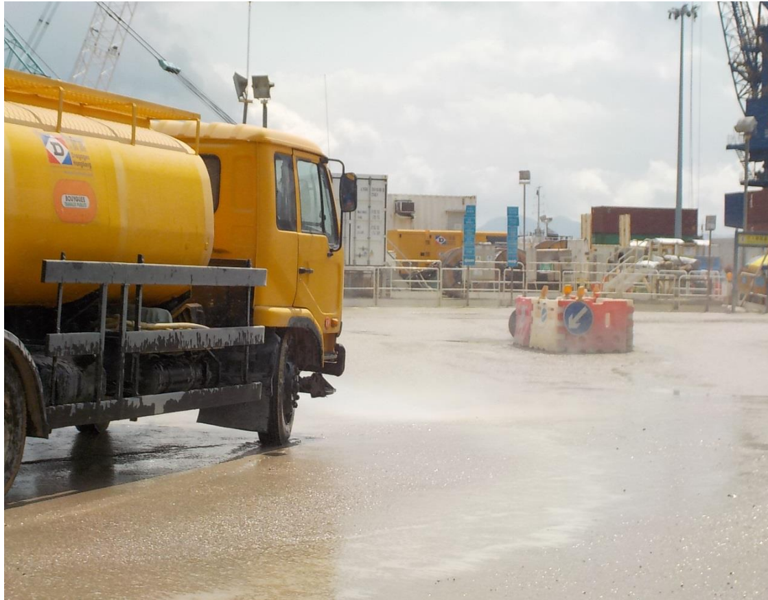
Water truck was used for water spraying on site.
