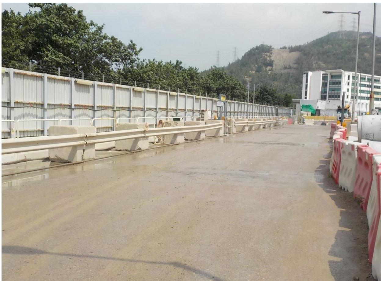
Water spraying was applied at the main haul road to prevent dust. (Works Area Portion N-A)
