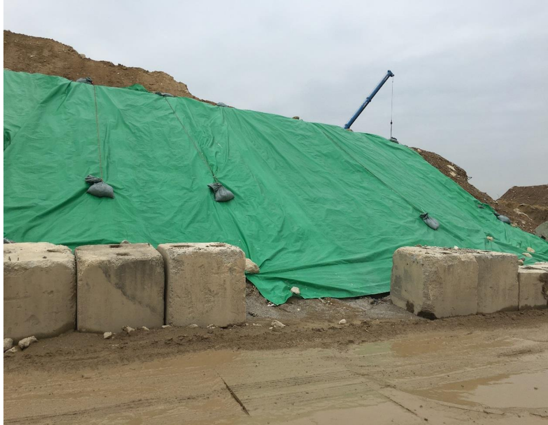
Exposed soil is covered by tarpaulin sheets
