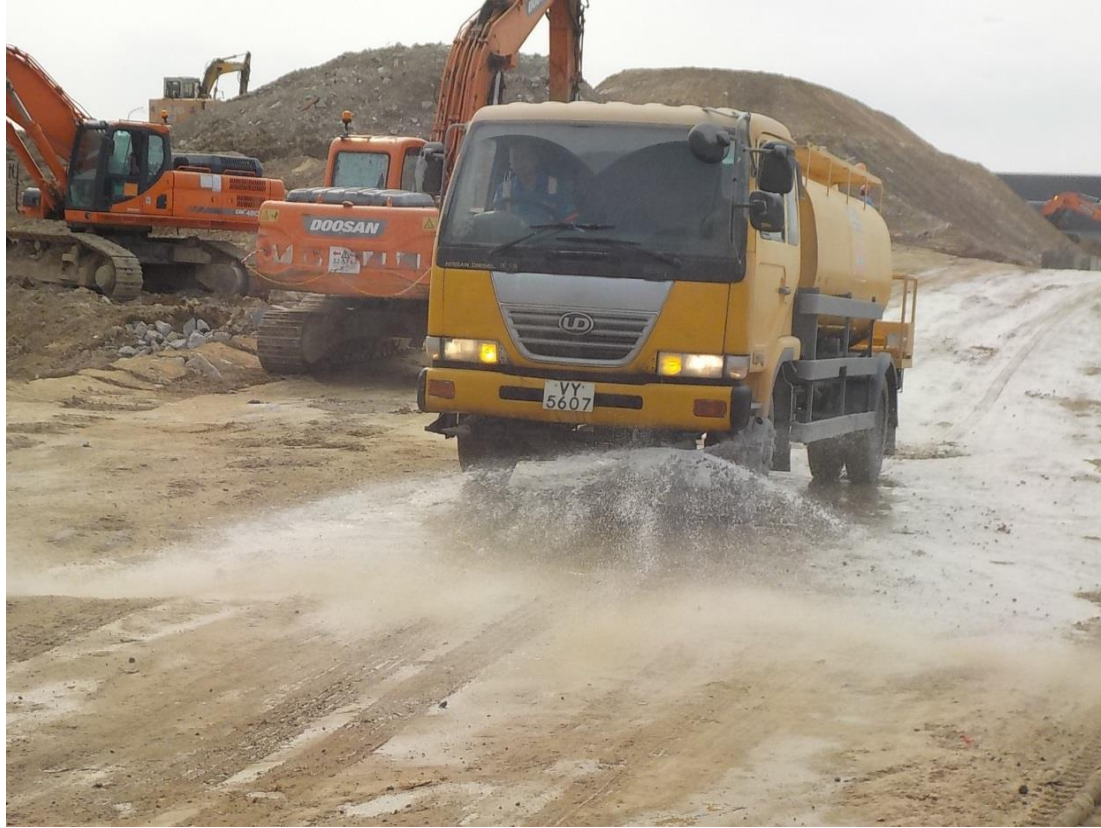
Water truck was used for water spraying on site.
