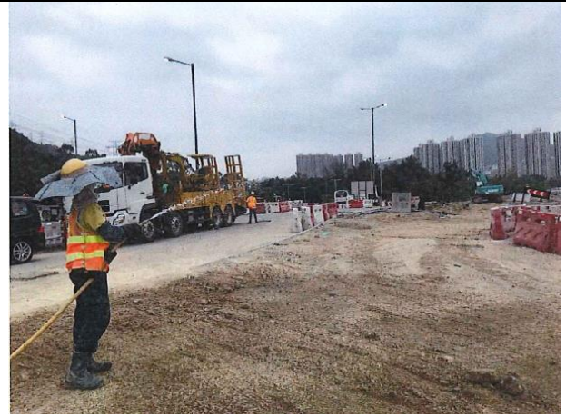
Photo 2 Water spraying by worker for un-accessible area.
