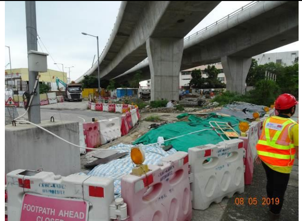
Photo 4 Covered stockpile by tarpaulin sheet.
