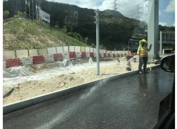
Photo 2 Water spraying by worker for un-accessible area.
