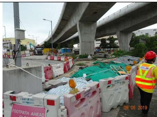
Photo 8 During the joint site inspection on 8 May 2019 stockpile storage on site was covered with tarpaulin.
