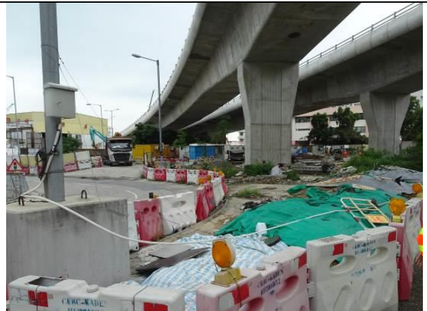
Photo 4 Covered stockpile by tarpaulin sheet.
