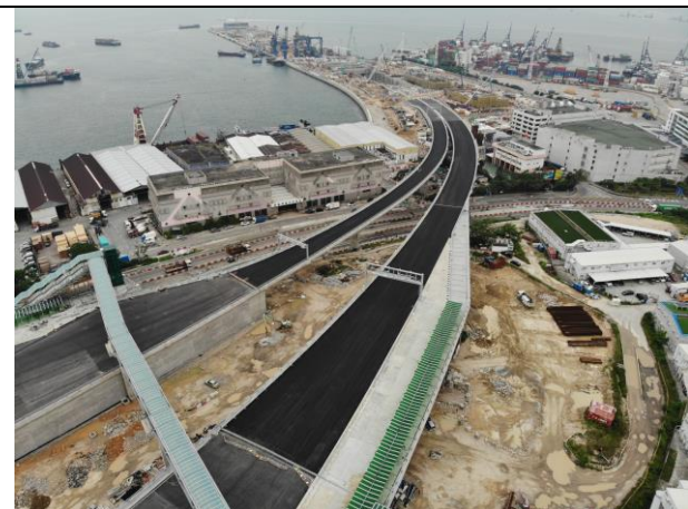
Photo 12 All of the site area at Portion F were hard paved
