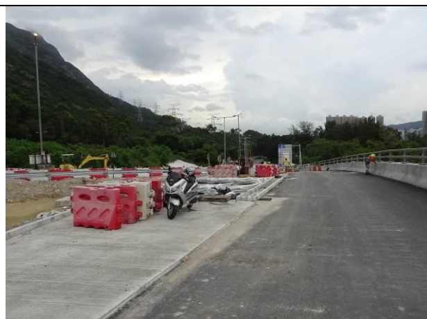
Photo 12 Installation of direction sign at Portion H
