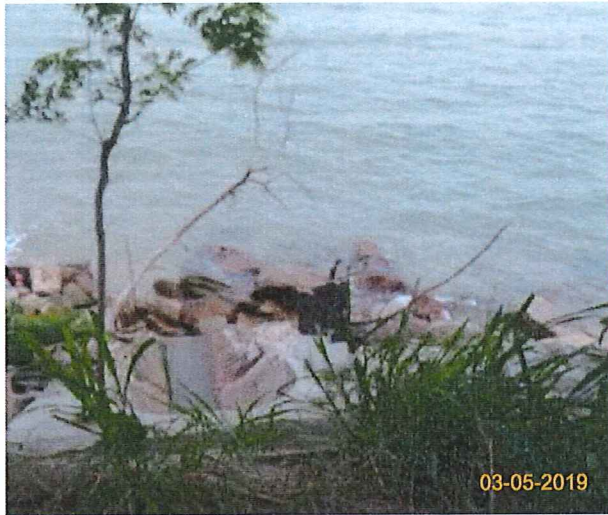
Item 7. Ensure no run-off into water body.(Outfall 1)
