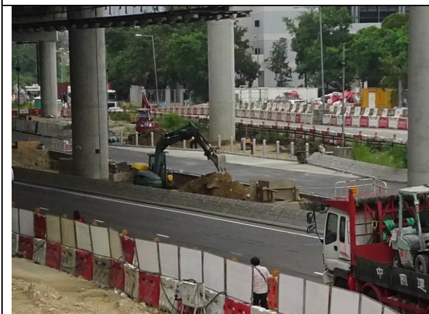
Photo 11 Construction of planter at Lung Mun Road
