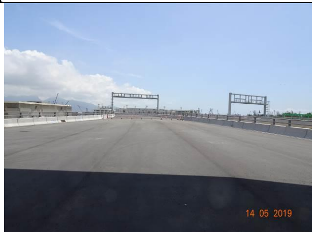
Photo 9 During the joint site inspection on 14 May 2019 most of the site area was hard paved.
