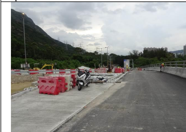
Photo 11 Installation of direction sign at Portion H
