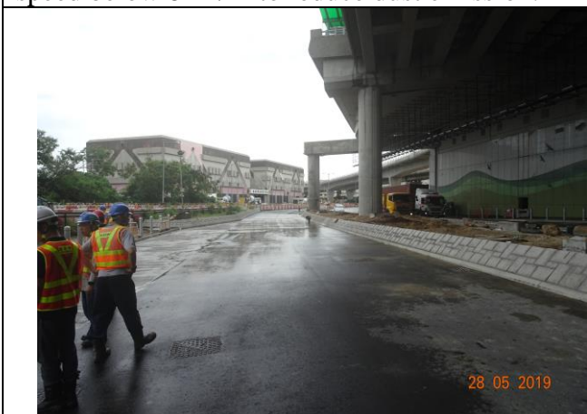
Photo 9 During the joint site inspection on 28 May 2019 works area was keeping wet to reduce dust impact.
