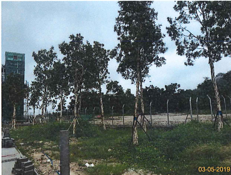
Item 2. Tree Transplanting works conducted on 22-May-17.
