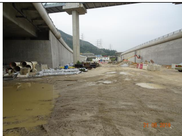
Photo 8 During the joint site inspection on 21 May 2019 haul road was keeping wet to reduce dust impact.
