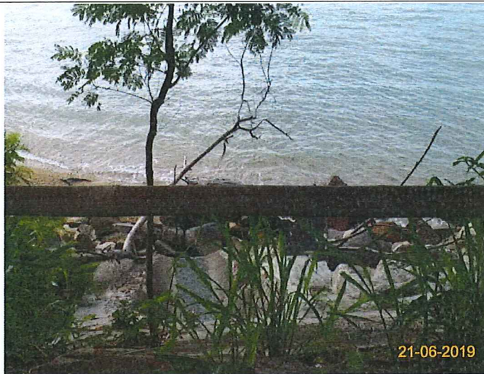
Item 7. Ensure no run-off into water body.(Outfall 1)
