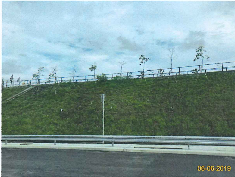
Item 3. Landscape works was commenced.
