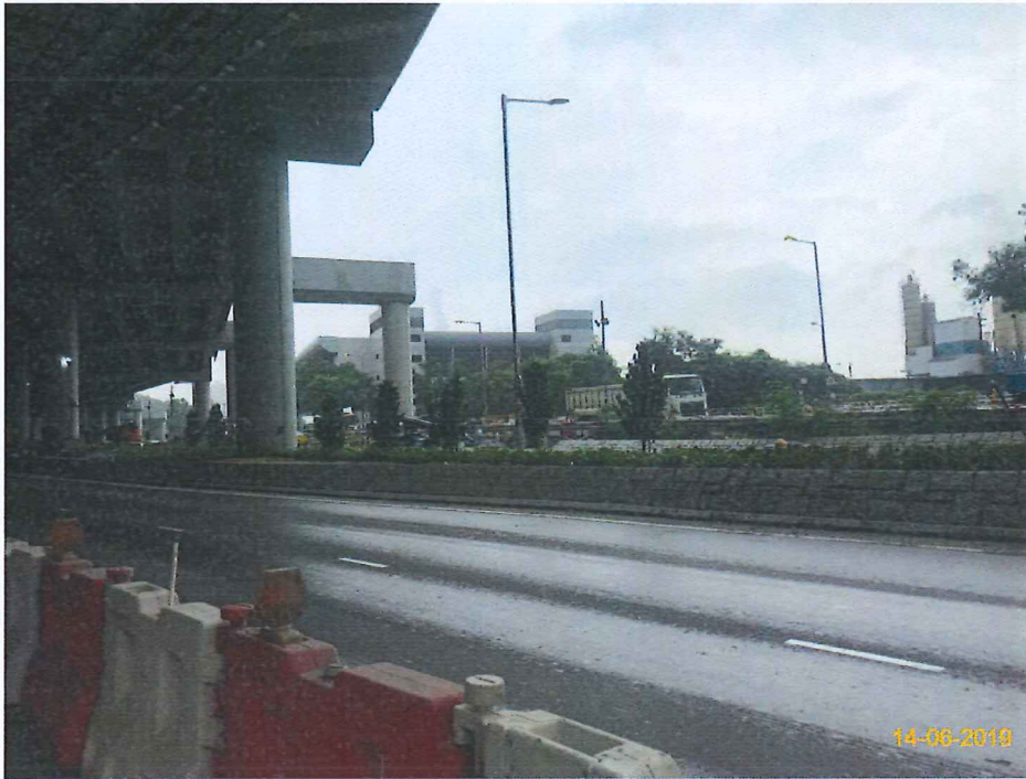
Item 3. Landscape works was commenced.
