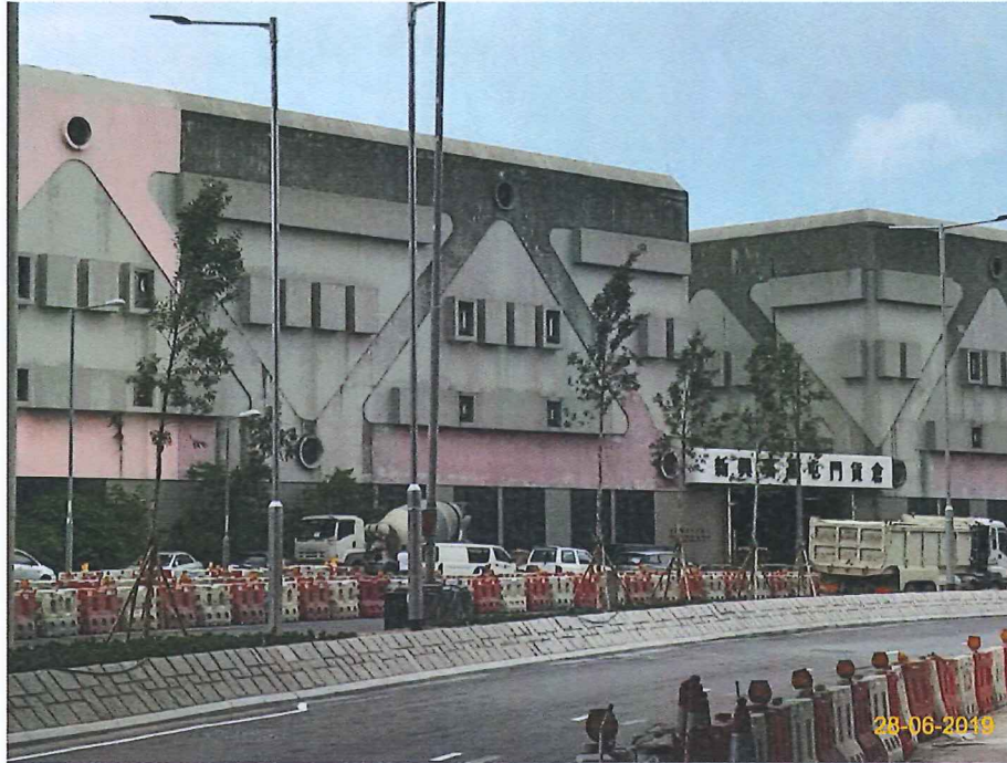
Item 3. Landscape works was commenced.
