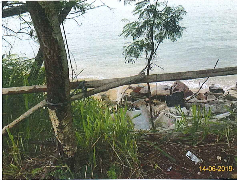
Item 7. Ensure no run-off into water body.(Outfall 1)
