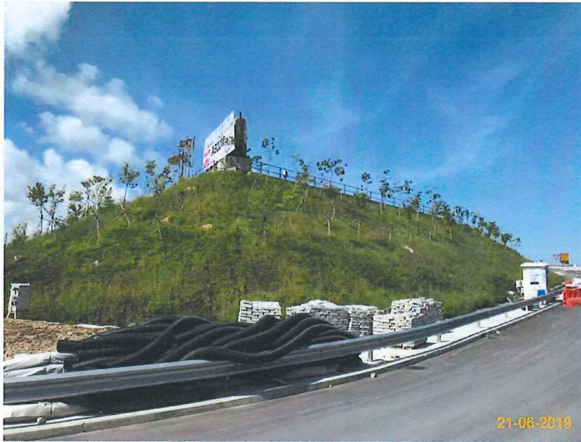
Item 3. Landscape works was commenced.
