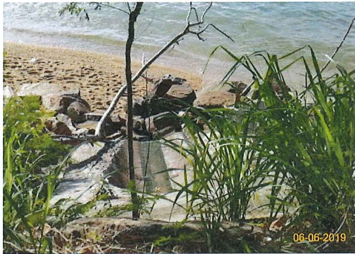
Item 7. Ensure no run-off into water body.(Outfall 1)
