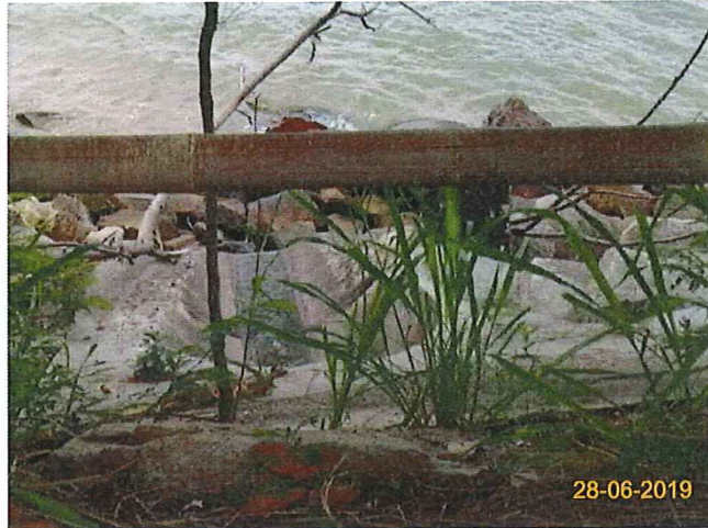
Item 7. Ensure no run-off into water body.(Outfall 1)
