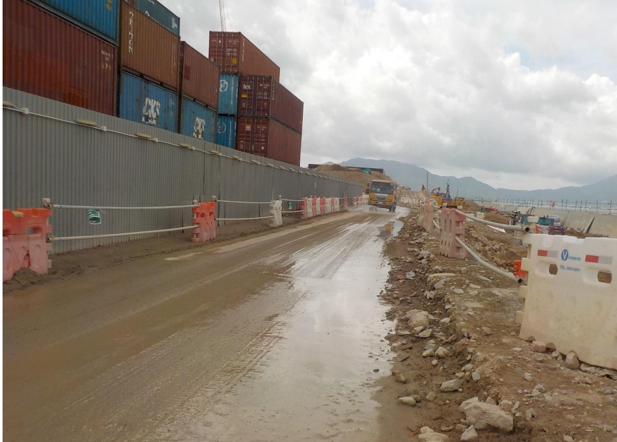
Water truck was used for water spraying to prevent dust. (Works Area Portion N-C)
