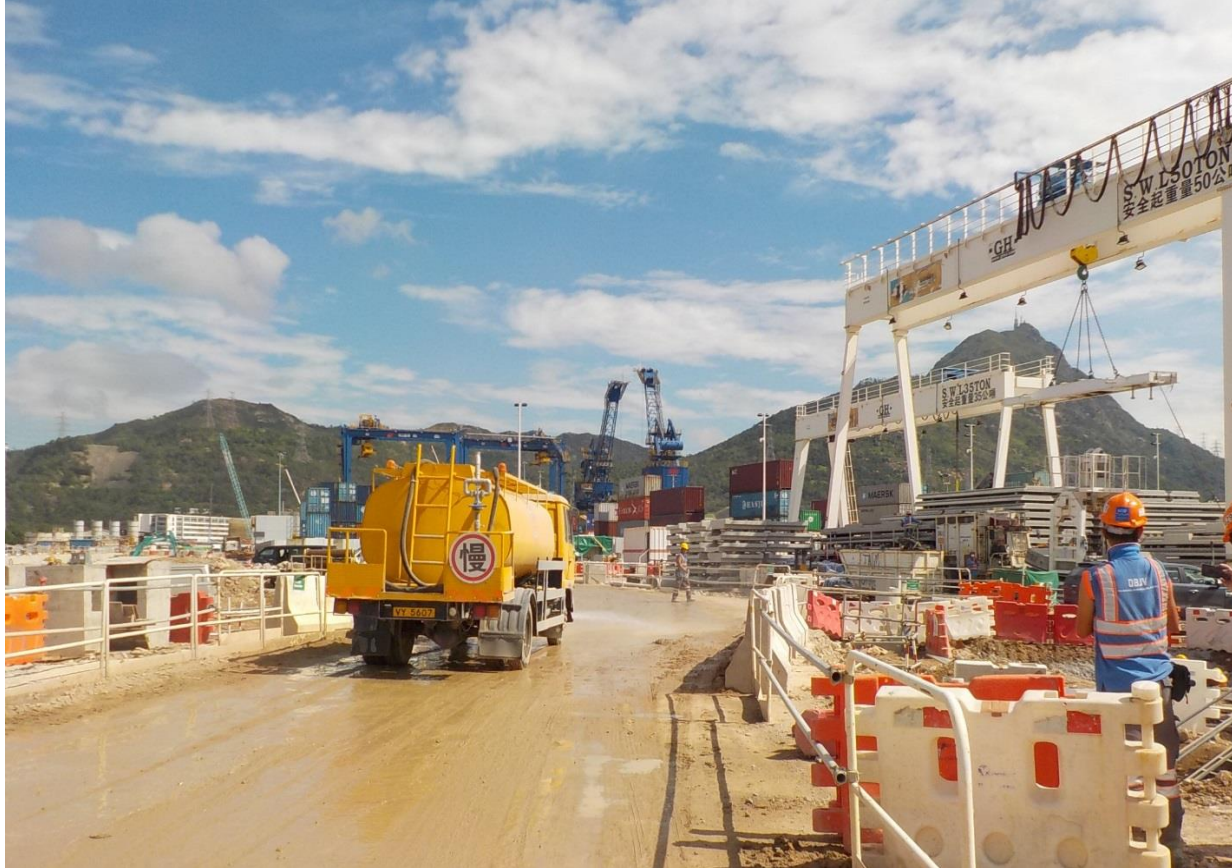
Water truck was used for water spraying to prevent dust. (Works Area Portion N-A)
