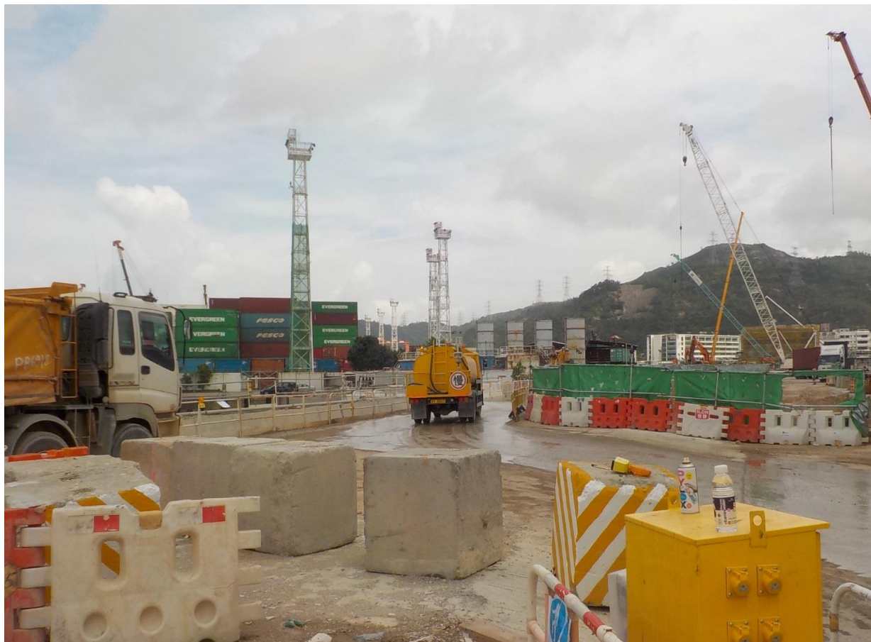
Water truck was used for water spraying to prevent dust. (Works Area Portion N-A)
