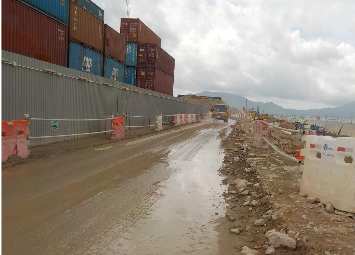
Water truck was used for water spraying to prevent dust. (Works Area Portion N-C)
