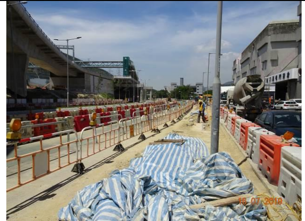
Photo 4 Covered stockpile by tarpaulin sheet.
