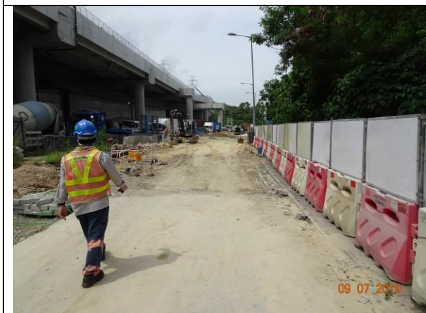
Photo 11 Drainage works at Lung Mun Road
