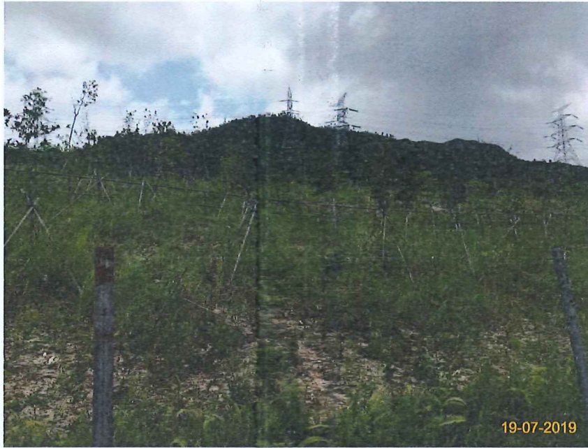
Item 3. Landscape works was commenced.
