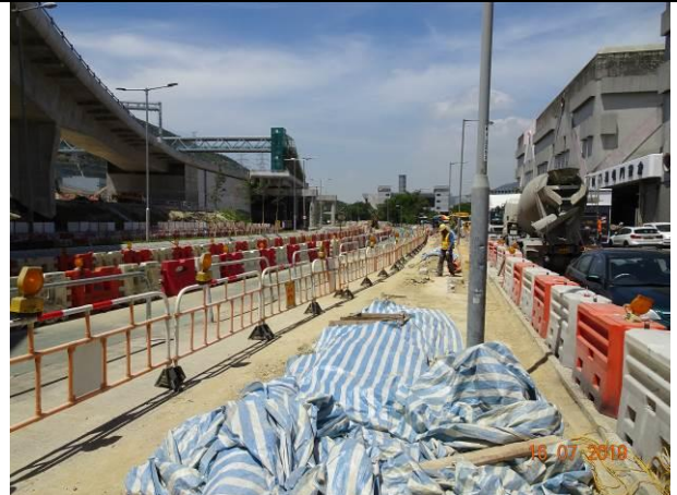
Photo 2 Covered stockpile by tarpaulin sheet.
