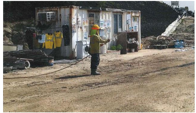
Photo 2 Water spraying by worker for un-accessible area.
