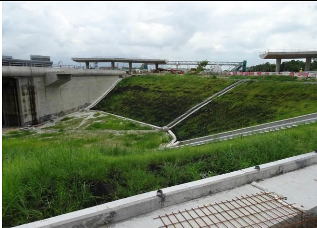
Photo 1 Hydro seeding for the exposed slope at Retaining Wall B.
