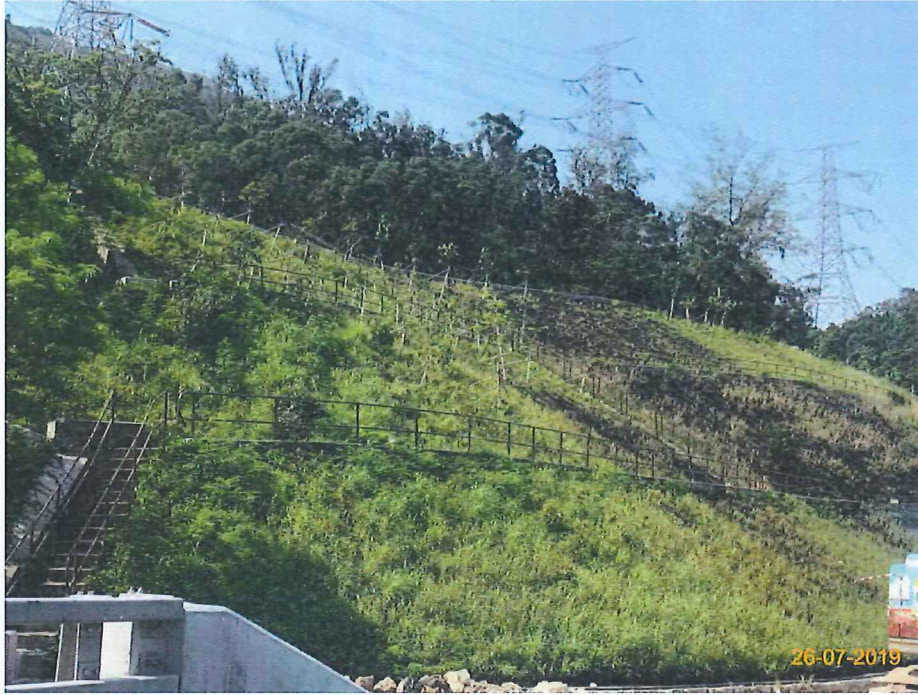
Item 3. Landscape works was commenced.
