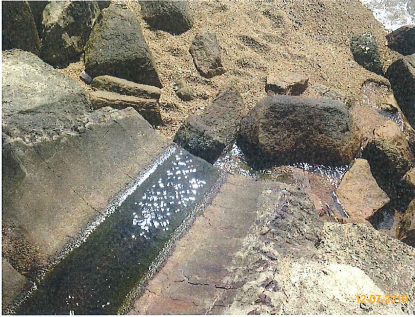
Item 7. Ensure no run-off into water body.(Outfall 1)
