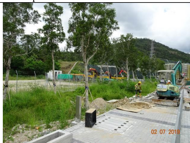
Photo 12 Landscape works at +19 Platform
