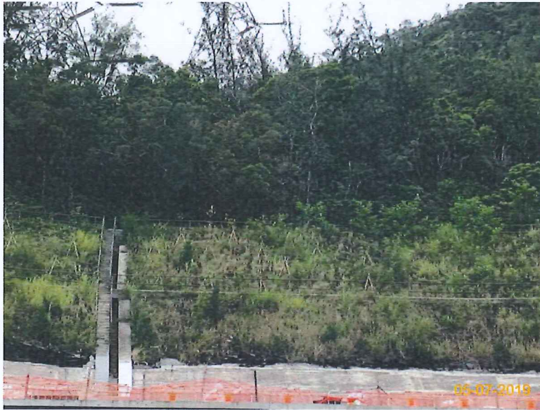
Item 3. Landscape works was commenced.
