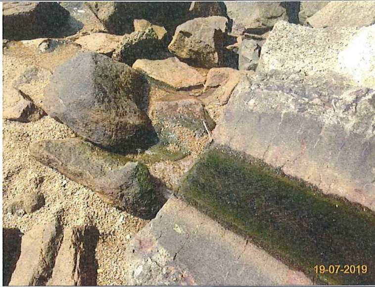
Item 7. Ensure no run-off into water body.(Outfall 1)
