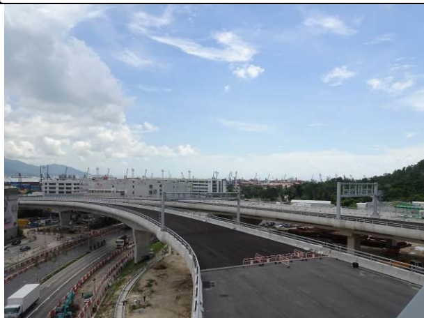
Photo 9 During the joint site inspection on 9 July 2019 most of the site area was hard paved.
