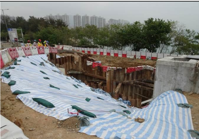
Photo 3 Covered part of the exposed slopes and stockpile by tarpaulin sheet.
