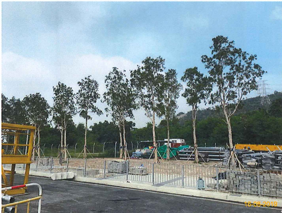
Item 2. Tree Transplanting works conducted on 22-May-17.
