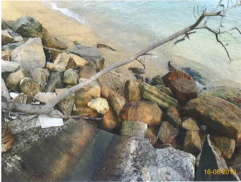
Item 7. Ensure no run-off into water body.(Outfall 1)
