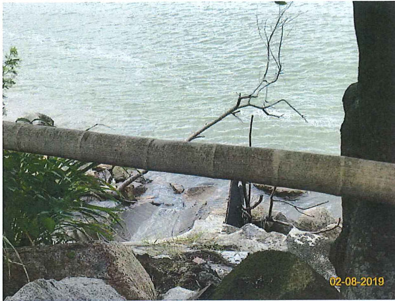
Item 7. Ensure no run-off into water body.(Outfall 1)
