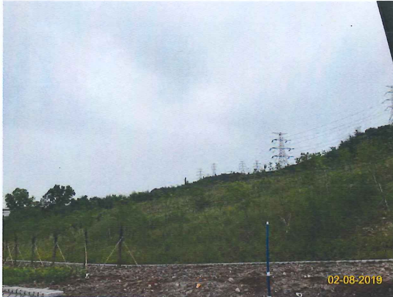
Item 3. Landscape works was commenced.
