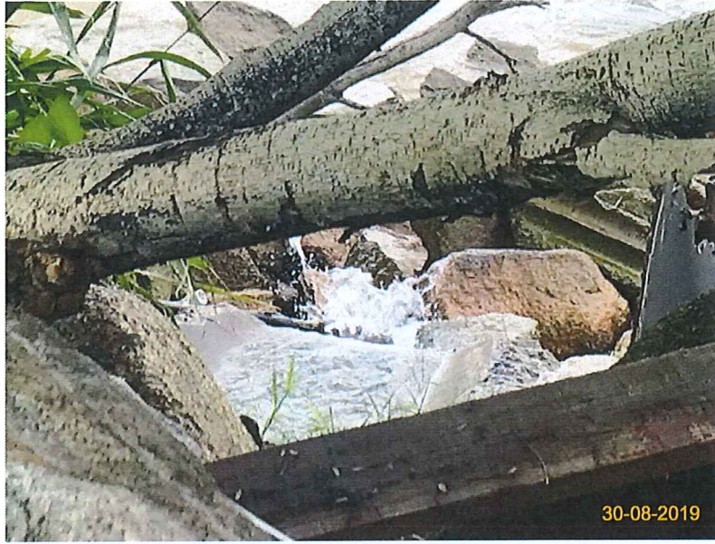
Item 7. Ensure no run-off into water body.(Outfall 1)
