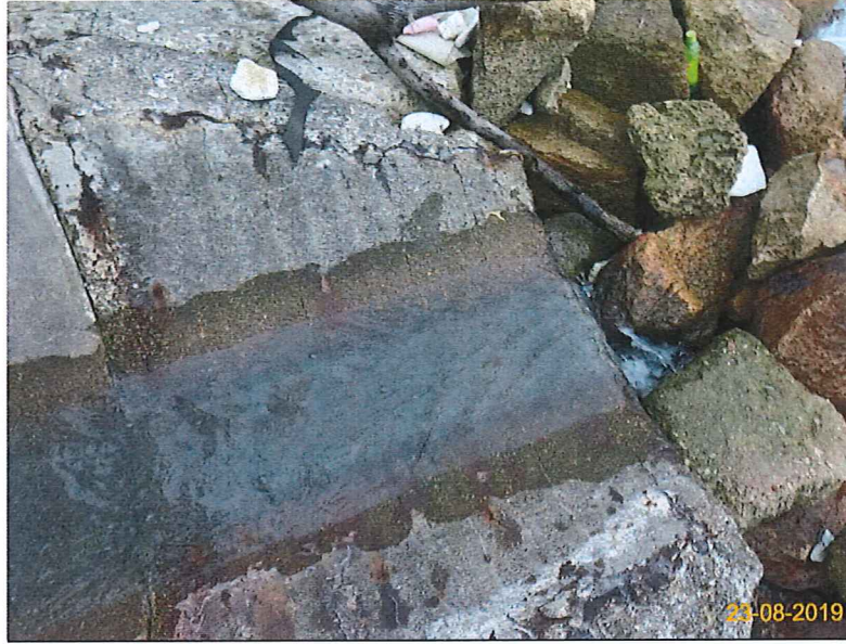
Item 7. Ensure no run-off into water body.(Outfall 1)
