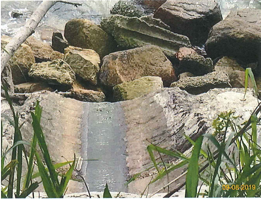
Item 7. Ensure no run-off into water body.(Outfall 1)
