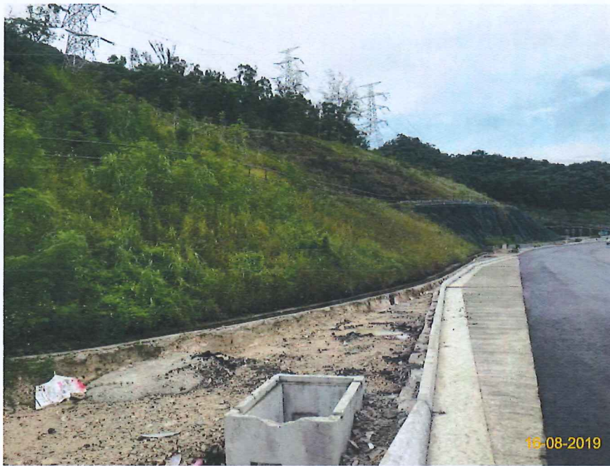
Item 3. Landscape works was commenced.
