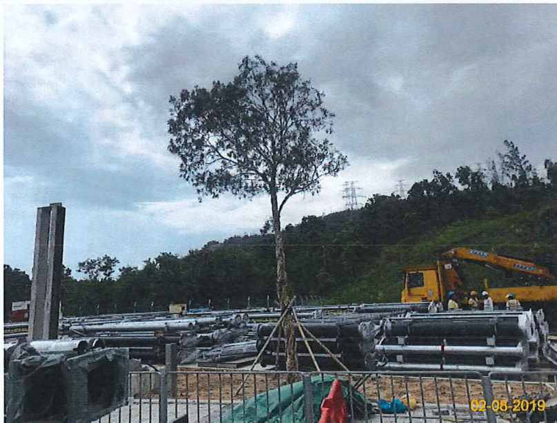
Item 2. Tree Transplanting works conducted on 22-May-17.
