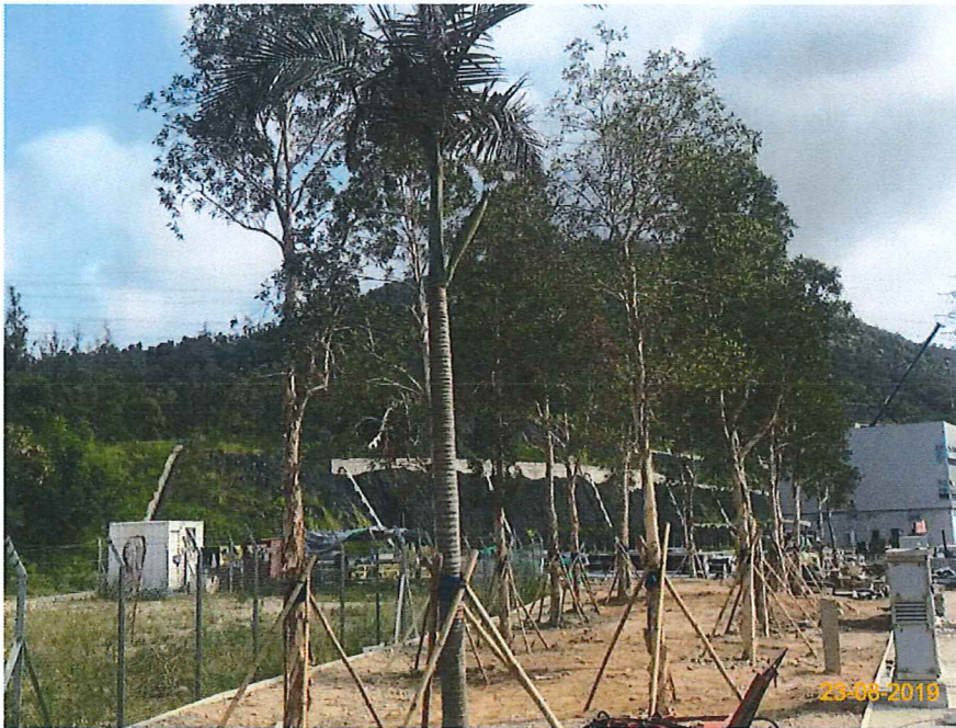
Item 2. Tree Transplanting works was conducted on 22-May-17.
