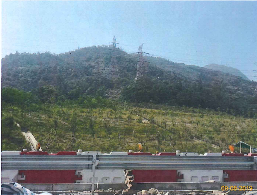
Item 3. Landscape works was commenced.
