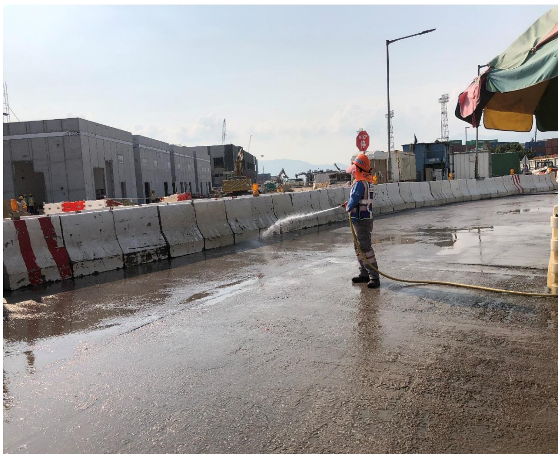
Water spraying was applied on main haul road to prevent dust. (Works Area Portion N-A)
