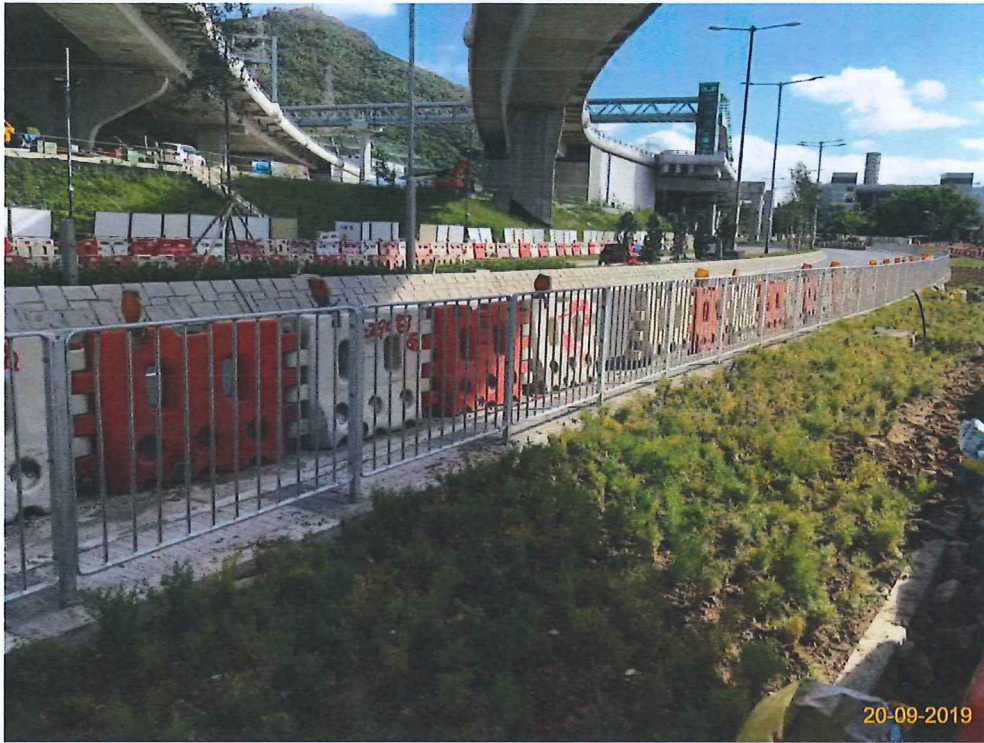
Item 3. Landscape works was commenced.
