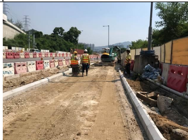
Photo 12 Roadside kerb work at Lung Mun Road
