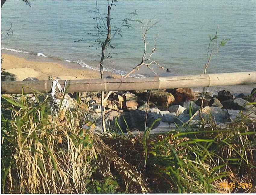
Item 7. Ensure no run-off into water body.(Outfall 1)
