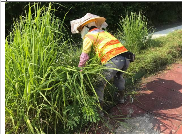
Photo 11 Weeding works at Portion H
