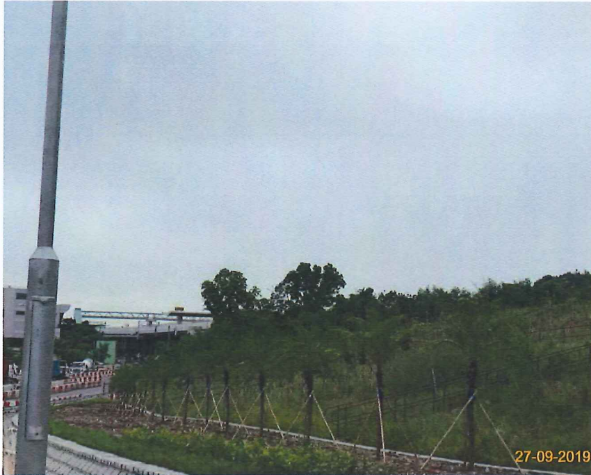
Item 3. Landscape works was commenced.
