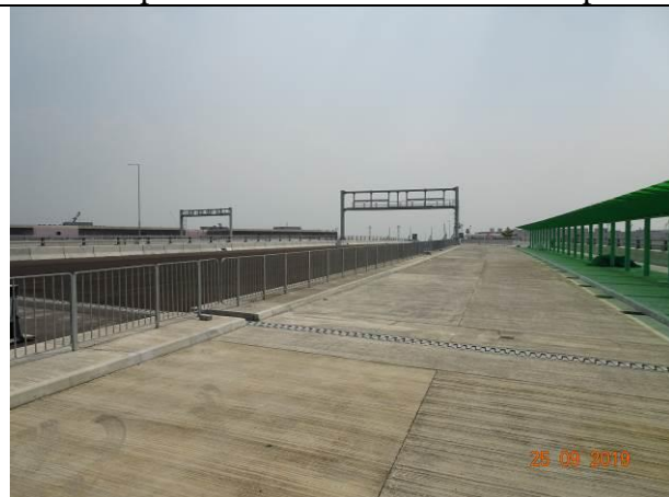
Photo 10 During the joint site inspection on 25 September 2019 most of the site area was hard paved.
