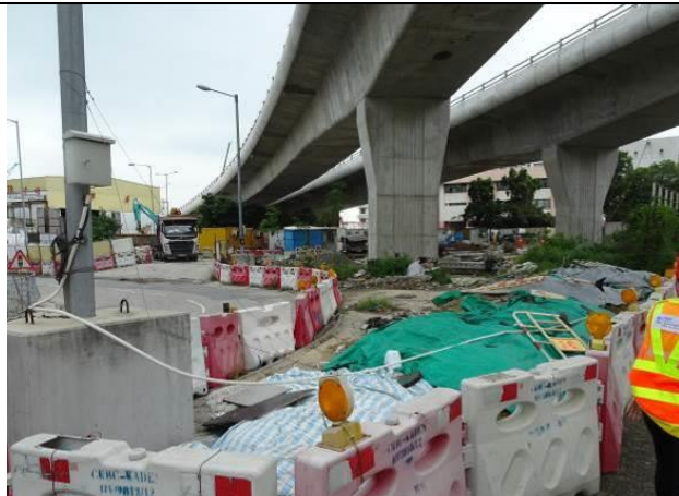
Photo 4 Covered stockpile by tarpaulin sheet.
