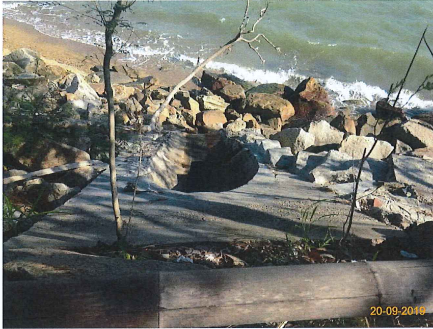
Item 7. Ensure no run-off into water body.(Outfall 1)
