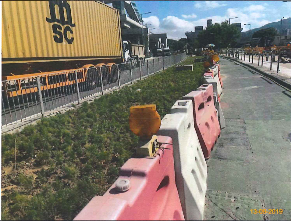
Item 3. Landscape works was commenced.
