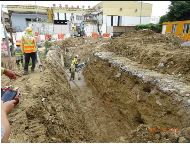
Photo 13 Sewerage works at Ho Yeung Street
