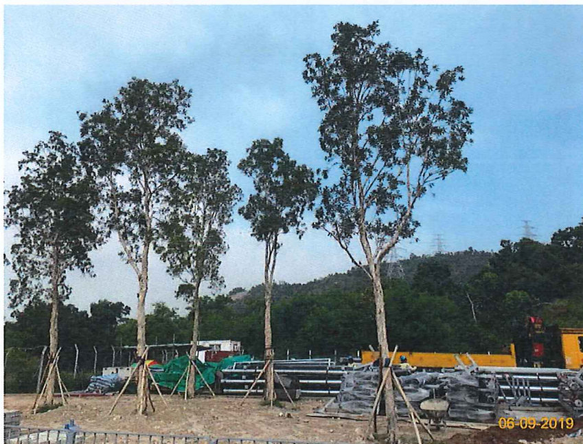
Item 2. Tree Transplanting works conducted on 22-May-17.
