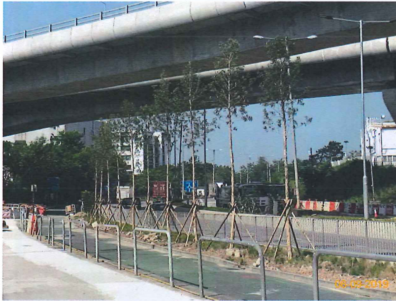
Item 3. Landscape works was commenced.
