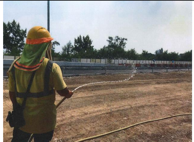
Photo 2 Water spraying by worker for un-accessible area.
