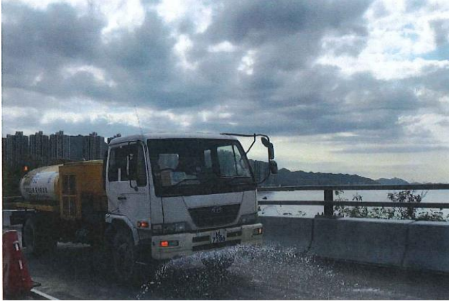
Photo 1 Watering of haul road by water truck to keep road surface wet
