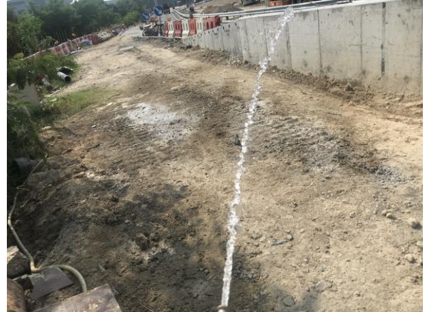
Photo 2 Water spraying by worker for un-accessible area.
