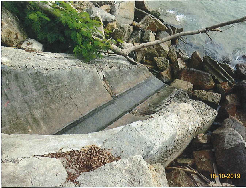
Item 7. Ensure no run-off into water body.(Outfall 1)
