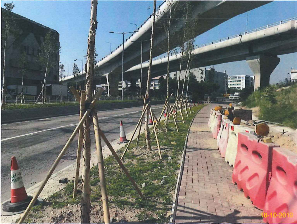
Item 3. Landscape works was commenced.
