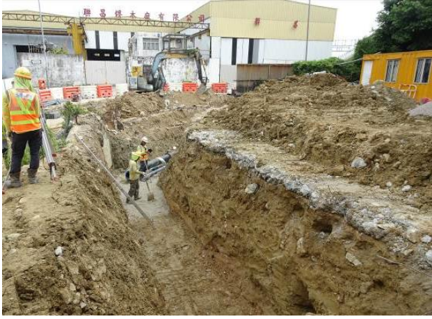
Photo 13 Sewerage works at Ho Yeung Street
