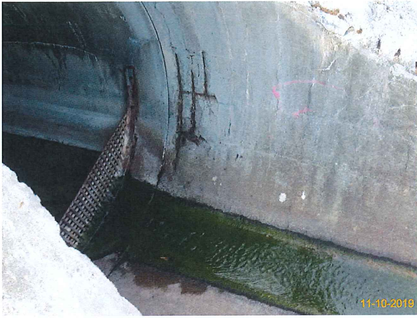
Item 7. Ensure no run-off into water body.(Outfall 1)
