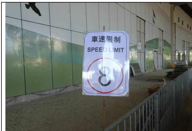
Photo 7 All vehicles passing through the haul road at Lung Mun Road has enhanced to control the speed below 8km/hr to reduce dust emission.
