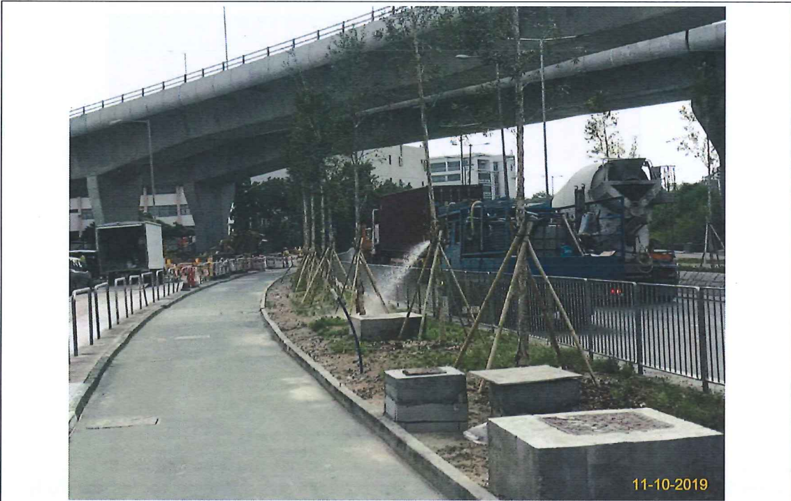
Item 3. Landscape works was commenced.
