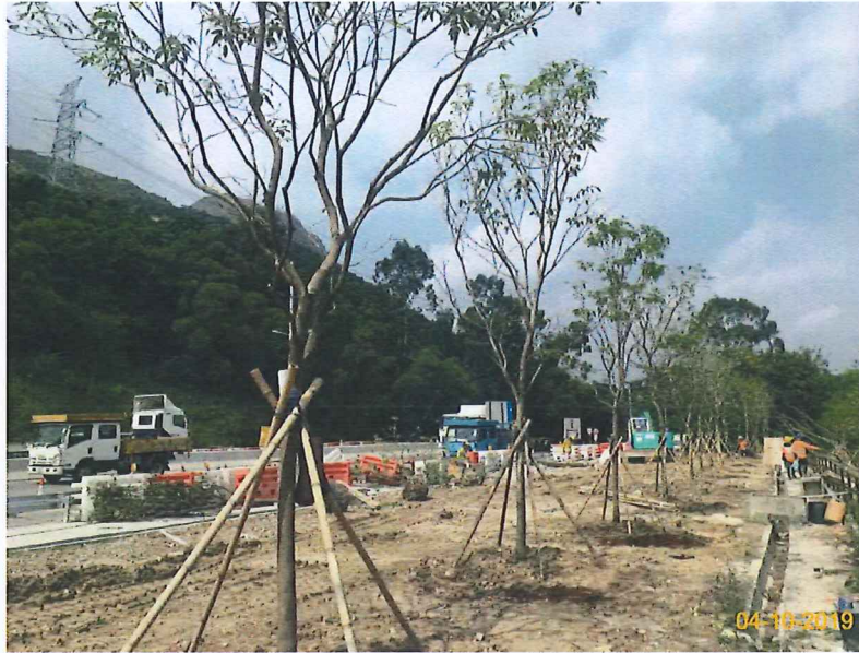
Item 3. Landscape works was commenced.
