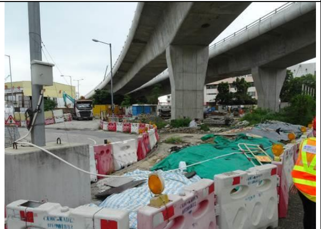
Photo 4 Covered stockpile by tarpaulin sheet.
