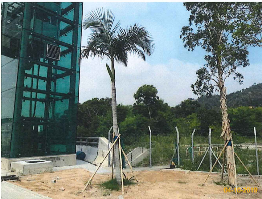
Item 2. Tree Transplanting works conducted on 22-May-17.
