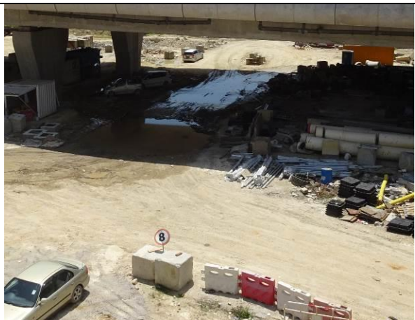
Photo 6 All vehicles using the haul road had enhanced to control the speed below 8km/hr to reduce dust emission.
