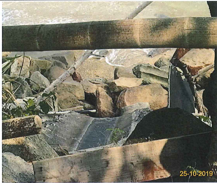
Item 7. Ensure no run-off into water body.(Outfall 1)
