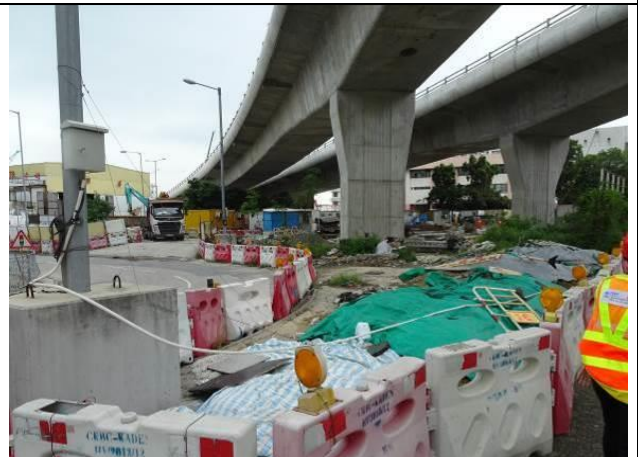
Photo 4 Covered stockpile by tarpaulin sheet.
