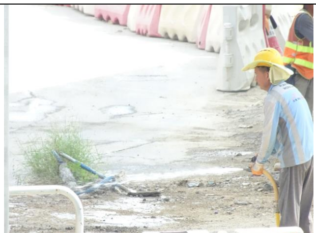
Photo 8 During the joint site inspection on 15 October 2019 water spraying was provided for the exposed surface to reduce dust impact.
