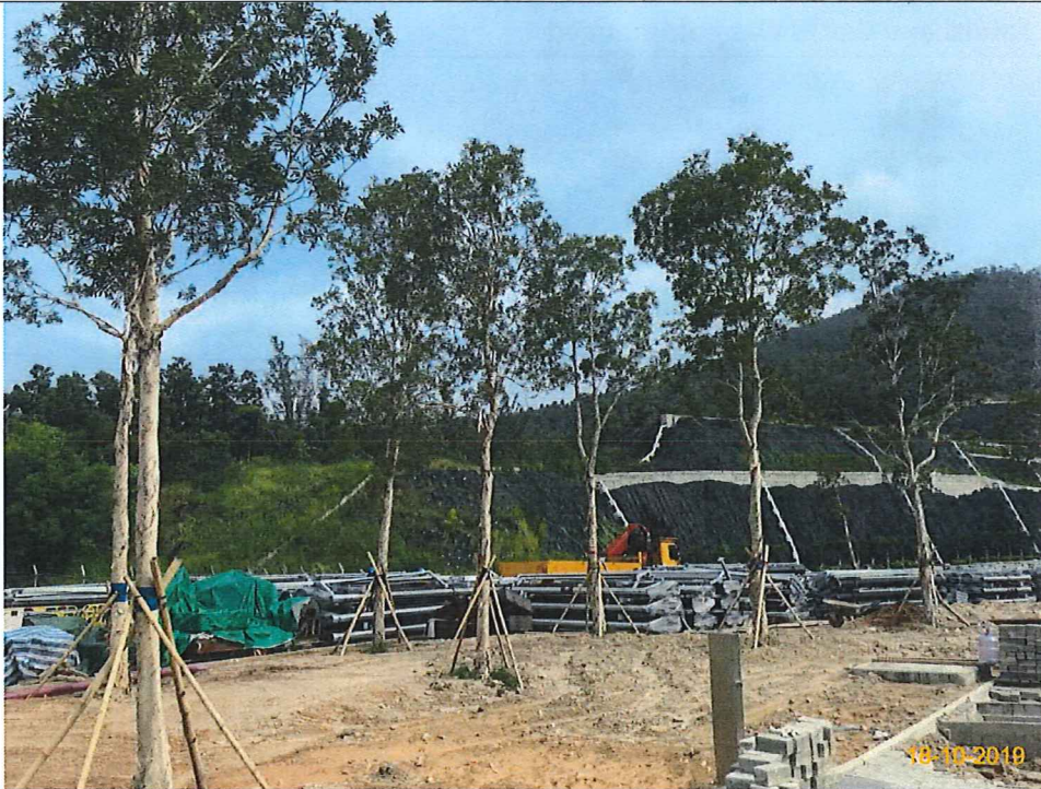
Item 2. Tree Transplanting works conducted on 22-May-17.
