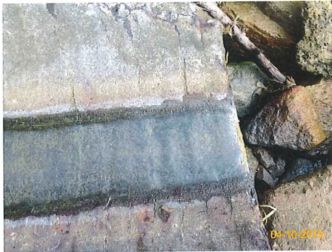
Item 7. Ensure no run-off into water body.(Outfall 1)
