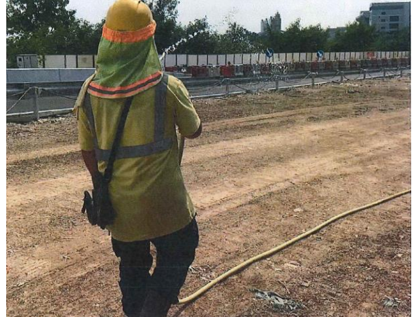
Photo 2 Water spraying by worker for un-accessible area.
