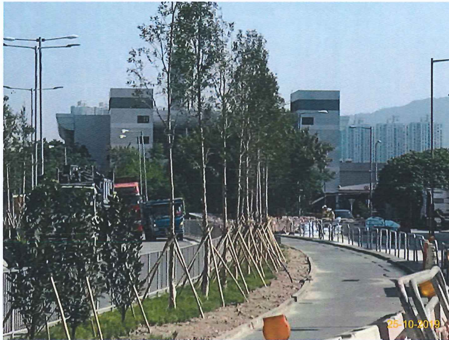
Item 3. Landscape works was commenced.
