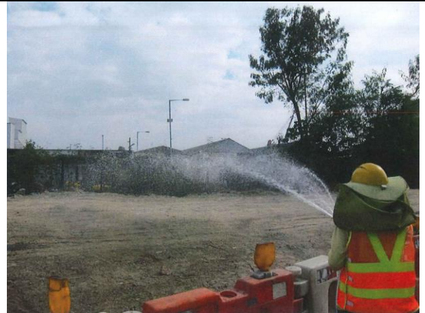
Photo 2 Water spraying by worker for un-accessible area.
