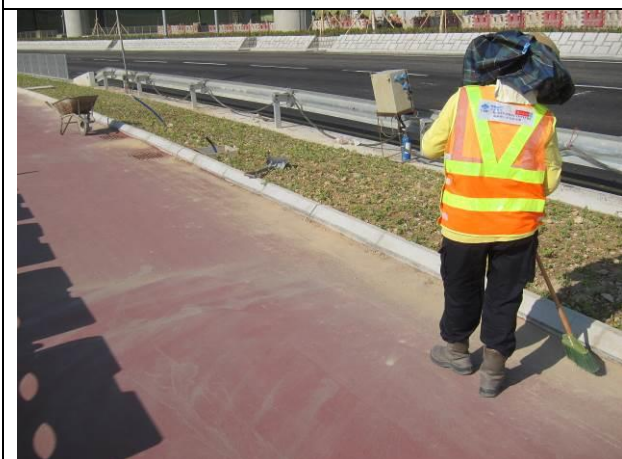
Photo 11 Housekeeping works at Lung Mun Road
