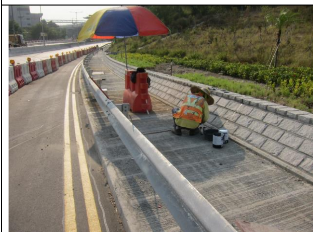
Photo 11 Housekeeping works at Lung Mun Road
