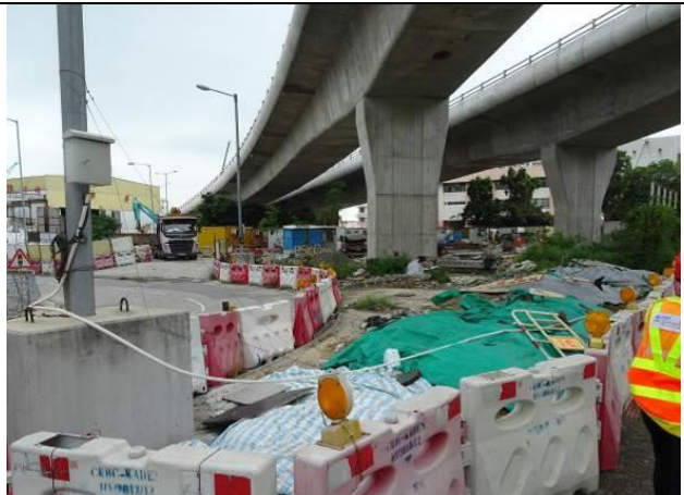
Photo 4 Covered stockpile by tarpaulin sheet.
