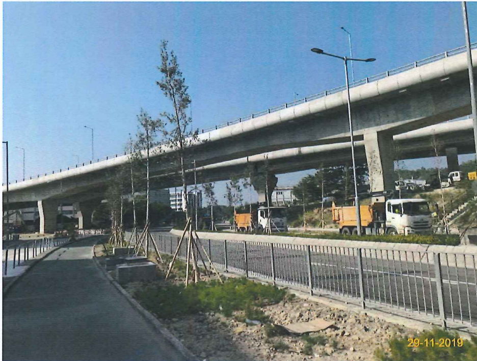
Item 3. Landscape works was commenced.
