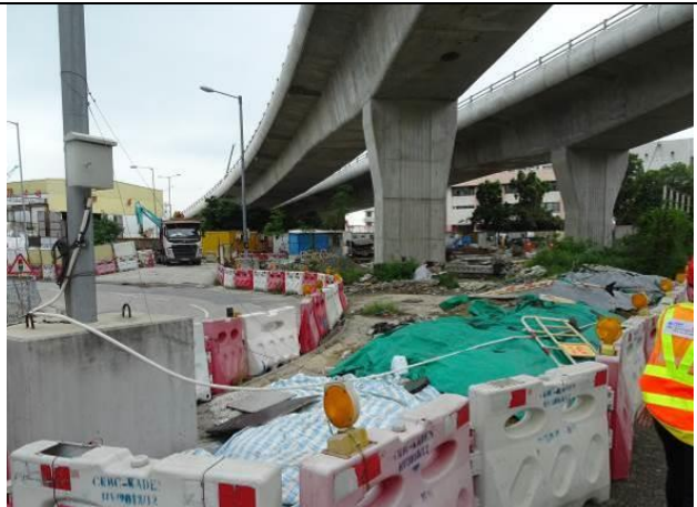
Photo 4 Covered stockpile by tarpaulin sheet.
