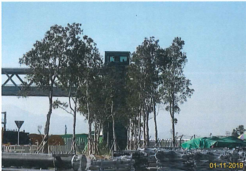
Item 2. Tree Transplanting works conducted on 22-May-17.
