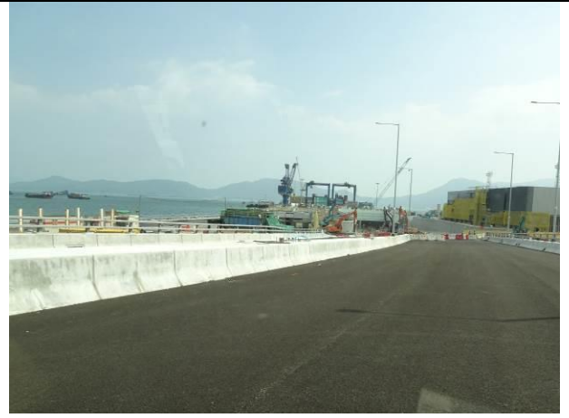
Photo 14 All of the site area at Portion F were hard paved
