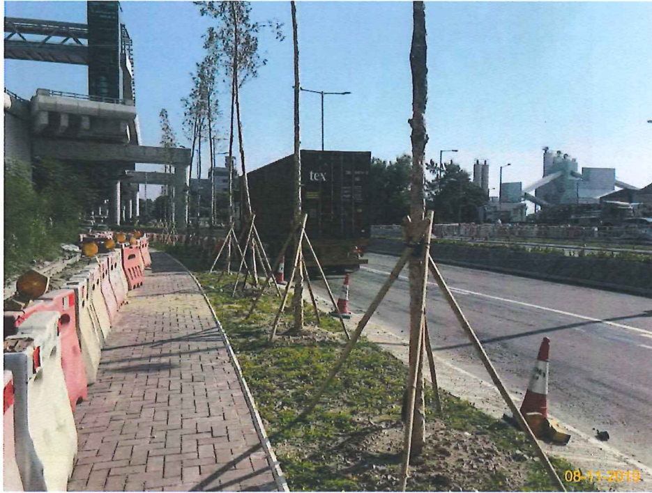
Item 3. Landscape works was commenced.
