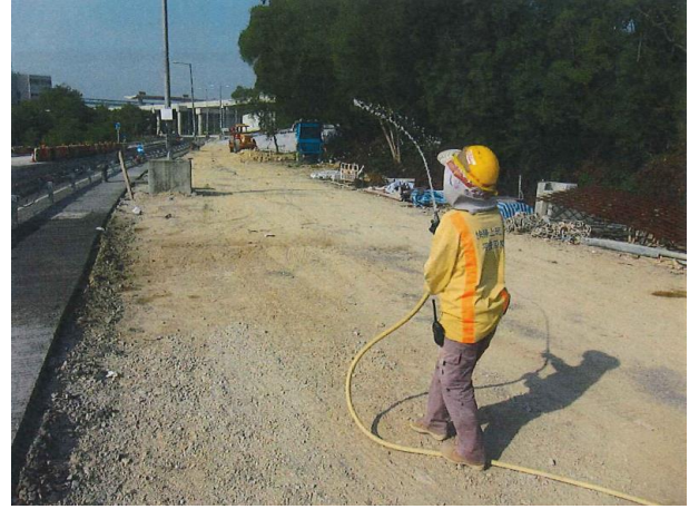
Photo 2 Water spraying by worker for un-accessible area.
