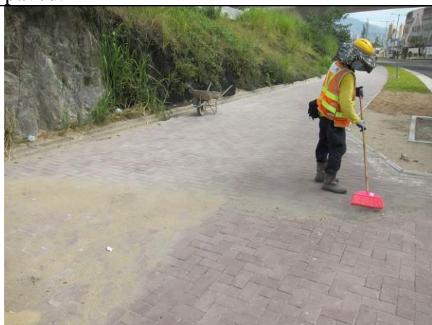
Photo 11 Remedial works at Lung Mun Road (Road paving)
