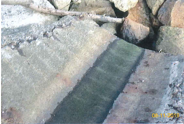
Item 7. Ensure no run-off into water body.(Outfall 1)
