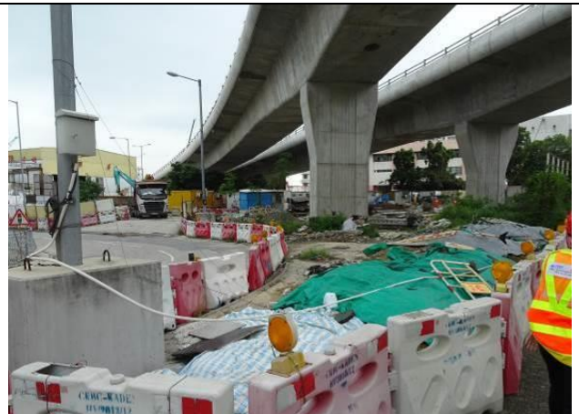
Photo 4 Covered stockpile by tarpaulin sheet.
