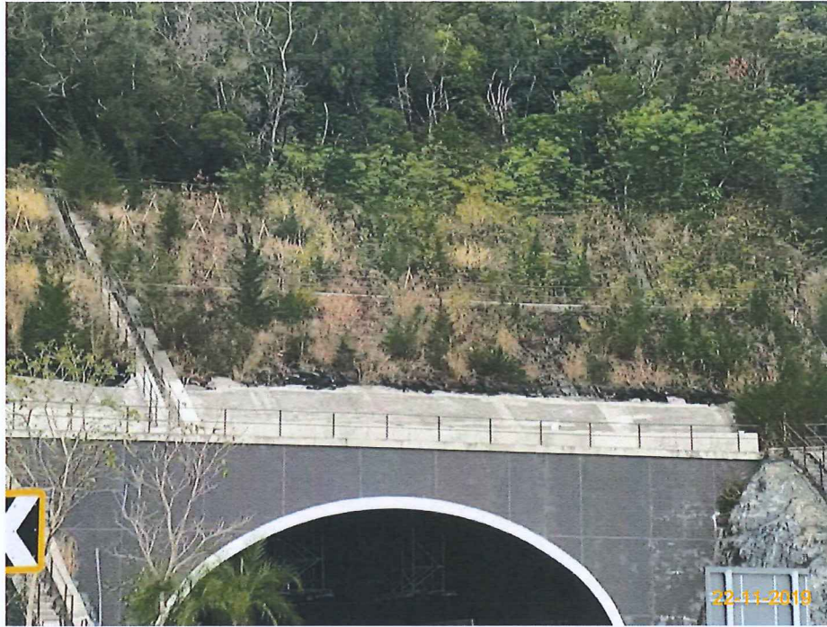
Item 3. Landscape works was commenced.
