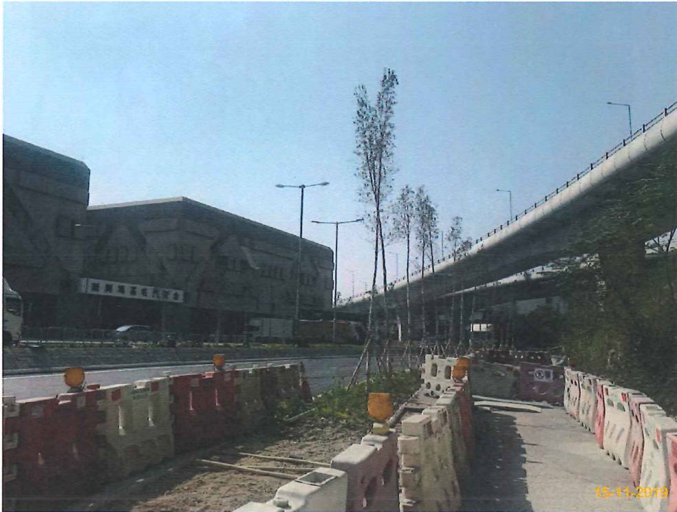
Item 3. Landscape works was commenced.
