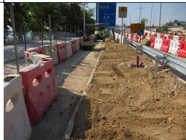
Photo 12 Construction of u-channel works at Portion H
