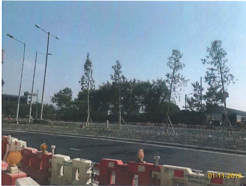
Item 3. Landscape works was commenced.
