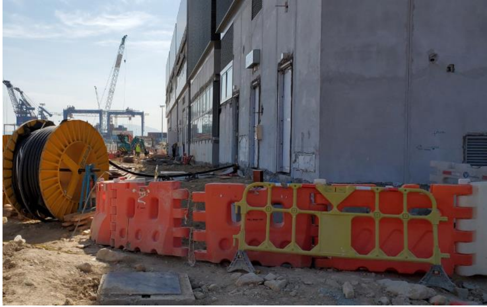
Photo 1 - Construction works at Administration Building
