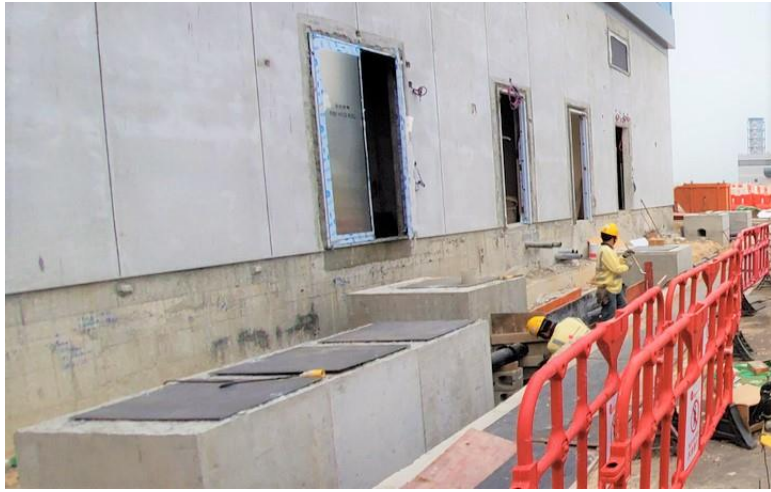
Photo 1 - Construction works at Toll Control Building
