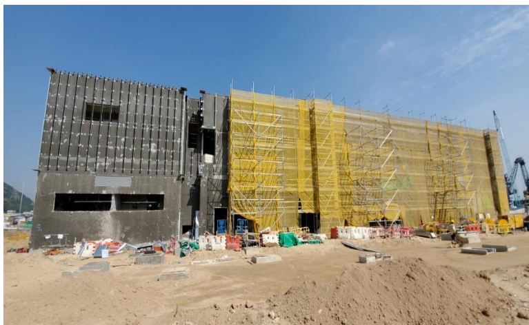
Photo 3 - Construction works at Administration Building
