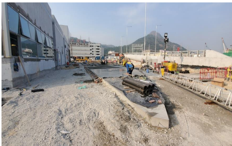
Photo 2 - Construction works at Maintenance Depot
