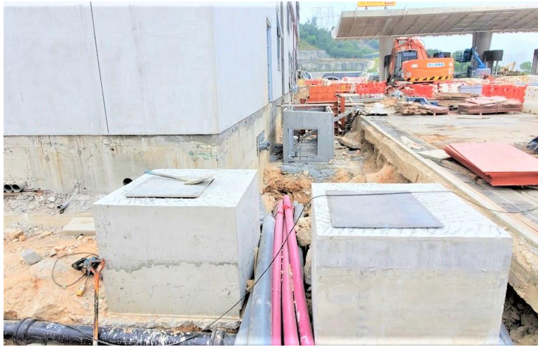
Photo 1 - Construction works at Toll Control Building
