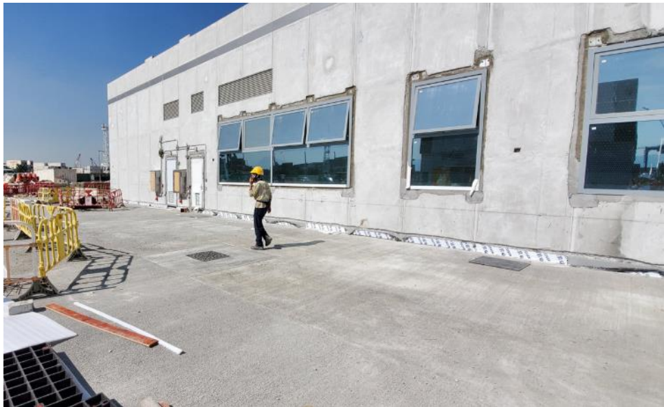
Photo 2 - Construction works at Maintenance Depot
