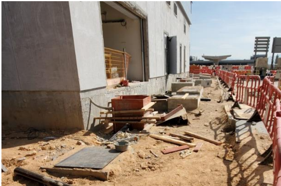
Photo 3 - Construction works at Toll Control Building
