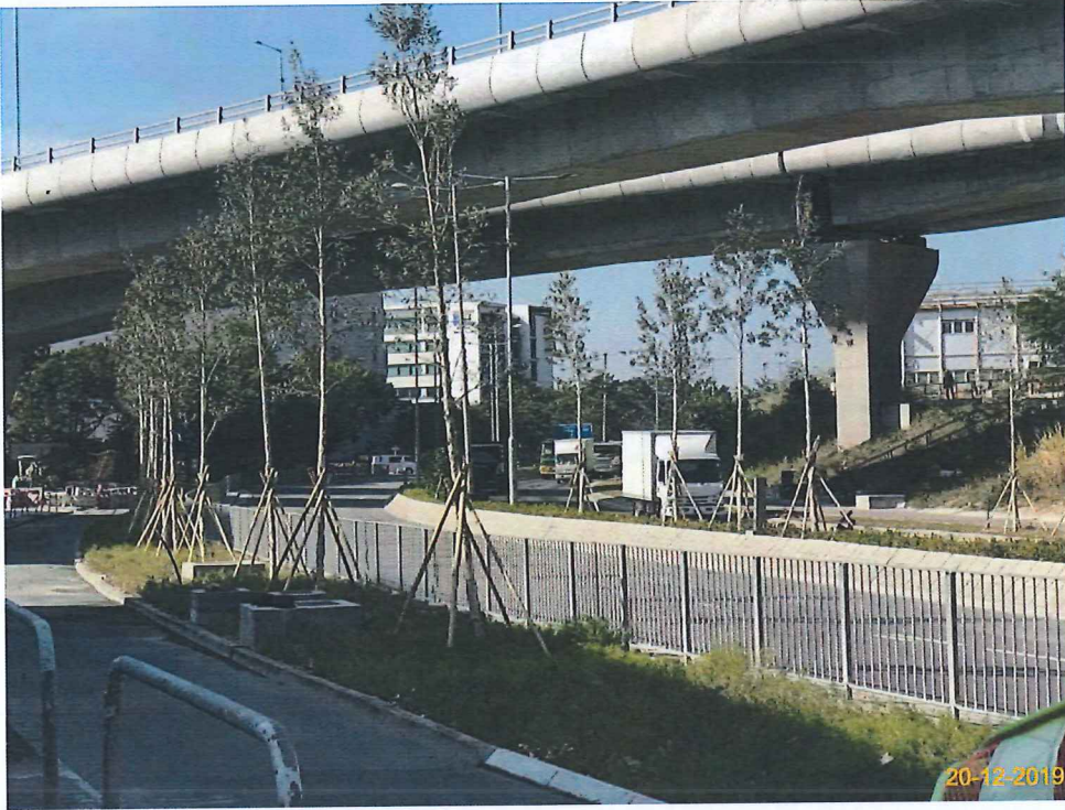
Item 3. Landscape works was commenced.
