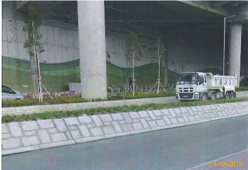
Item 3. Landscape works was commenced.
