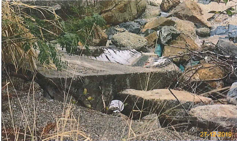
Item 7. Ensure no run-off into water body.(Outfall 1)
