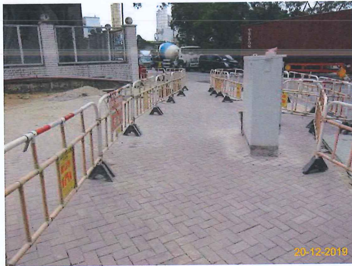
Item 6. Temporary traffic management lighting.
