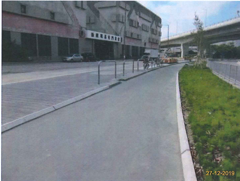
Item 3. Landscape works was commenced.
