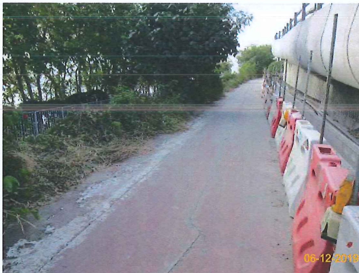
Item 6. Temporary traffic management lighting.
