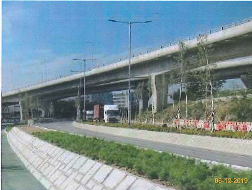
Item 3. Landscape works was commenced.
