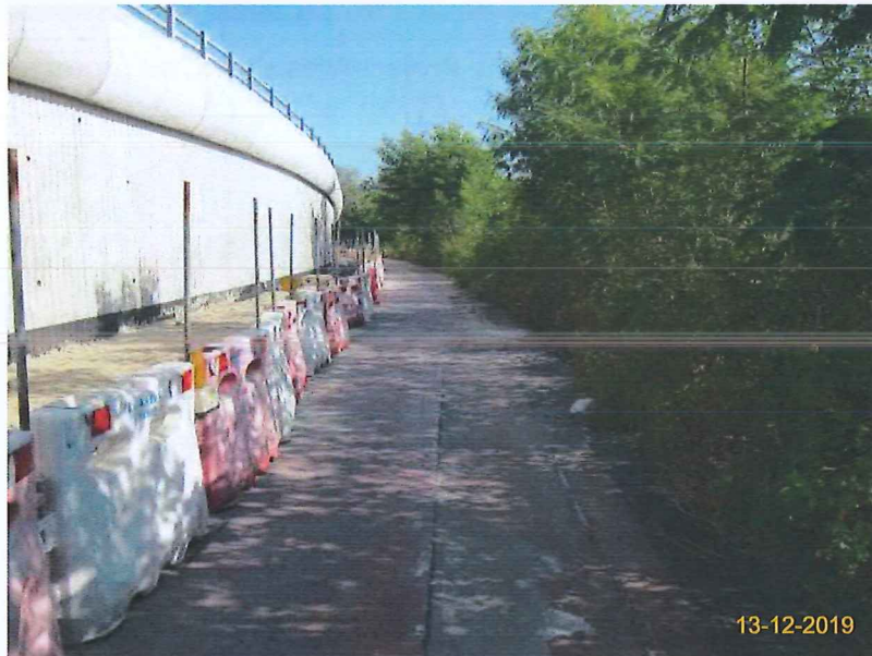
Item 6. Temporary traffic management lighting.
