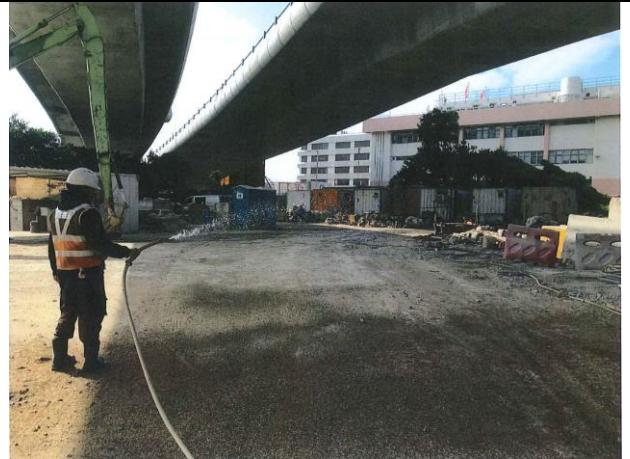
Photo 2 Water spraying by worker for un-accessible area.
