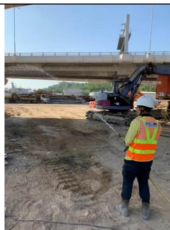
Photo 8 During the joint site inspection on 26 November 2019 water spraying had been provided for the exposed area to reduce dust impact.
