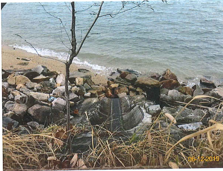
Item 7. Ensure no run-off into water body.(Outfall 1)
