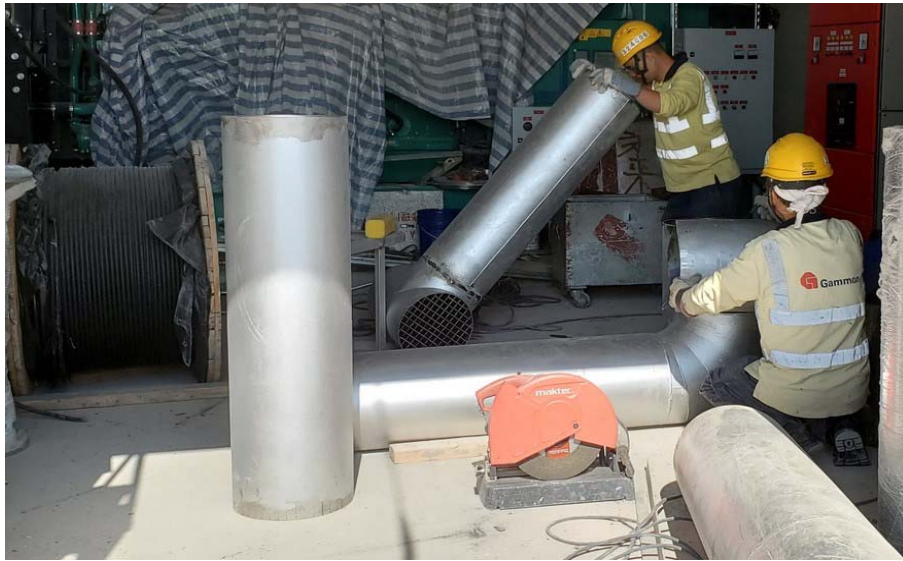
Photo 1 - Construction works at Administration Building
